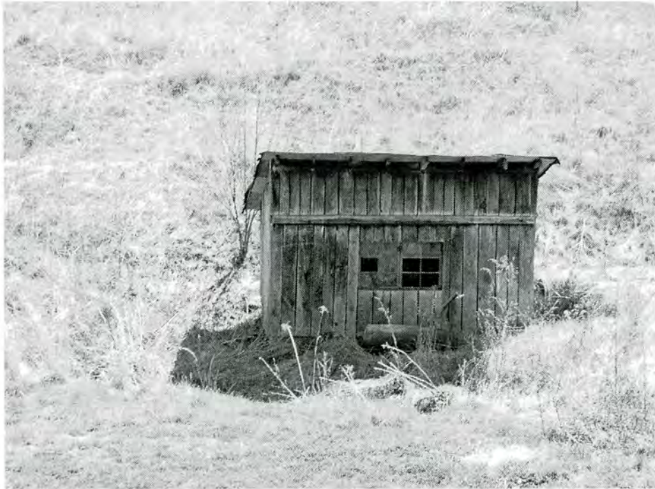
Springhouse, West Elevation
