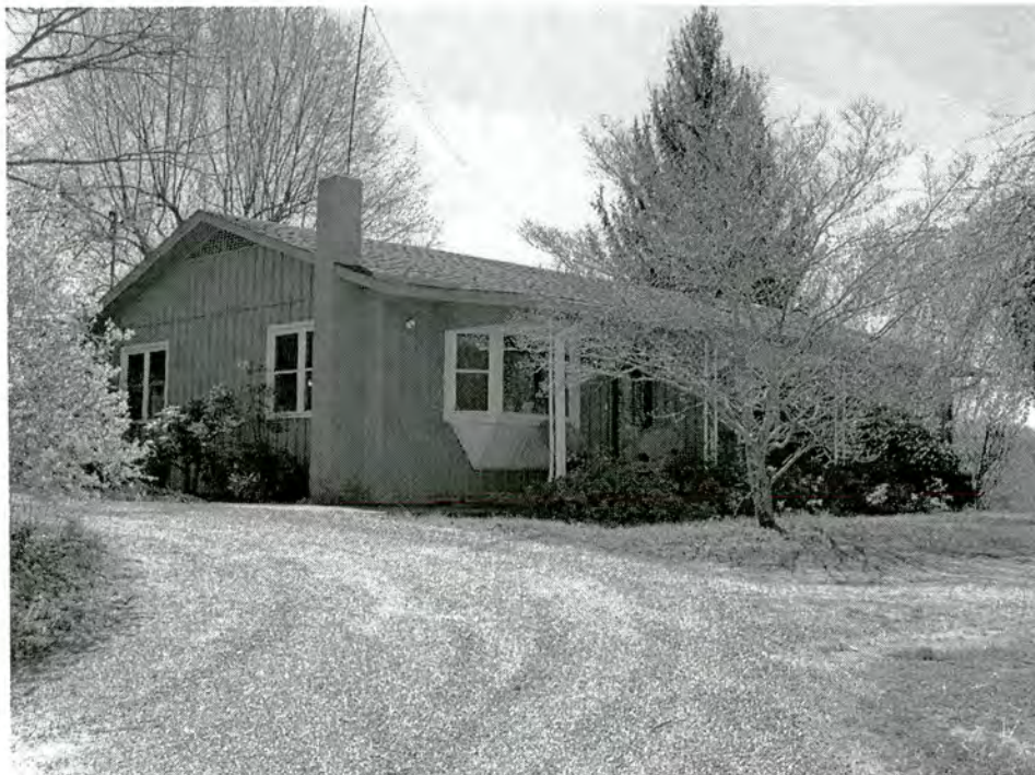
Jim and Sue Waldrop House, North and West Elevations
