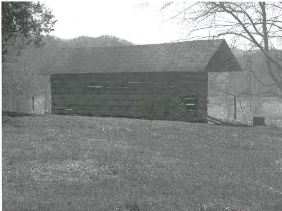
Log Corn Crib, North and West Elevations
