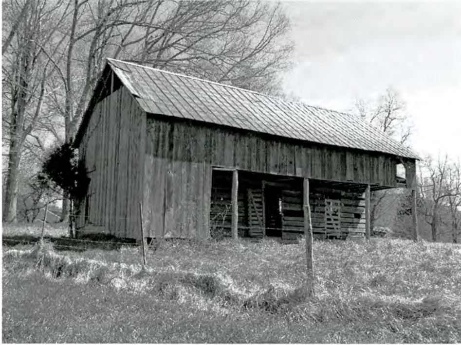
Field Barn, South and West Elevations
