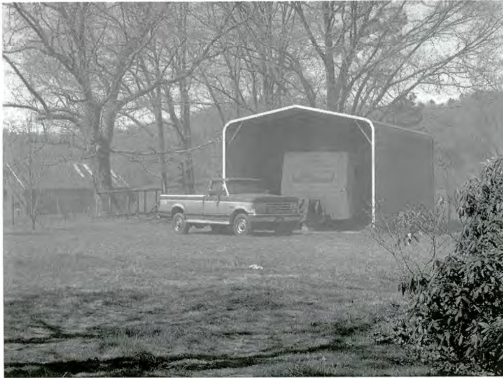
Metal Shed, North and East Elevations
