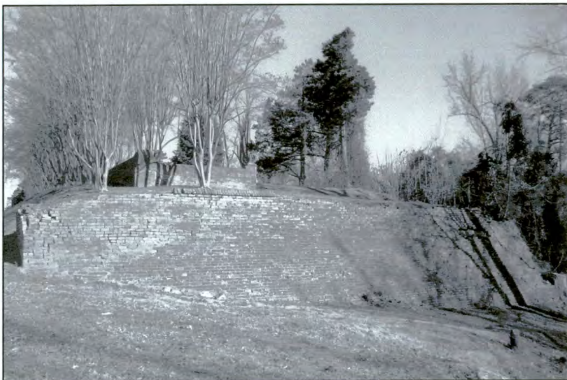
Plate 6: Southern retaining wall
