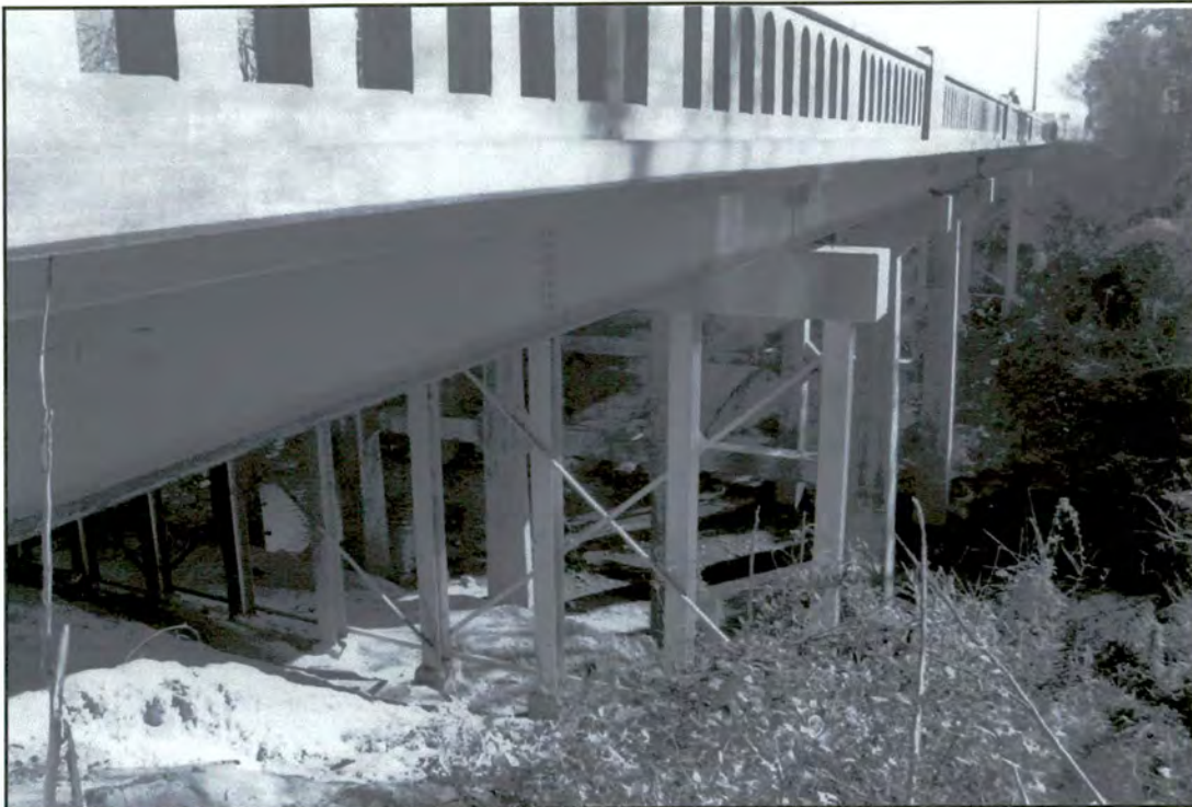
Plate 29: Bridge No. 125, south elevation
