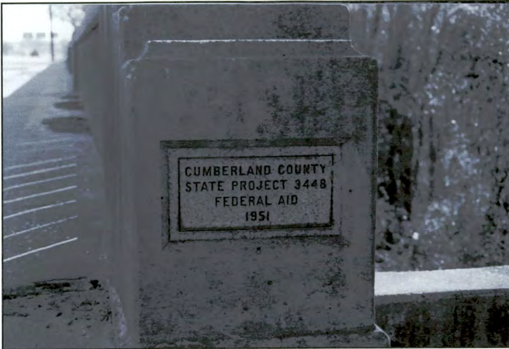
Plate 27: Bridge No. 125 detail: "Cumberland County, State Project 3448, Federal Aid, 1951"
