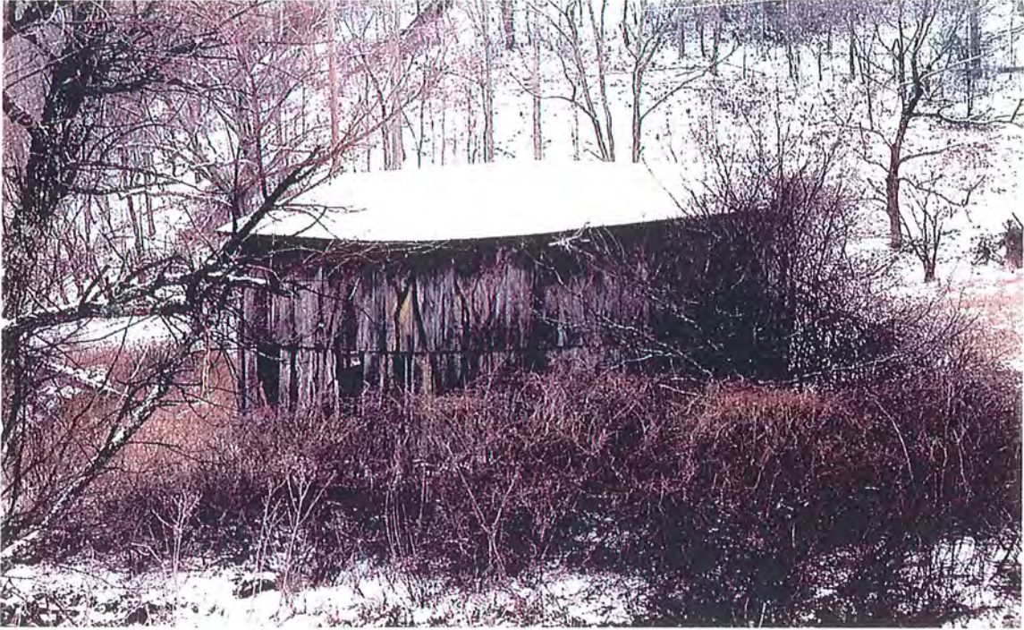
Plate 5. Graham-Brooks Farm – outbuilding 2
