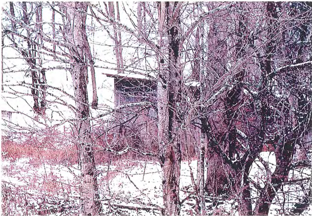
Plate 4. Graham-Brooks Farm – outbuilding 1 (shed)
