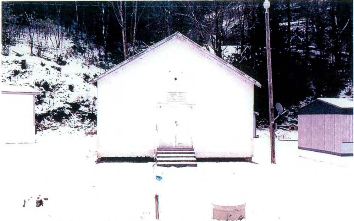
Plate 1. Laurel Hill Baptist Church - façade (west elevation)
