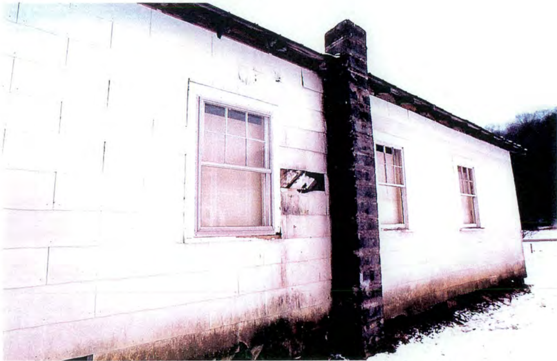
Plate 2. Laurel Hill Baptist Church - north elevation
