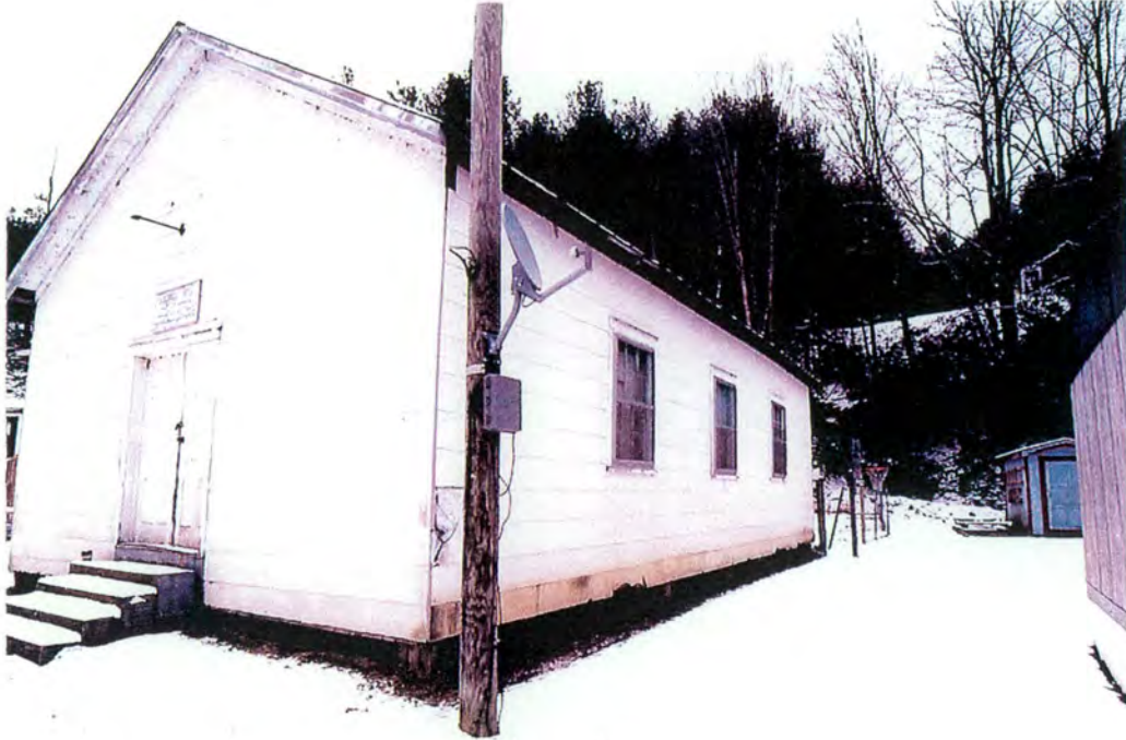
Plate 3. Laurel Hill Baptist Church – south elevation
