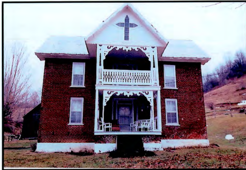
Plate 21. Hardin-Sutherland Farm house - south elevation
