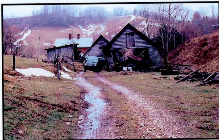
Plate 28. View of Barn #1, Log Barn, and Shed#1
