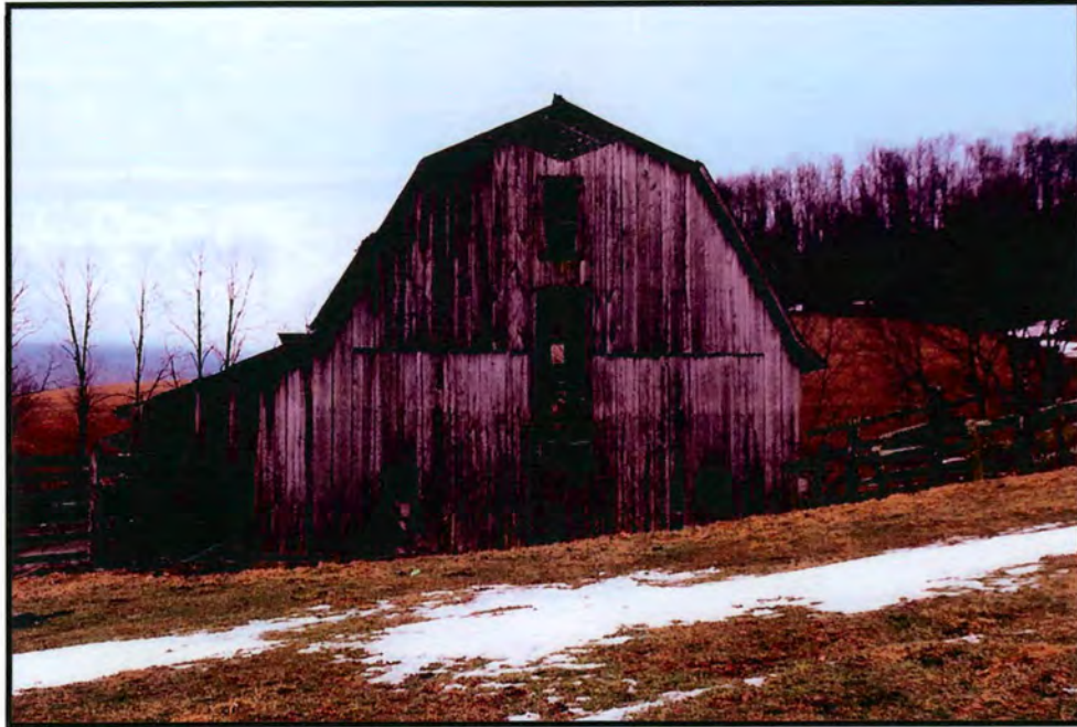
Plate 60. Gambrel roof barn
