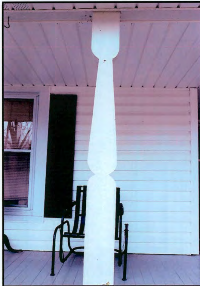
Plate 90. porch post detail
