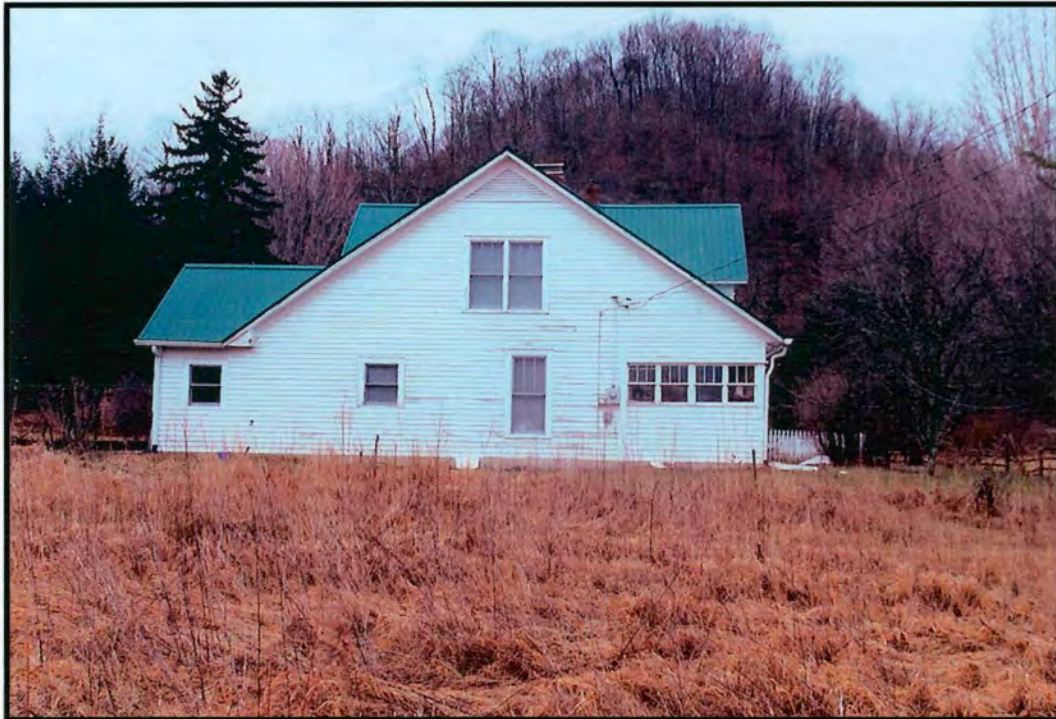
Plate 6. House - east elevation
