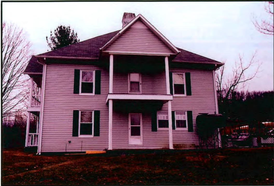
Plate 56. Wilson Farm house - west elevation
