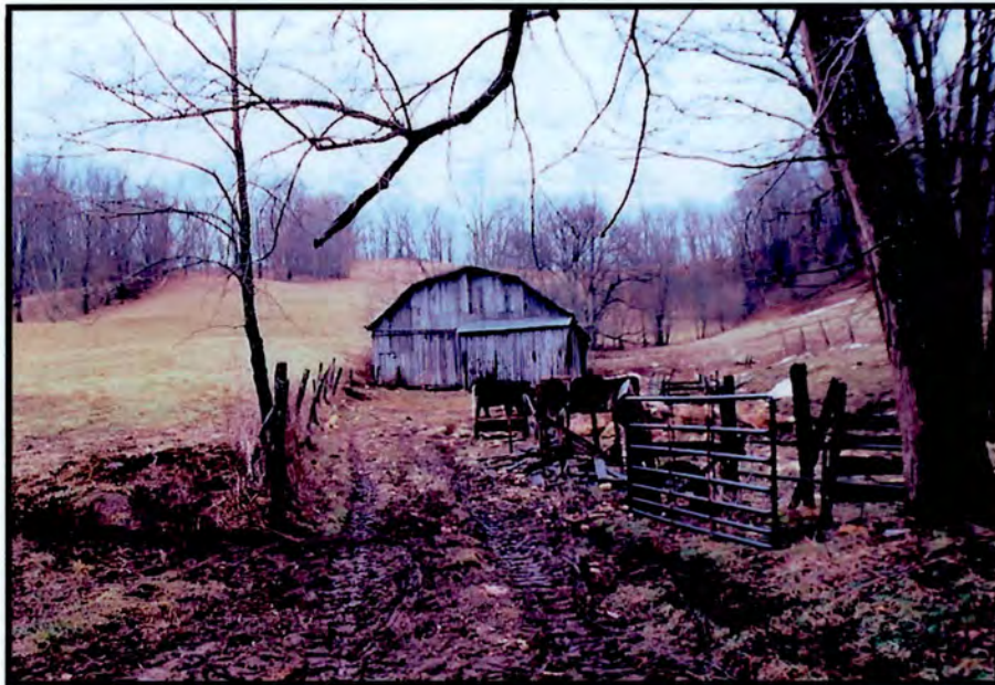
Plate 34. Gambrel Roof Barn
