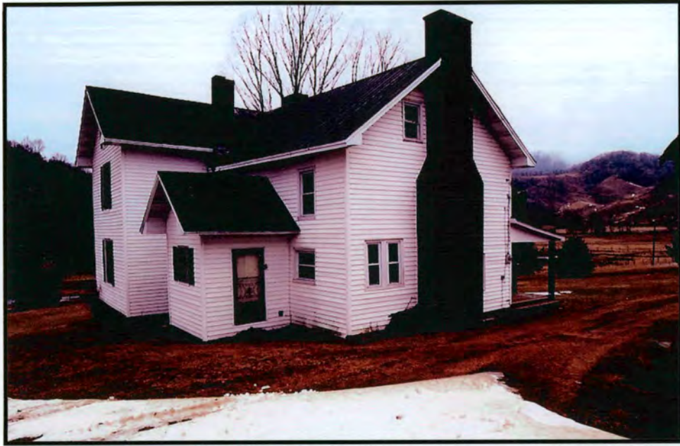
Plate 68. Thomas "Red" Sutherland Farm house -south elevation
