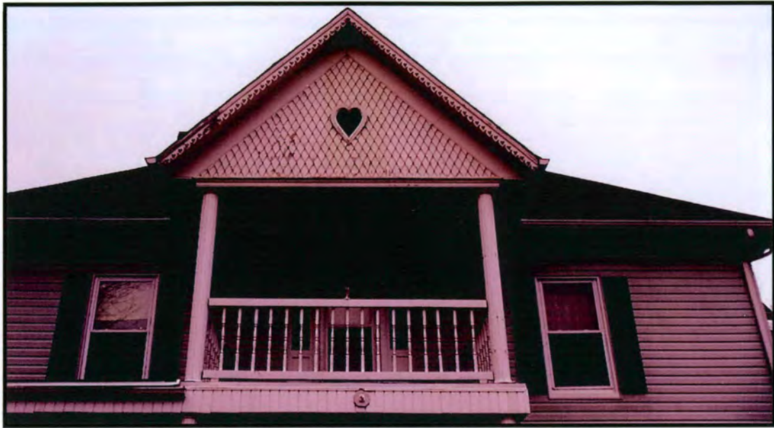
Plate 58. Wilson Farm house - front porch detail
