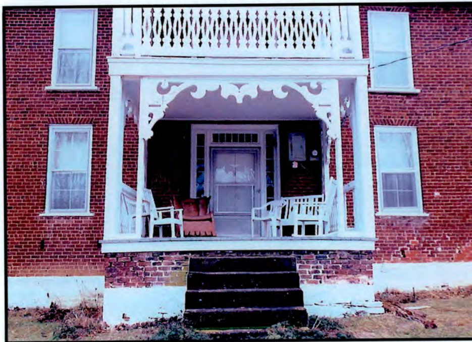
Plate 24. Hardin-Sutherland Farm house - entry detail
