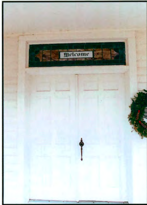
Plate 18. Church - entry detail
