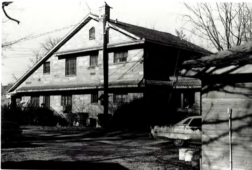
Plate 8. House, 201 South Main Street, South and Rear Elevations, Looking Northwest.
