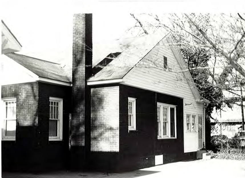
Plate 14. House, 203 South Main Street, South and Rear Elevations, Looking North.
