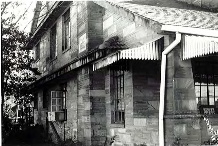
Plate 7. House, 201 South Main Street, North Elevation and Porch, Looking East.
