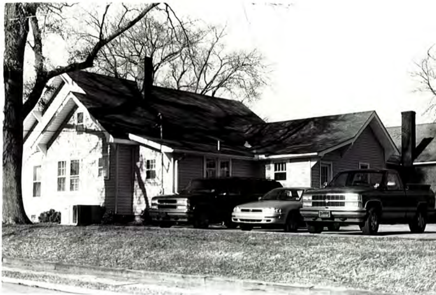
Plate 16. House, 205 South Main Street, South and Rear Elevations, Looking Northwest.
