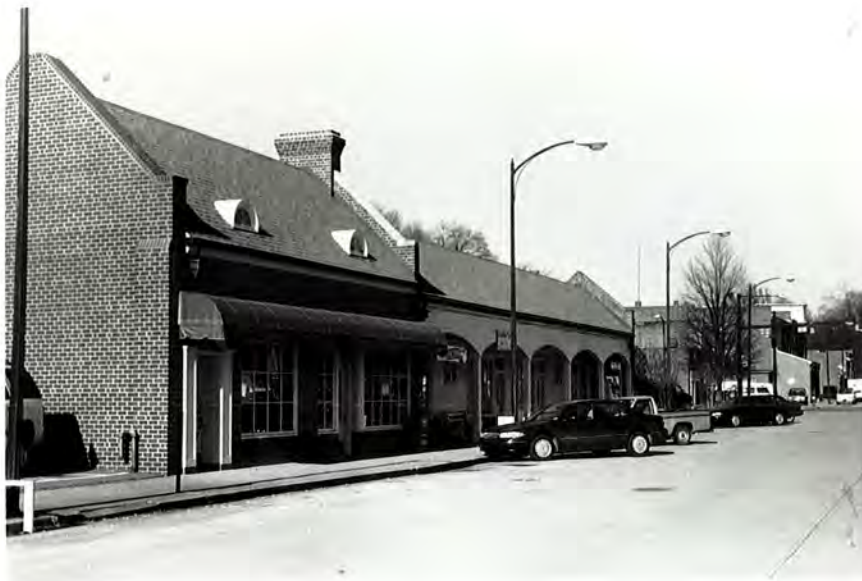
Plate 2. Commercial Block, Kannapolis Central Business District, Looking South.
