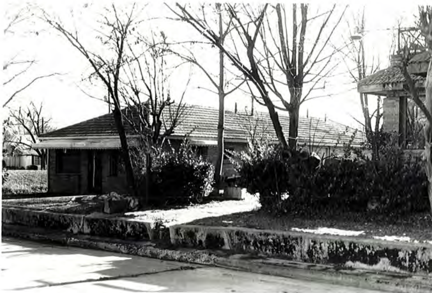
Plate 10. Garage, 201 South Main Street, Looking Southeast.
