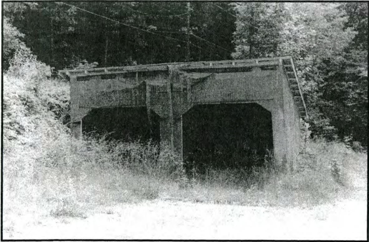
Figure No. 56. Thorpe worker's housing, associated garage.
