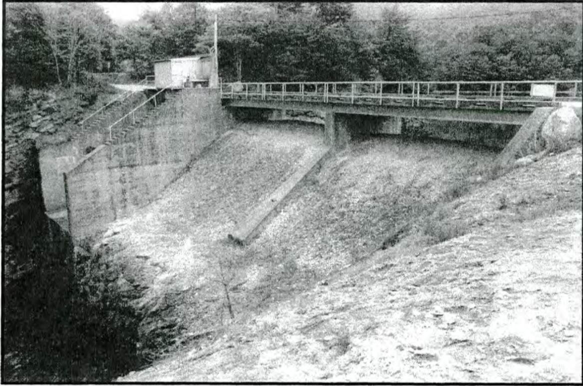
Figure No. 108. The Wolf Creek Dam, view of spillway below dam.
