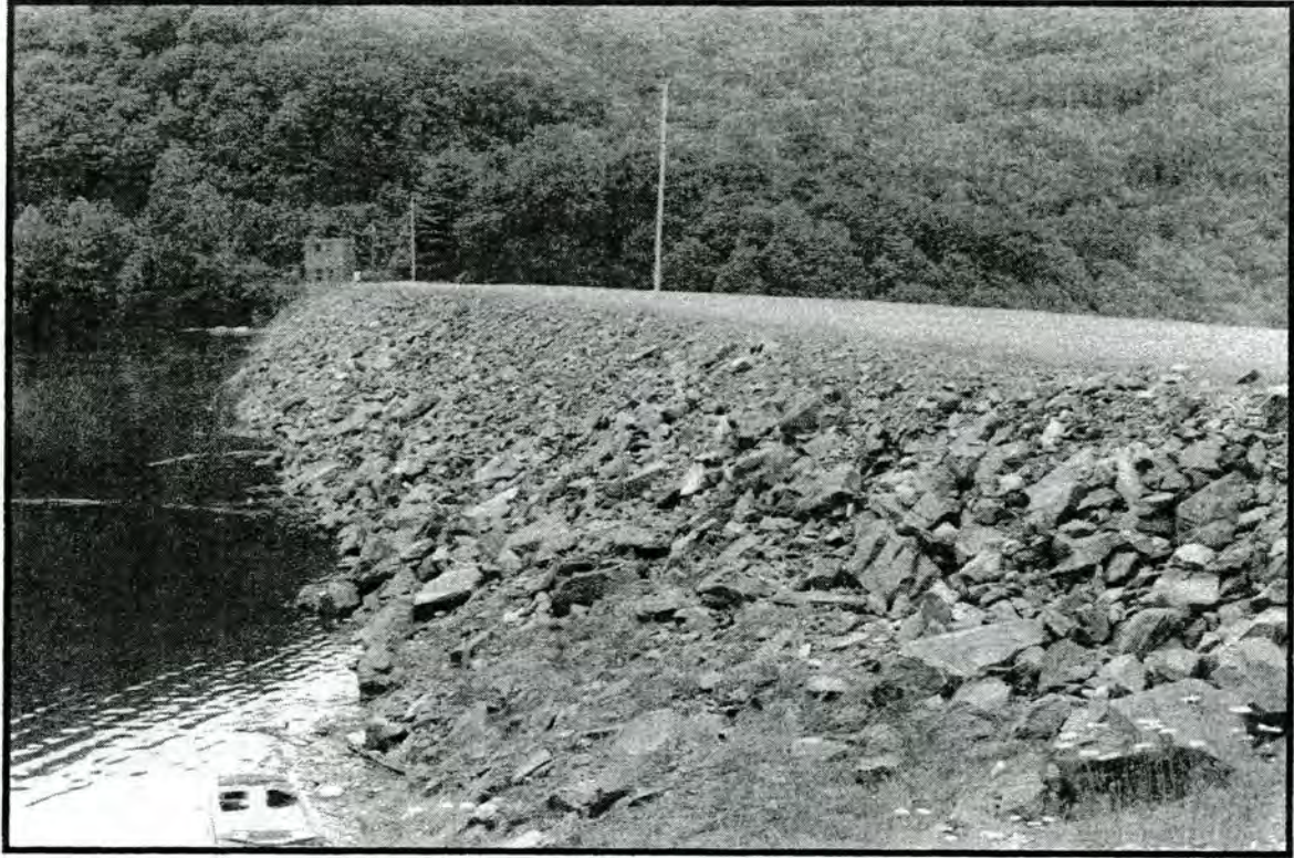
Figure No. 72. The Nantahala Dam, view above dam.
