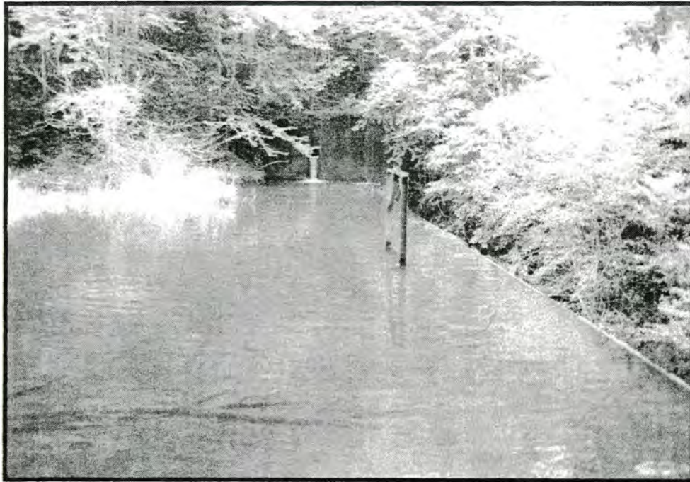
Figure No. 88. The Dicks Creek Dam, view above dam.
