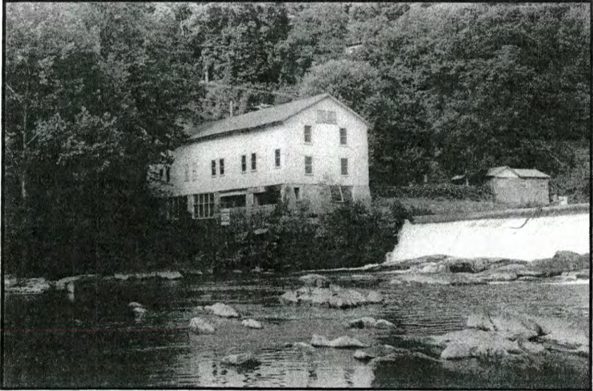
Figure No. 7. The Dillsboro Powerhouse, south and west facades.
