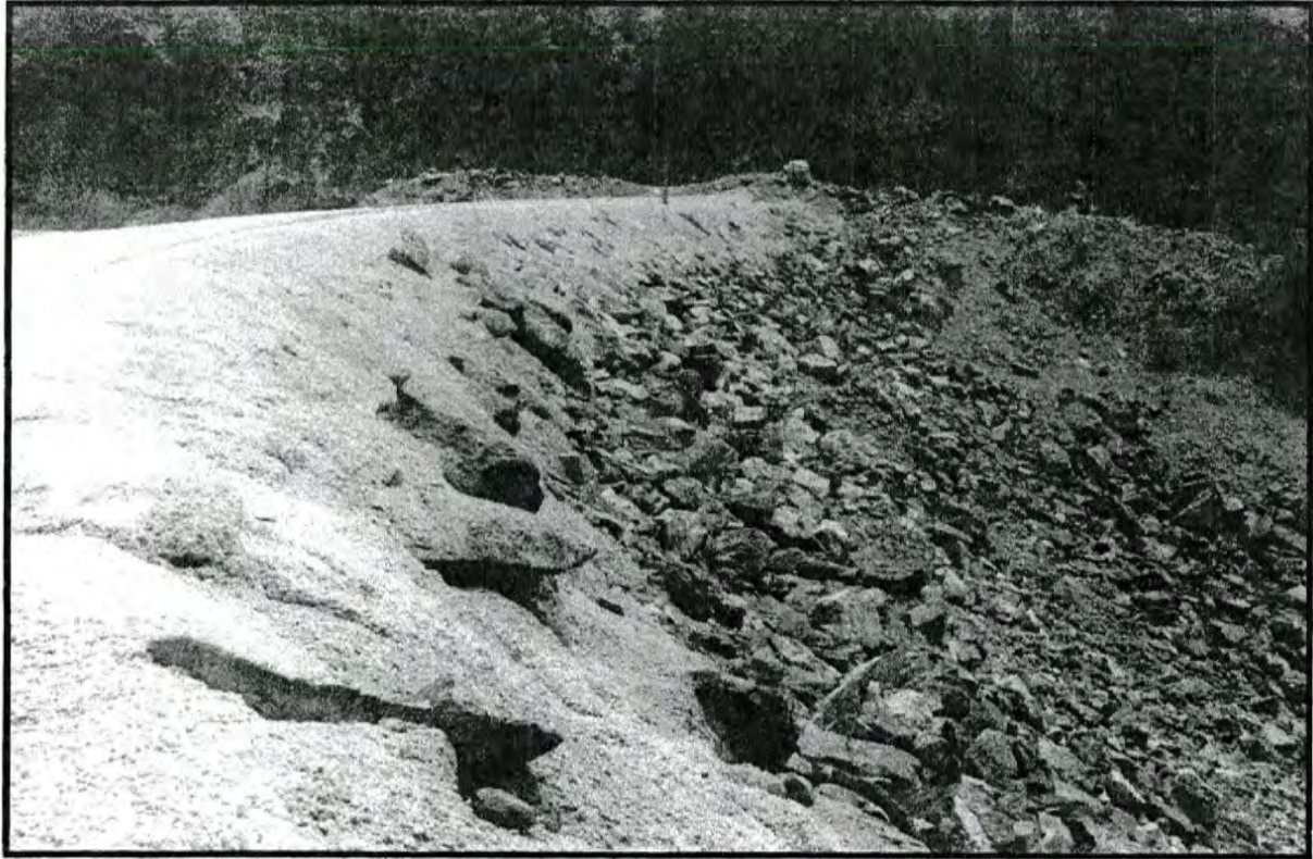
Figure No. 99. The Cedar Cliff Dam, view below dam.
