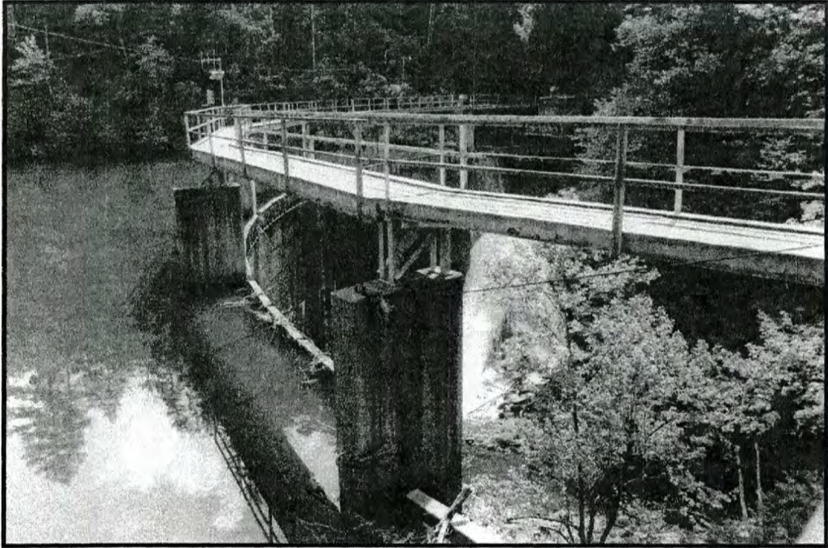
Figure No. 60. The Tuckasegee Dam, view from above.
