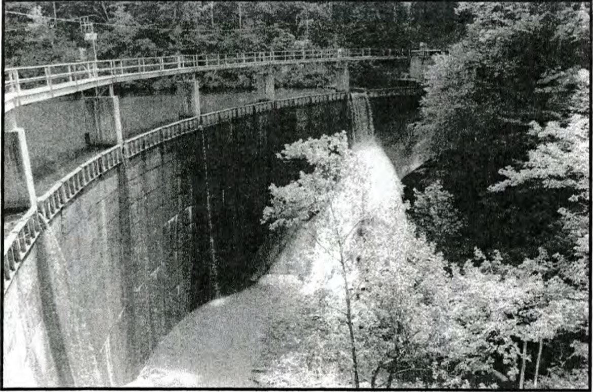
Figure No. 61. The Tuckasegee Dam, view from below.
