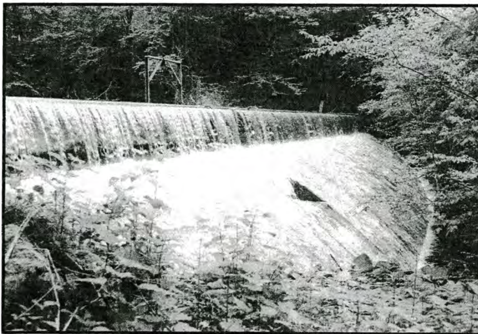
Figure No. 89. The Dicks Creek Dam, view below dam.
