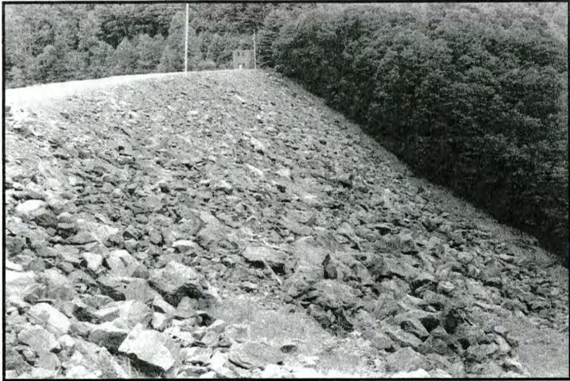
Figure No. 73. The Nantahala Dam, view below dam.
