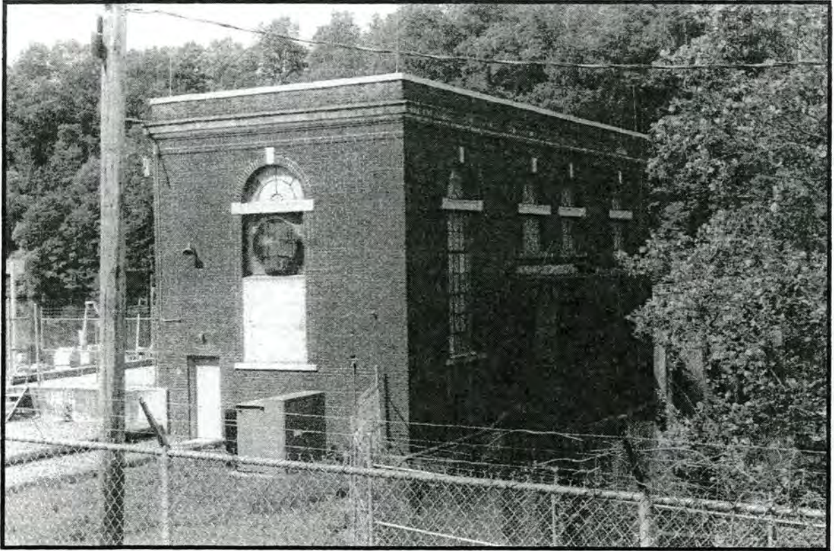
Figure No. 32. The Franklin Powerhouse, south and east facades.
