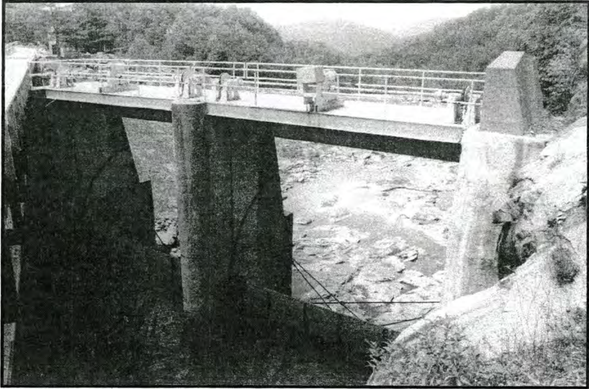
Figure No. 48. The Thorpe Dam, concrete spillway and tainter gates.
