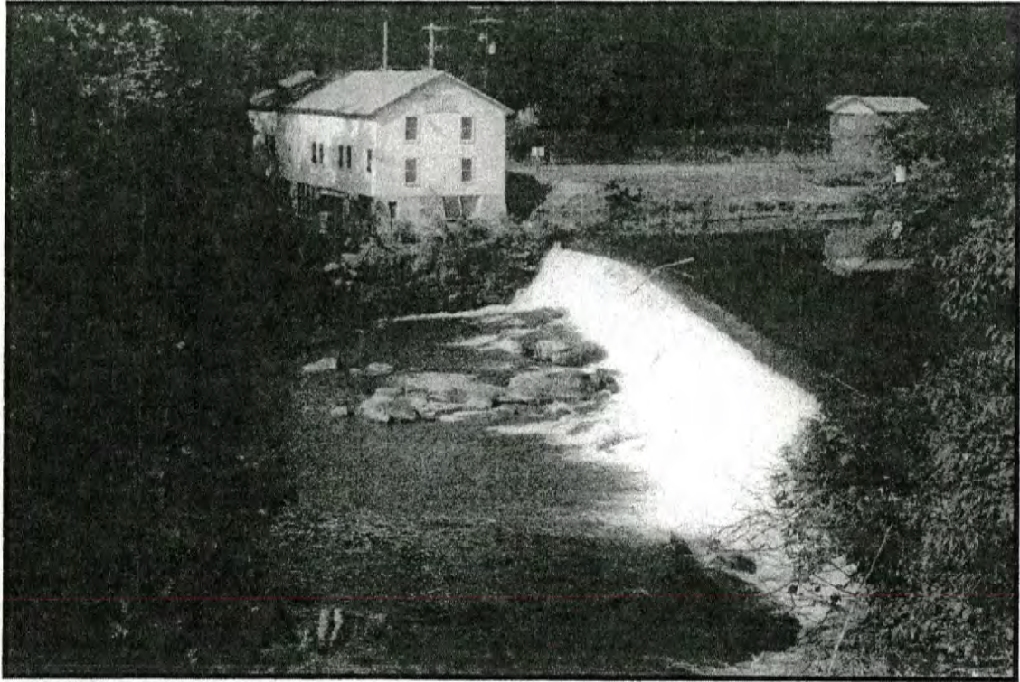
Figure No. 6. The Dillsboro Powerhouse and Dam.
