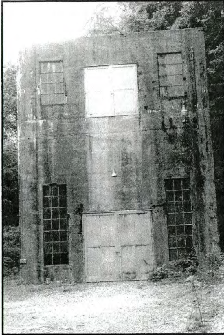
Figure No. 77. Nantahala Dam intake gatehouse.
