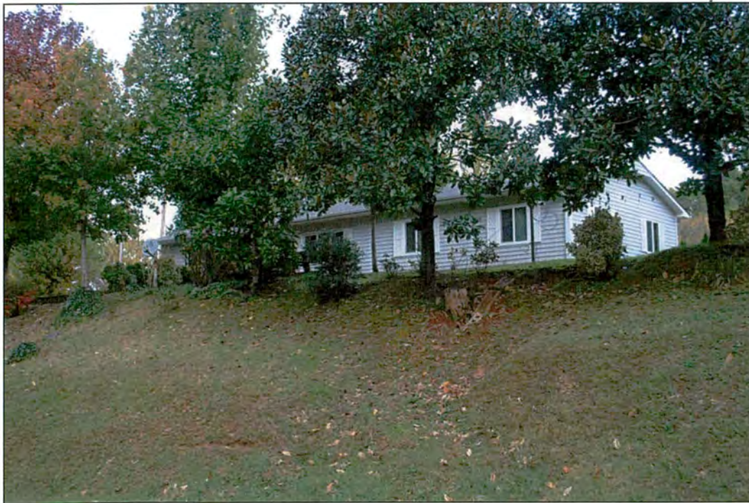
Property No. 51: 3263 Massey Branch Road PIN: N/A No architectural or archaeological significance
