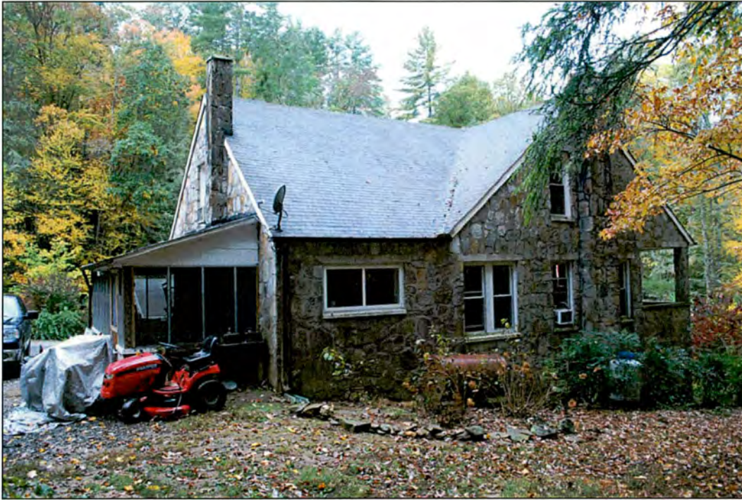
Figure 7: Garland House, south and east elevations. Katherine Husband, NCDOT, October 2011.
