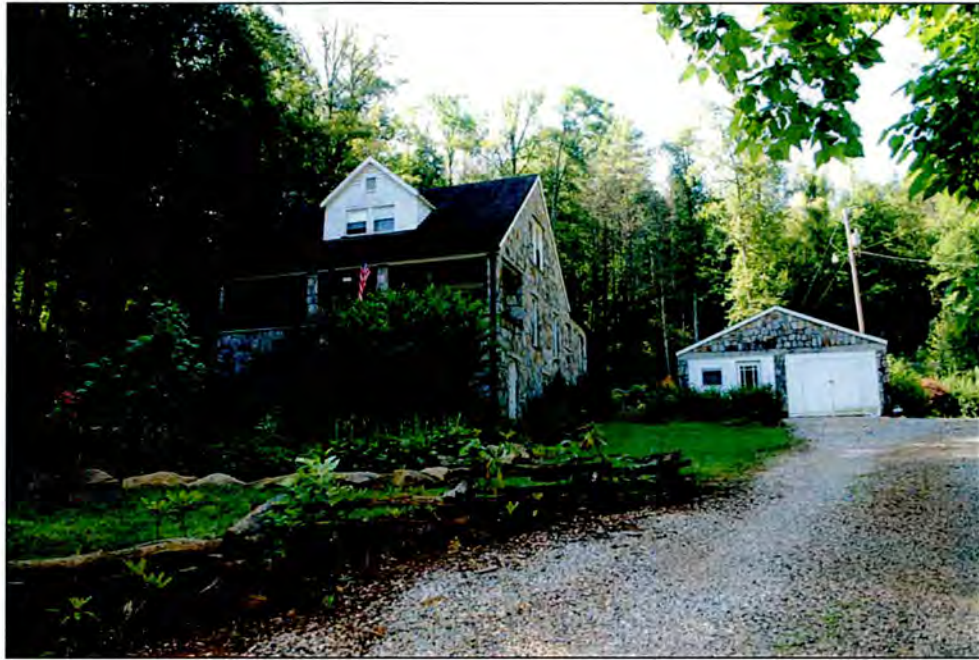
Figure 3: Garland House, looking south. Katherine Husband, NCDOT, June 2011.
