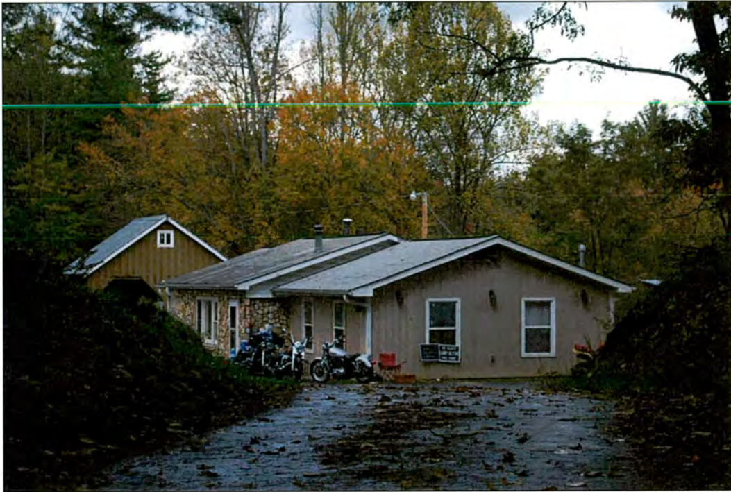
Property No. 48: 3341 Massey Branch Road PIN: N/A No architectural or archaeological significance
