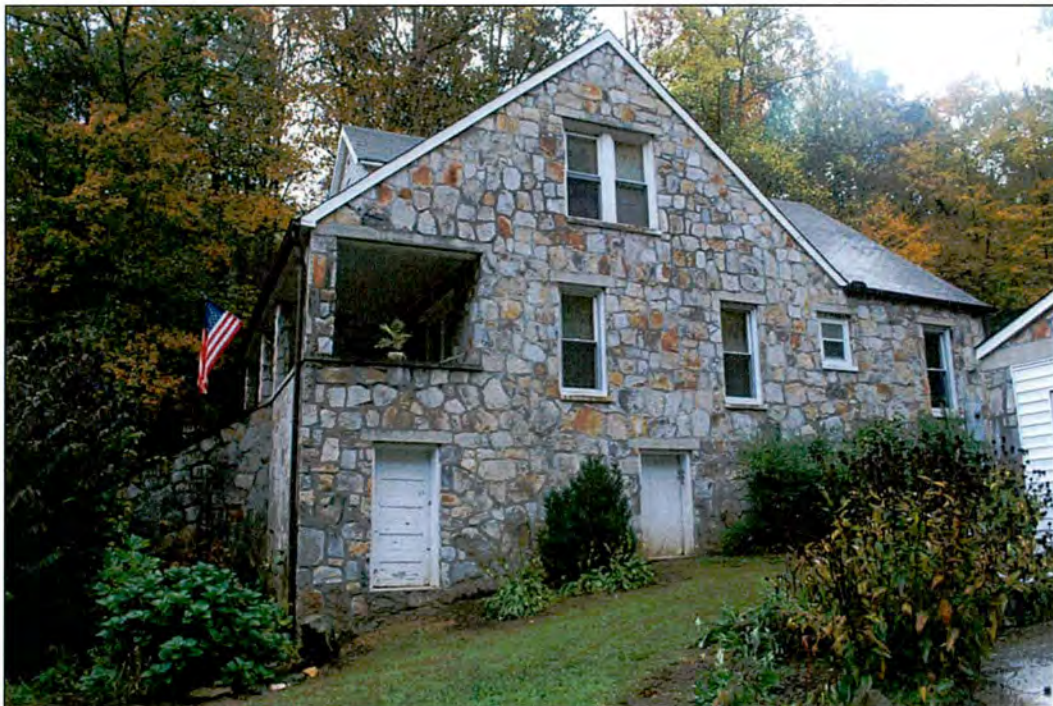
Figure 6: Garland House, west elevation. Katherine Husband, NCDOT, October 2011.
