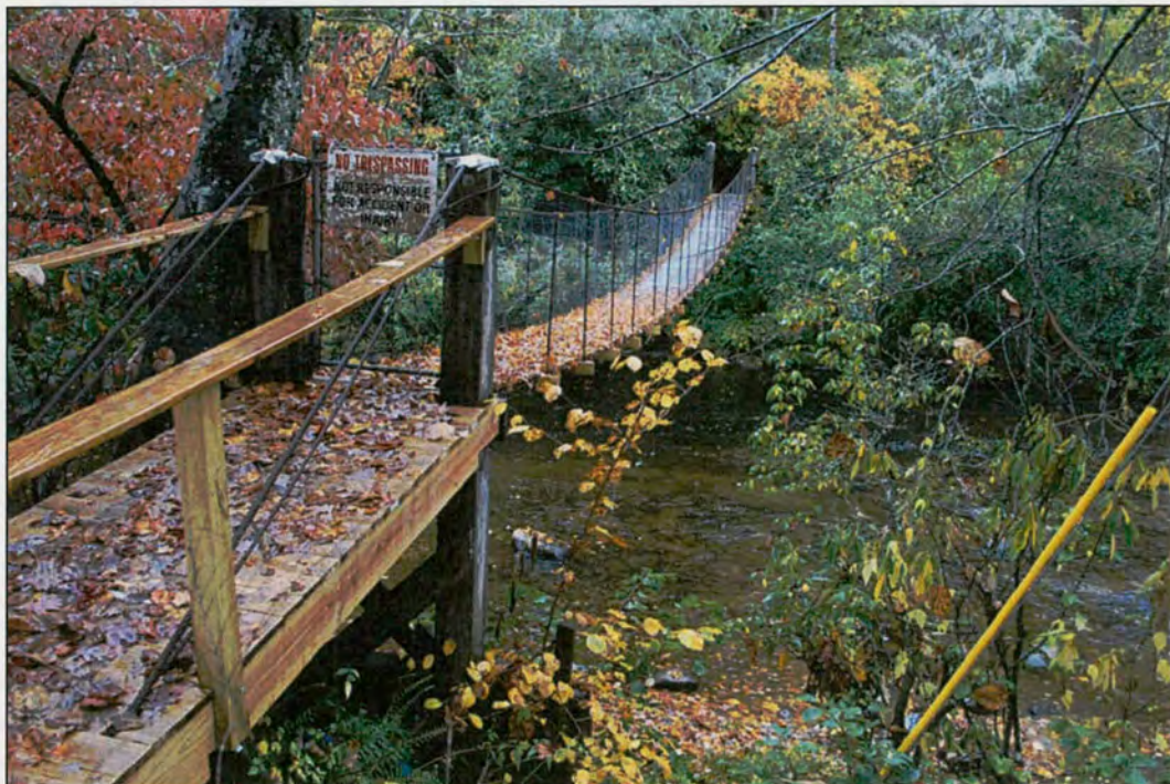
Property 16: Snowbird Suspension Bridge PIN: N/A Loss of integrity, architectural or archaeological significance.
