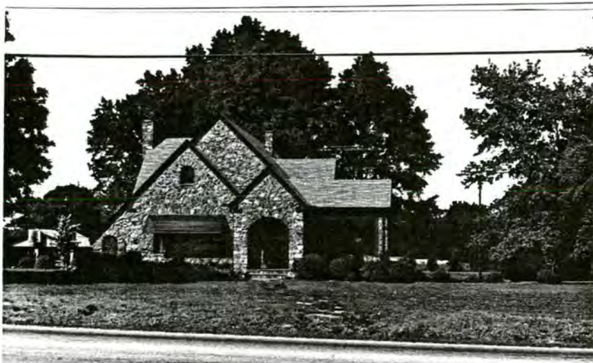
Plate 19. Barringer-Lanning House, Facade, Looking East.
