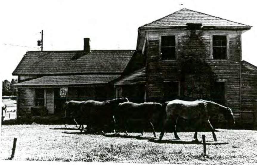
Plate 167. Victor Melchor House, East Elevations, Looking West.
