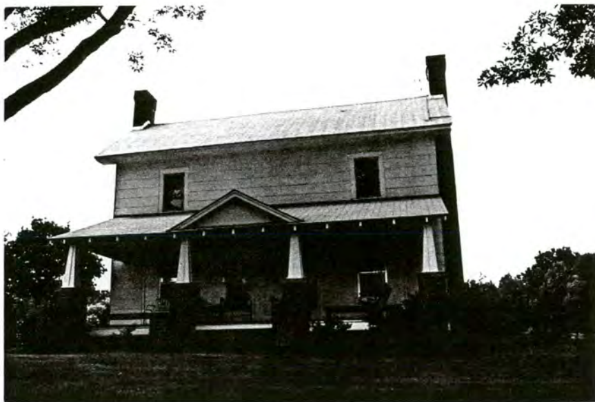
Plate 107. Arey House, Facade, Looking North.
