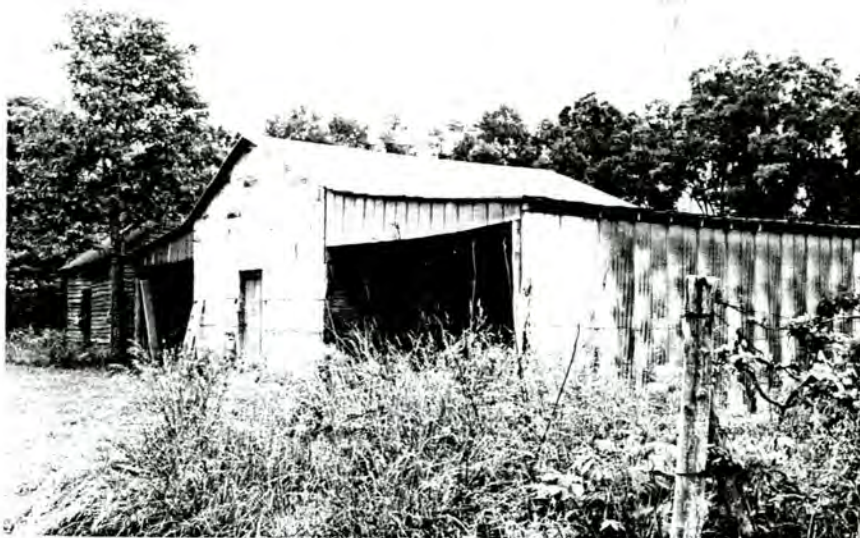
Plate 140. Daniel C. Faggart House, Outbuildings, Looking South.
