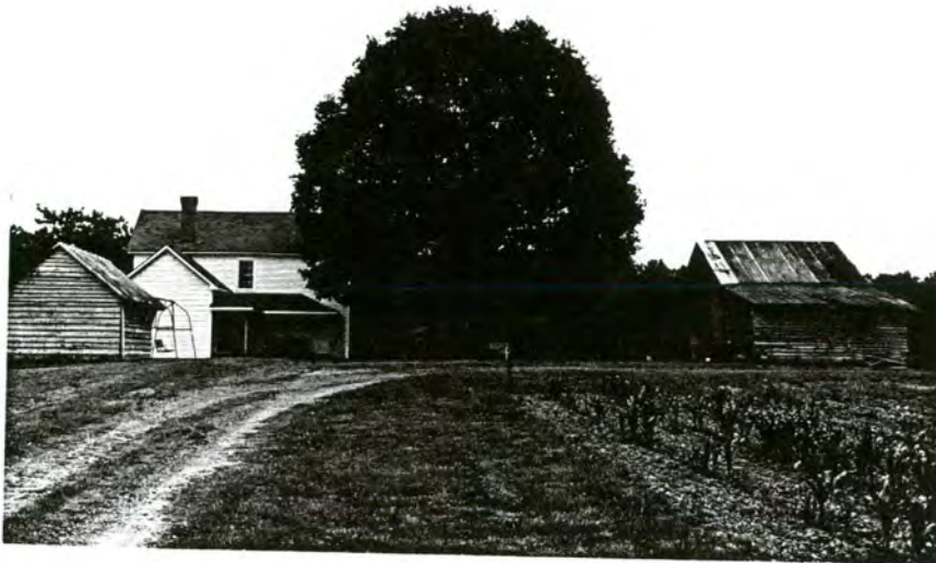
Plate 165. McLester-Fraley House, Rear Elevation, Outbuildings, Looking South.
