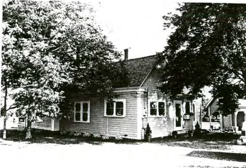
Plate 62. George Miller House, Rear Ell, Looking South.
