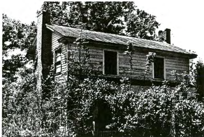
Plate 100. Morgan Walker House, Facade and South Elevation, Looking West.
