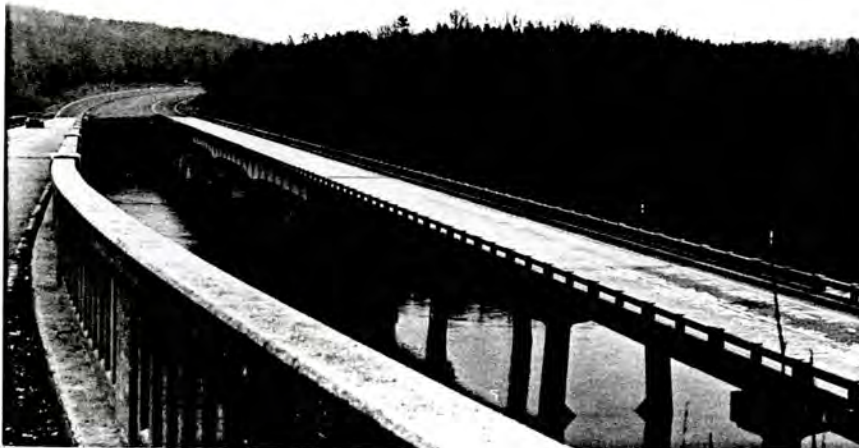
Plate 84. Stokes Ferry Bridge and 1960 Bridge, Looking East.
