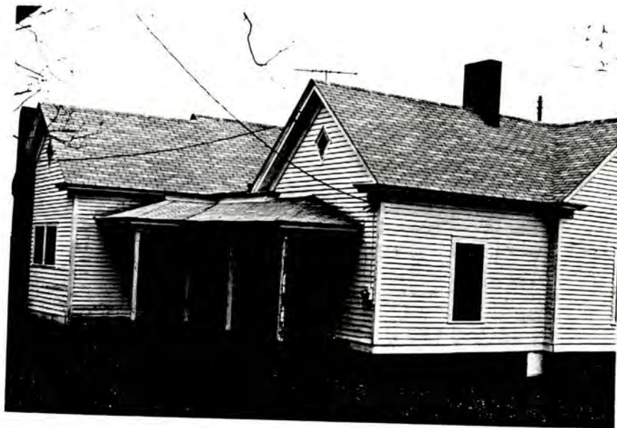
Plate 157. House, Rear Elevation, Looking Southeast.
