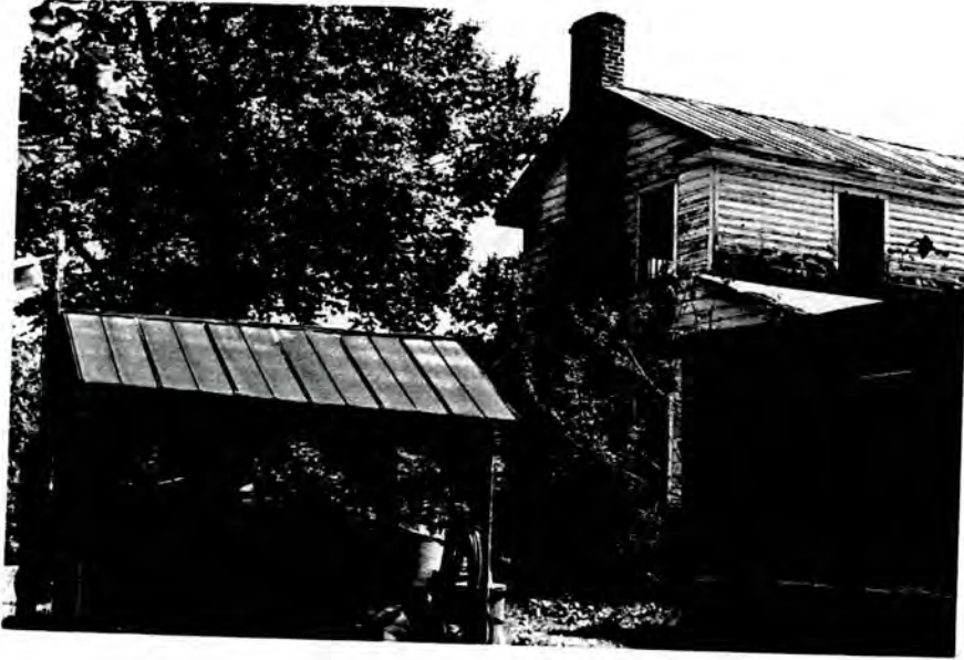
Plate 105. Morgan Walker House Property, Well Canopy, Looking East.
