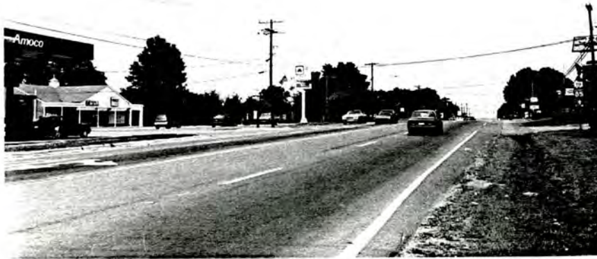
Plate 1. Western Terminus of Project, Looking East.
