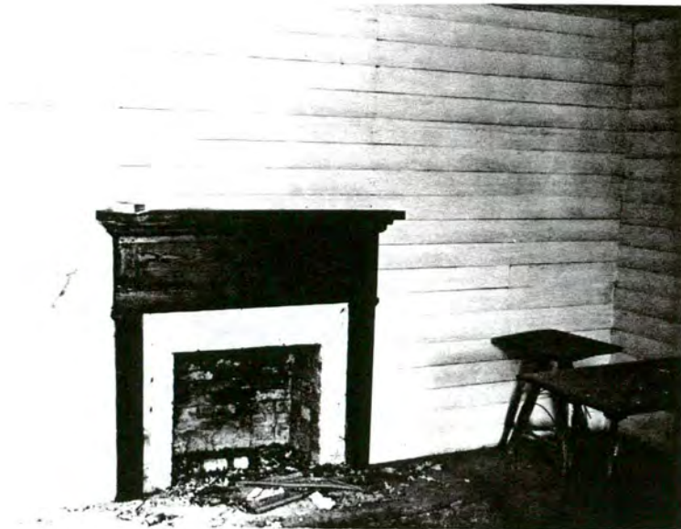
Plate 15. Daniel Luther Barringer House, Mantel in Upstairs Bedroom.
