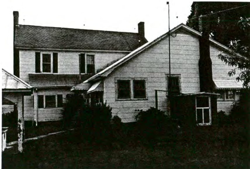
Plate 50. A. C. Lentz House, Rear Elevation, Looking West.
