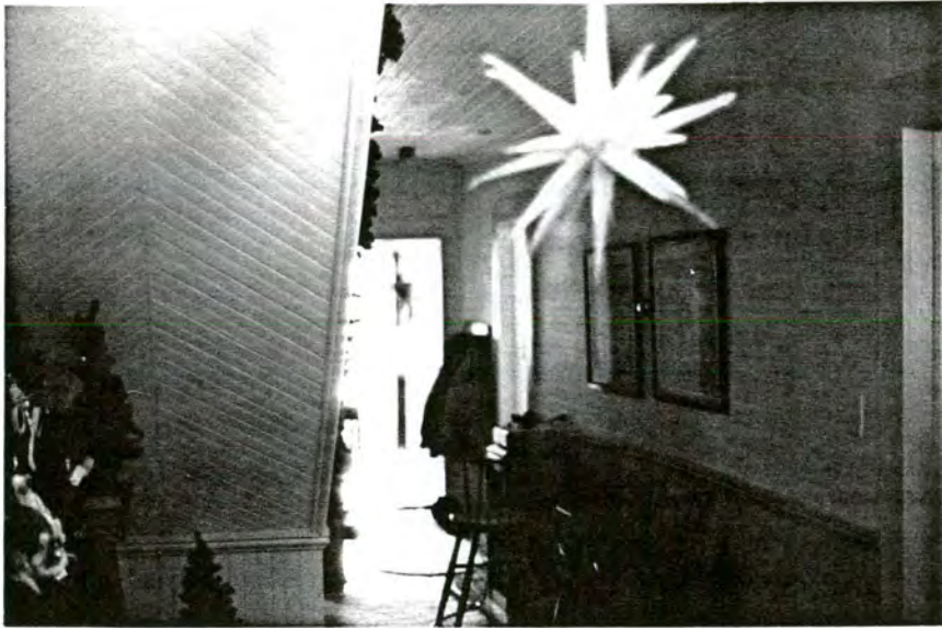
Plate 65. George Miller House, Stairhall.
