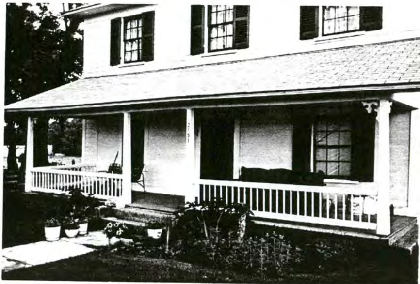
Plate 27. Barringer-Melchor House, Facade, Looking North.
