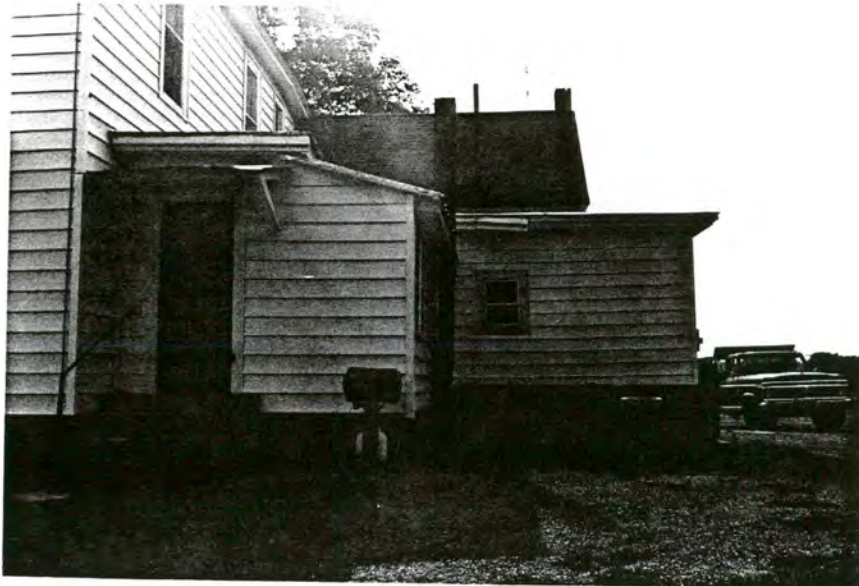
Plate 144. Walter Fisher House, Rear Wings, Looking North.
