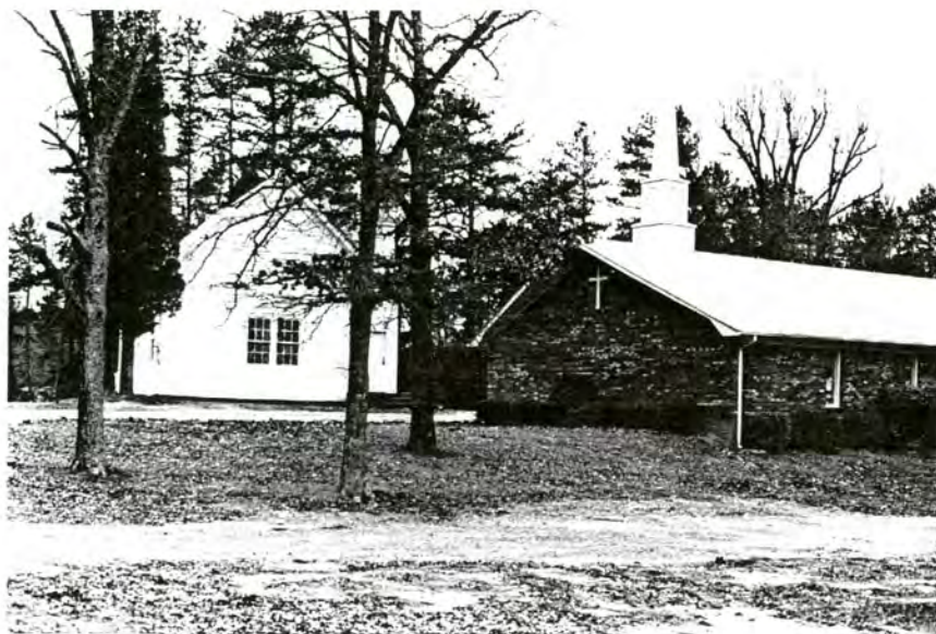
Plate 73. St. Peter's Lutheran Church and Modern Church Building, Looking West.
