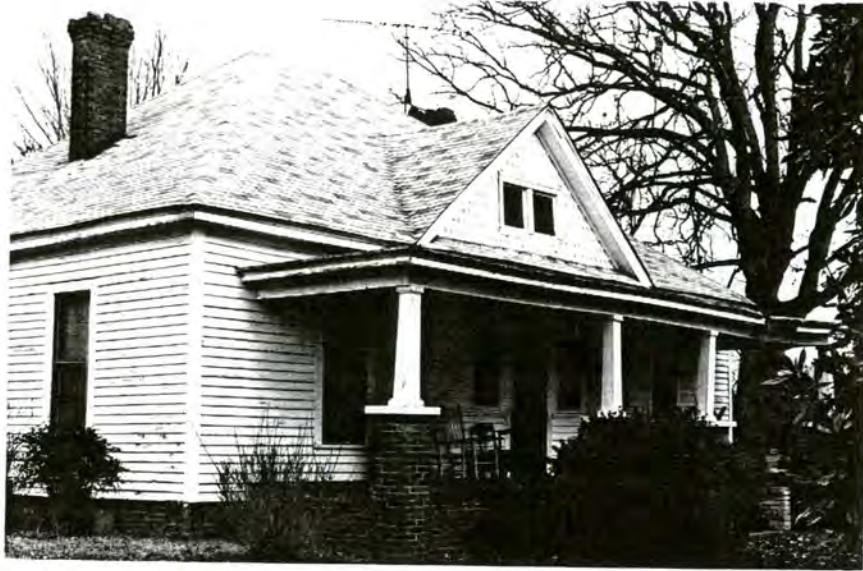
Plate 111. Corum Barbee House, Facade, Looking North.
