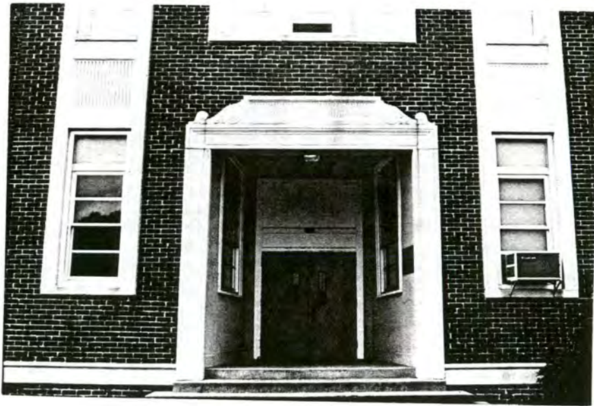
Plate 171. Mount Pleasant High School, Detail Of Entrance Bay, Looking West.
