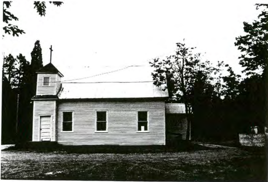
Plate 76. St. Peter's Lutheran Church, North Elevation, Looking South.
