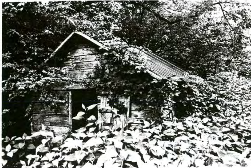
Plate 104. Morgan Walker House Property, Smokehouse, Looking West.
