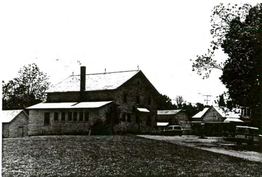
Plate 52. A. C. Lentz Farm Complex, Looking South.
