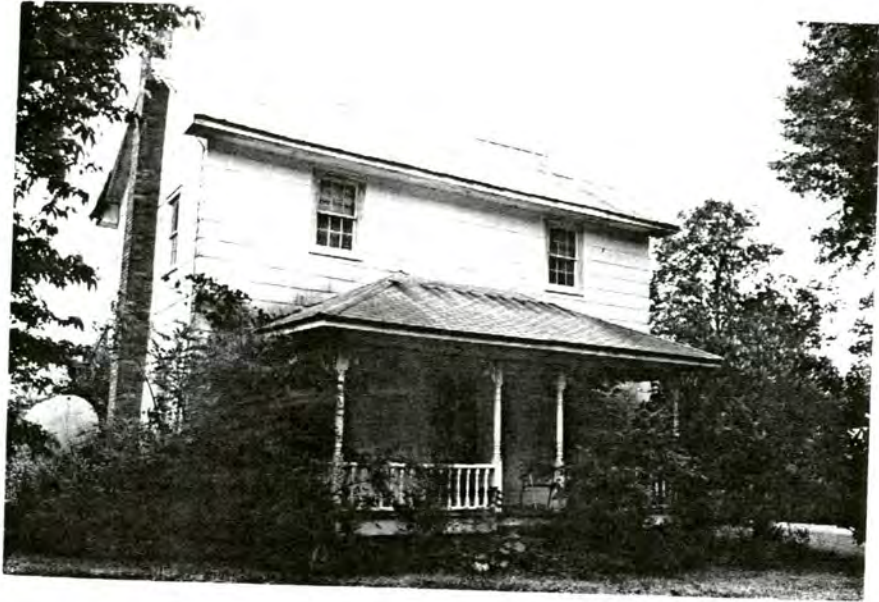
Plate 177. George H. Walker House, Facade and South Elevation, Looking Northwest.
