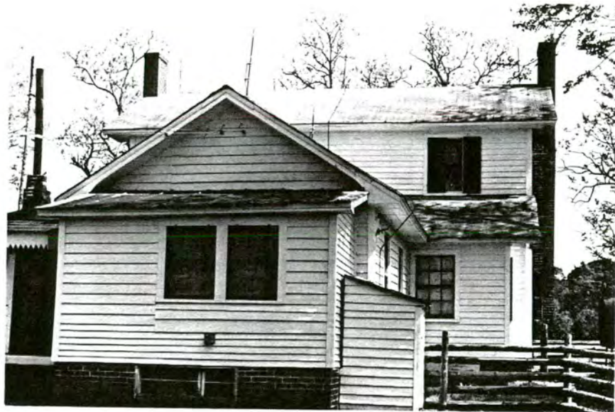
Plate 28. Barringer-Melchor House, Rear Elevations, Looking South.
