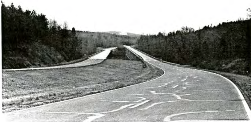
Plate 81. Stokes Ferry Bridge and Setting, Looking Southwest.
