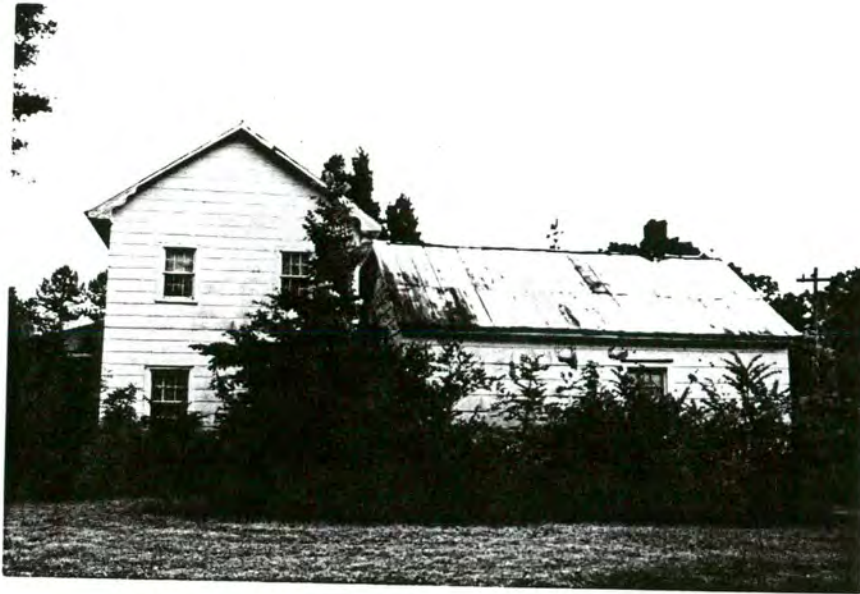
Plate 180. George H. Walker House, North Elevations of Main Block and 1885 Wing, Looking South.
