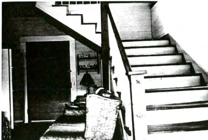
Plate 139. Daniel C. Faggart House, Stairhall.
