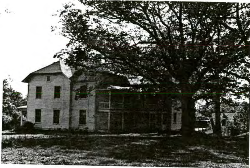
Plate 6. Daniel Luther Barringer House, East and Rear Elevations, Looking Southwest.
