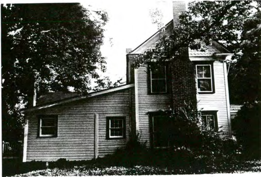
Plate 37. Bessie Dry House, East Elevation, Looking West.
