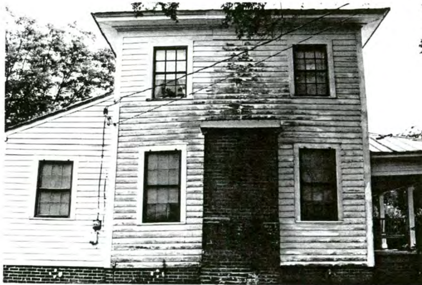
Plate 136. Daniel C. Faggart House, North Elevation, Looking South.
