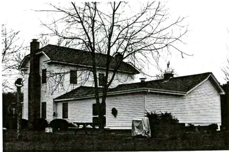
Plate 160. V. C. Lentz House, Rear and East Elevations, Looking South.
