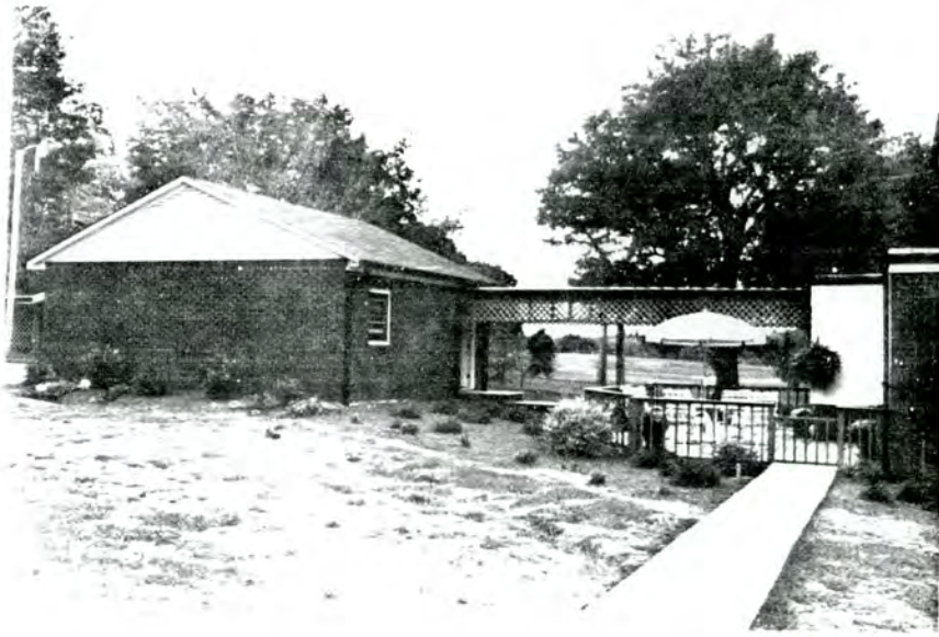
Plate 185. H. H. Cassil House, Garage and Patio, Looking West.
