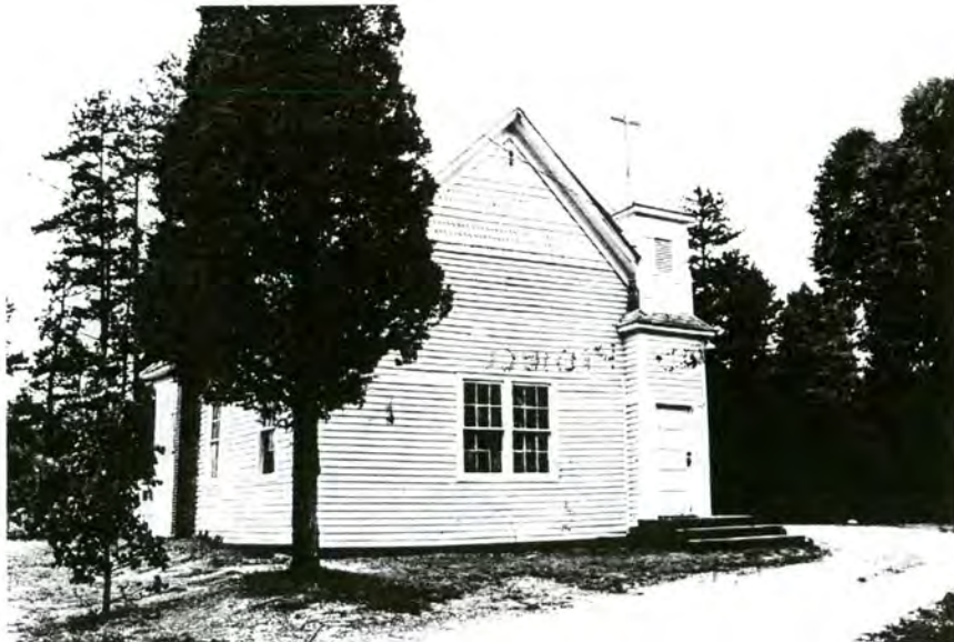
Plate 74. St. Peter's Lutheran Church, Facade, Looking West.
