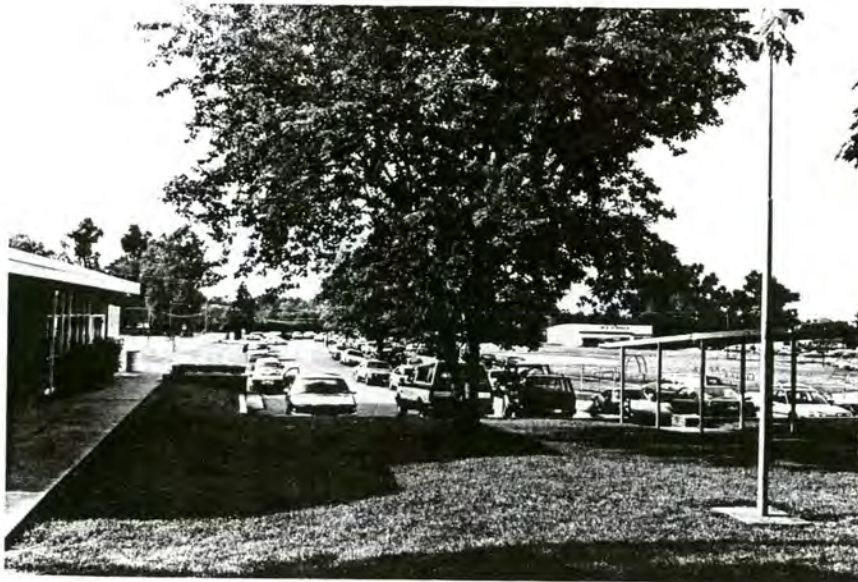
Plate 153. Harrisburg School, Looking North Towards NC 49.
