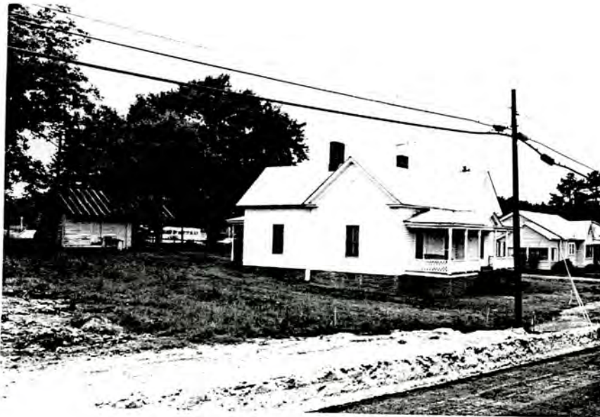
Plate 156. House, South Elevation and Well House, Looking North.
