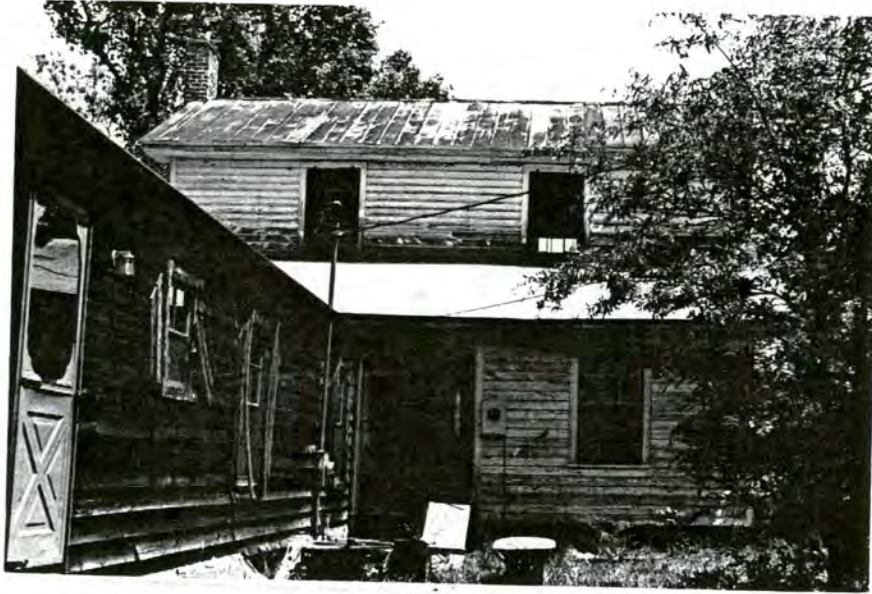
Plate 99. Morgan Walker House, Rear Elevation, Looking East.
