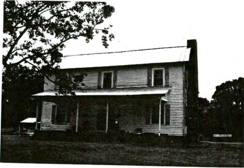
Plate 114. Barnhardt House, Facade, Looking West.
