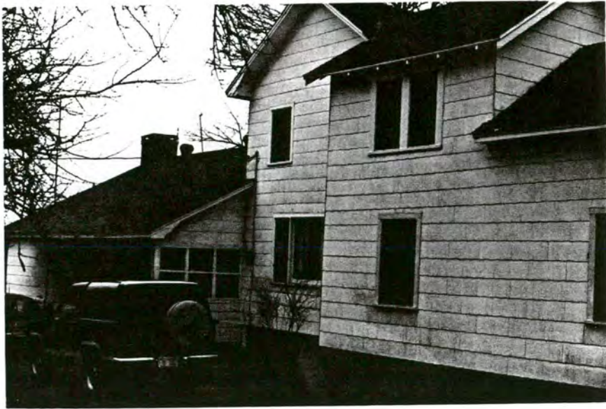
Plate 131. William Dry House, East Elevations, Looking West.
