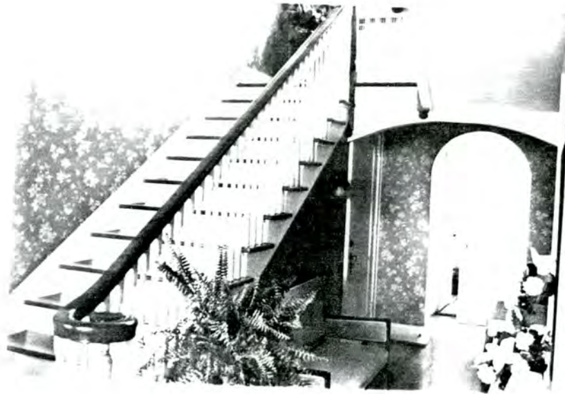
Plate 186. H. H. Cassil House, Stairhall.
