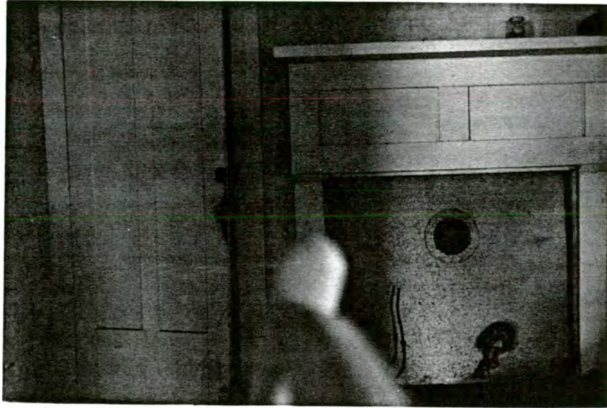
Plate 14. Daniel Luther Barringer House, Mantel in Upstairs Bedroom.
