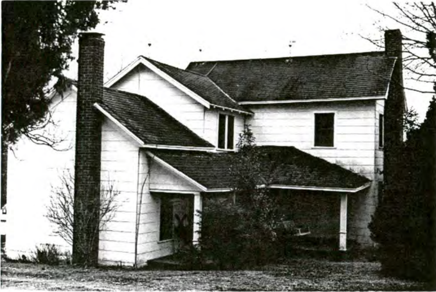
Plate 130. William Dry House, North Elevations, Looking South.
