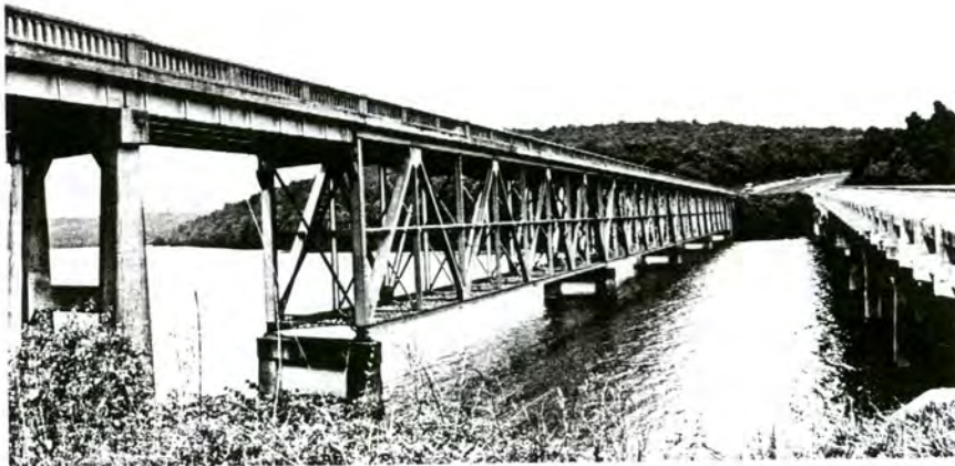
Plate 82. Stokes Ferry Bridge, Looking Northeast.
