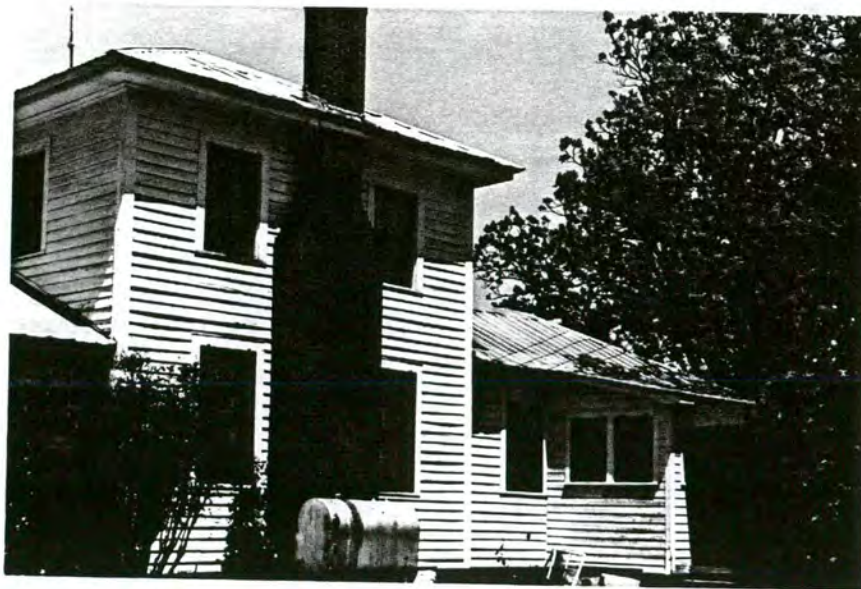
Plate 137. Daniel C. Faggart House, South Elevation, Looking Northeast.
