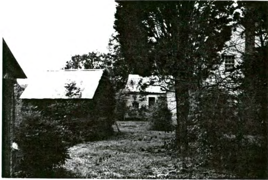
Plate 179. George H. Walker House, Smokehouse and 1885 Wing, South Elevation, Looking North.
