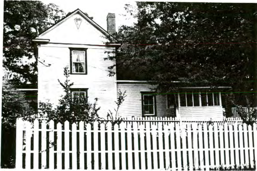
Plate 38. Bessie Dry House, West Elevation, Looking East.
