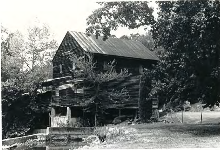
Plate 5. Whitley Mill, Rear (East) and North Elevations, Looking Southwest.
