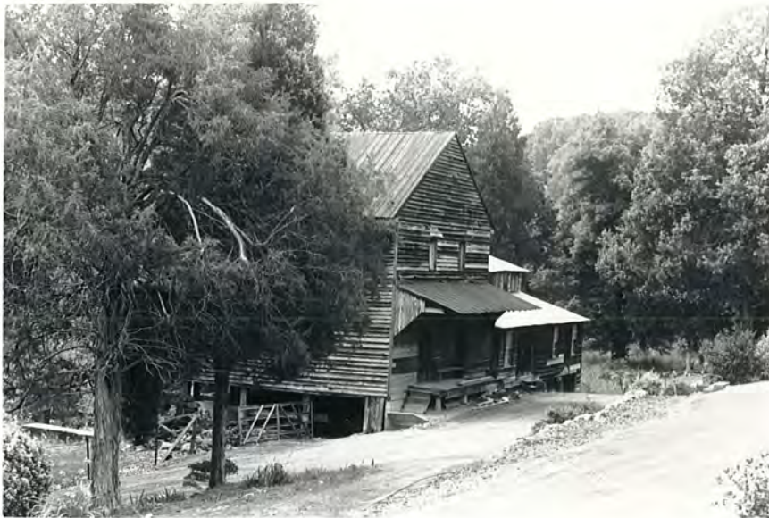
Plate 2. Whitley Mill, Facade (West Elevation) and North Elevation, Looking Southeast.
