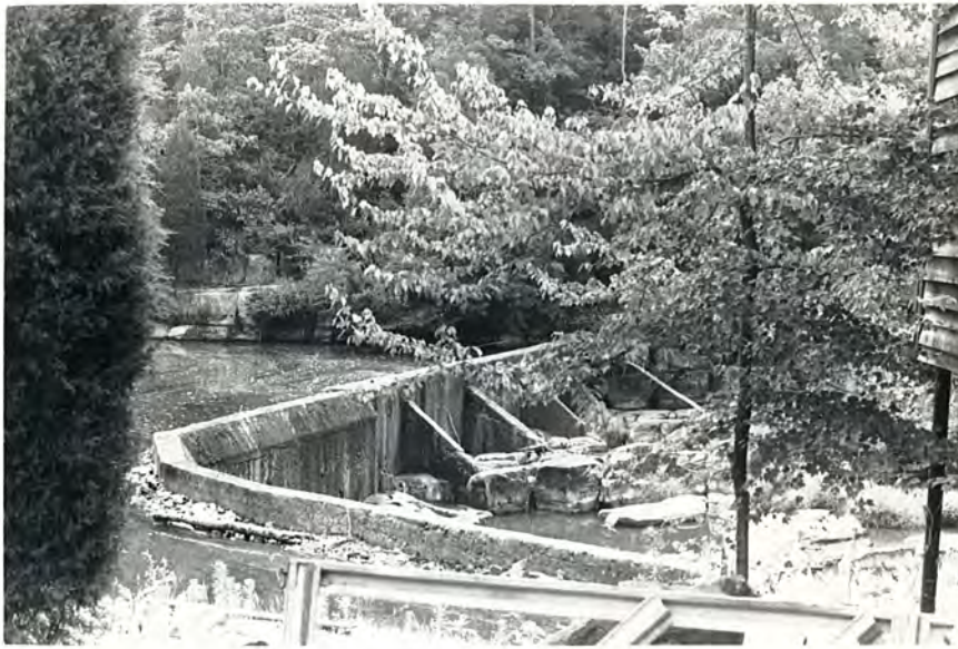
Plate 7. Whitley Mill, Concrete Dam and Big Bear Creek, Looking East.
