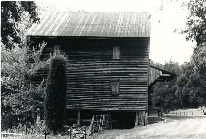
Plate 1. Whitley Mill, North Elevation, Looking South.
