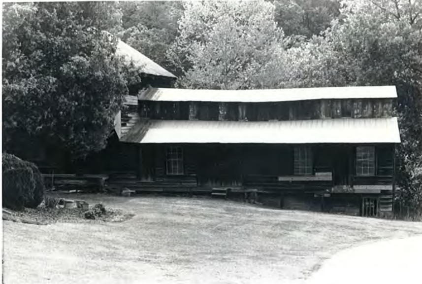
Plate 3. Whitley Mill, Woodworking Shop Appendage, Facade (West Elevation), Looking East.
