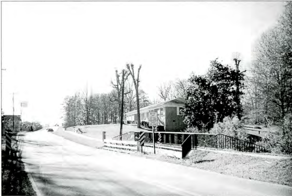
DETERMINED NOT ELIGIBLE FOR THE NATIONAL REGISTER AND NOT WORTHY OF FURTHER EVALUATION - SEE NCDOT-HPO CONCURRENCE FORM
