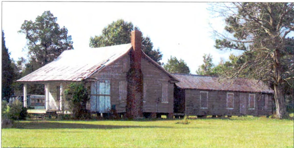
Figure 20, below: Hopkins House, north elevation
