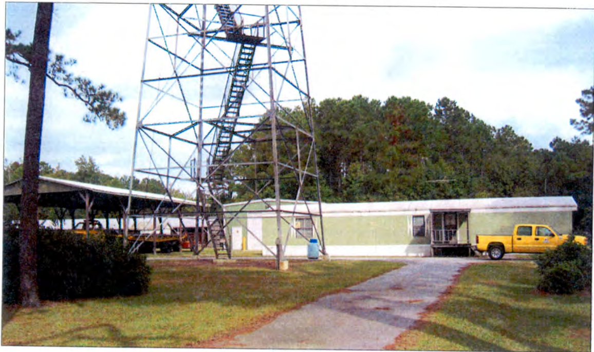
Figure 46, below: Scuppernong Tower, office trailer in background
