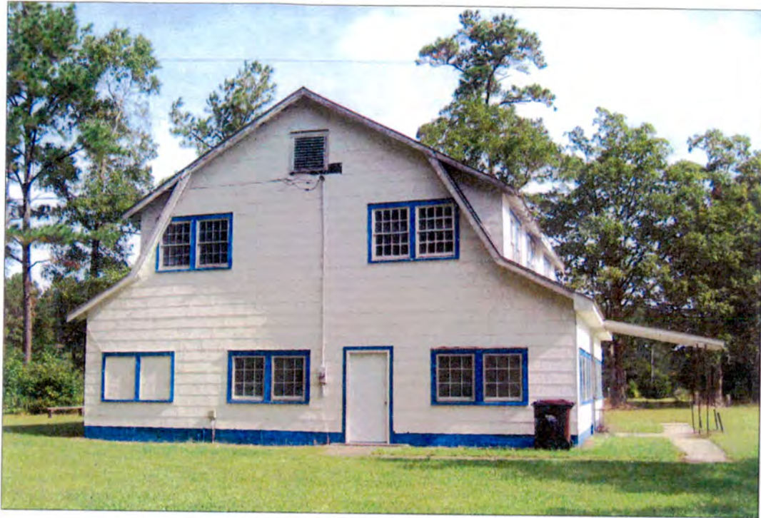
Figure 27, above: Albemarle Grill, south elevation
