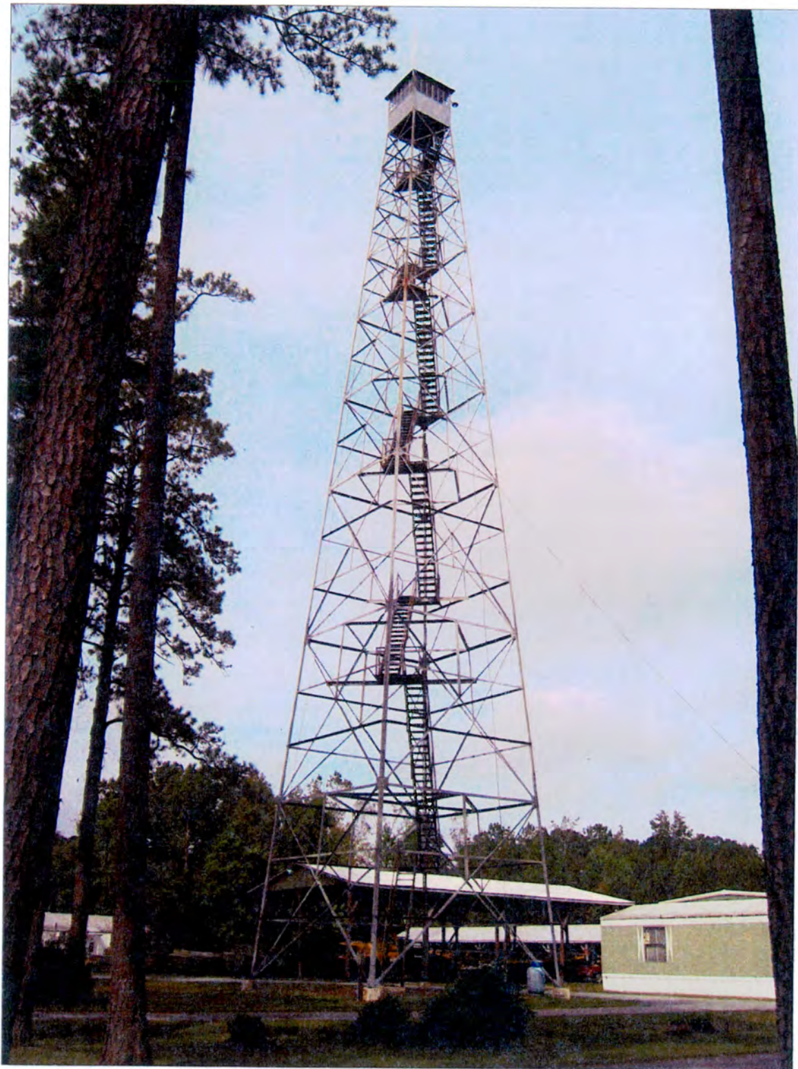
Figure 42, above: Scuppernong Tower, southeast corner
