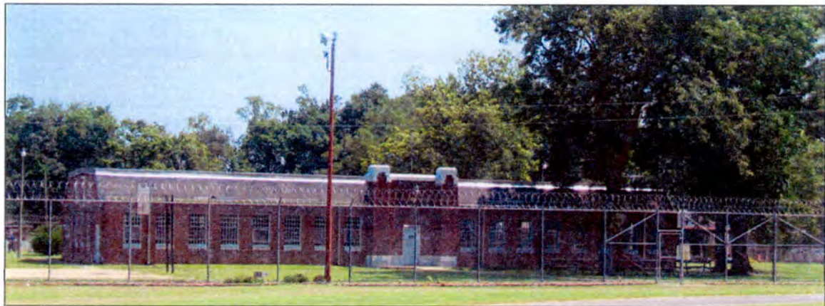
Figure 13: Washington County Prison Camp, main prison block, southwest elevation.
