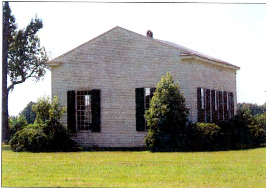
Figure 15: Rehoboth Methodist Church, north elevation.
