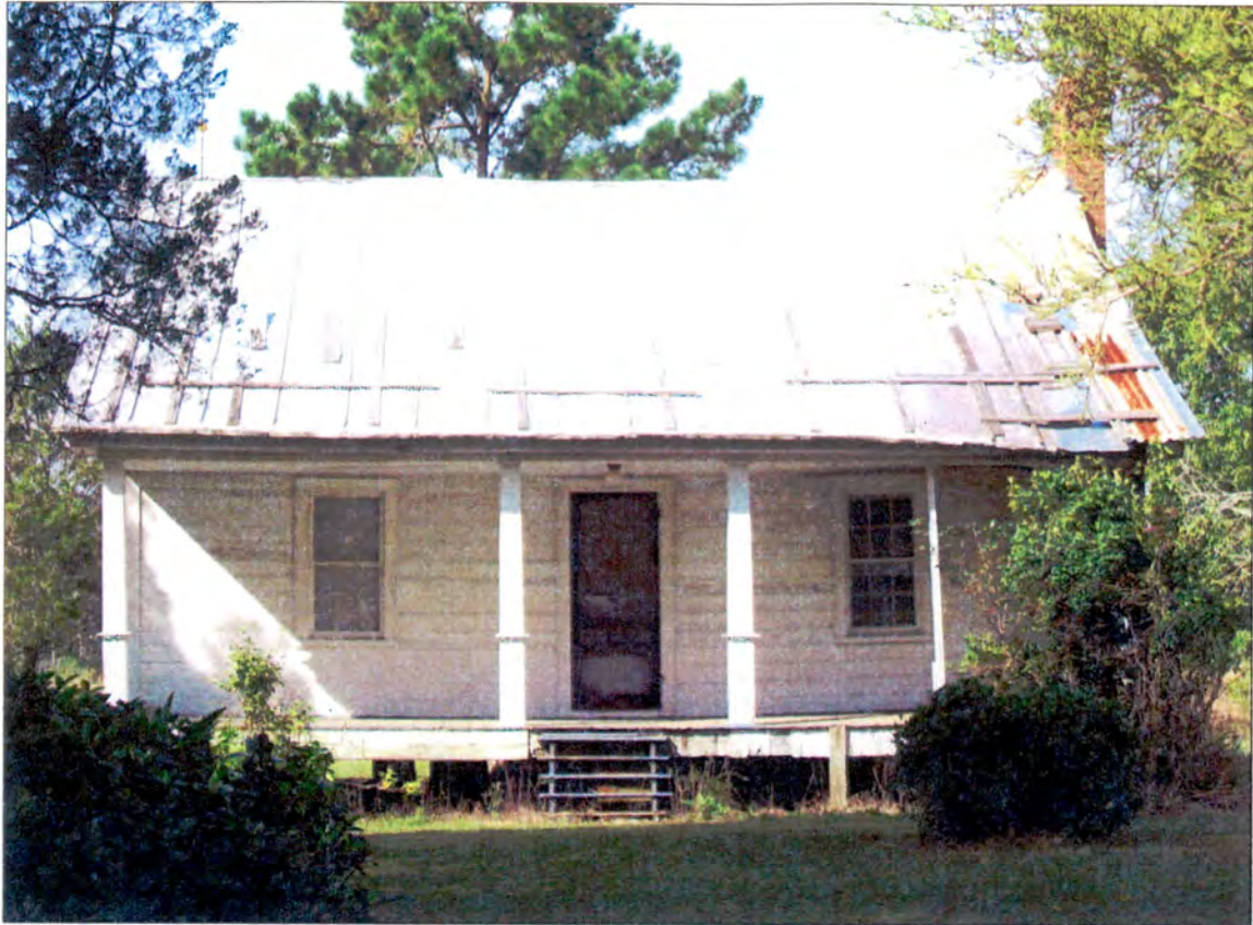
Figure 19, above: Hopkins House, east elevation
