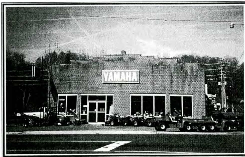
Figure 10 - Property No. 2- Lacks historical or architectural significance
