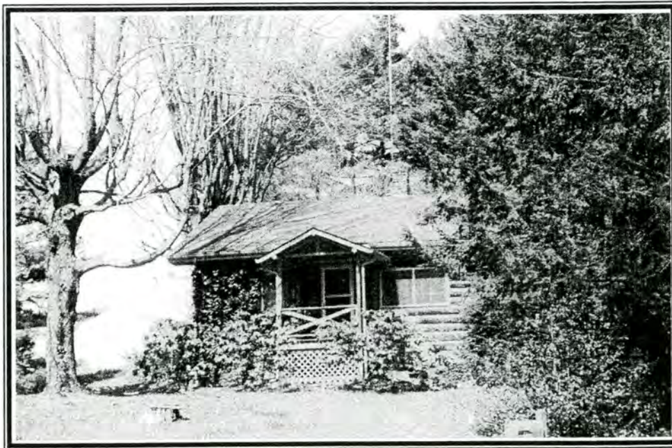
Figure 14 - Property No. 7- Lacks historical or architectural significance
