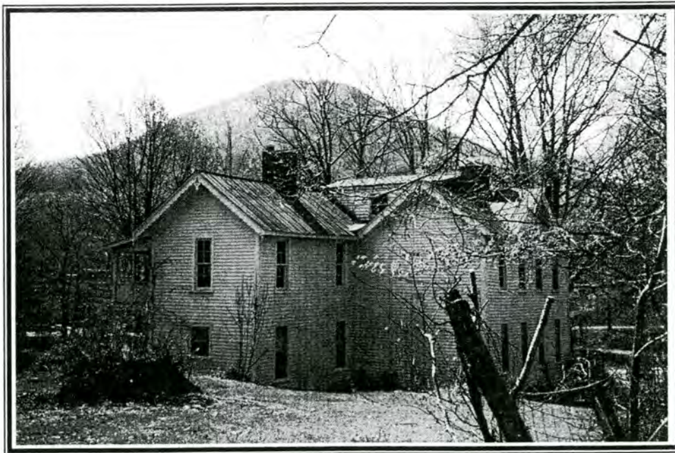
Figure 5 - Joseph Benjamin Neal House- North (Rear) and West Elevations
