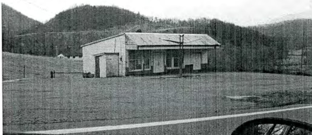
9.1 Gas Station (vacant), NC 18 west of SR 1193
