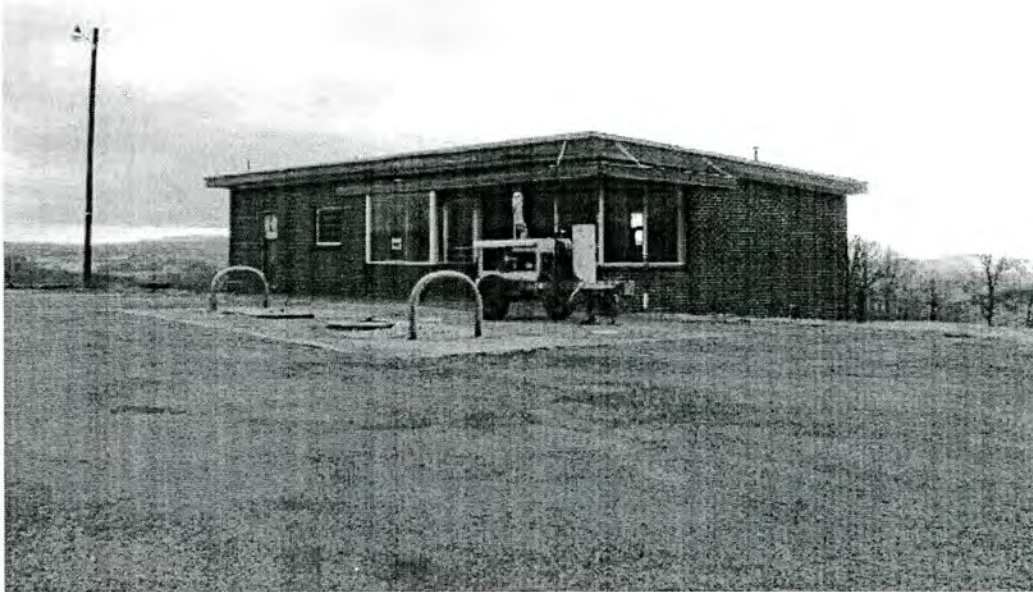
4.1 Gas Station (vacant), NC 18 east of SR 1433
