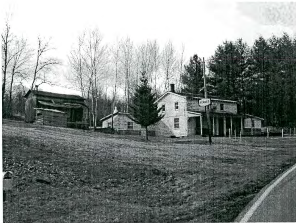
17.2 Hill's Grocery, Setting with residential and outbuildings
