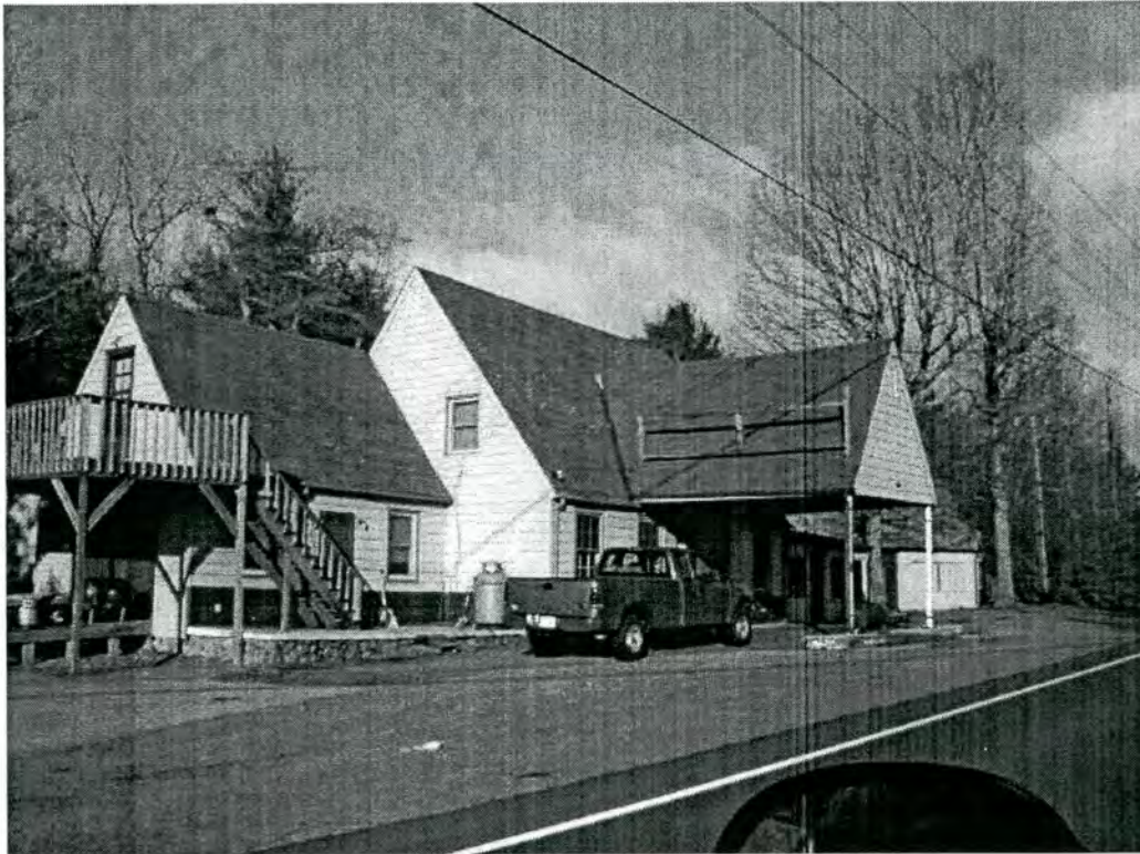
7.1 Gas Station (converted), US 21, north of SR 1106
