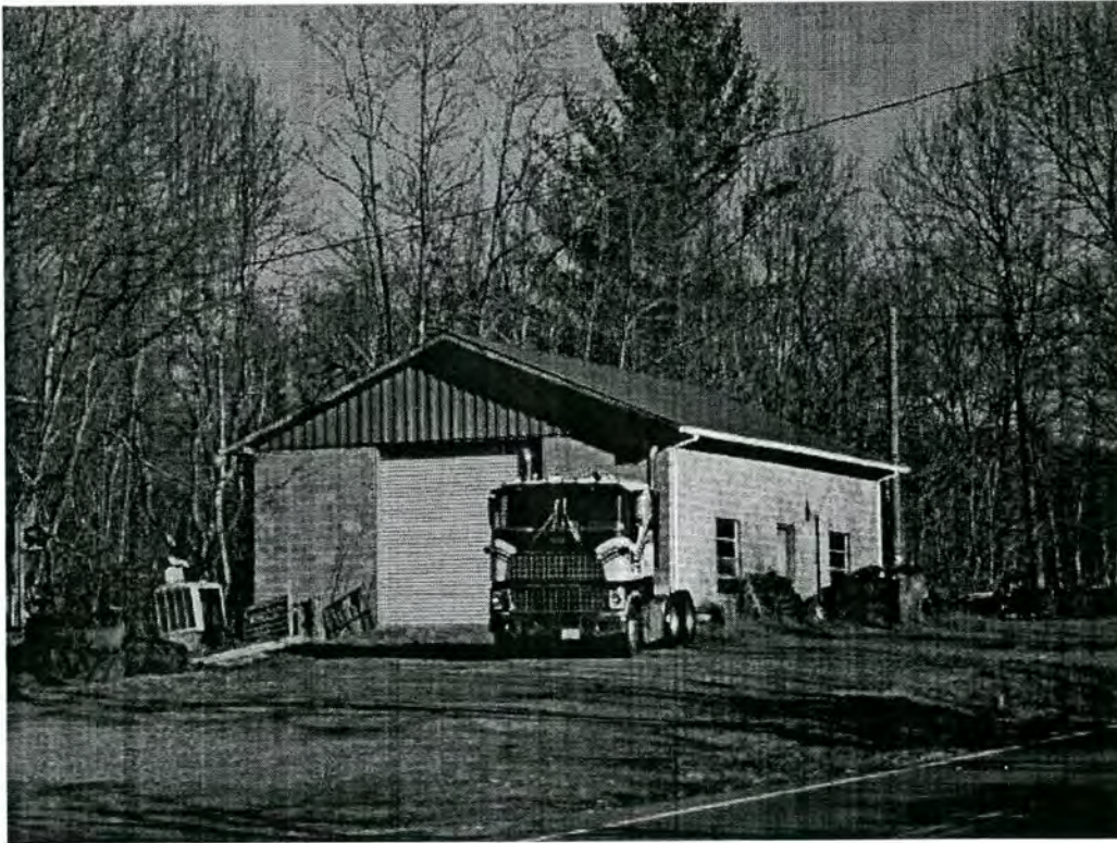
2.7 Edwards Property: Industrial building
