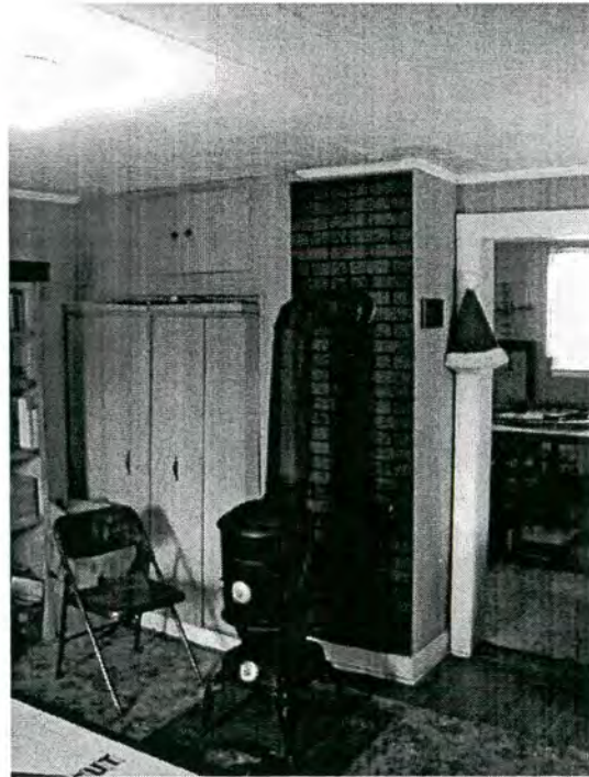
2.14 Spurling's Gas Station with interior additions/modifications showing added casework, non-original stove, and tiled ceiling concealing original materials.
