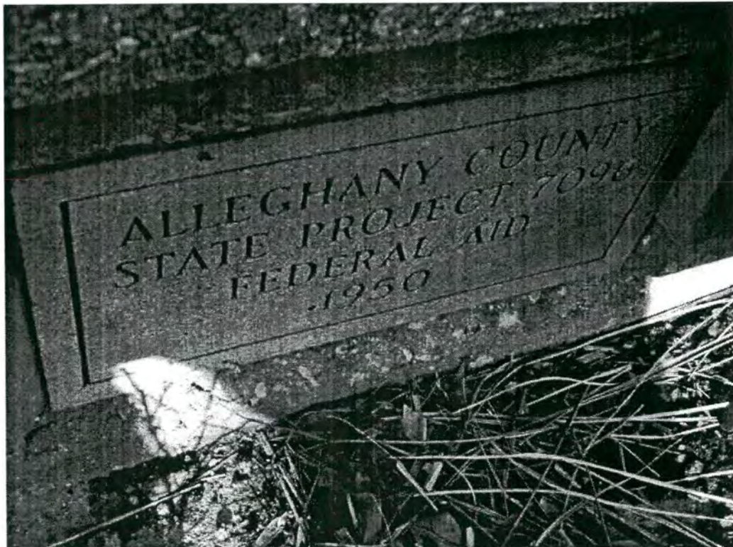
1.4 Bridge #38 (built 1950) on NC 18 over Crab Creek
