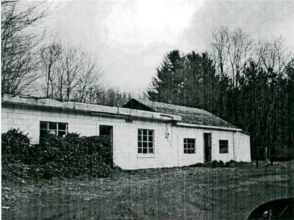
11.1 Finney's Grocery and Service (vacant), NC 18 west of SR 1142
