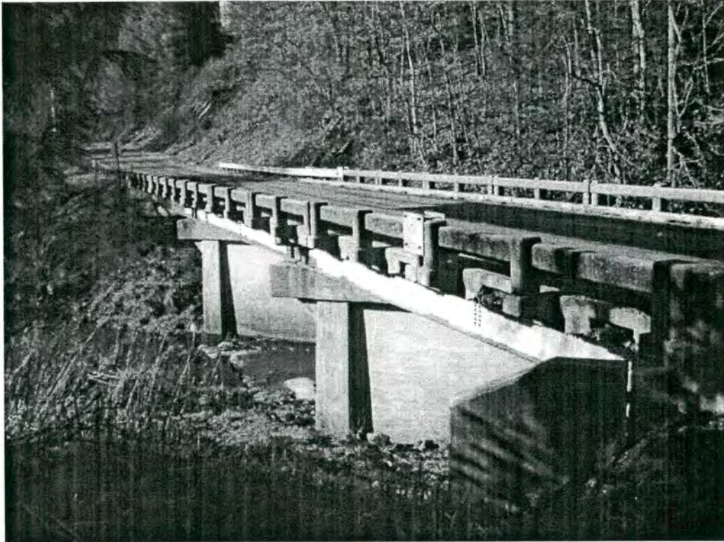
1.3 Bridge #38 (built 1950) on NC 18 over Crab Creek
