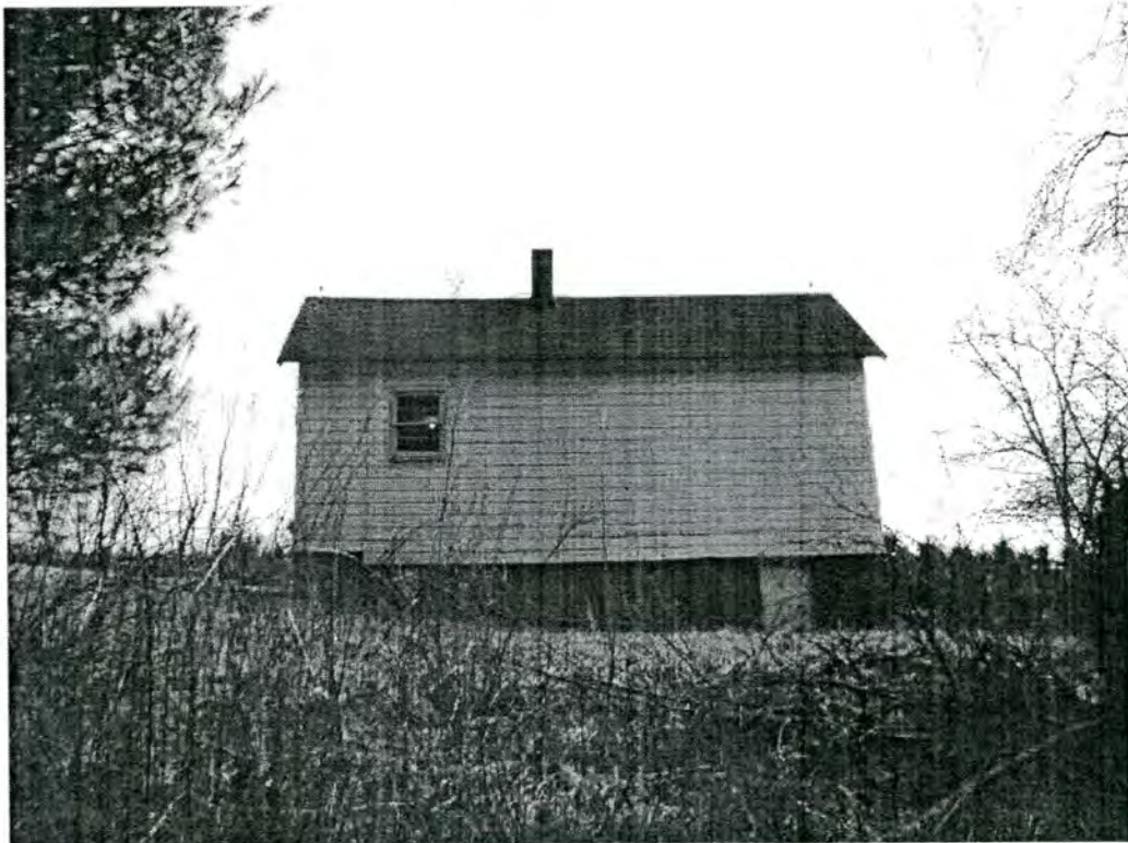
2.11 Edwards Property: Spurling's Gas Station- side and rear elevations
