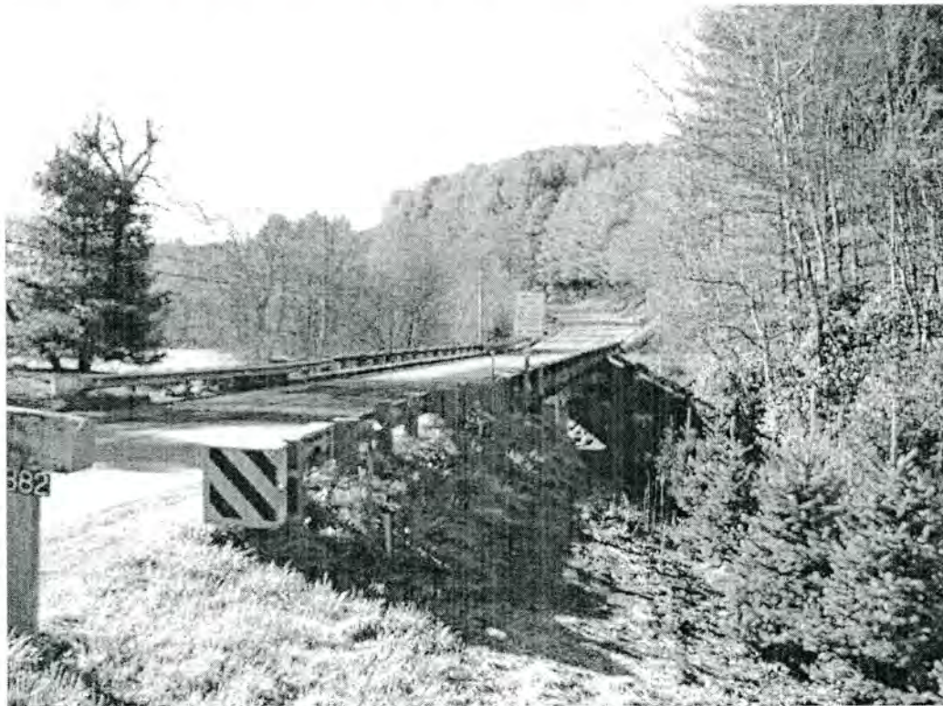
1.2 Bridge #38 (built 1950) on NC 18 over Crab Creek
