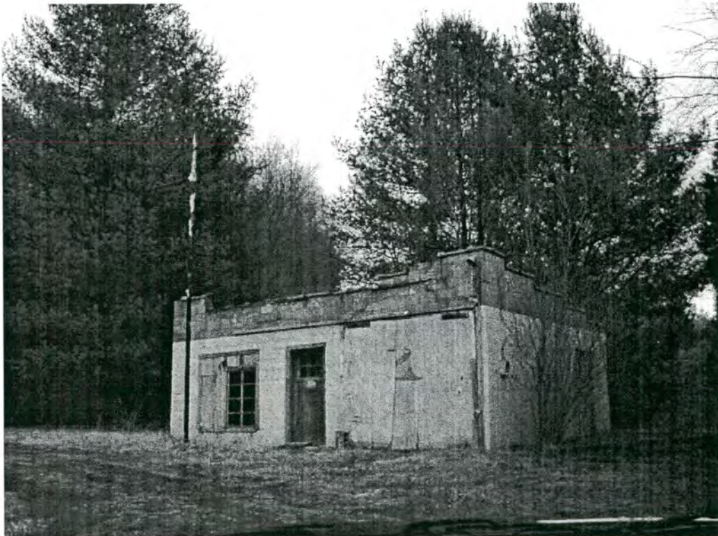
14.1 Gas Station (vacant), NC 113 north of SR 1153
