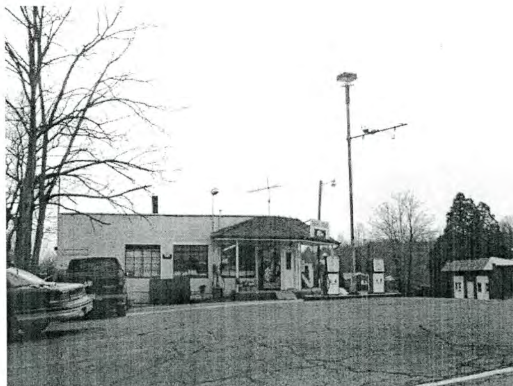
16.1 Pugh's Store, NW corner of NC 93 and SR 1317
