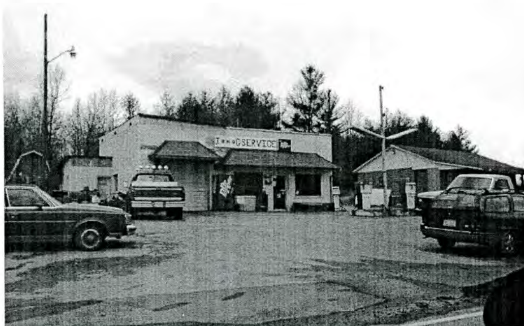
15.1 J & C Service, NC 113 south of SR 1316
