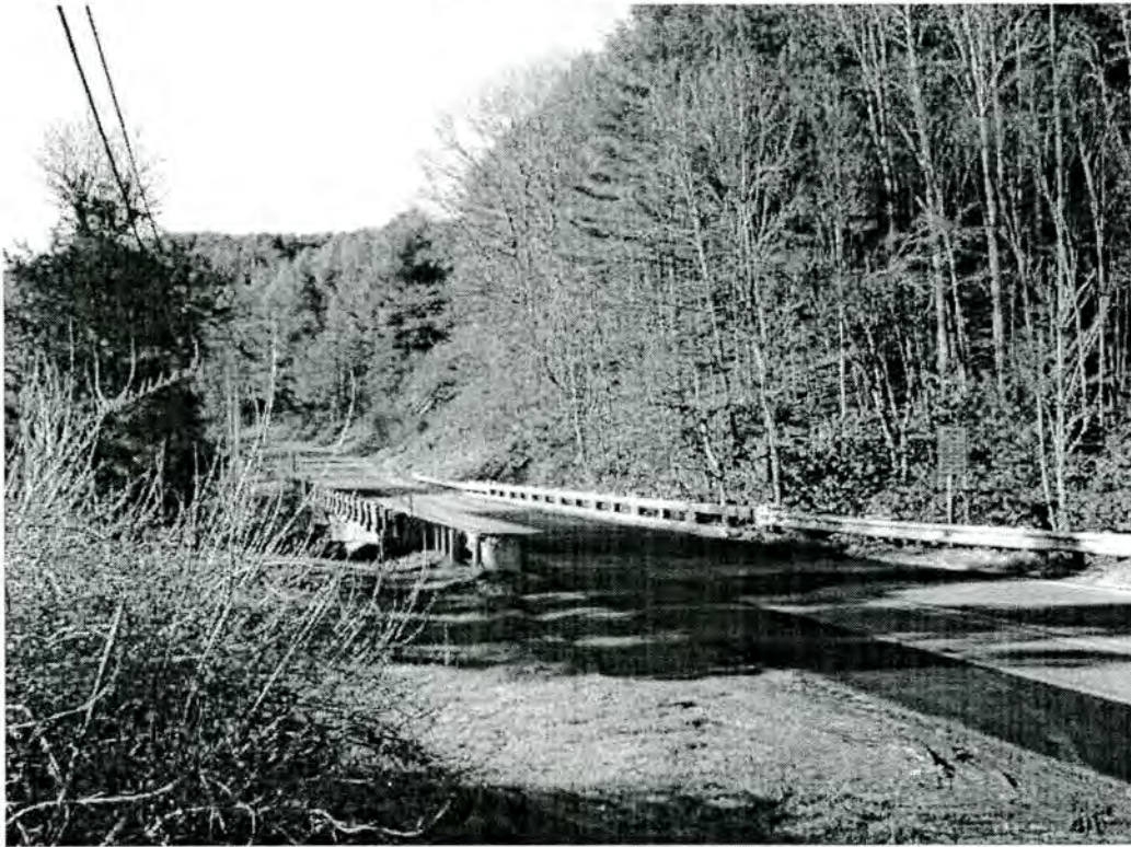
1.1 Bridge #38 (built 1950) on NC 18 over Crab Creek
