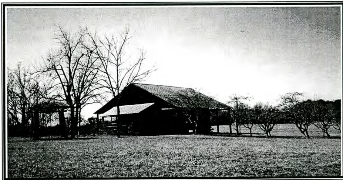
Figure 9 - Barn in large complex of outbuildings, SR 2414, Reidsville
