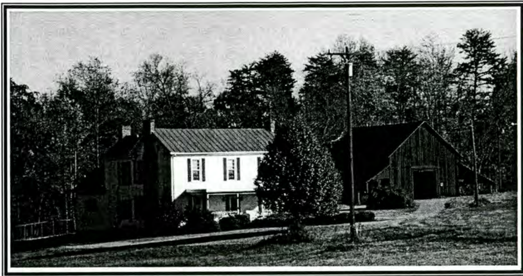
Figure 2 - Trent House and Barn
