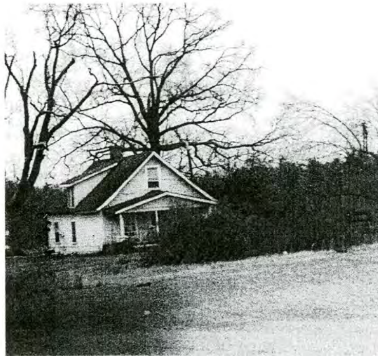
Figure 34: Property # 9 – House (McAtter Farm)
