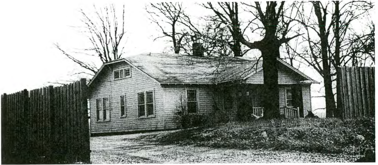
Figure 22: Property # 21 – A. M. Secret House North (front) and east (side) elevations. Photographed April 4, 2001.
