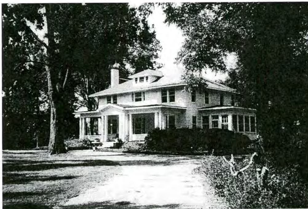
Figure 6: Property # 28b – The Waxhaw-Weddington Historic District The Ed Crow House. Photographed September 11, 2001.
