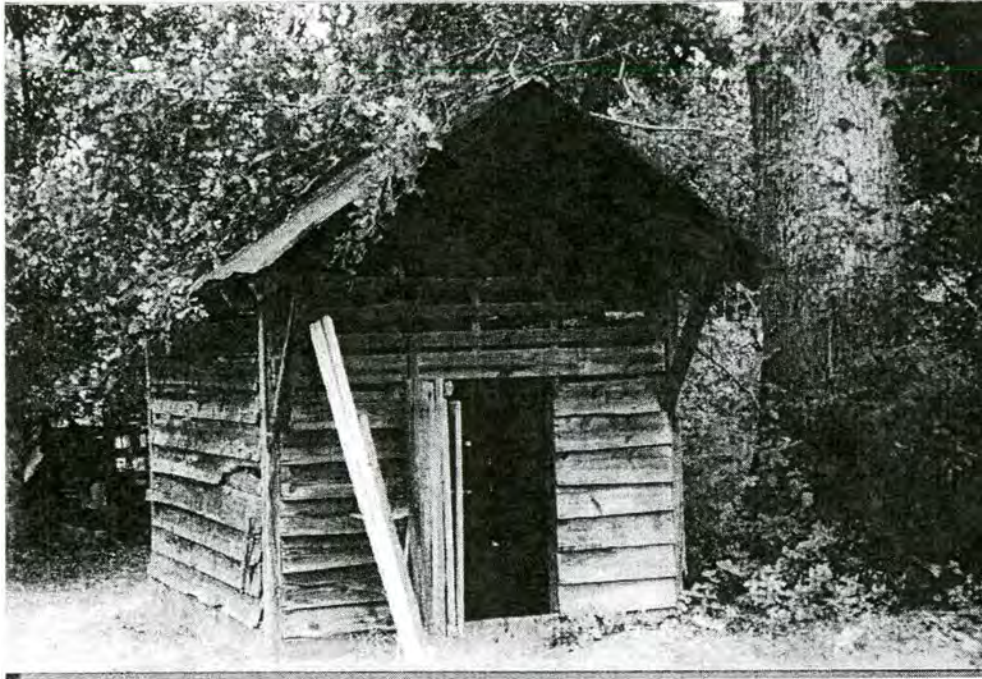
Figure 19: Property # 5 – C. L. Helms Tenant House Outbuilding. Photographed September 11, 2001.
