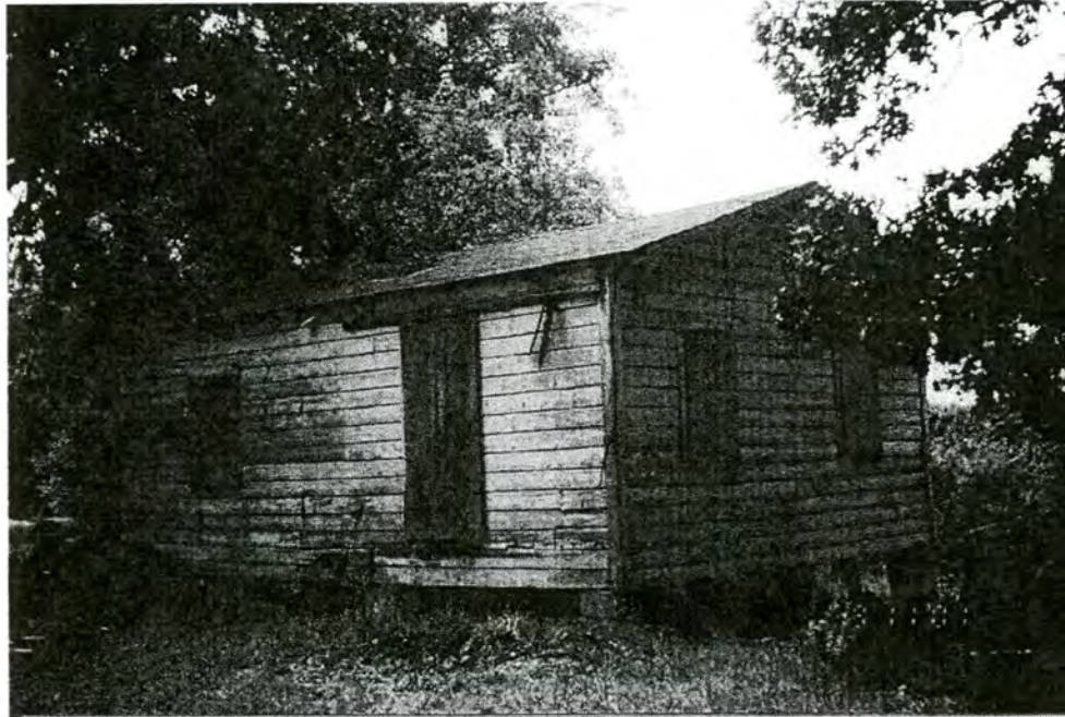
Figure 20: Property # 5 – C. L. Helms Tenant House Outbuilding.
