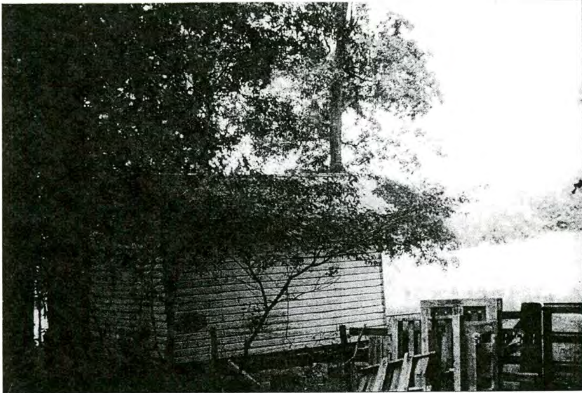
Figure 21: Property # 5 – C. L. Helms Tenant House Outbuilding. Photographed September 11, 2001.
