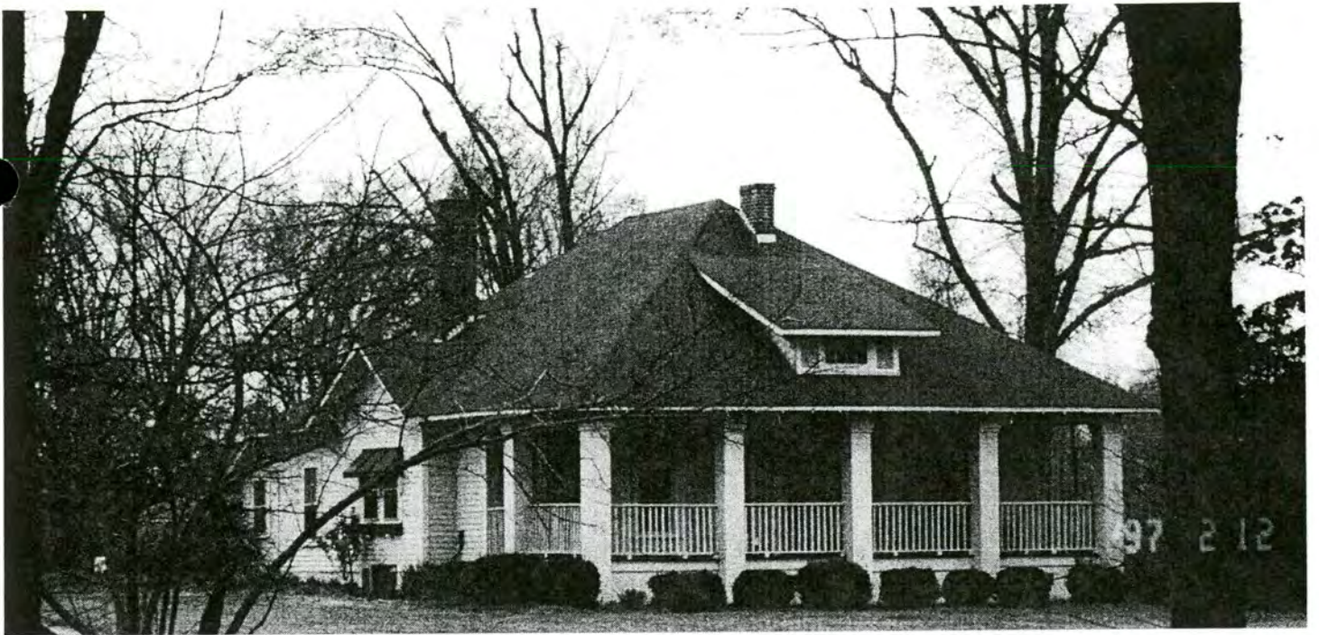
Figure 11: Property # 16 – The Robert Ney McNeely House North (front) and east (side) elevations. Photographed April 4, 2001.
