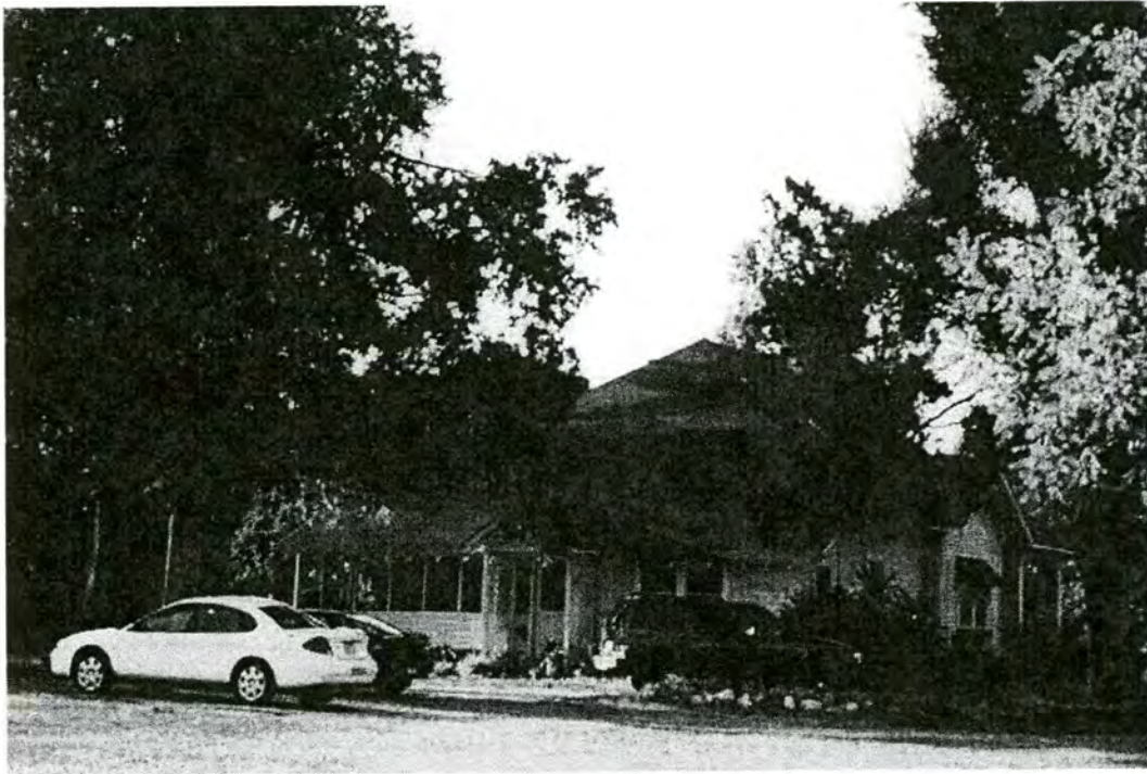
Figure 12: Property # 16 – The Robert Ney McNeely House South (back) and east (side) elevations. Photographed August 22, 2001
