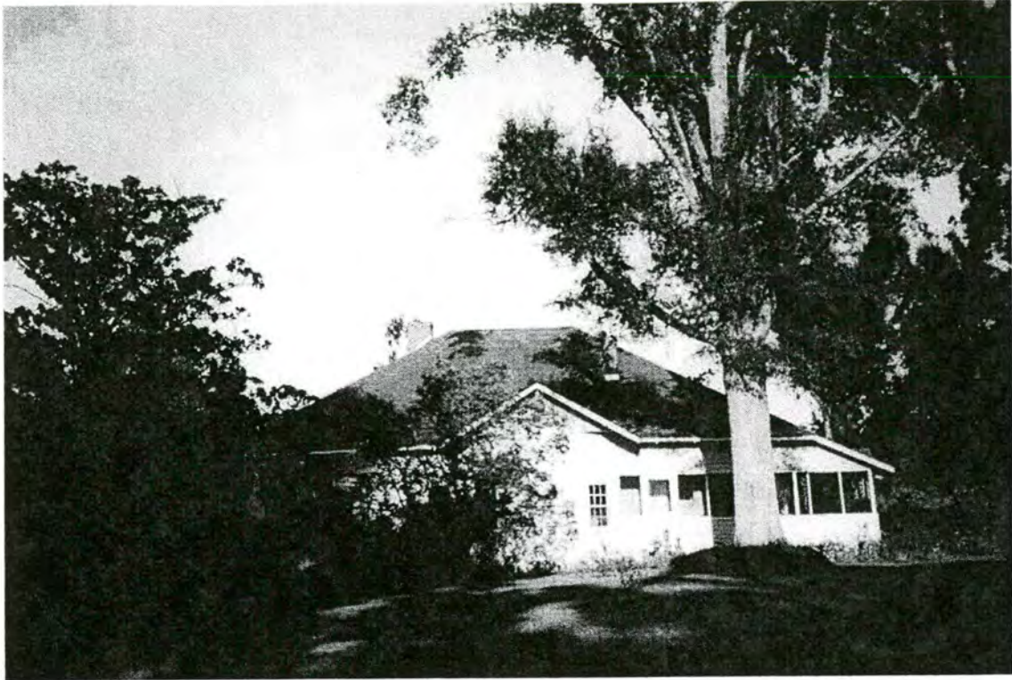
Figure 13: Property # 16 – The Robert Ney McNeely House West elevation. Photographed August 22, 2001
