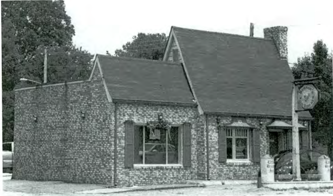
Pure Oil Filling Station (Property 3) South and West Elevations
