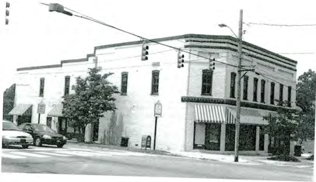
Stevens Building (Property 6) South and East Elevations
