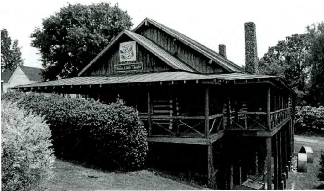
American Legion Hall (Property 2) North Elevation
