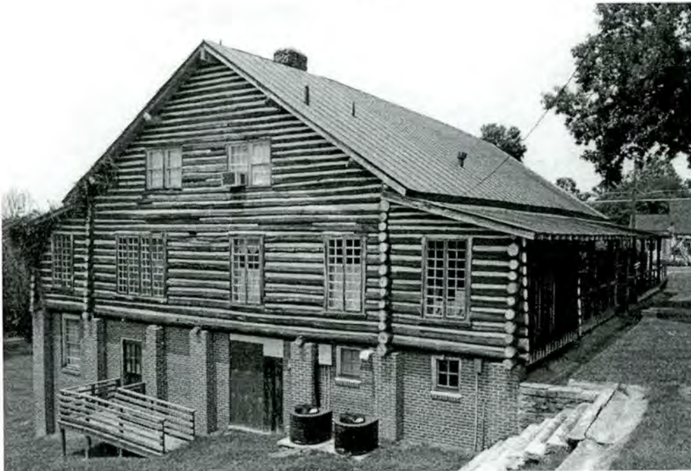
American Legion Hall (Property 2) South and East Elevations
