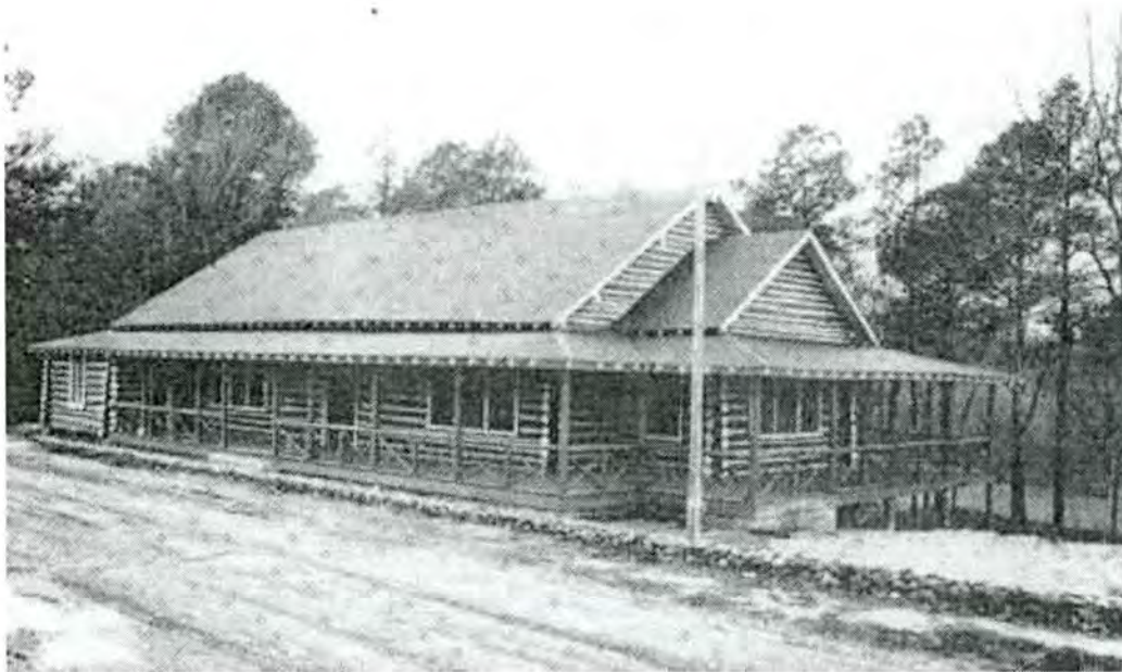
Photograph of American Legion Hall circa 1935 North and East Elevations (from Emergency Relief in North Carolina , p. 226)
