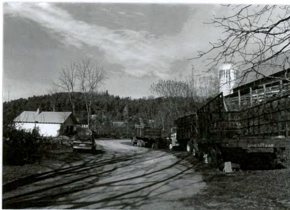
4. View of Riverside store (left) and main farm complex (right)
