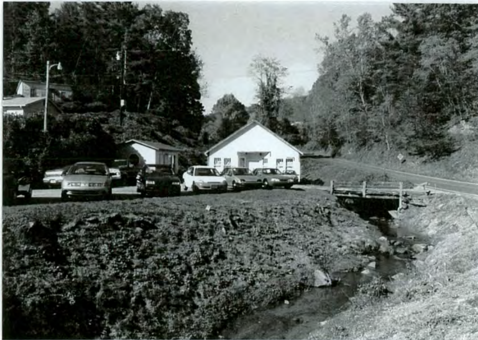
2. View of store and Shoal Creek from US 19E looking north
