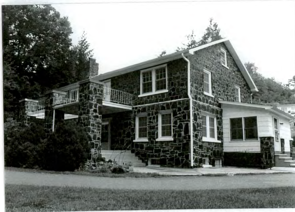
4. North front and west side facades
