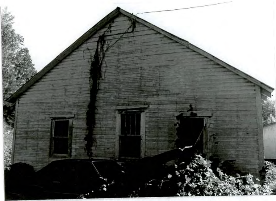
8. North rear facade
