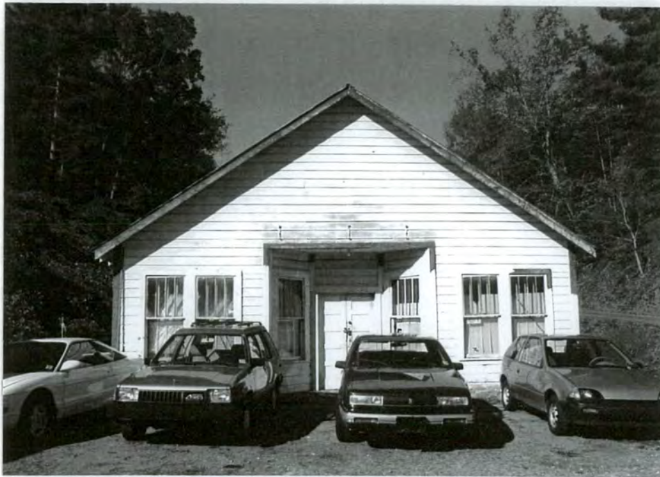
4. South front facade
