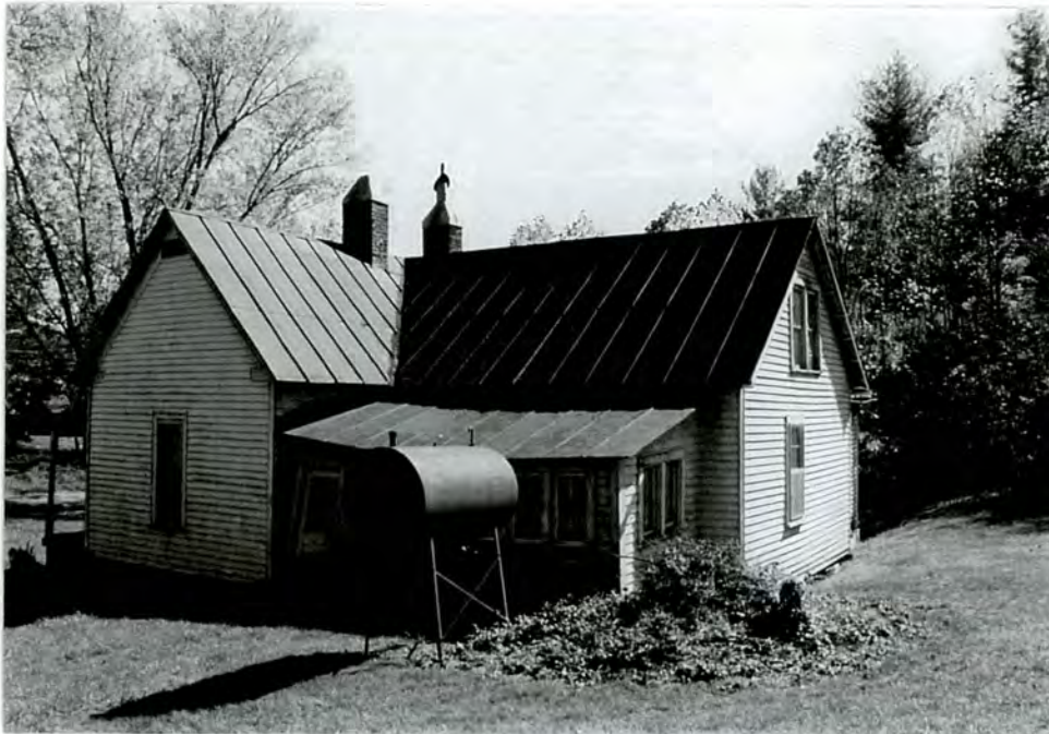
12. North side facade showing added shed porch
