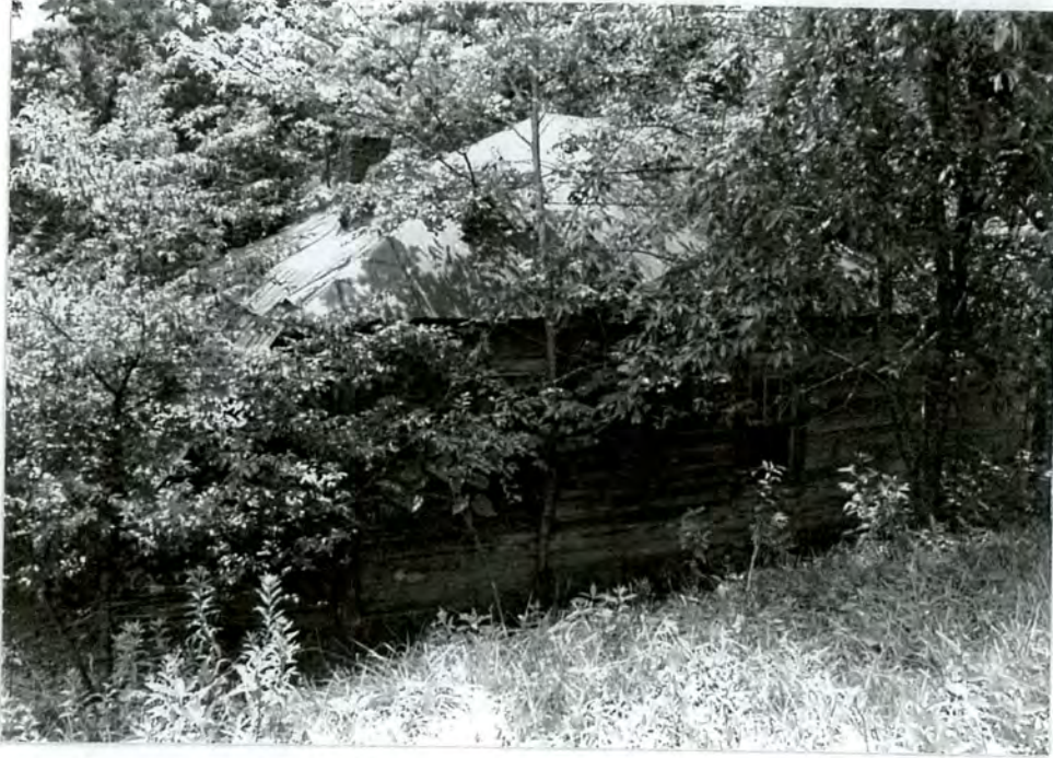
17. Rear facade of 1910s farm house
