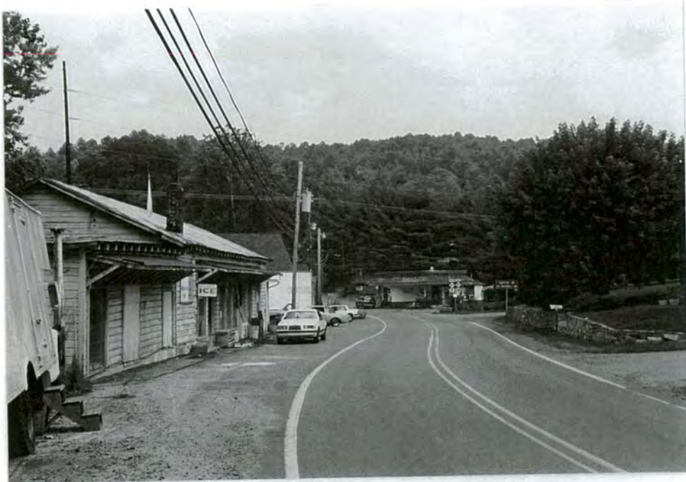
7. View down SR 1186 toward intersection with NC 80, looking southeast
