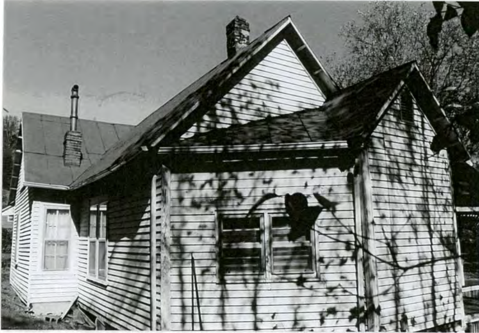
9. South side and west rear facades showing nonhistoric infill
