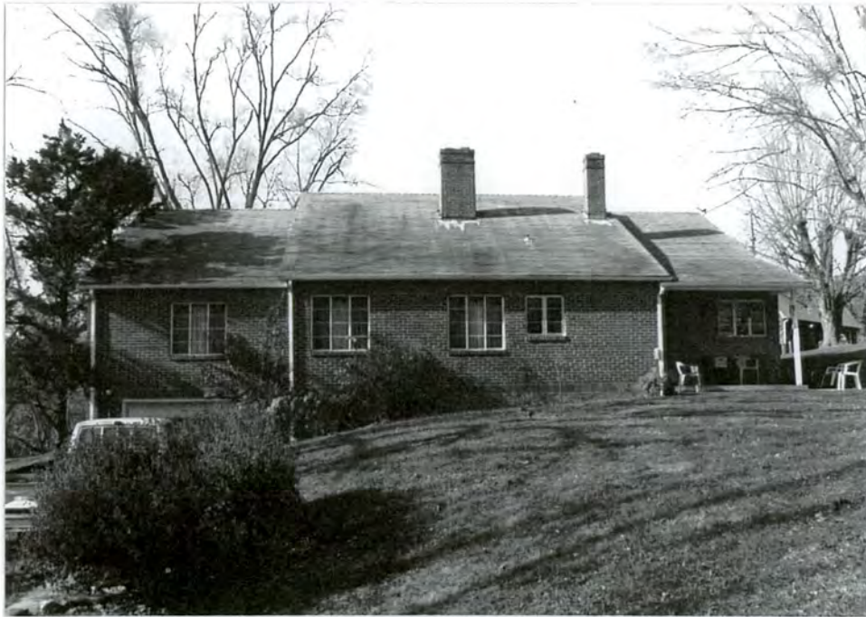
10. Rear facade of 1950s brick farm house
