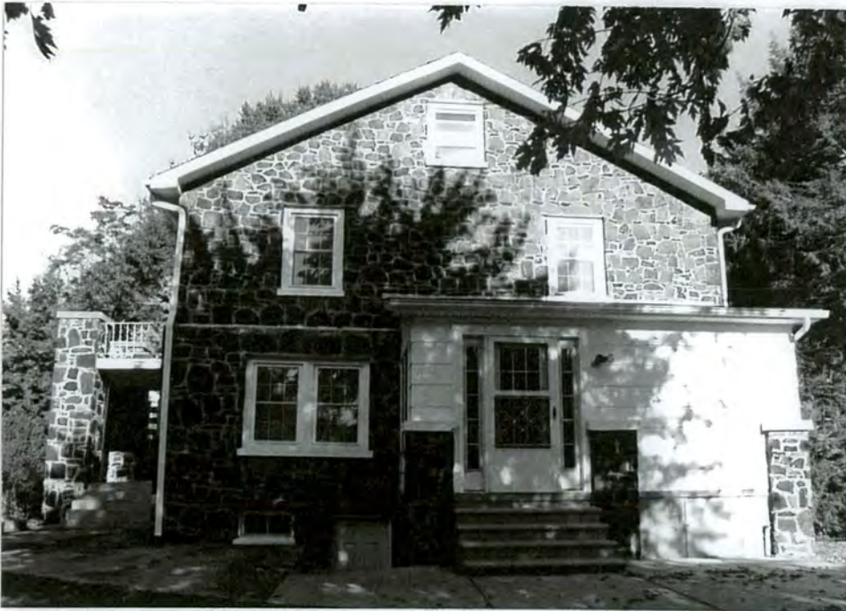
12. West side facade with enclosed side porch
