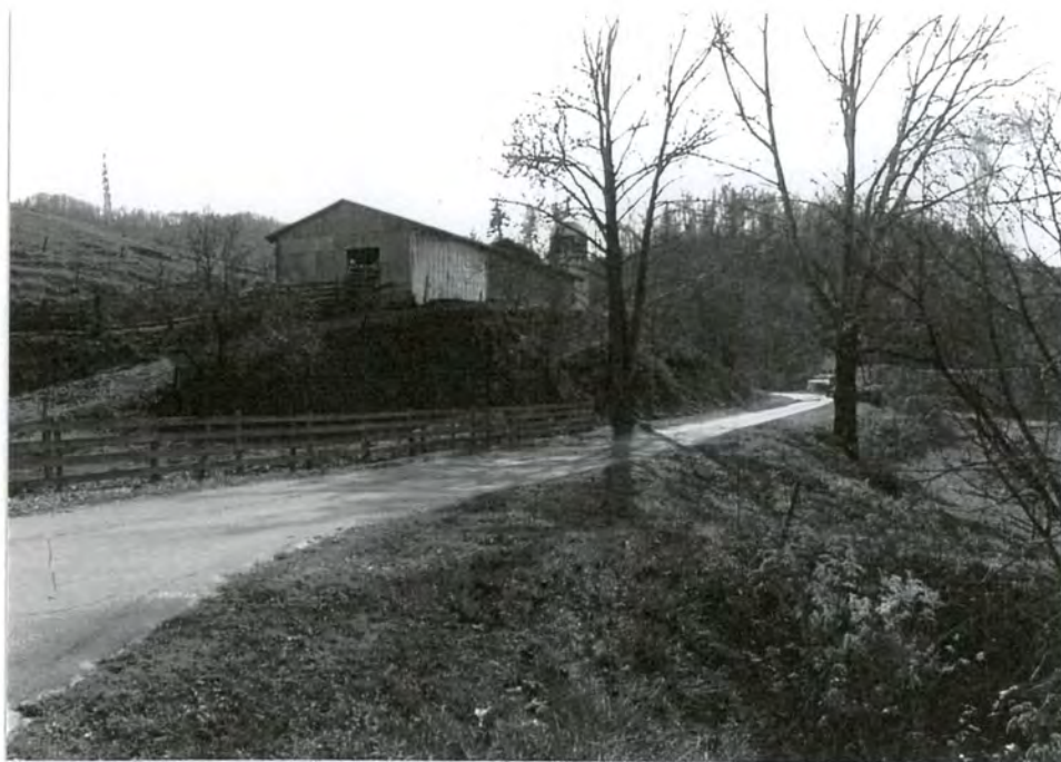
3. View of main farm complex from farm entrance road
