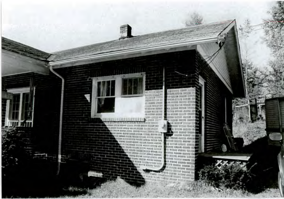
7. North rear facade
