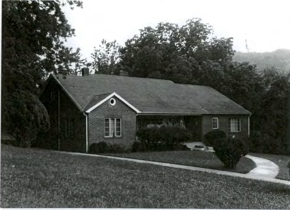
9. Front facade of 1950s brick farm house
