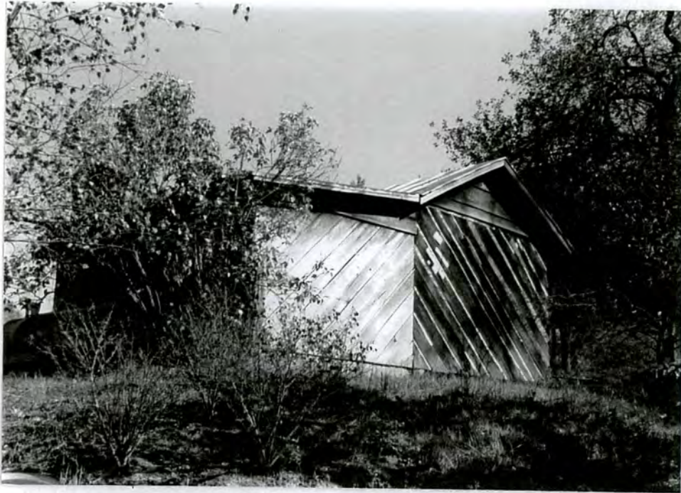
13. Frame storage building
