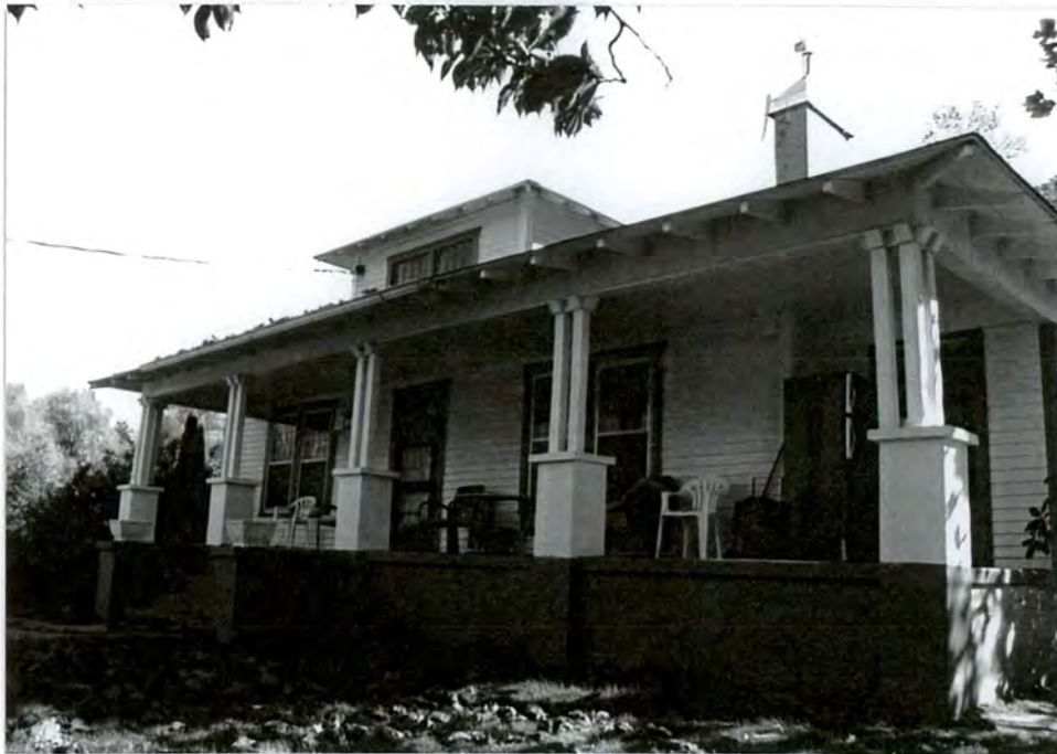
6. North front facade and front porch
