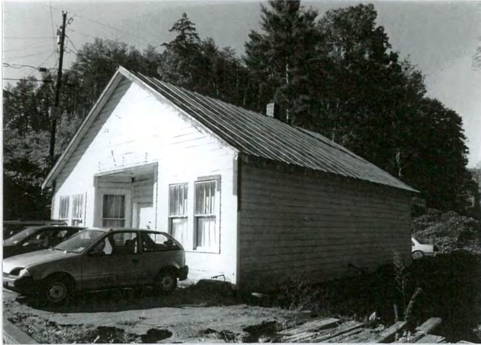
6. South front and east side facades
