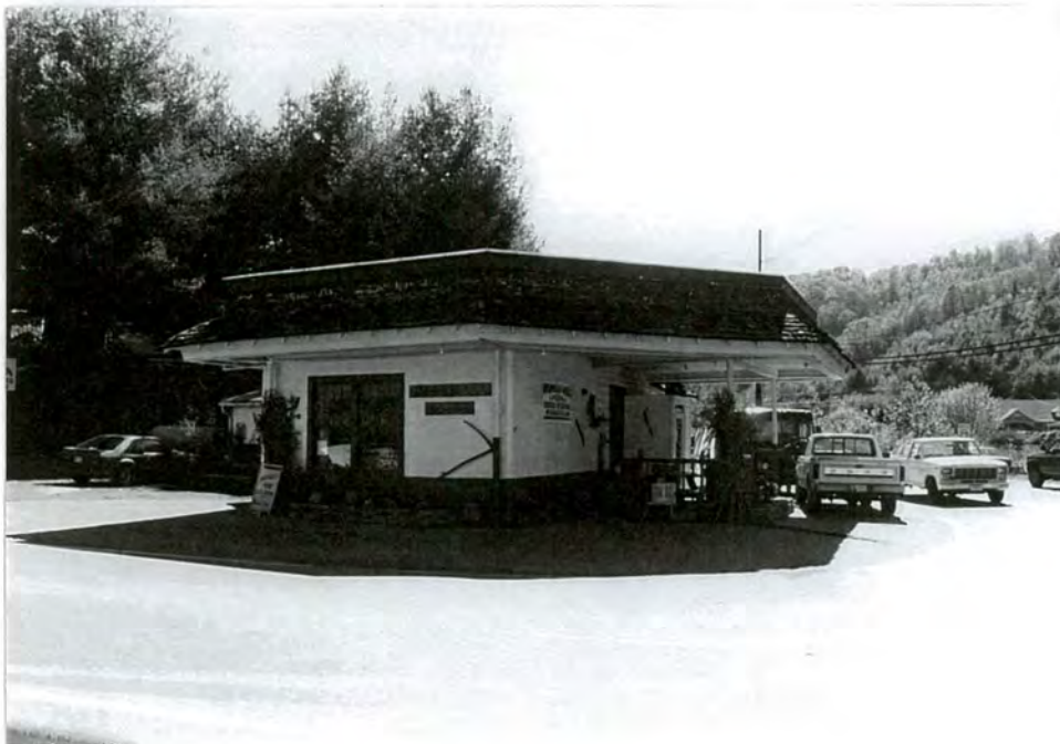
12. Former gas station showing canopy
