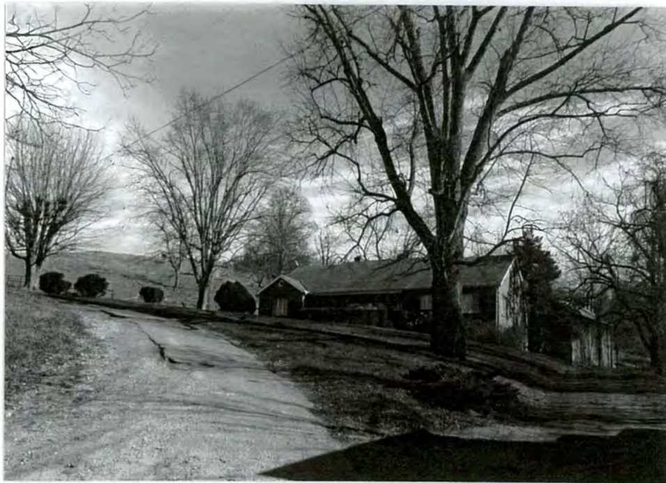
8. View of 1950s brick farm house
