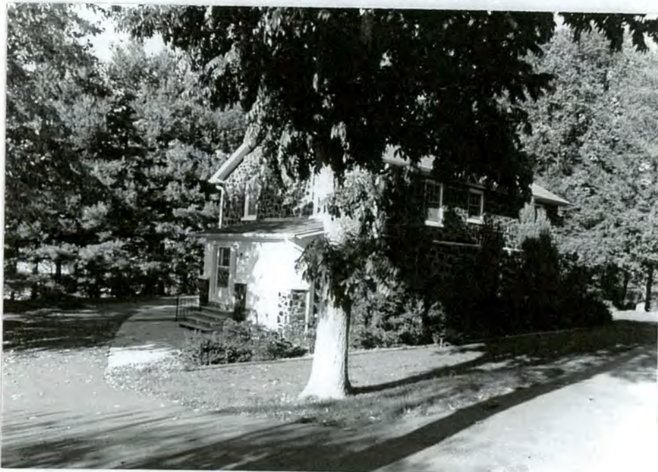
2. View of rear facade from Pineola Street
