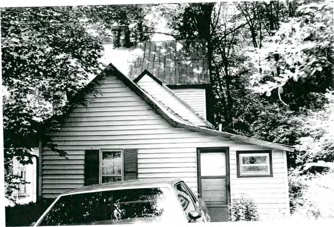
Plate 41: R.L. Young House – east rear elevation
