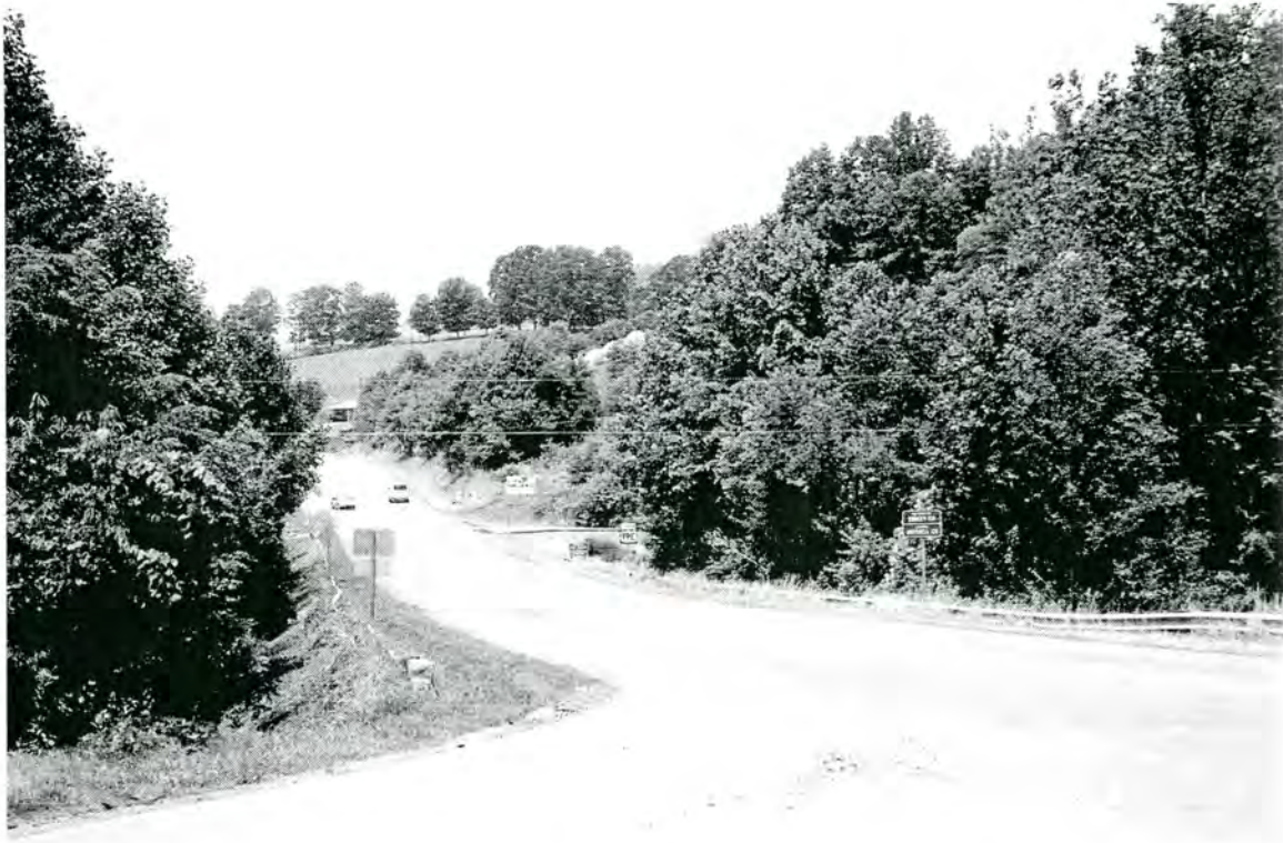
Plate 5: Looking northwest along US 19E at Big Crabtree Creek/Yancey-Mitchell county line
