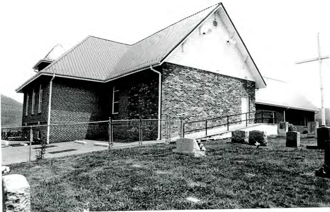
Plate 56: Liberty Hill Baptist Church – north rear and west side elevations
