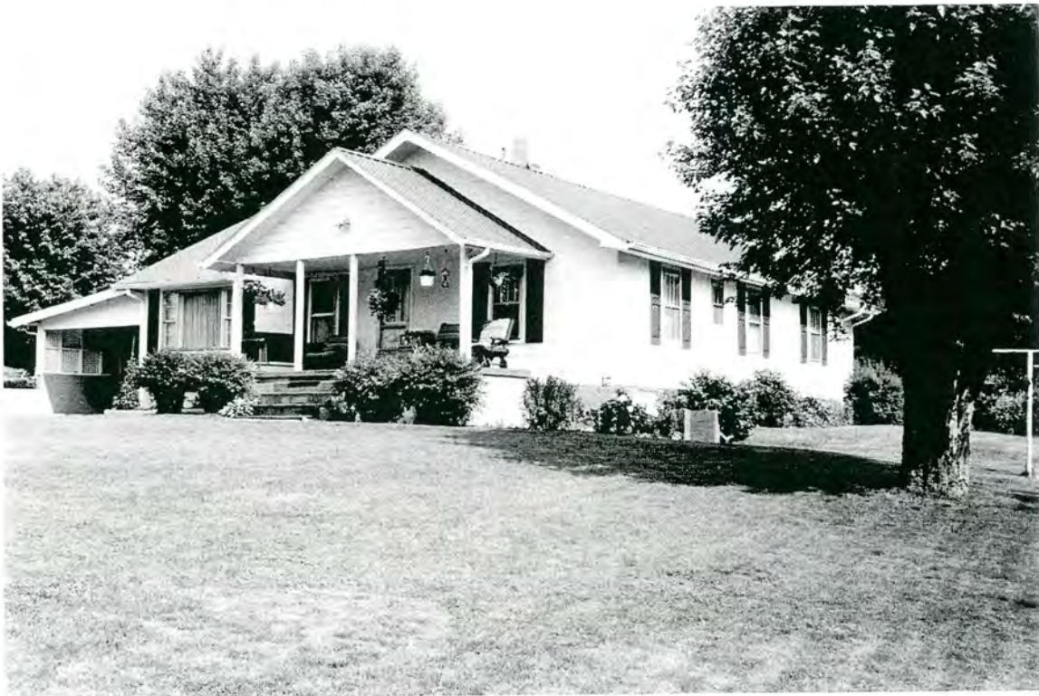
Plate 60: House (#2) – south front elevation of house at 5347 US 19E, Newdale, Yancey County
