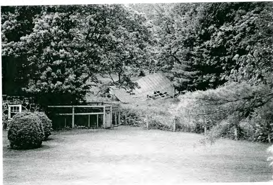
Plate 20: E.W. and Dollie Huskins House – looking southeast across lawn toward stone shed, fence, and collapsed outbuilding
