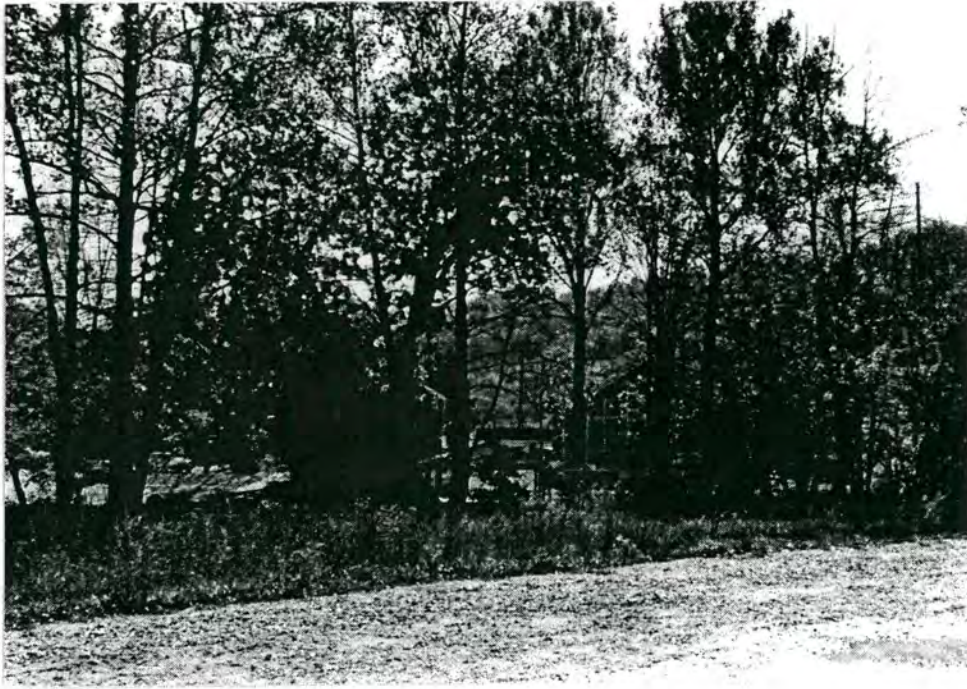
3. View of rear of Harris Clay Company Office from US 19E, looking south
