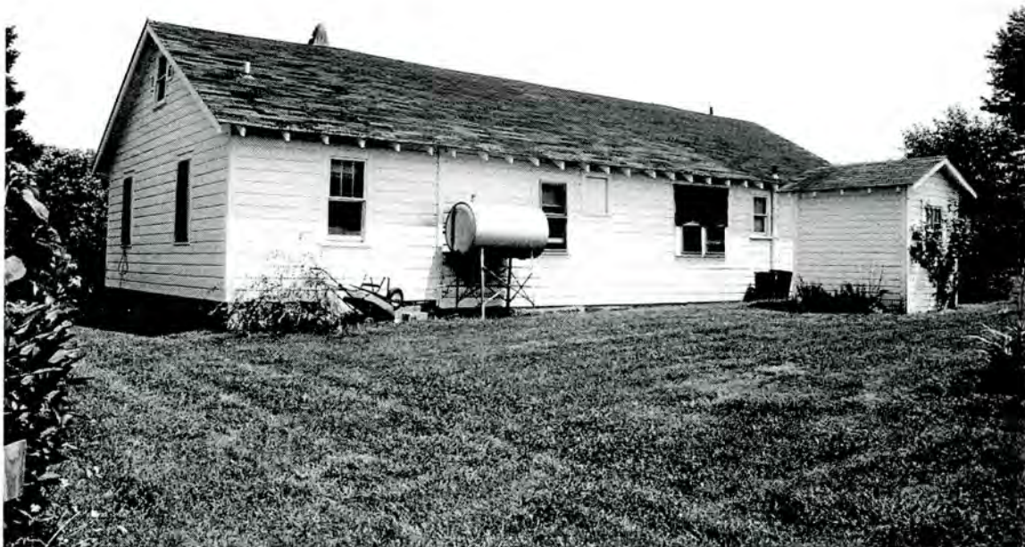
Plate 24: C. Lee and Herma Howell House – west rear and north side elevations; shed at far right
