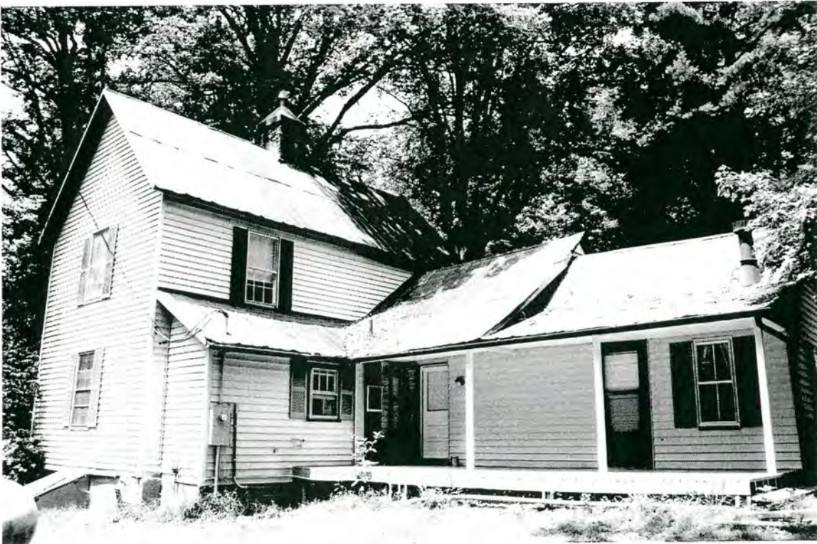
Plate 40: R.L. Young House – south side and east rear elevations
