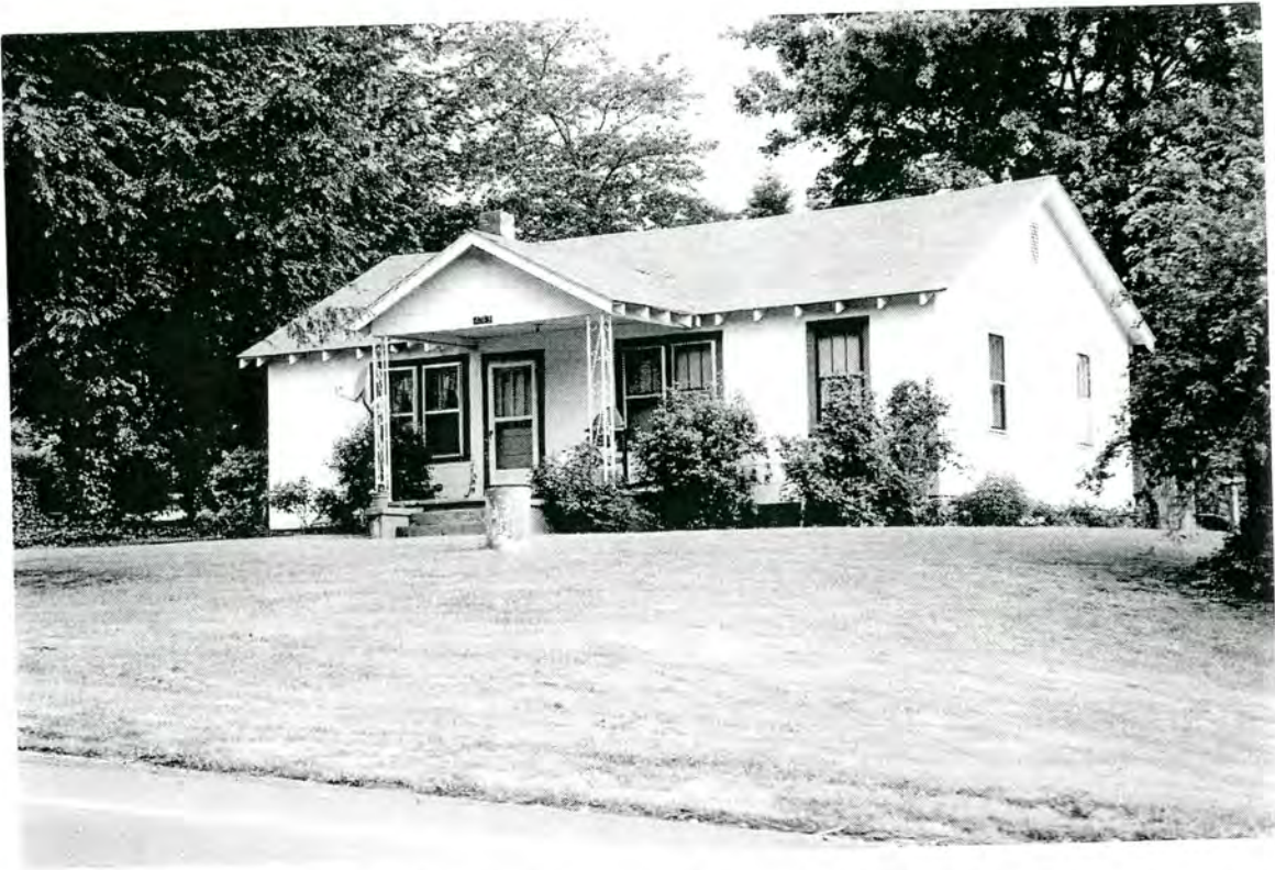
Plate 59: House (#1) –south front elevation of house at 4743 US 19E, Newdale vicinity, Yancey County
