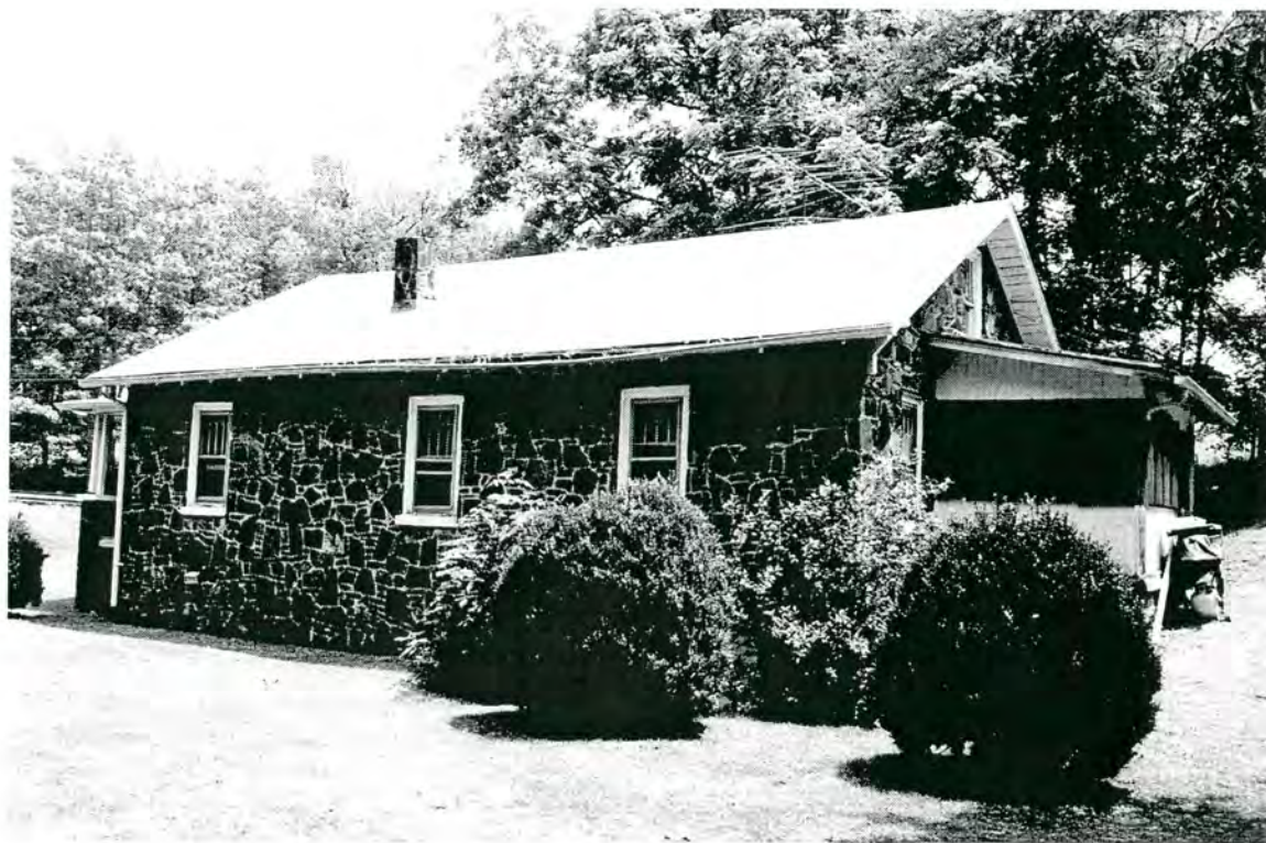
Plate 16: E.W. and Dollie Huskins House – south rear and west side elevations
