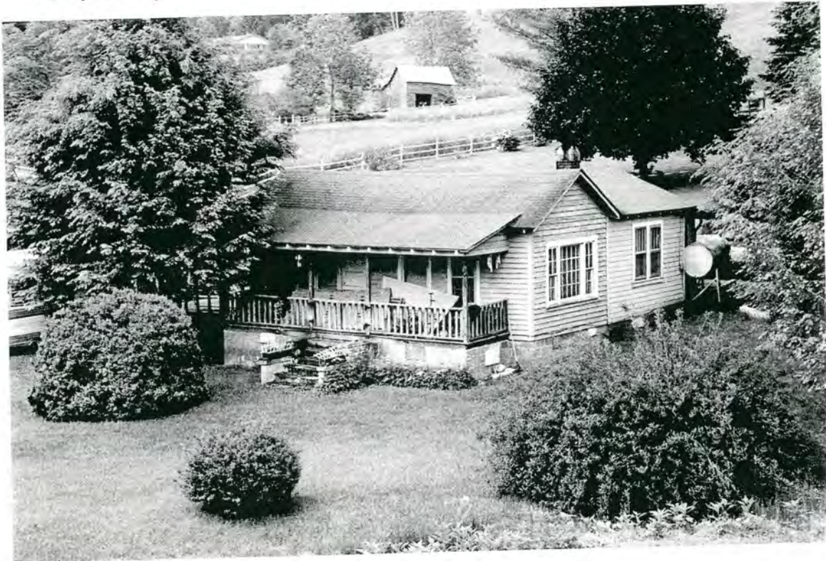
Plate 74: House (#21) – north front elevation of house on north side of Hemlock Road, 0.1 mile east of junction with US 19E, Estatoe vicinity, Yancey County
