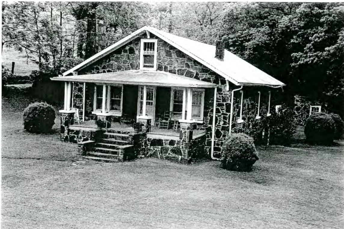
Plate 13: E.W. and Dollie Huskins House – north front and west side elevations; stone shed at far right
