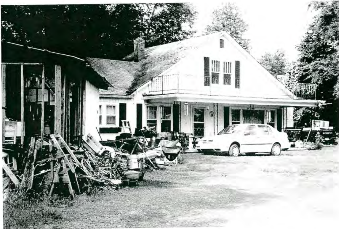
Plate 62: House (#4) – north front elevation of house south side of US 19E, 0.05 miles west of junction with Hicks Road, Newdale, Yancey County
