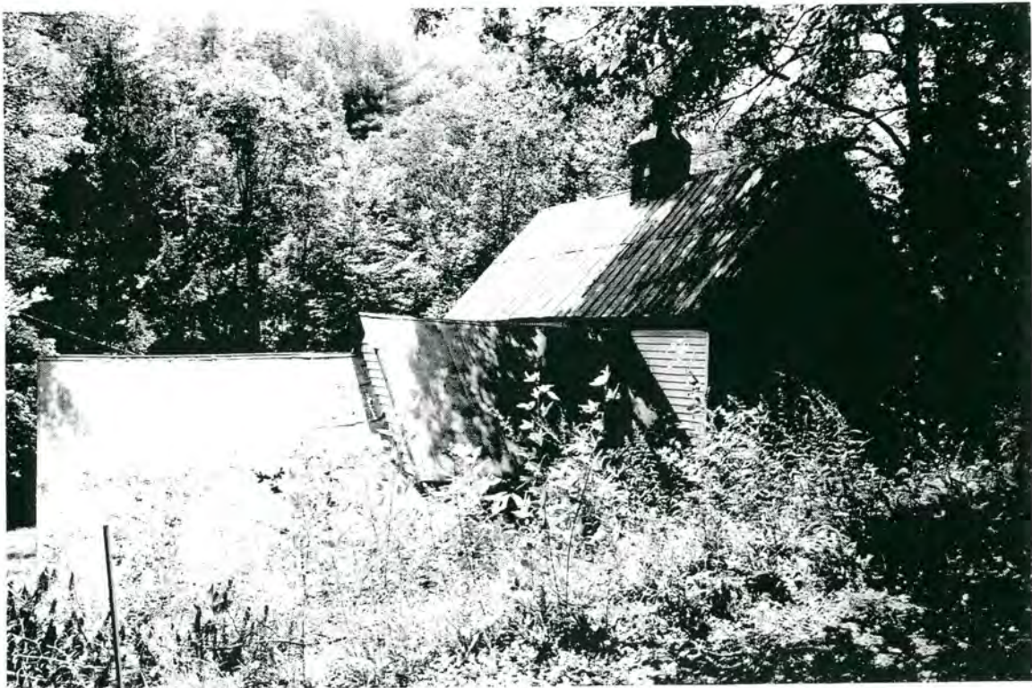
Plate 42: R.L. Young House – north side elevation
