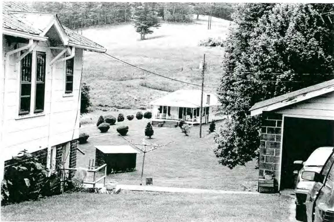
Plate 6: Looking south from US 19E toward House (#19), at left, and House (#20), at center
