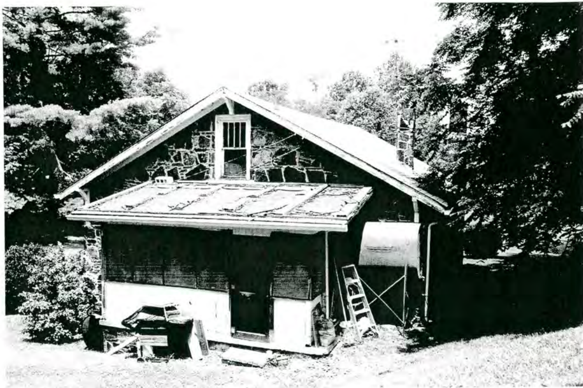
Plate 15: E.W. and Dollie Huskins House – east side and south rear elevations
