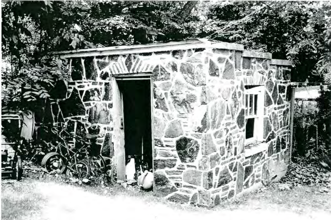
Plate 17: E.W. and Dollie Huskins House – east front and north side elevations of stone shed
