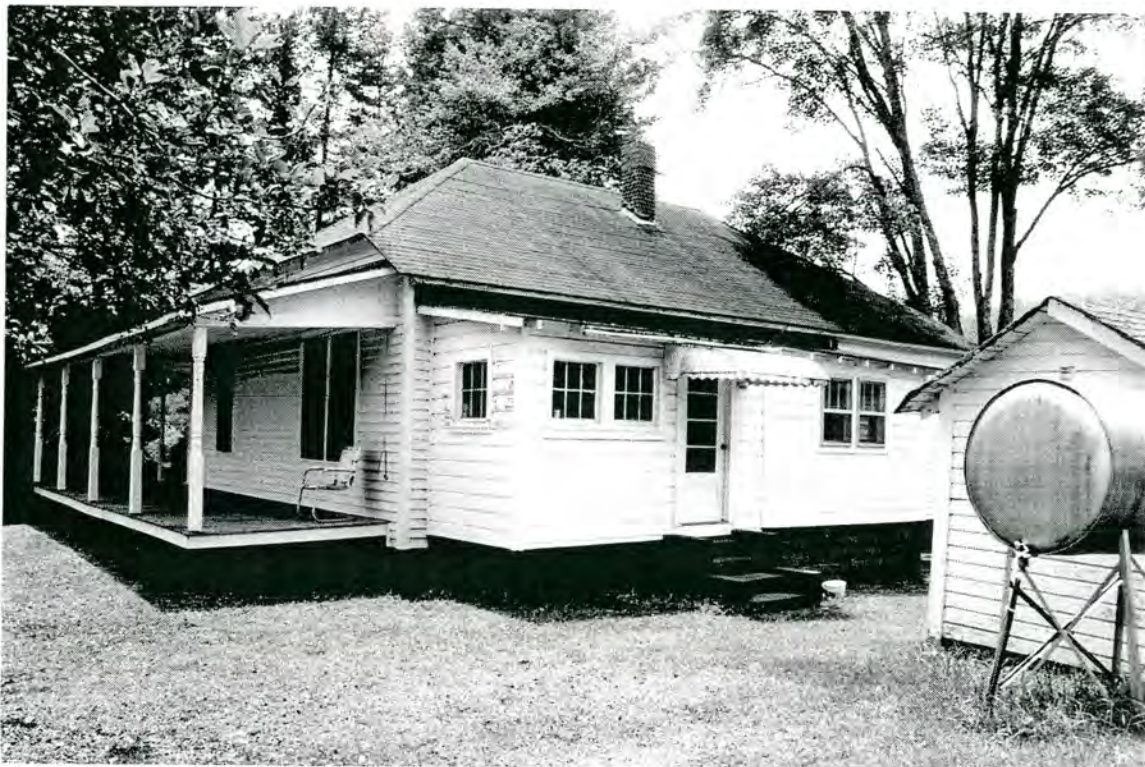
Plate 47: Lattie and Nora Young House – north rear and east side elevation
