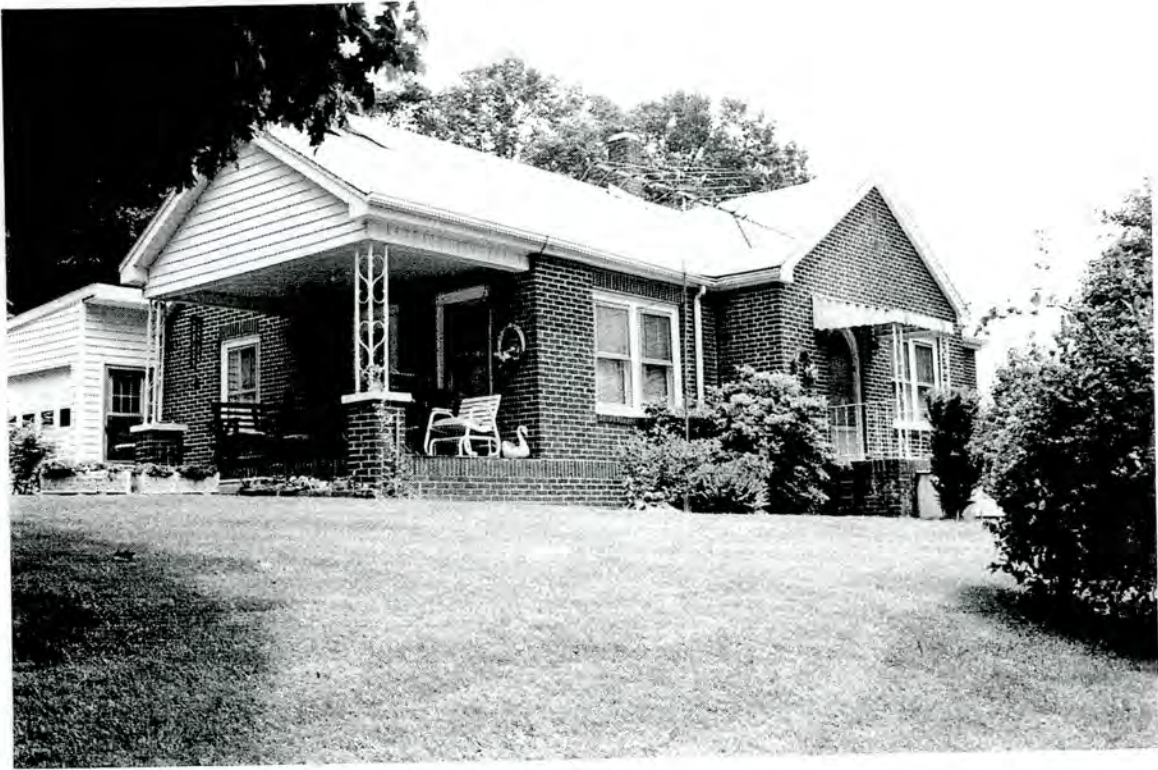
Plate 77: House (#25) – south front elevation of house at 18 Earl’s Repair Shop Road, Spruce Pine vicinity, Mitchell County
