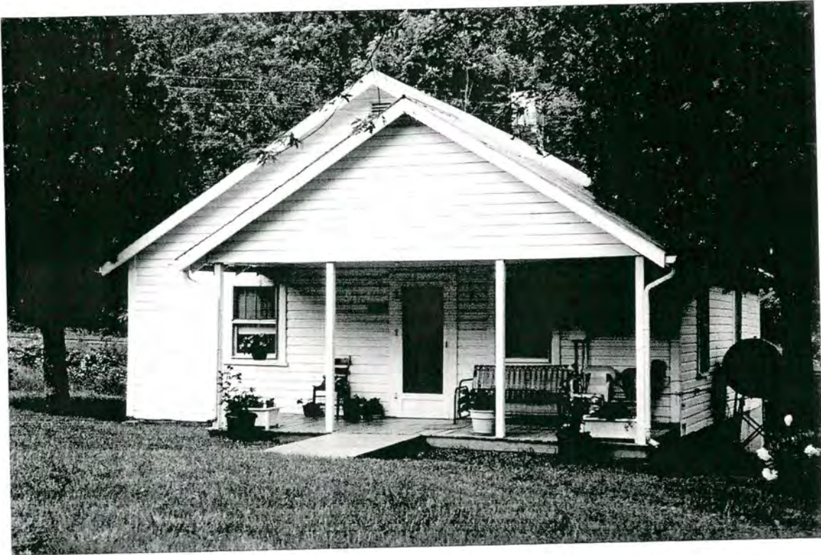
Plate 67: House (#13) – north front elevation of house at 400 Newdale Church Road, Newdale vicinity, Yancey County
