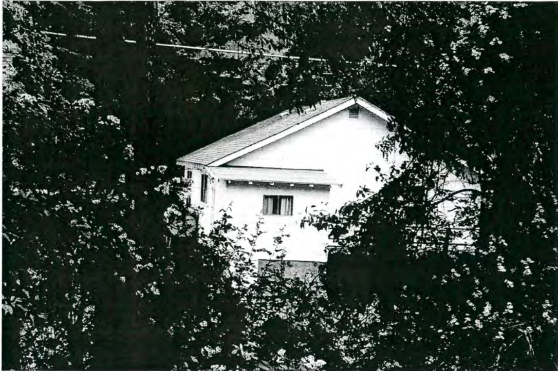
Plate 7: Looking north at rear of House (#13), which fronts on Newdale Church Road
