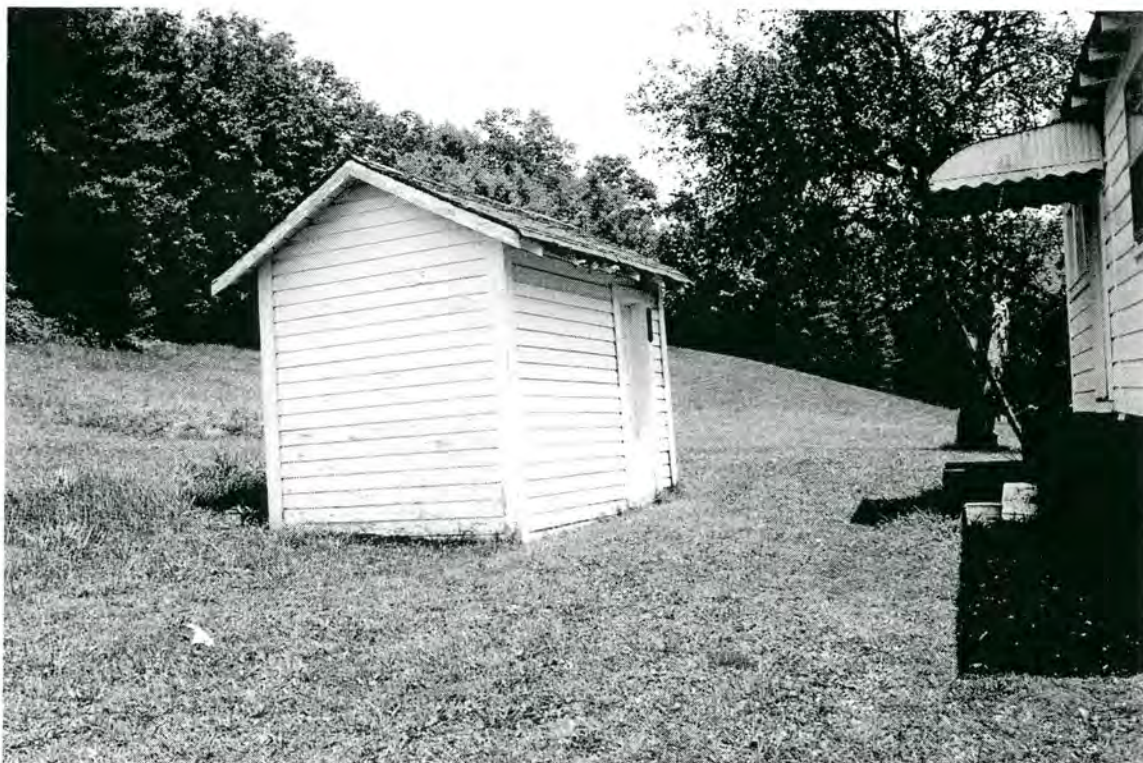
Plate 48: Lattie and Nora Young House – looking northeast at shed to rear of house
