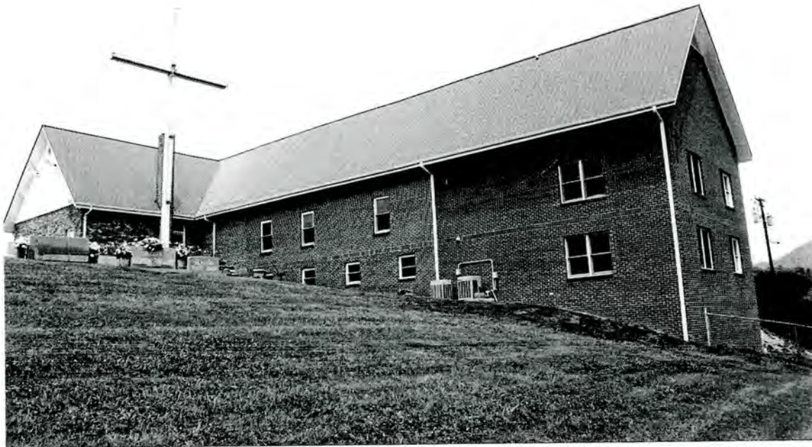
Plate 55: Liberty Hill Baptist Church – north rear and east side elevations
