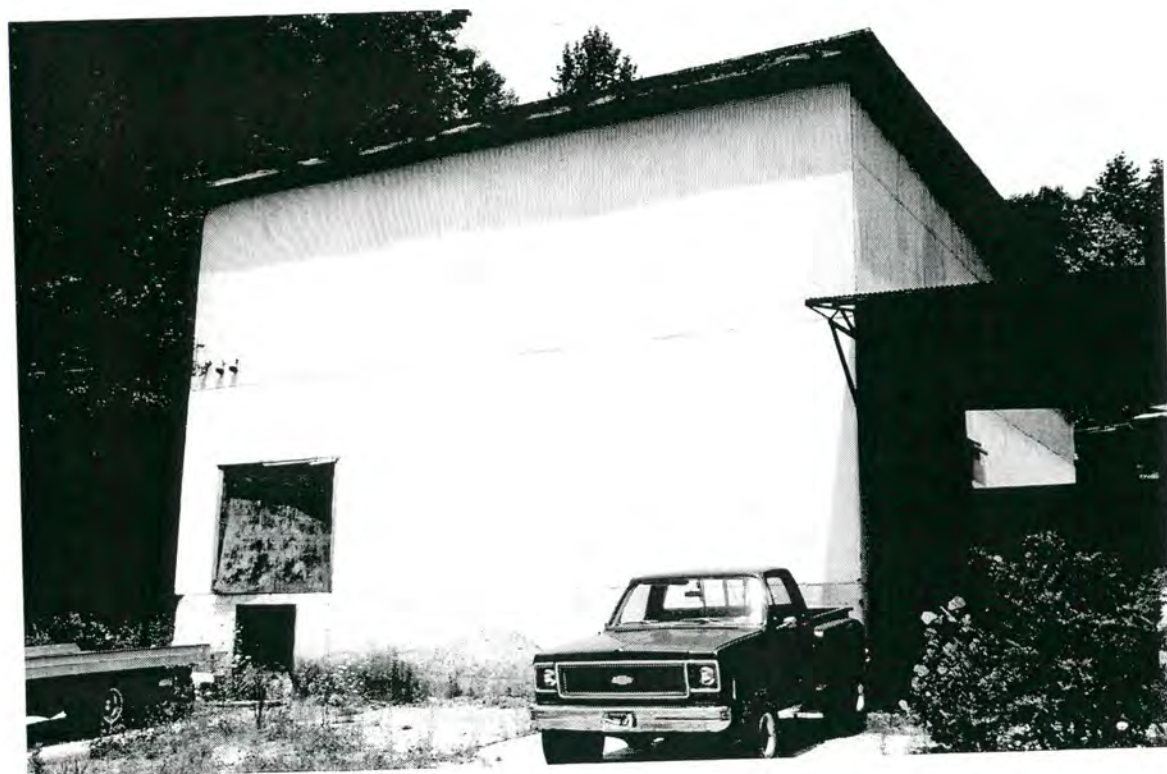
Plate 28: Deneen Mica Company Processing Mill – west end of complex looking northwest
