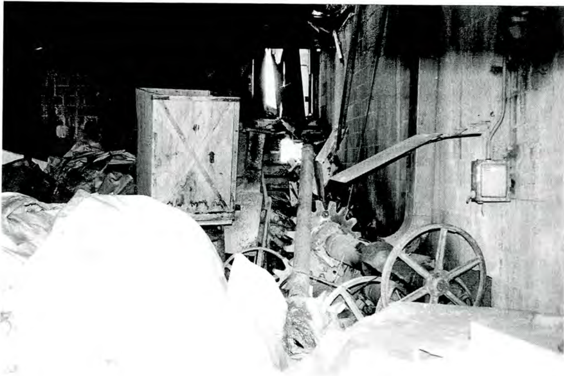
Plate 32: Deneen Mica Company Processing Mill – remnant equipment viewed from window opening on loading dock
