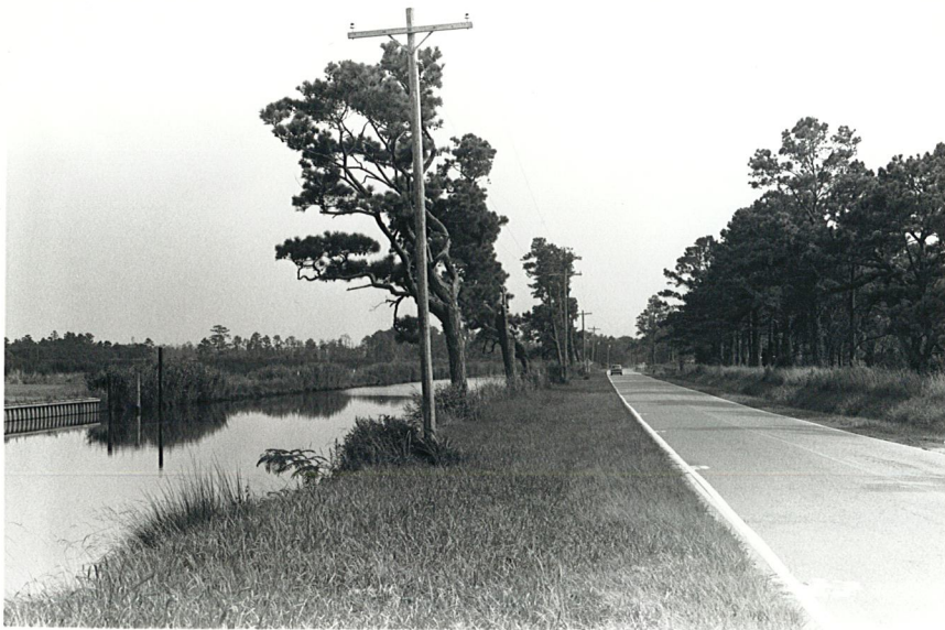
Plate 8. Great Ditch and S.R. 1110, Looking South from Bridge No. 6.
