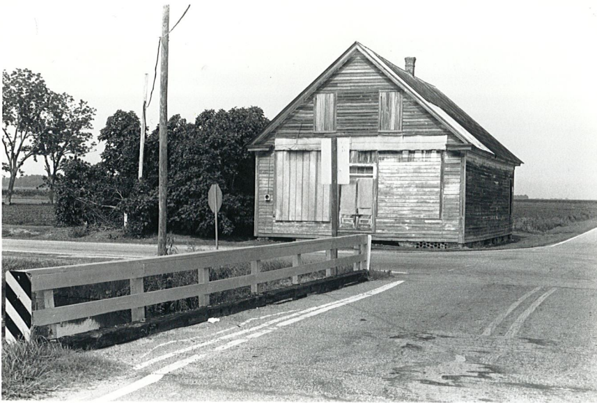
Plate 1. Bridge No. 6 and Watson's Store, Looking Northeast.
