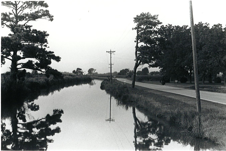
Plate 3. Great Ditch, Looking North From Bridge No. 6.
