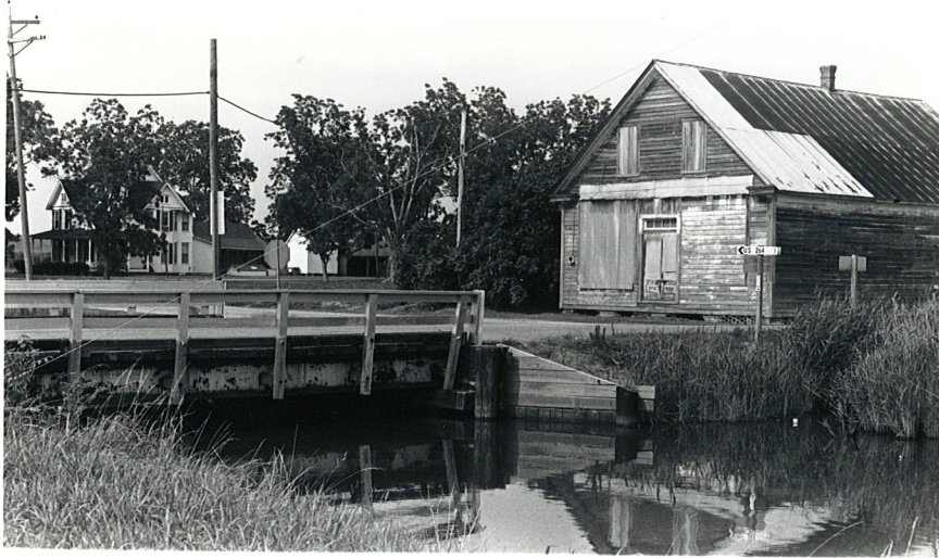
Plate 5. Watson's Store, Bridge No. 6, and George Israel Watson Farm, Looking Northeast from S.R. 1110.
