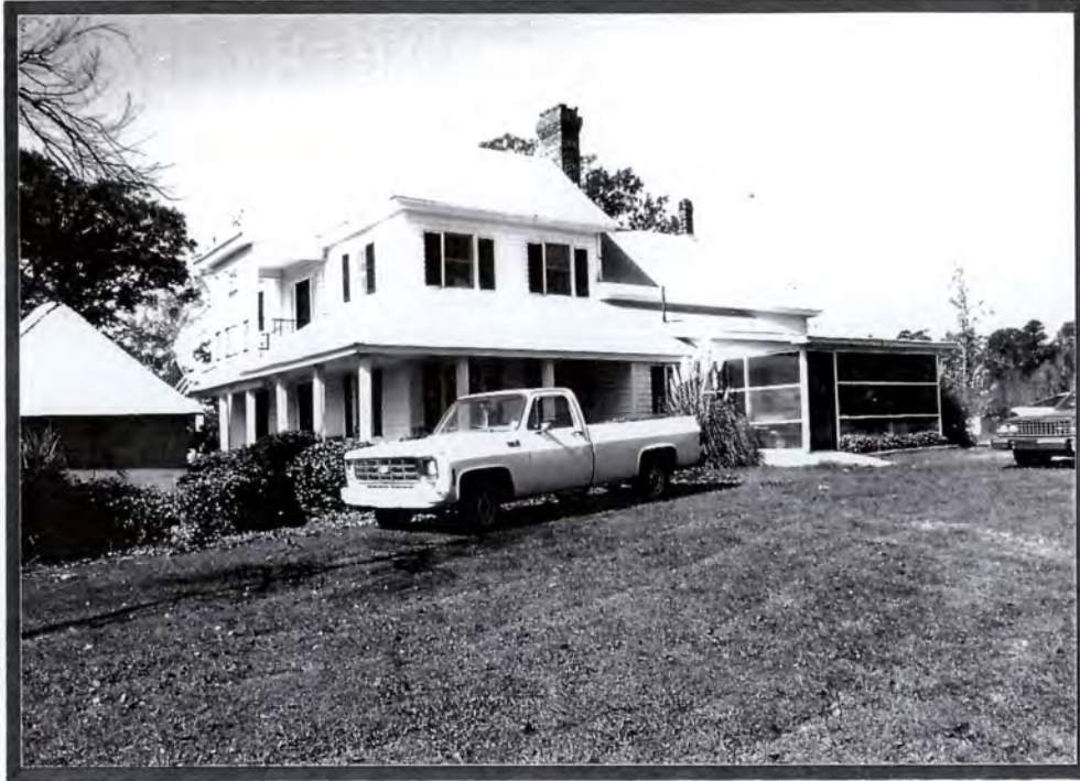
Plate IX.11 Rollins House (#42), US 601, Oblique-Facade (South Elevation), East Elevation, Well House.
