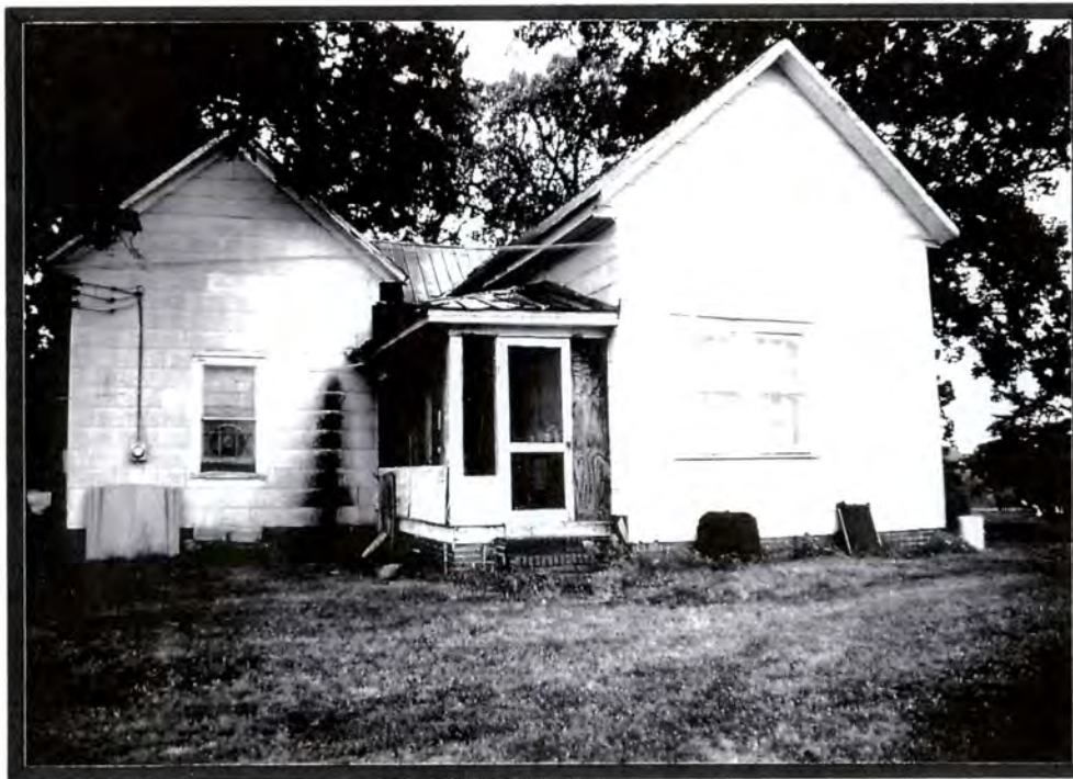
Plate V.16a House and Outbuilding, 5313 Pageland Road (#43), Rear (Northeast) Elevation
