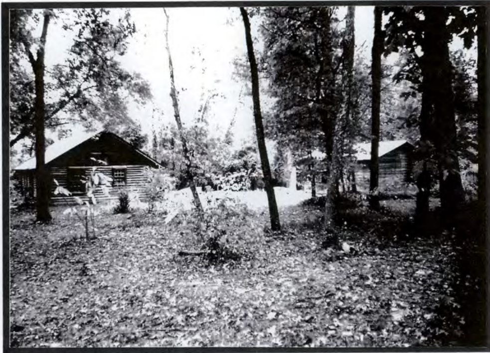
Plate V.11a Marcus Bruce Liles, Sr. House and Outbuilding (#2), North Elevation and Garage
