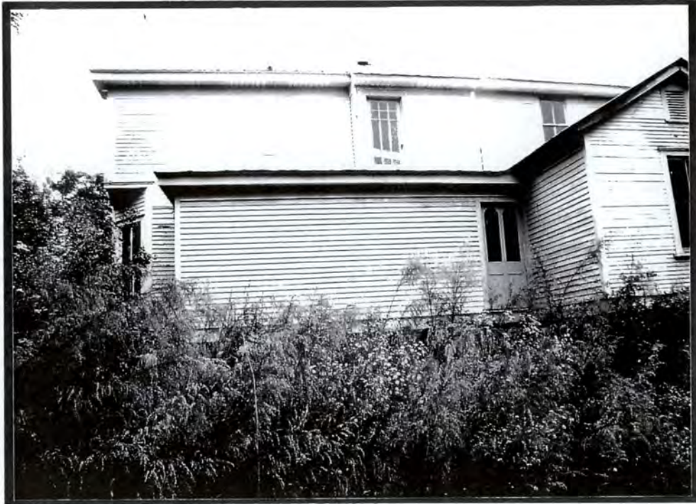
Plate V.24a Evans-Whitt House (#46) (UN113), Rear (East) Elevation
