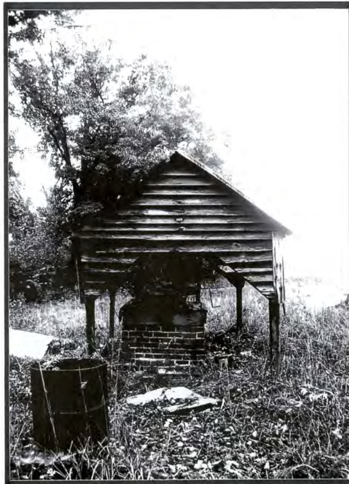
Plate V.31a Ervin Thomas House (#49) (UN385), Well and Well House
