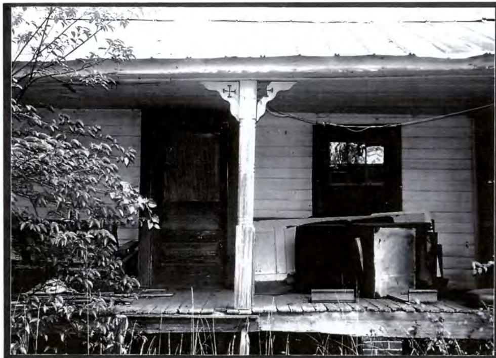
Plate V.27a Ervin Thomas House (#49) (UN385), Facade, Detail of Porch with Central Entrance, Facade Window, Flushboard Sheathing, Decorative Porch Post
