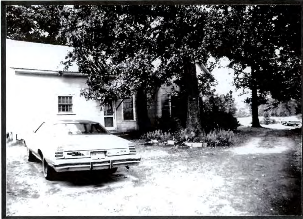
Plate V.17a House and Outbuilding, 5313 Pageland Road (#43), North Elevation South Elevations)
