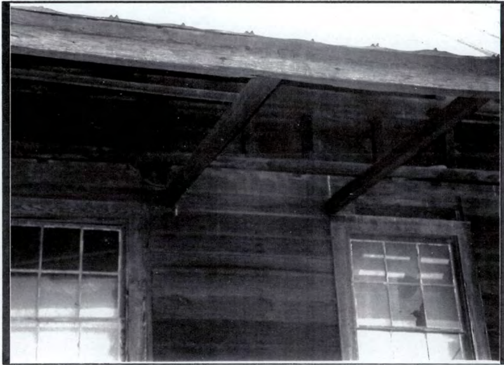
Plate V.37a Harrison Lee House (#55) (UN211), Detail of Facade Porch Roof Structure
