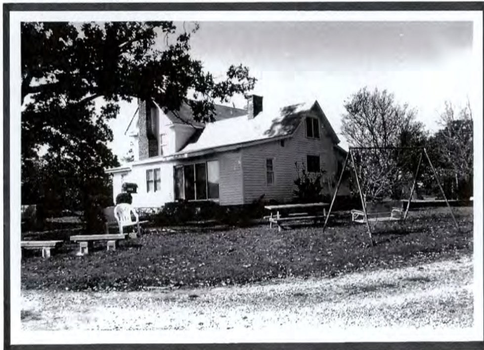
Plate IX.6 Henry Griffin House (#25), US 601, Oblique, South and East (Rear) Elevations.
