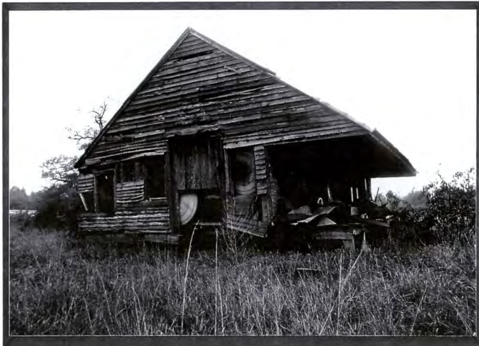
Plate V.36a Harrison Lee House (#55) (UN211), East Elevation, Location of Removed Chimney
