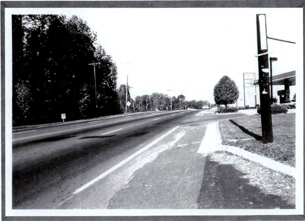
Plate V.1 Intersection of US 601 and US 74 at Northern Terminus of Project.
