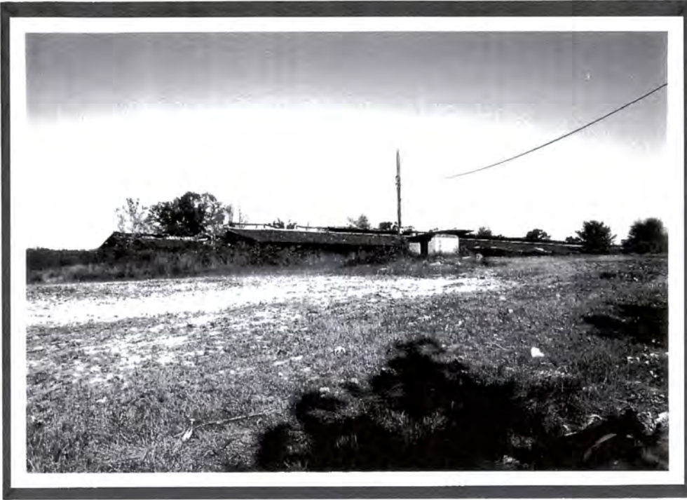
Plate VI.5 Abandoned Poultry Houses Adjacent to Property #50, US 601.
