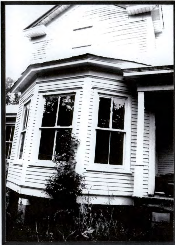
Plate V.22a Evans-Whitt House (#46) (UN113), Projecting Polygonal Bay, First Story, North Elevation; Shows Only Remaining Original Porch Post
