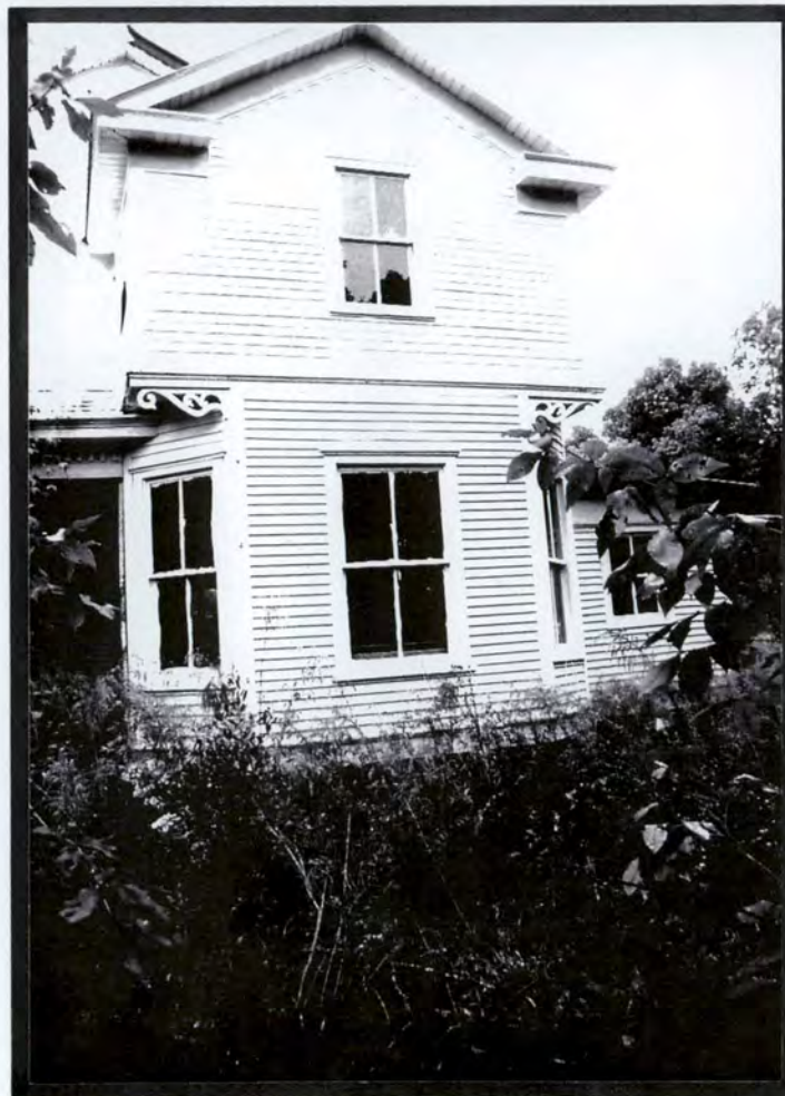
Plate V.23a Evans-Whitt House (#46) (UN113), Two-Story Projecting Bay on South Elevation With Clipped Corners at First Story
