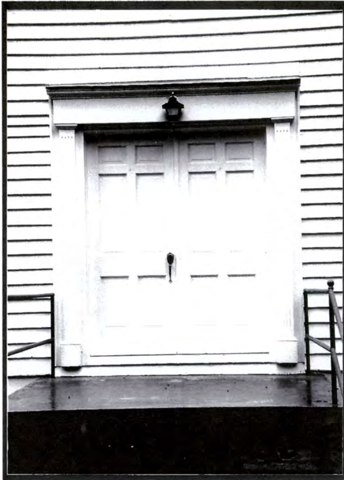
Plate V.6a Center United Methodist Church (#20), Detail, Main Entrance (West Elevation)
