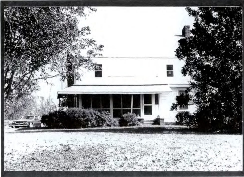
Plate IX.5 Henry Griffin House (#25), US 601, Facade, West Elevation.
