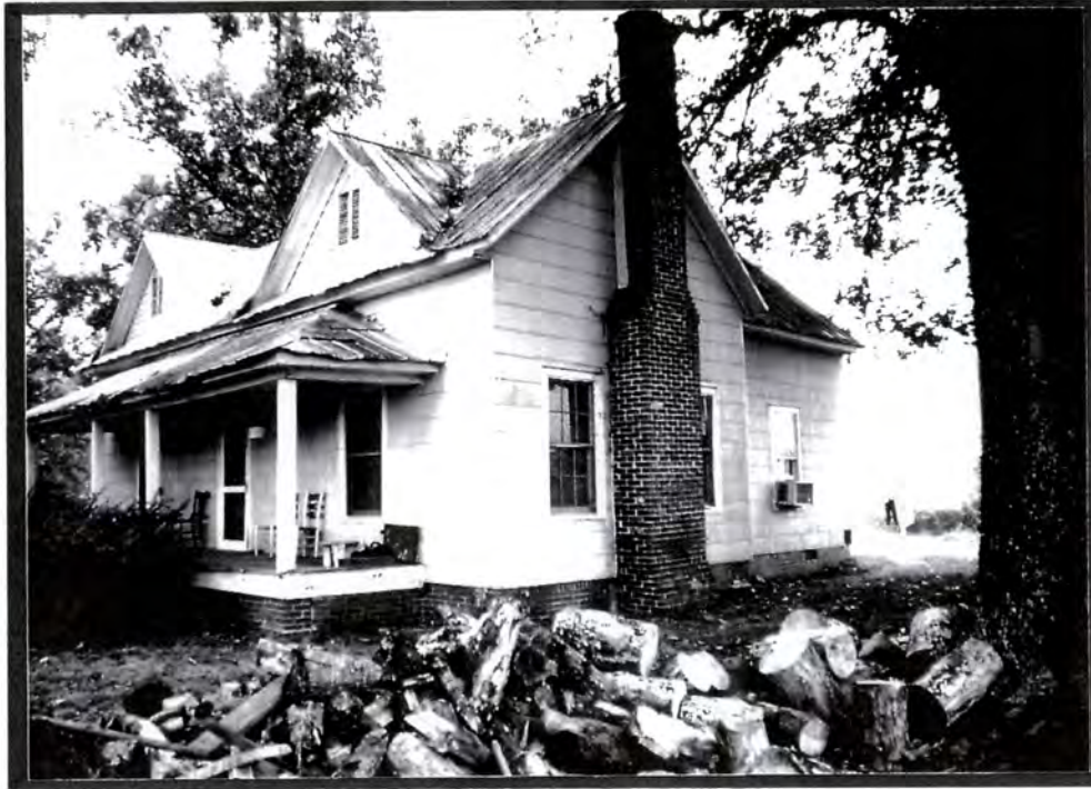
Plate V.15a House and Outbuilding, 5313 Pageland Road (#43), Oblique (Southwest and South Elevations)
