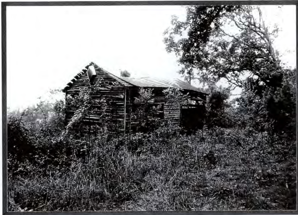
Plate V.32a Ervin Thomas House (#49) (UN385), Log Barn, Roof Collapsed
