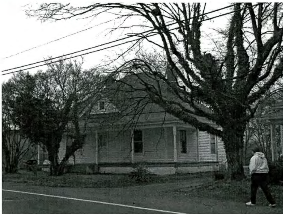
Property #10, House, 220 Klumac Road: This house has been determined not eligible for the National Register because it is neither historically nor architecturally significant.
