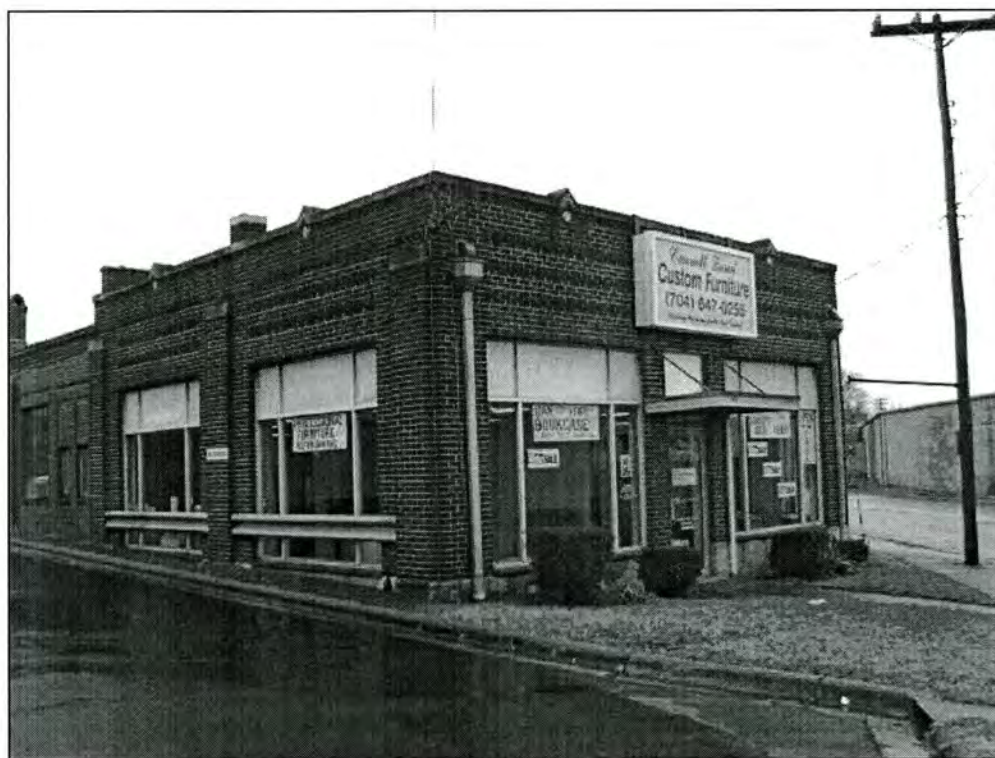
Figure 22: Custom Furniture Company, north and east elevations of front section.
