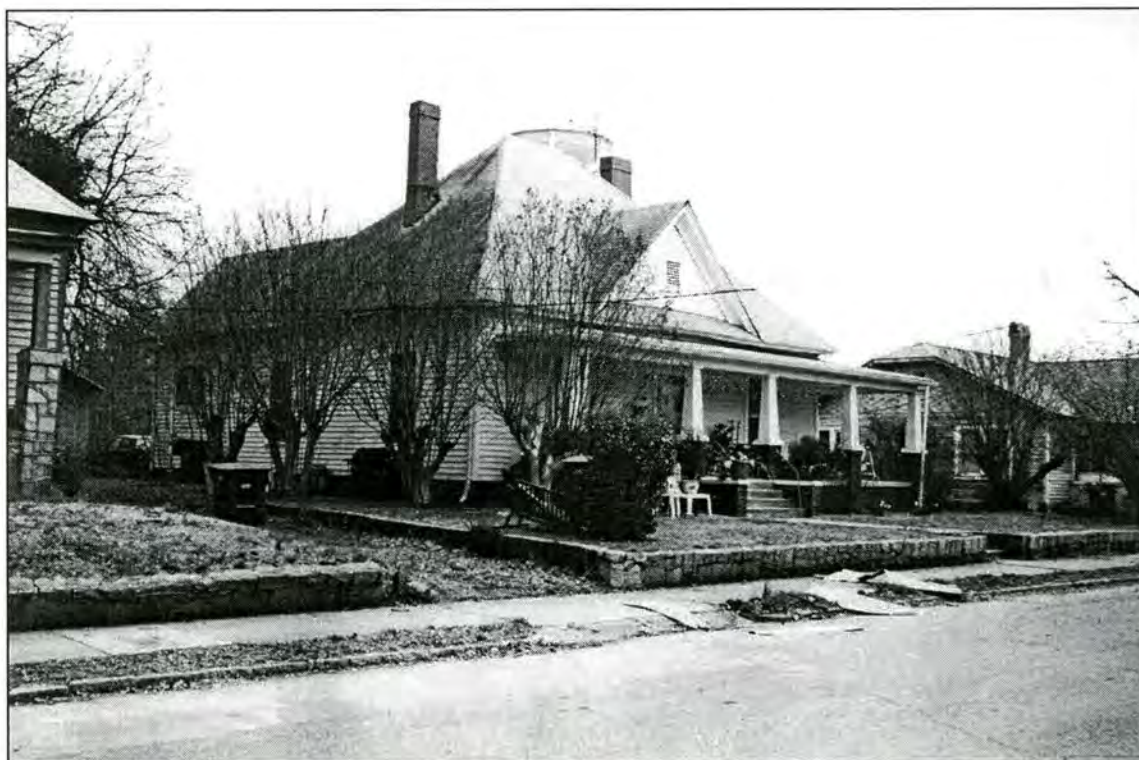
Figure 6: House, 118 Heilig Avenue (north and west elevations)
