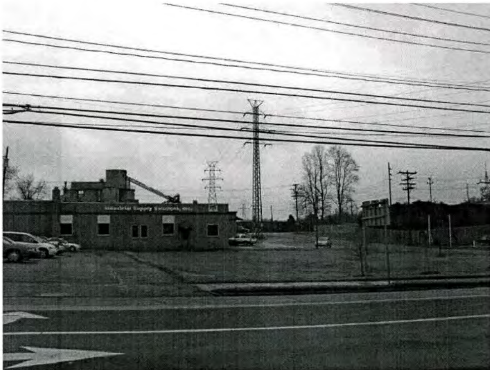
Property #5, Industrial Supply Solutions, 1551 S. Main Street: This property has been determined not eligible for the National Register because it is neither historically nor architecturally significant.
