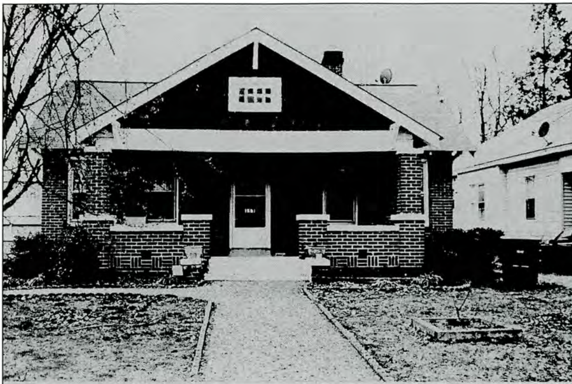
Figure 7 : House, 117 Heilig Avenue (east elevation)
