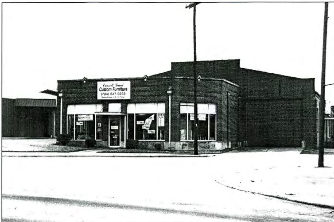
Figure 21: Custom Furniture Company, front elevation (from southwestern angle)
