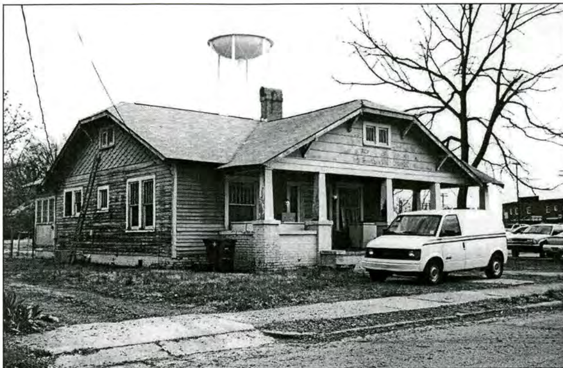
Figure 5 : House, 114 Heilig Avenue (north and west elevations)
