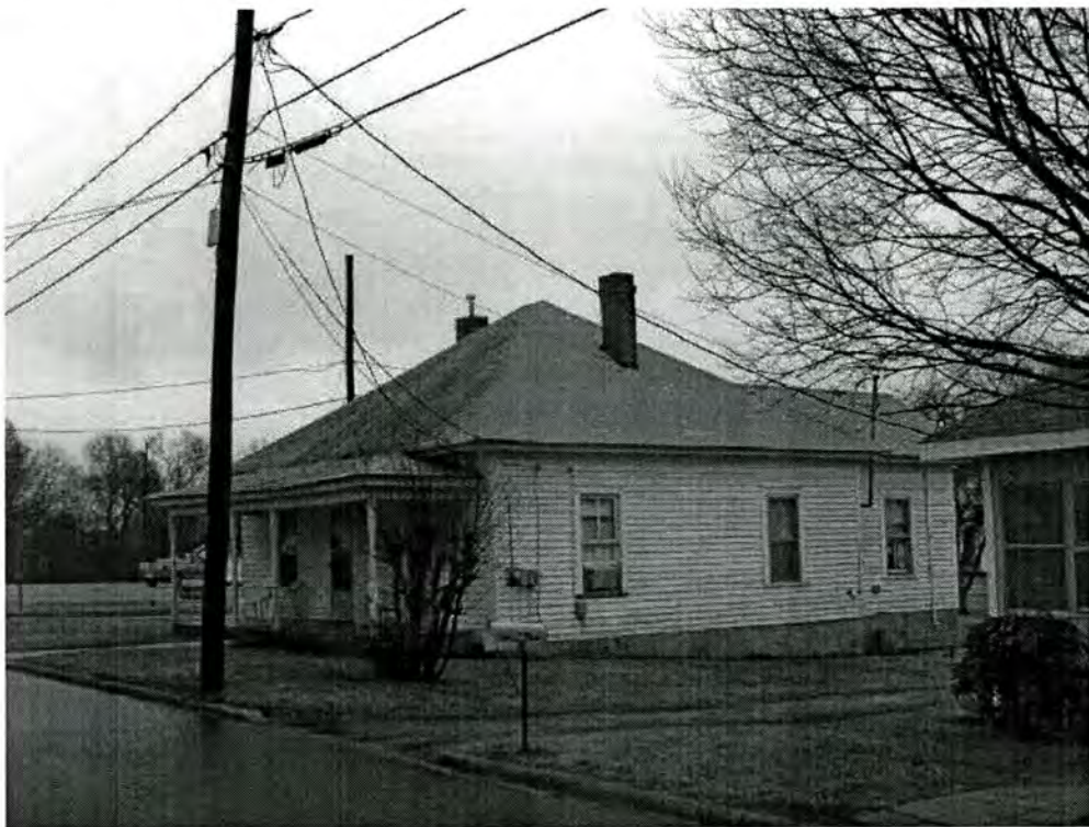
Property #16, House, 5 Carolina Street: This house has been determined not eligible for the National Register because it is neither historically nor architecturally significant.
