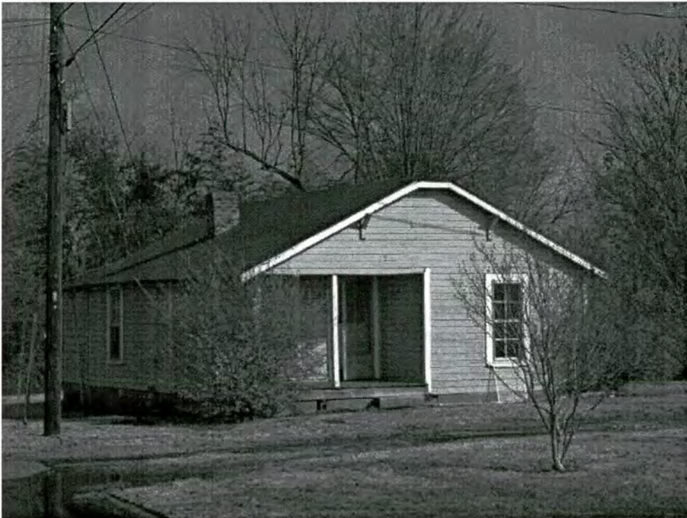
Property # 20, 18 Carolina Street: This house has been determined not eligible for the National Register because it is neither historically nor architecturally significant.
