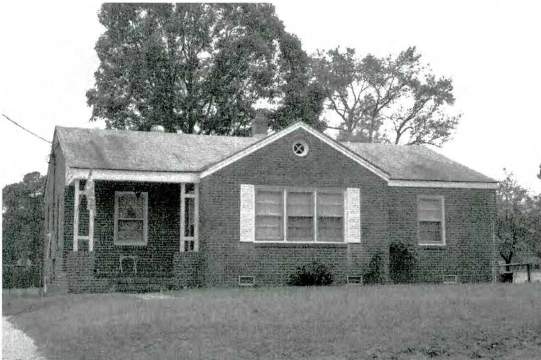
Figure 16. Property No. 12 - House (representative example). The property has been determined not eligible for the National Register because it is neither historically nor architecturally significant. Photographed November 3, 2004.
