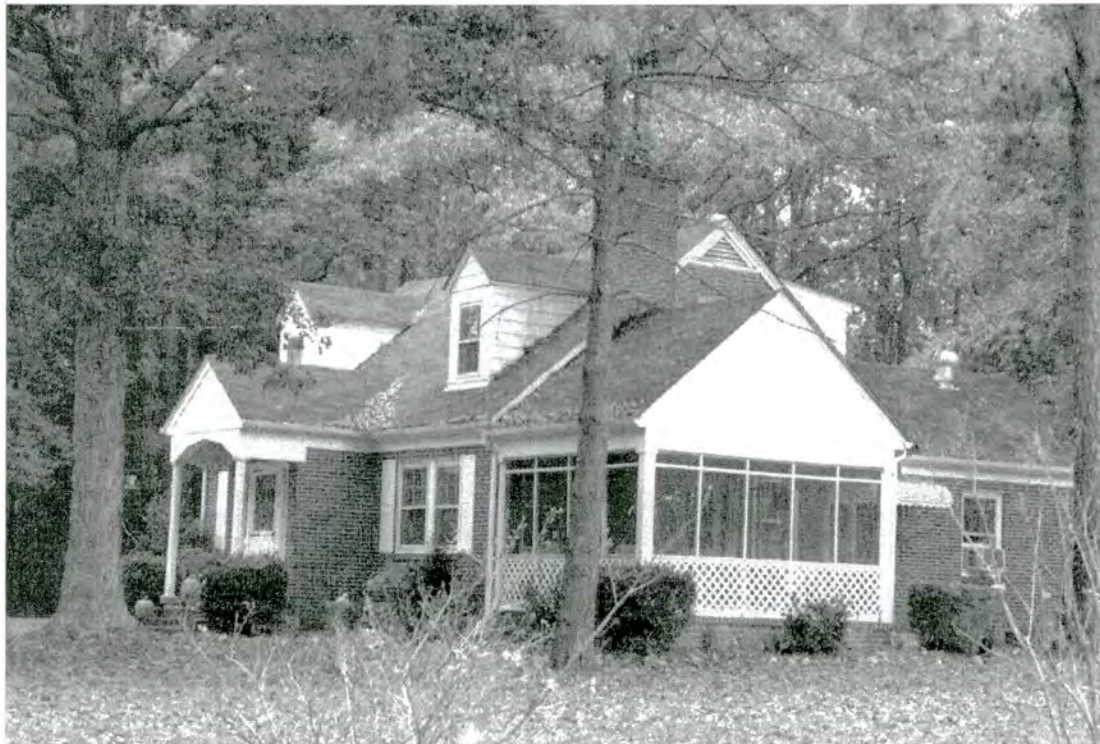
Figure 14. Property No. 10 - House (Parsonage of First Church of the Nazarene). The property has been determined not eligible for the National Register because it is neither historically nor architecturally significant. Photographed November 3, 2004.
