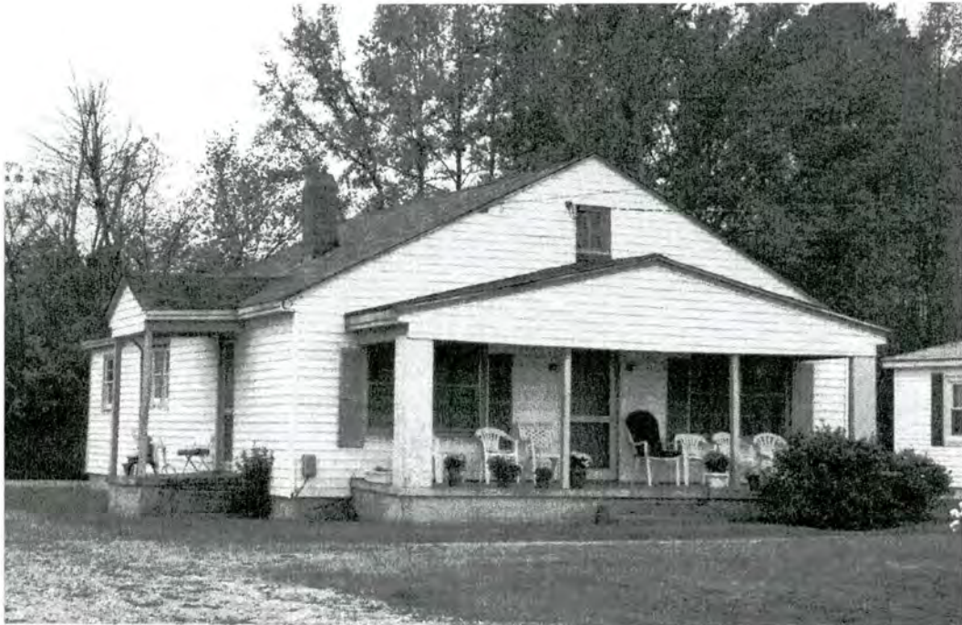
Figure 26. Property No. 25 - House. The property has been determined not eligible for the National Register because it is neither historically nor architecturally significant. Photographed November 3, 2004.
