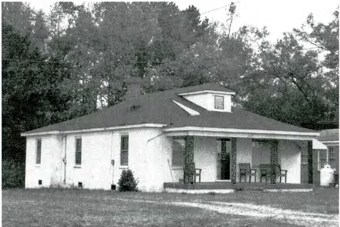
Figure 28. Property No. 28 - House. The property has been determined not eligible for the National Register because it is neither historically nor architecturally significant. Photographed November 3, 2004.
