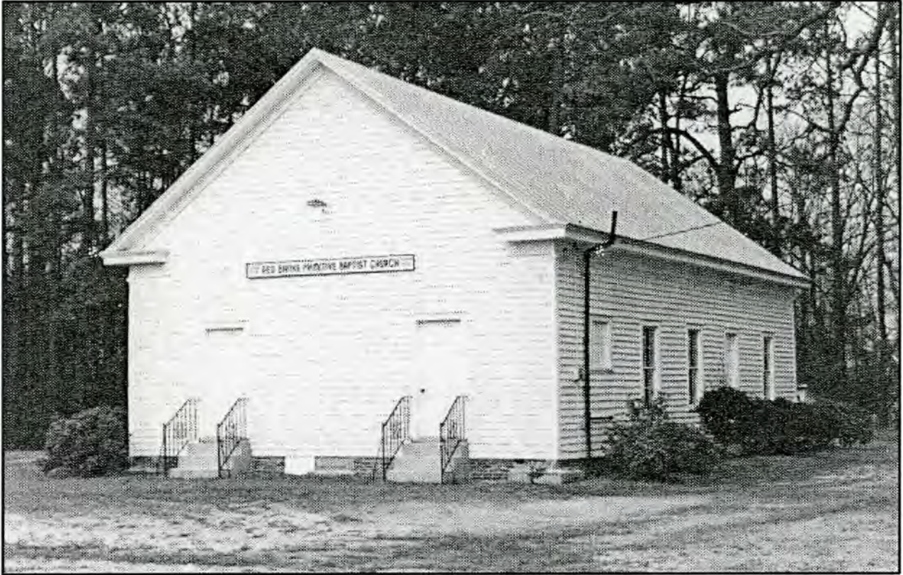
Figure 14. Traditional Primitive Baptist Church Exterior. The Red Banks meetinghouse in Pitt County, built in 1893, perfectly exemplifies the architectural conventions of the denomination. The one-story, frame structure displays characteristic features like the paired entry, boxed cornice with returns, and simplicity of ornament and finish. From Scott Power, The Historic Architecture of Pitt County , North Carolina (1991), p. 361.
