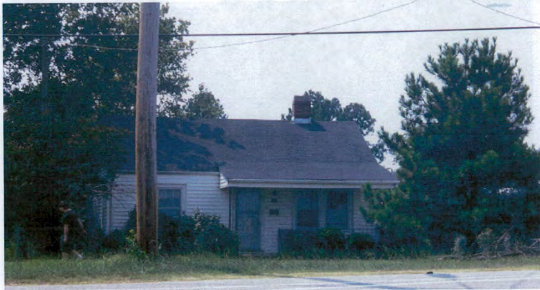
Figure 26. Property 5 - House. The property has been determined not eligible for the National Register because it is neither historically nor architecturally significant. Photographed September 11, 2002.
