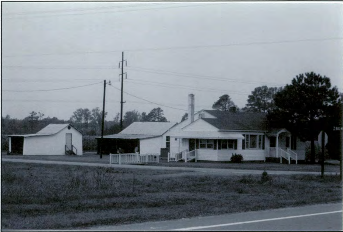
1. House, SW jct. of U.S. 158 and SR 1175
