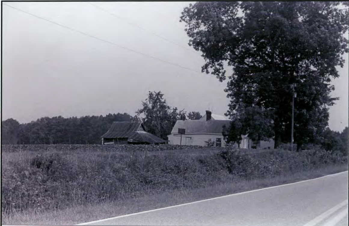
William Kiff House, view to north, showing rear of kitchen and oblique view of smokehouse
