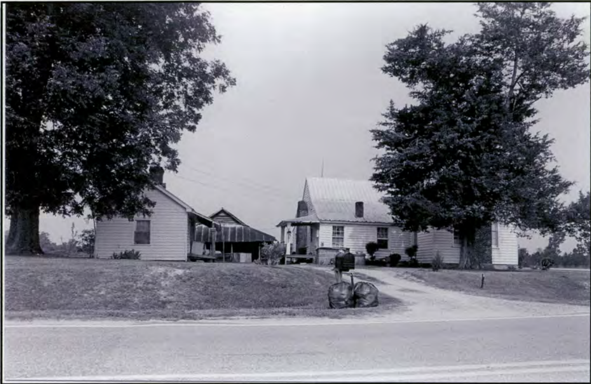
William Kiff House, view to west showing rear ell, kitchen, and smokehouse
