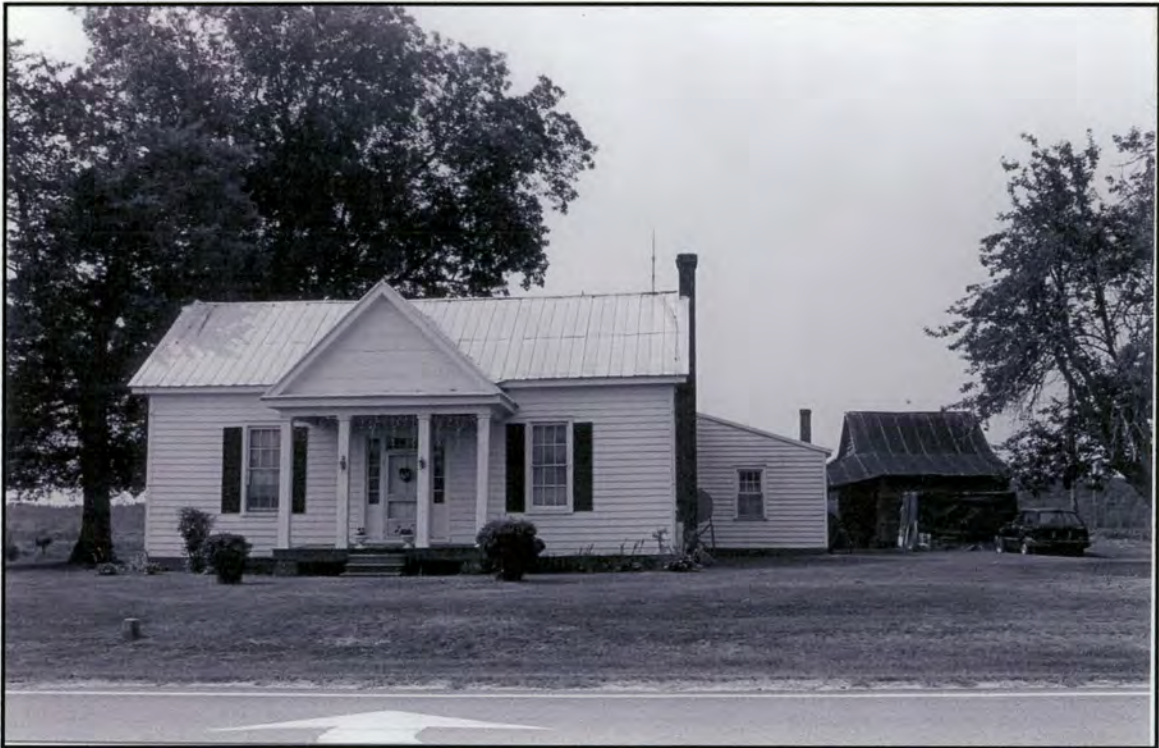
William Kiff House, view to south showing facade and smokehouse at right
