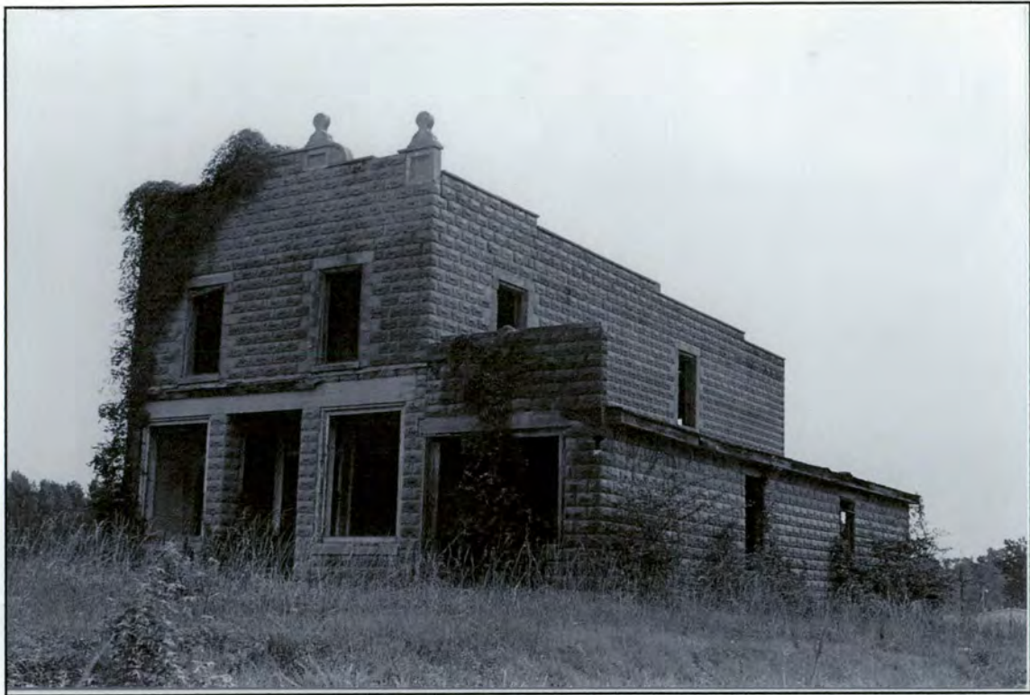
27. Commercial building, NE corner of jct. of SR 1305 and SR 1303
