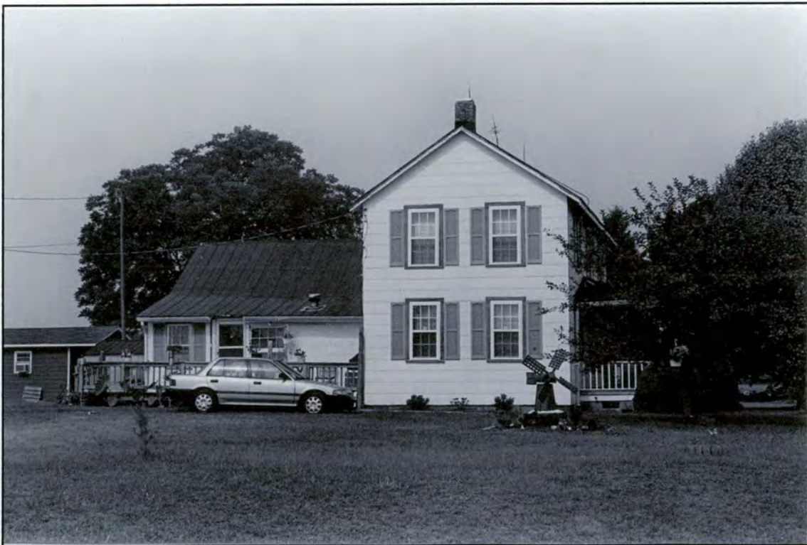
35. House, SW jct. of U.S. 158 and SR 1178
