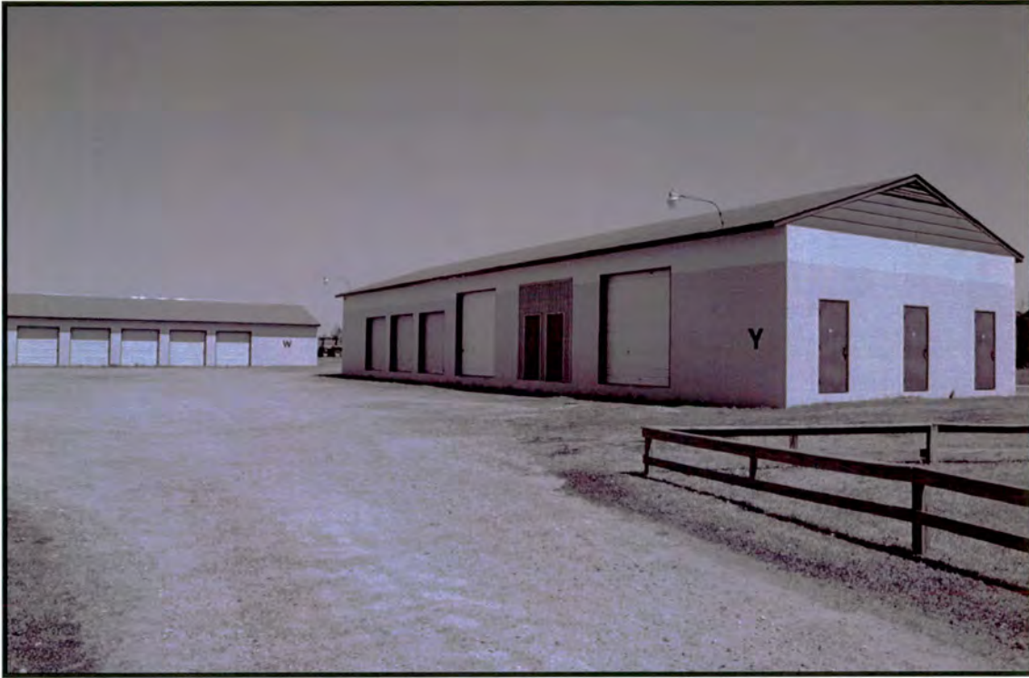
Plate 61: Twilite Drive-In – looking northeast at modern concrete-block storage buildings
