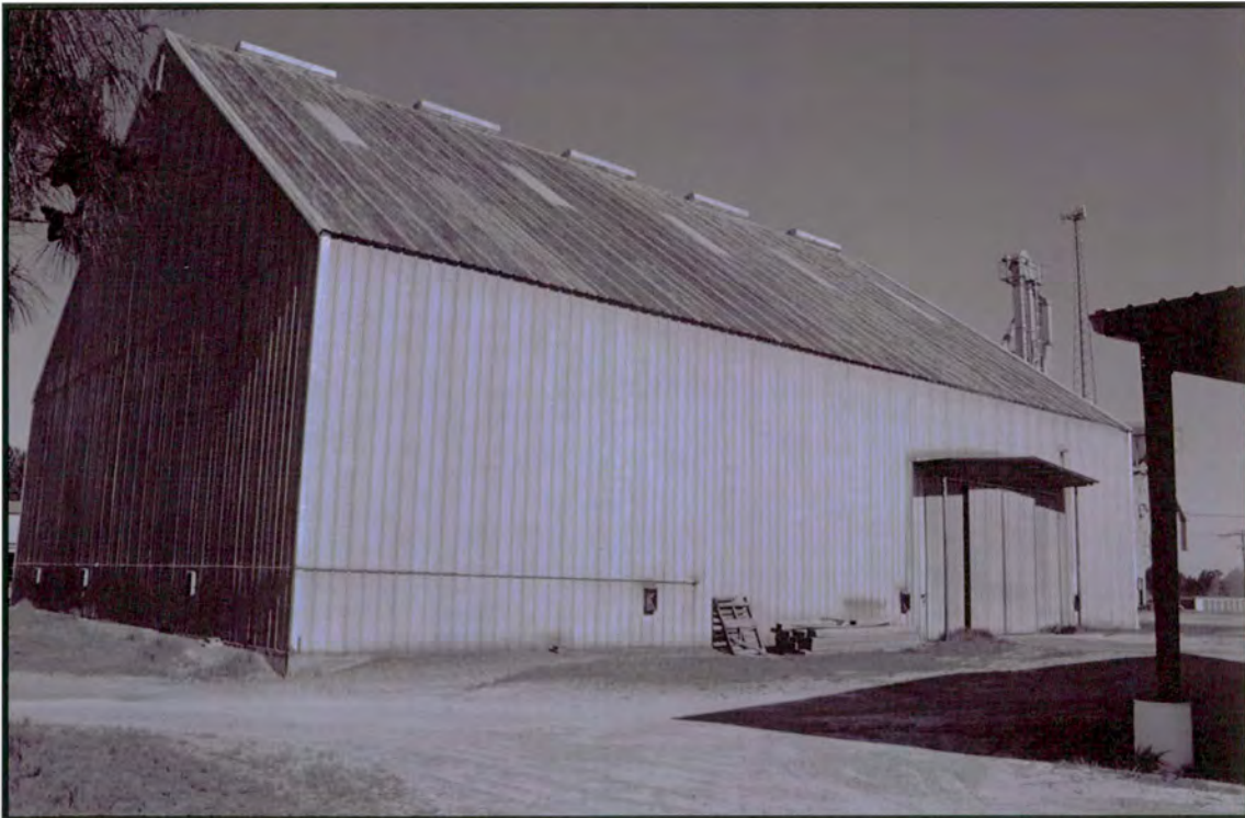
Plate 37: Golden Peanut Buying Station – looking northwest at Warehouse [I]
