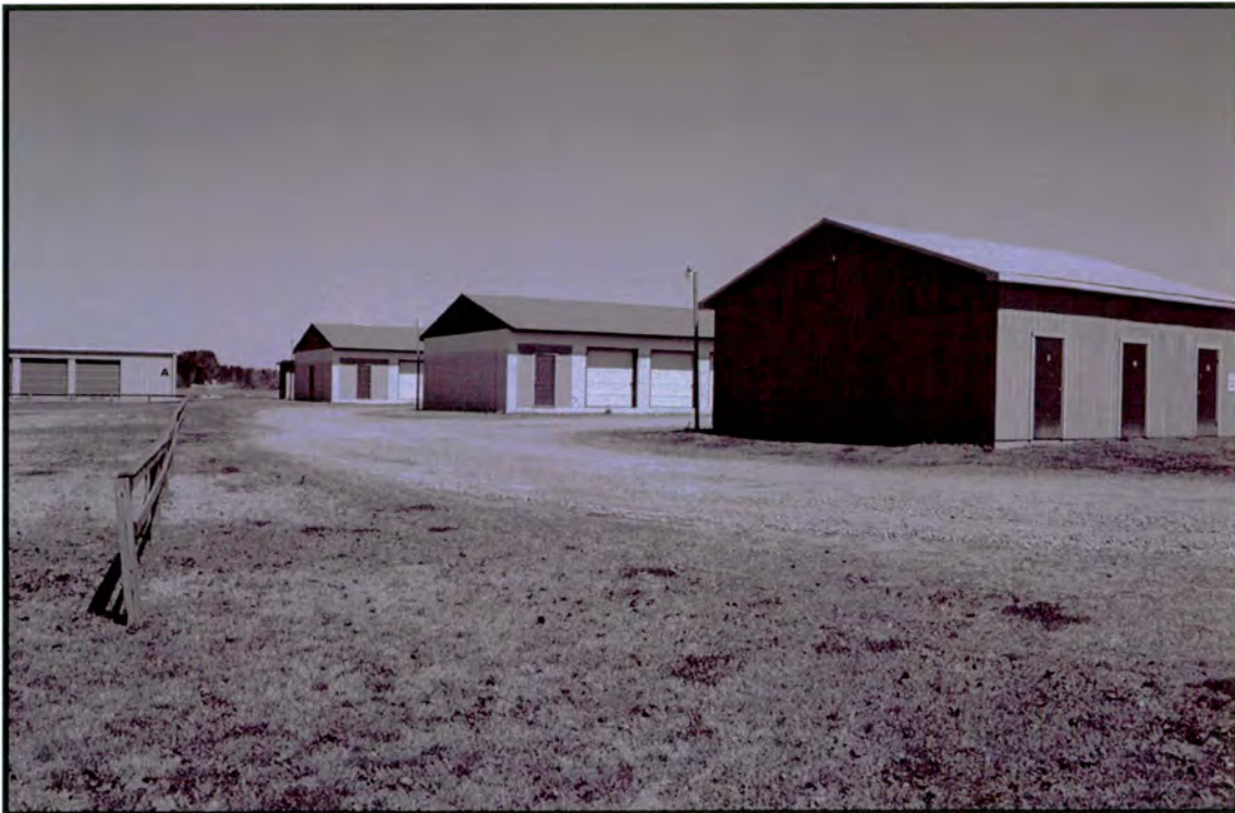
Plate 62: Twilite Drive-In – looking northeast at modern composition-board-sheathed, concrete-block, and metal-clad storage buildings
