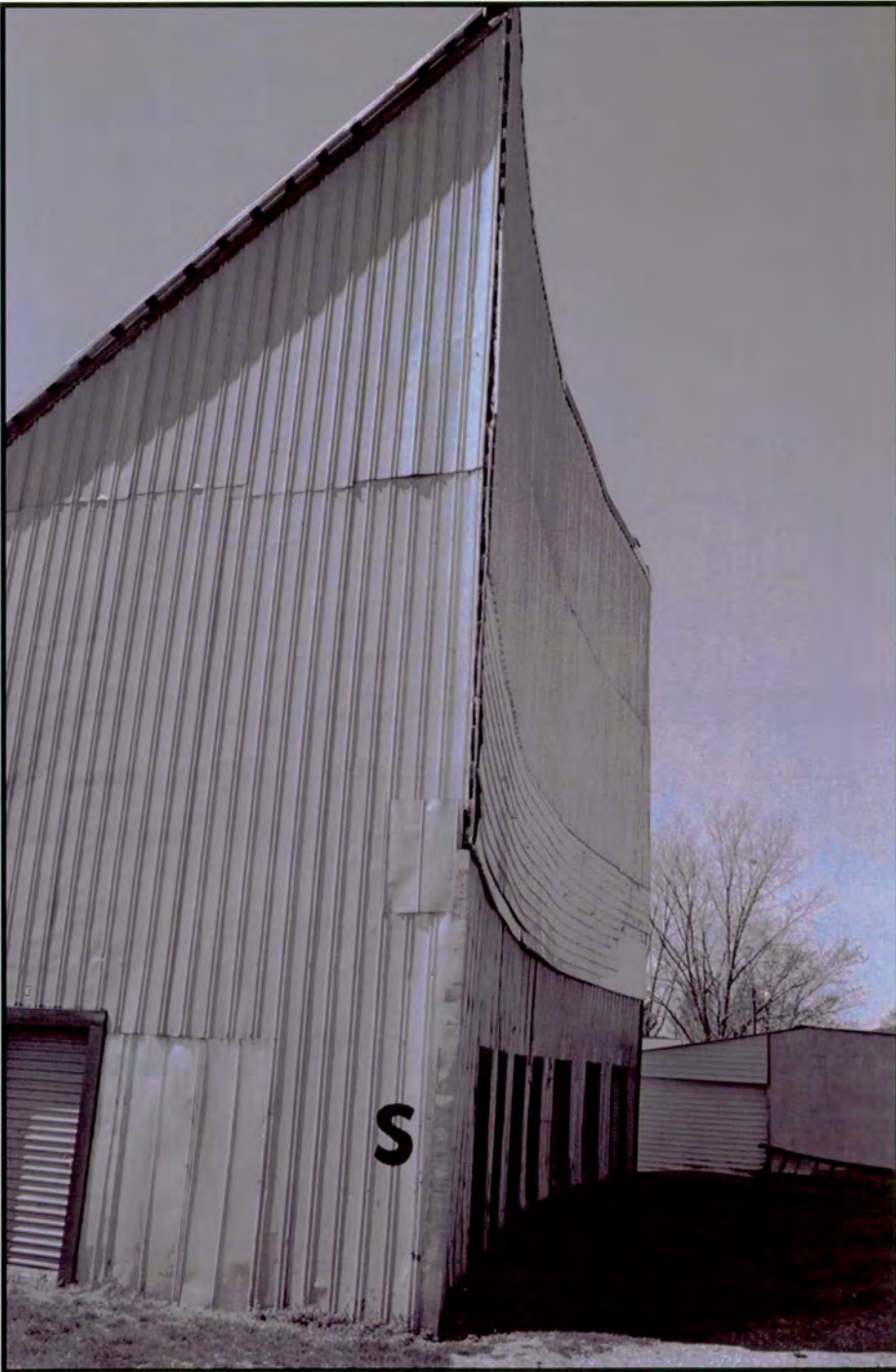
Plate 58: Twilite Drive-In – looking west at screen tower; note doors cut into front of screen, storage building extension to rear, and truncating of end of screen
