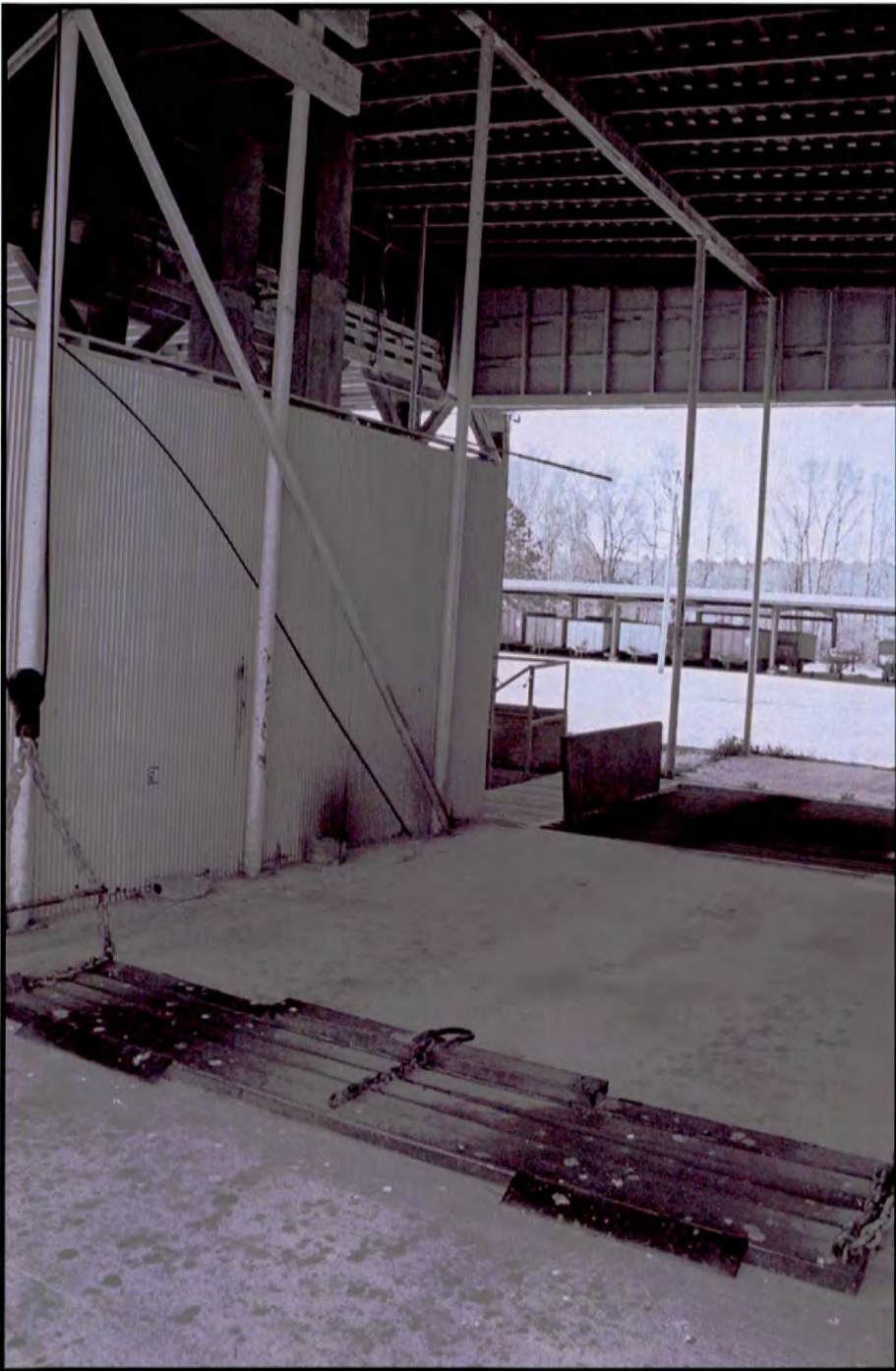
Plate 35: Golden Peanut Buying Station – interior of Overhead [F]; plate for lifting trailers in foreground, dumping grate to rear
