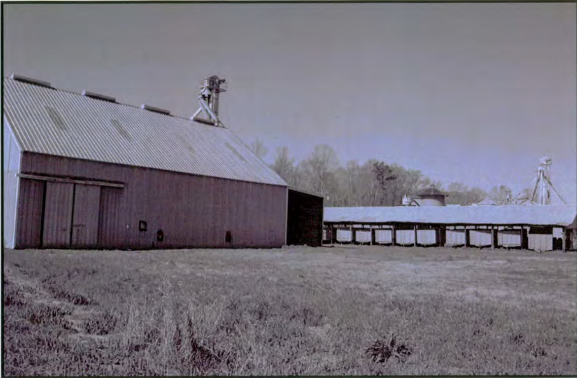
Plate 38: Dixie Peanut Buying Station – looking southwest at east warehouse on left and drying shed on right
