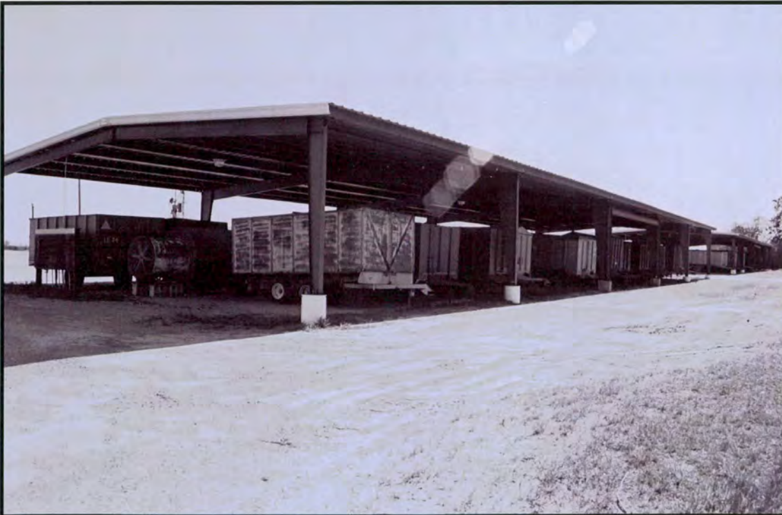
Plate 31: Golden Peanut Buying Station – looking northeast at Drying Shed No. 4 [D]
