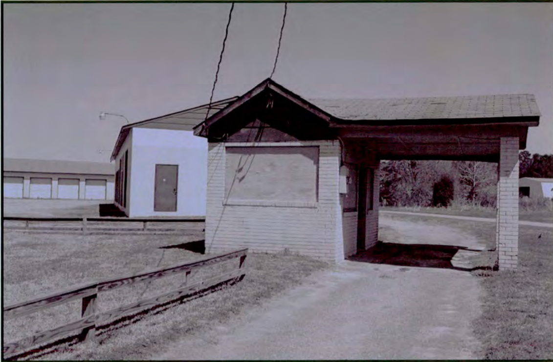
Plate 59: Twilite Drive-In – looking north at ticket booth/concession stand; note location of original entry road at right beneath carport and modern storage buildings at left
