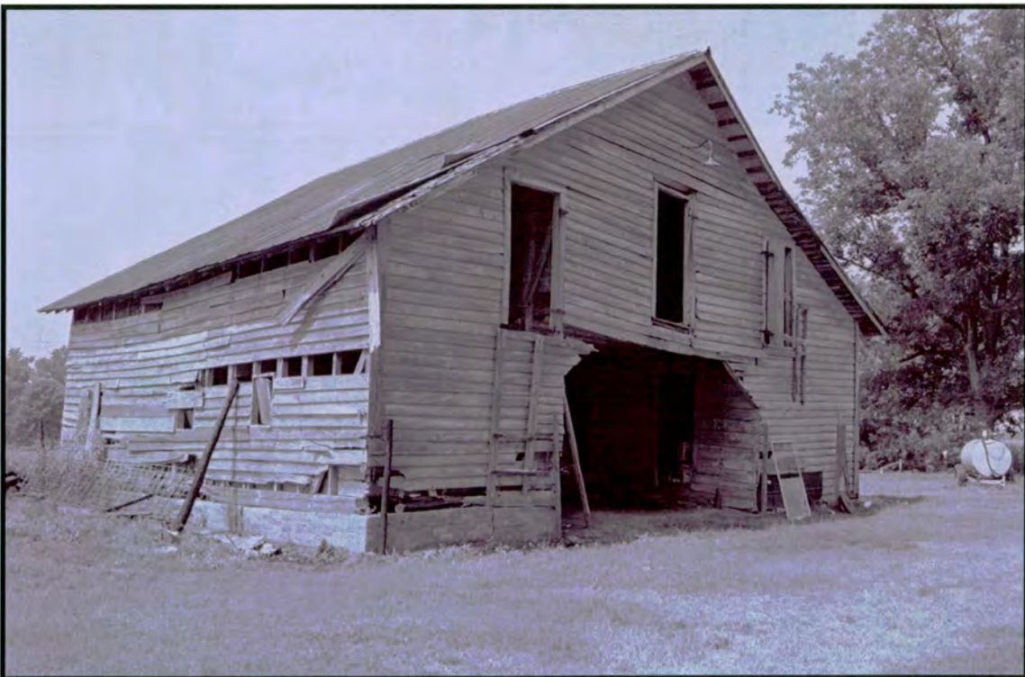
Plate 55: Slade Cemetery – looking southwest at barn
