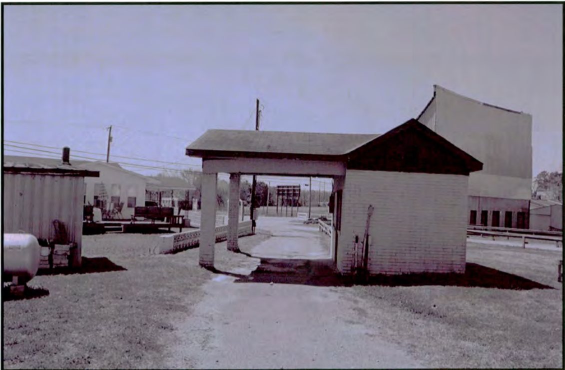
Plate 60 Twilite Drive-In – looking south toward US 64 at ticket booth/concession stand at center and screen at right
