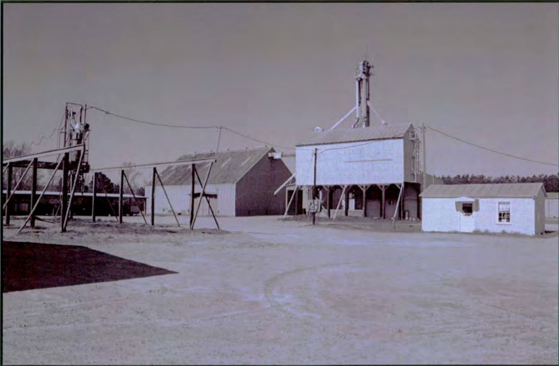
Plate 27: Golden Peanut Buying Station – looking southwest at Grading Sampler at left, Warehouse at left center, Overhead at right center, and Office at right
