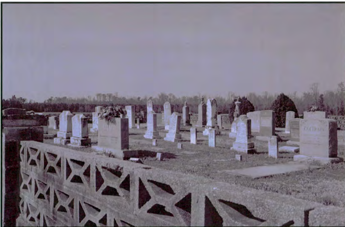
Plate 22: Manning Cemetery – openwork, concrete-block wall enclosing family cemetery
