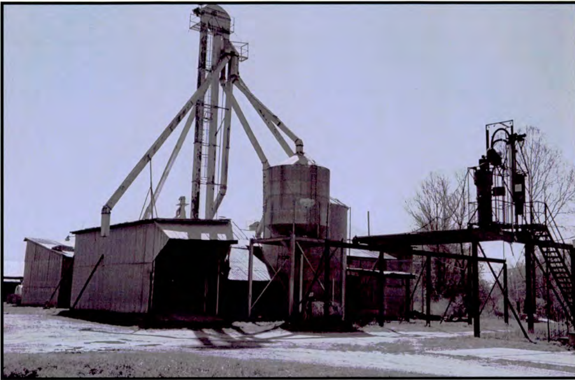
Plate 40: Dixie Peanut Buying Station – looking southeast at dumper/elevator at right, silos at center, and grading sampler, at right, associated with central warehouse
