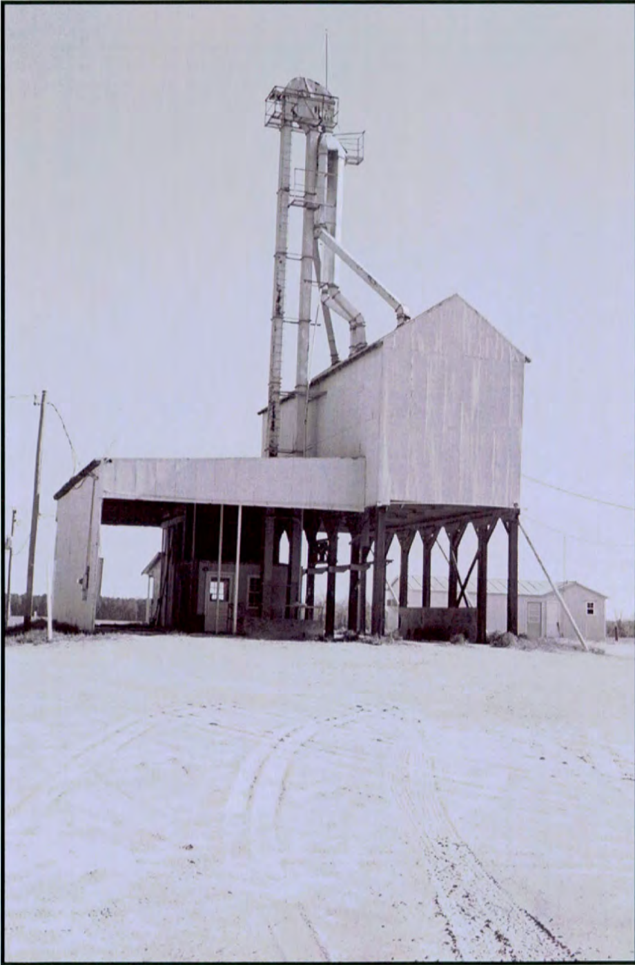
Plate 34: Golden Peanut Buying Station – looking northeast at Overhead [F]
