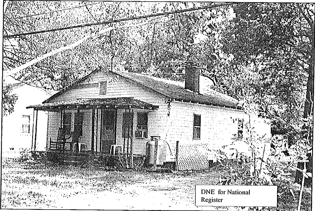
Property 50: House, 3291 McCaskey Road
