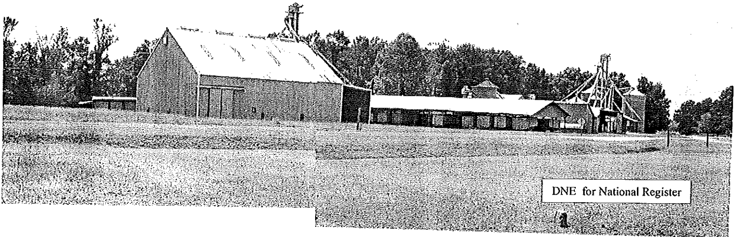
Property 33: Abbitts Mill (MT 619), S side NC 125, .2 mile east of SR 1420 Jct.
