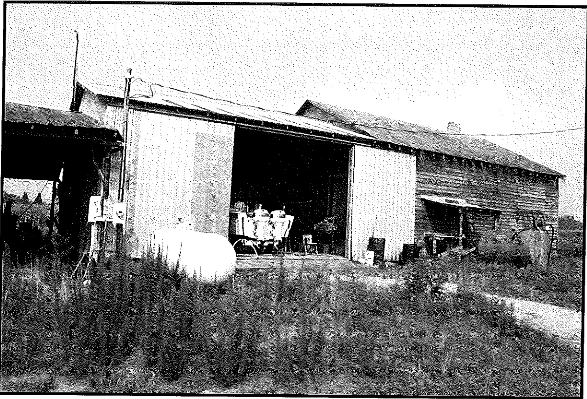
Plate 9: Whitley Farm – looking west at barn and attached sheds [C]
