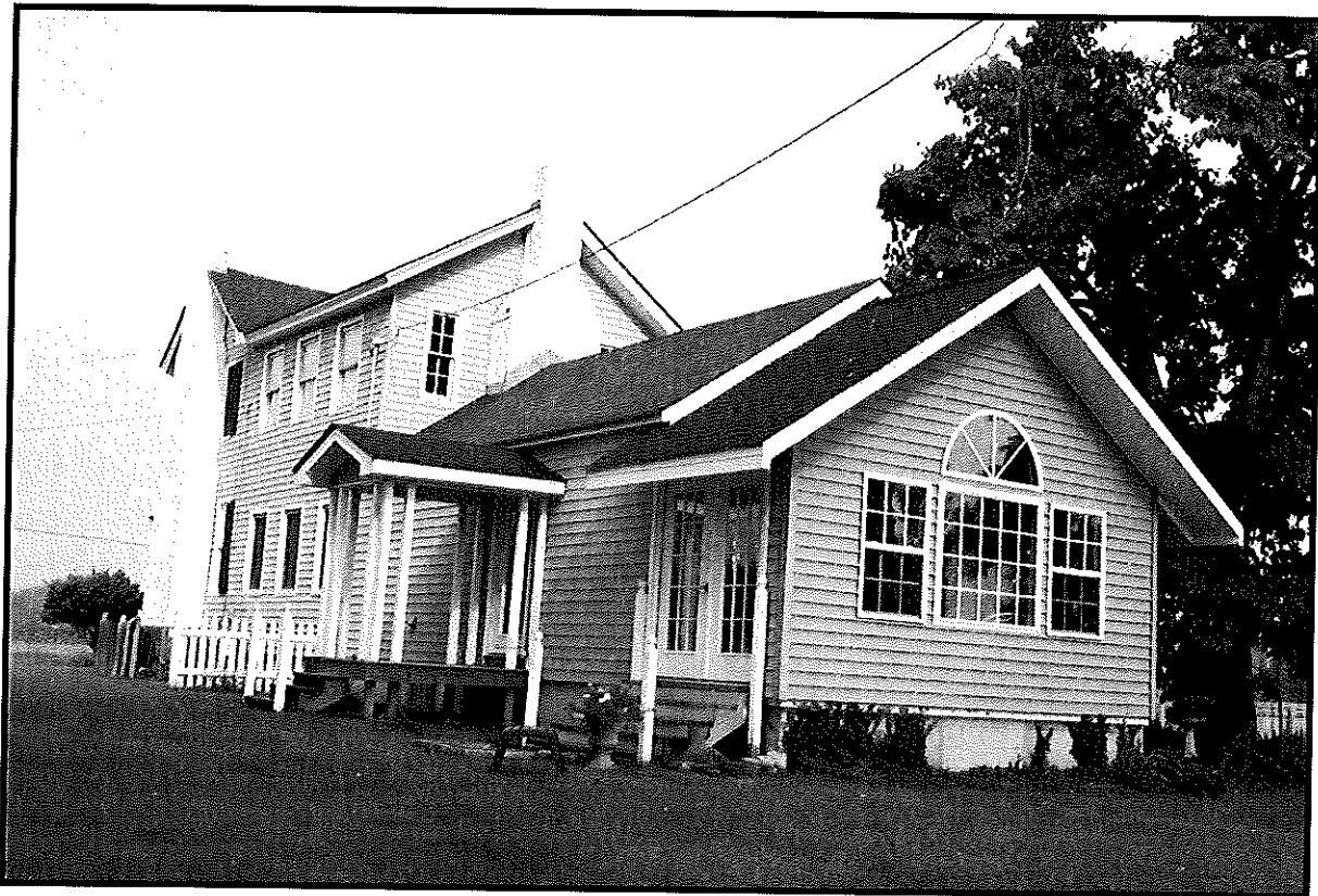
Plate 4: Whitley Farm – northeast rear and southeast side elevations of farmhouse [A]
