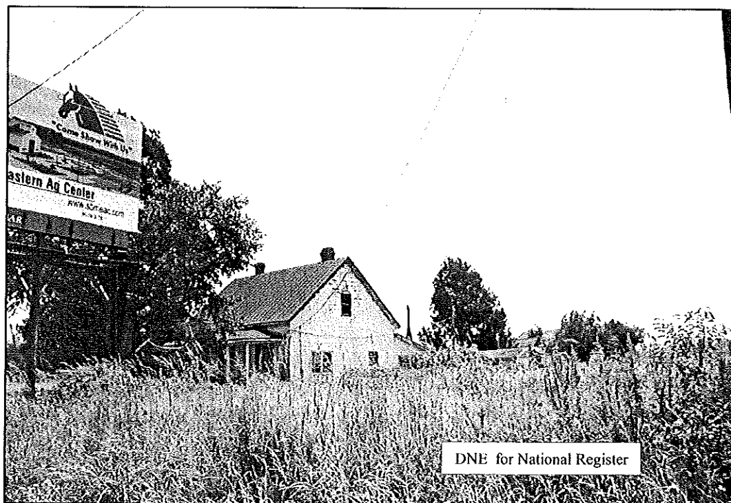
Property 59: west elevation
