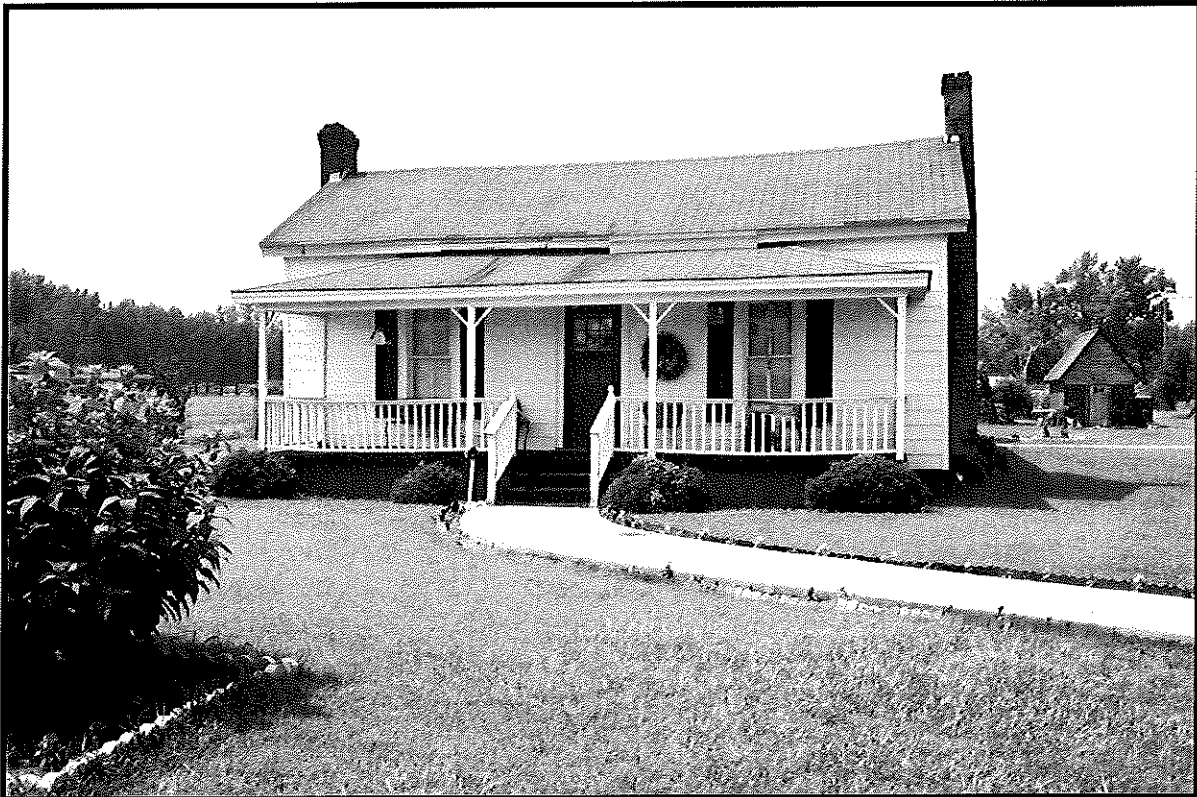
Plate 44: Bennett-Smith House – north front elevation; shed at right
