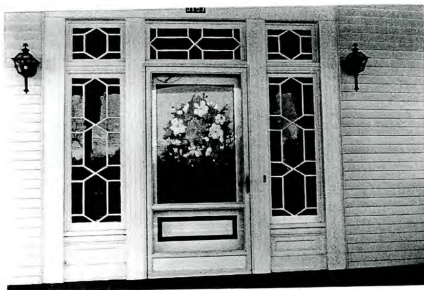
Plate 3. Currin-Bowling House, Rear Elevation, Looking East.
