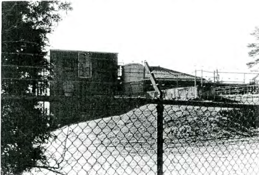
Plate 16. Oxford Water Works, North Elevations of Building, Basins, and Tank, Looking South.
