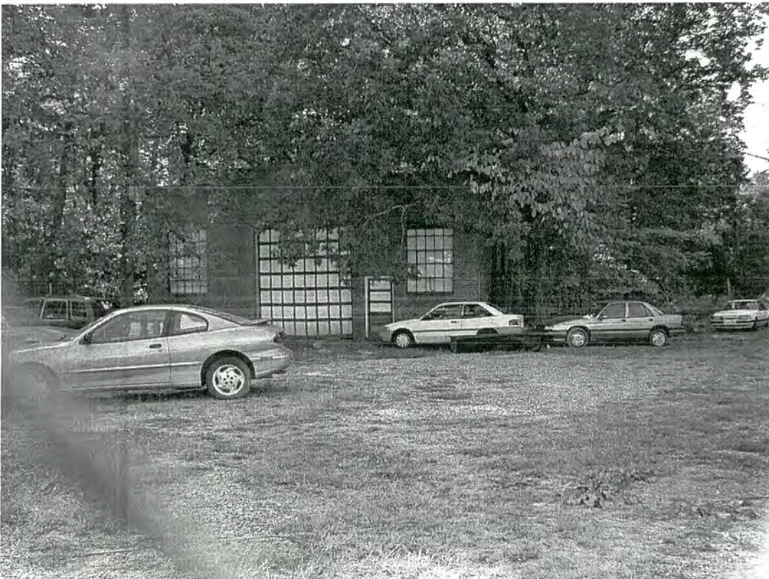
12. McCoy's Service Station - 5315 Wilkinson Blvd
