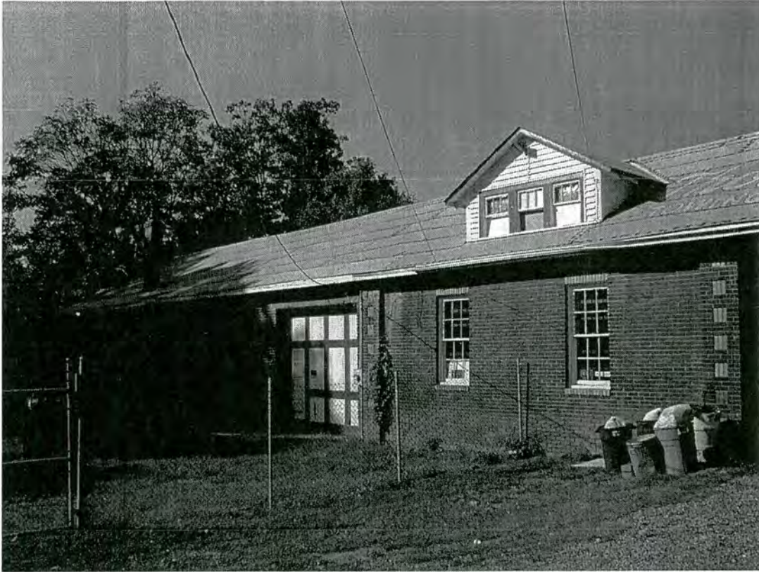
12. McCoy's Service Station - 5315 Wilkinson Blvd
