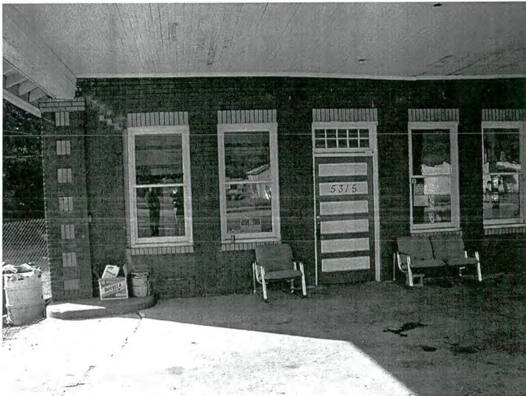
12. McCoy's Service Station - 5315 Wilkinson Blvd
