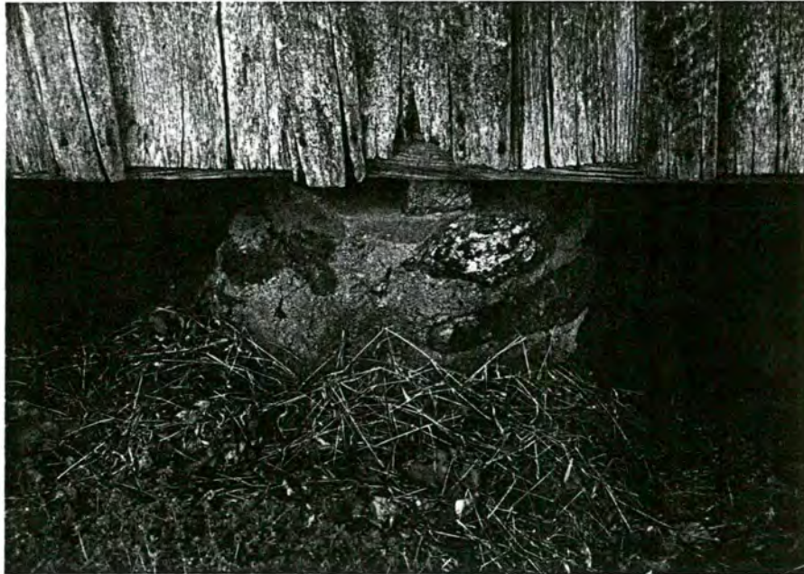
Plate 3. Stone Foundation Pier on North Elevation of Palmer Ford Mill
