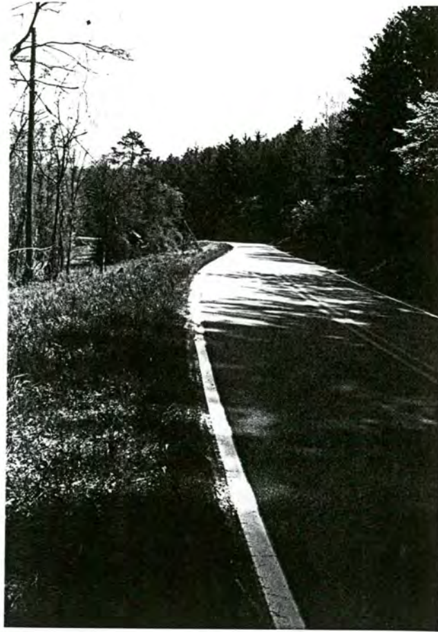
Plate 10. Approach to Bridge No. 56 from the South on SR 1250, Facing Northeast
