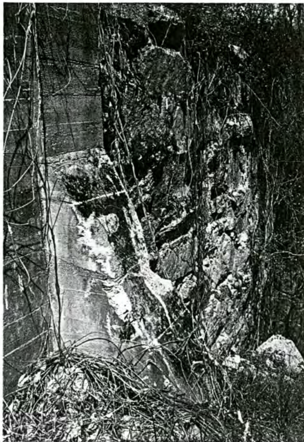
Plate 4. J.D. Pitts Dam with Detail of Concrete Abutment, Facing Northwest from South Bank of Canoe Creek
