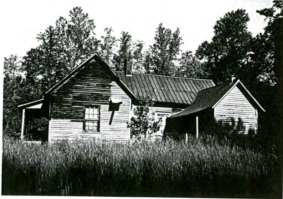
Plate 8. House No. 1, East Elevation, Facing West
