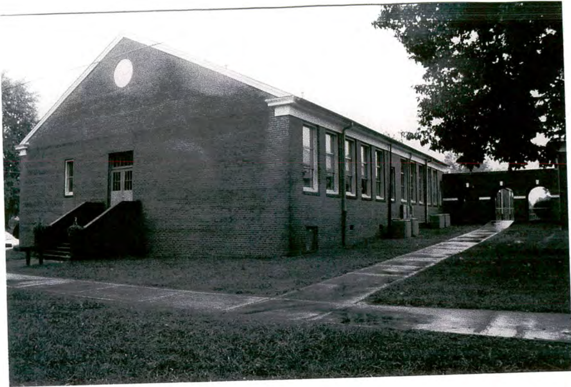
Plate 9: Former Balfour Elementary School – looking southwest
