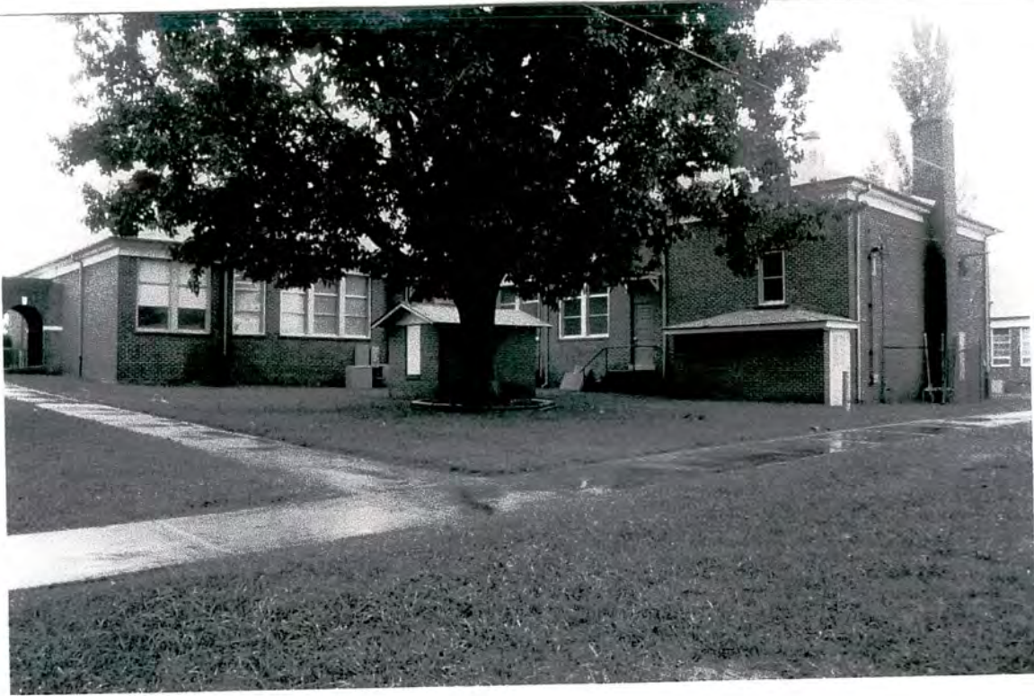
Plate 5: Former Balfour Elementary School – looking northwest
