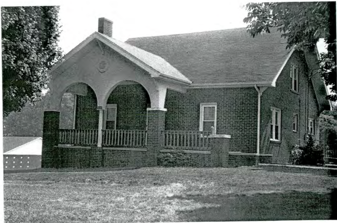
Plate 28: House (URS #6) - 1702 North Fayetteville Street/US220B, Asheboro
