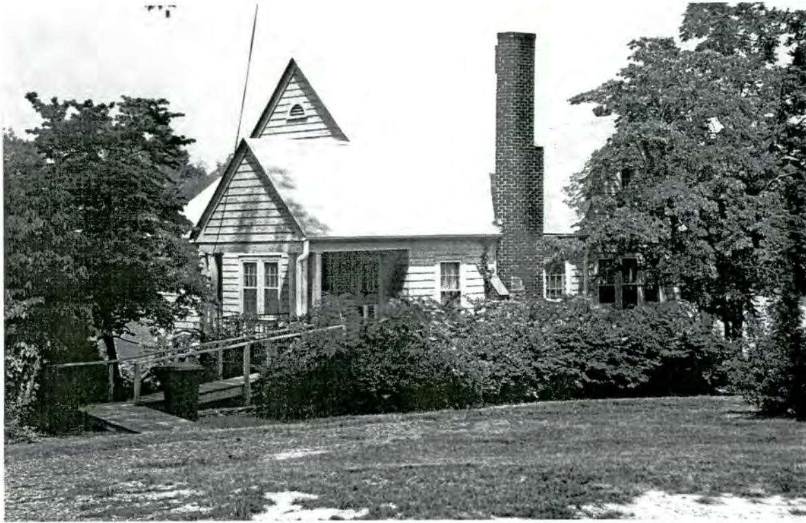
Plate 45: House (URS #24) - 2019 North Fayetteville Street/US220B, Asheboro
