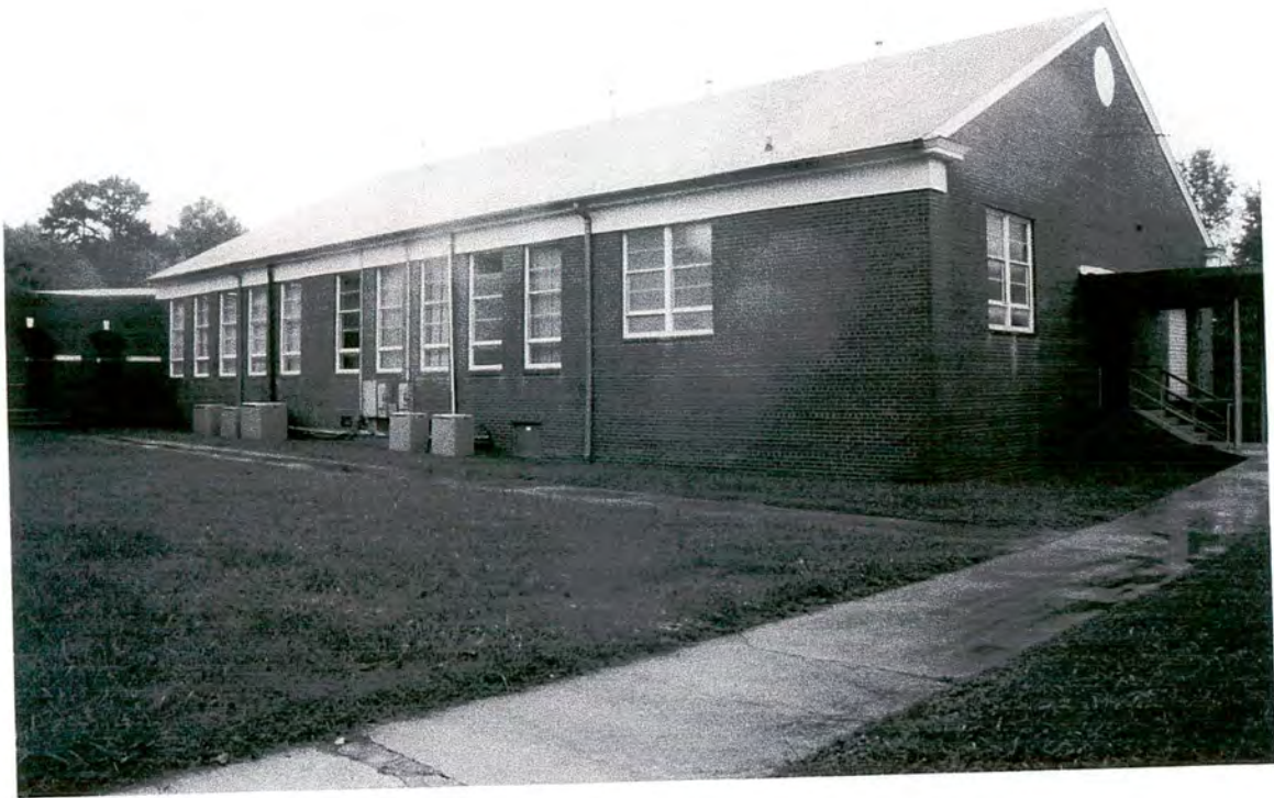
Plate 10: Former Balfour Elementary School – looking northwest
