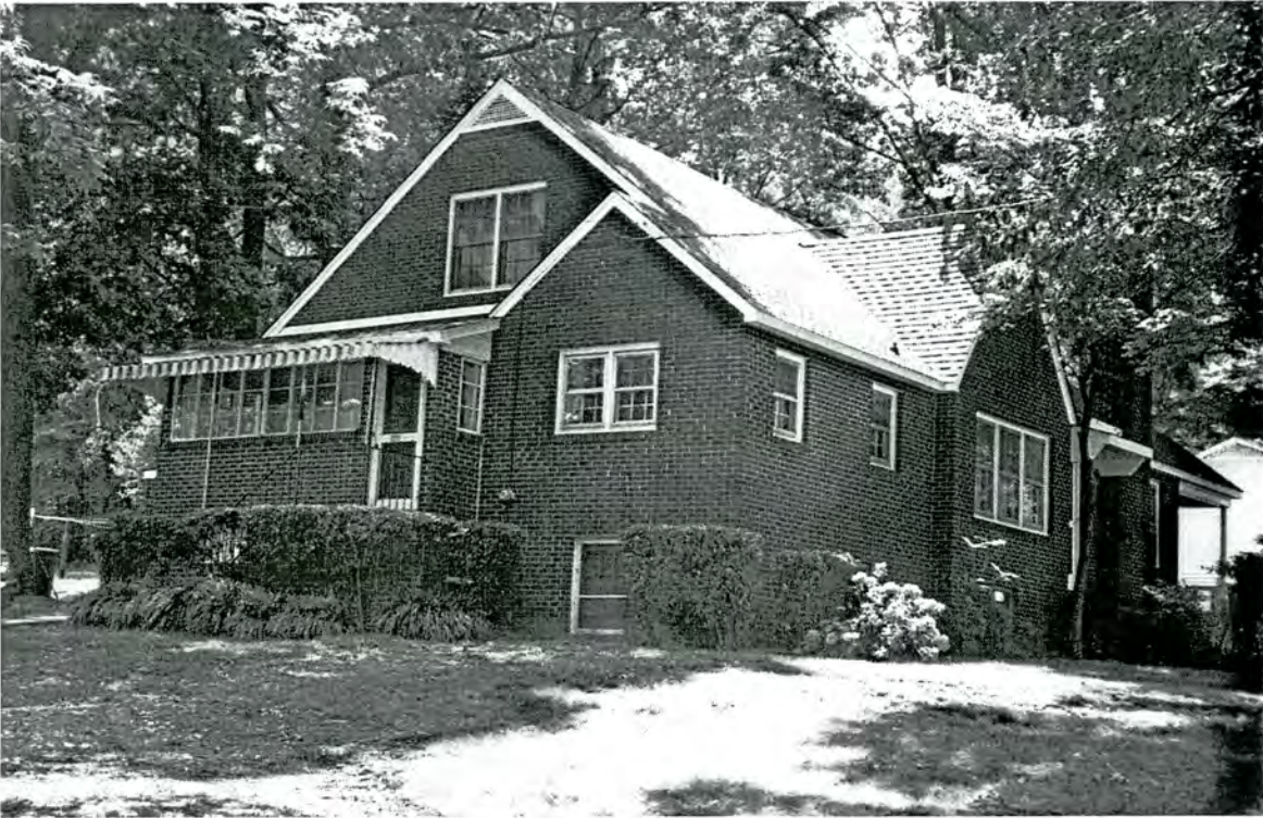
Plate 46: House (URS #25) - 2030 North Fayetteville Street/US220B, Asheboro
