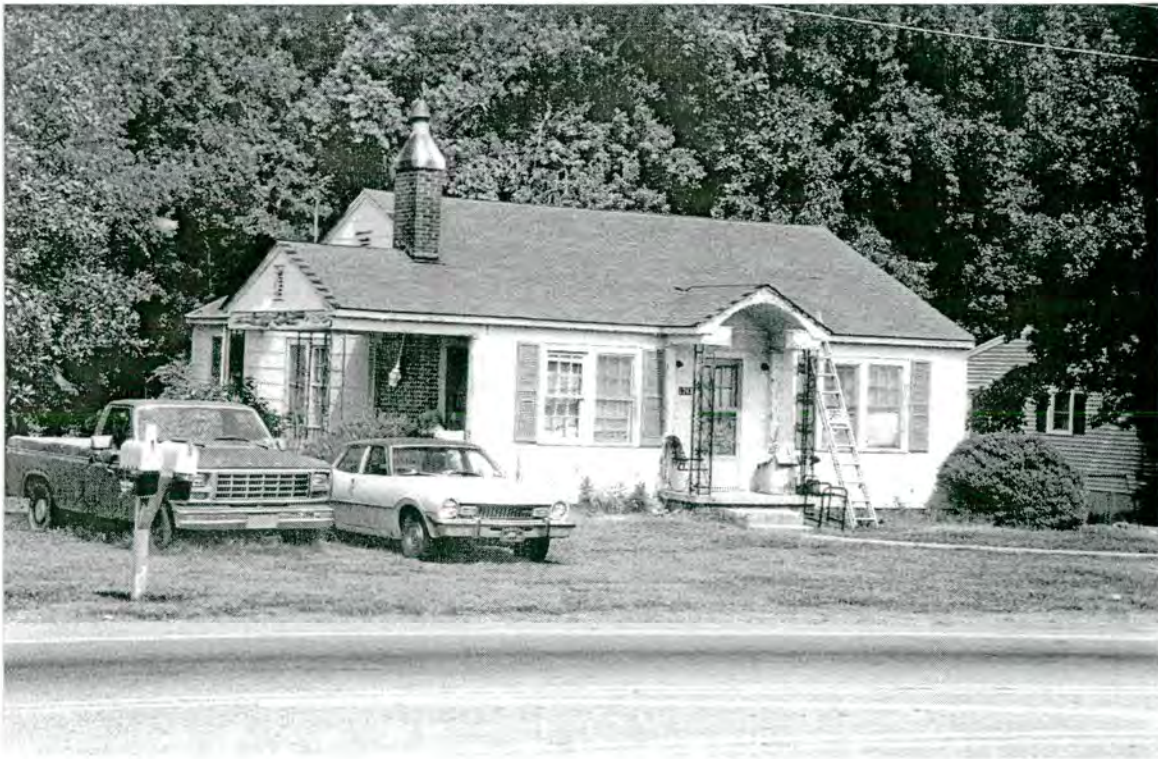
Plate 34: House (URS #12) - 1743 North Fayetteville Street/US220B, Asheboro
