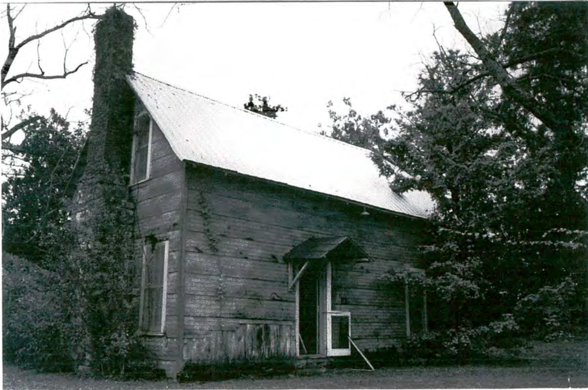
Plate 16: Pritchard House – west rear and north side elevations, looking southeast
