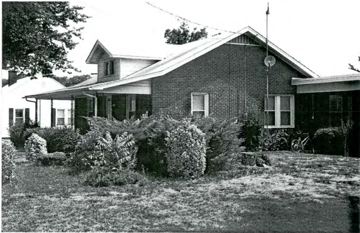
Plate 40: House (URS #19) - 1934 North Fayetteville Street/US220B, Asheboro
