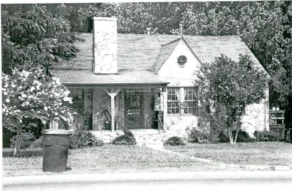
Plate 31: House (URS #9) - 1705 North Fayetteville Street/US220B, Asheboro
