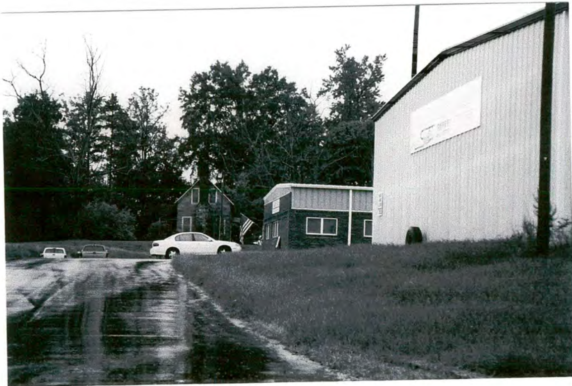
Plate 22: Pritchard House – north side elevation of house in background, looking south from modern industrial buildings.
