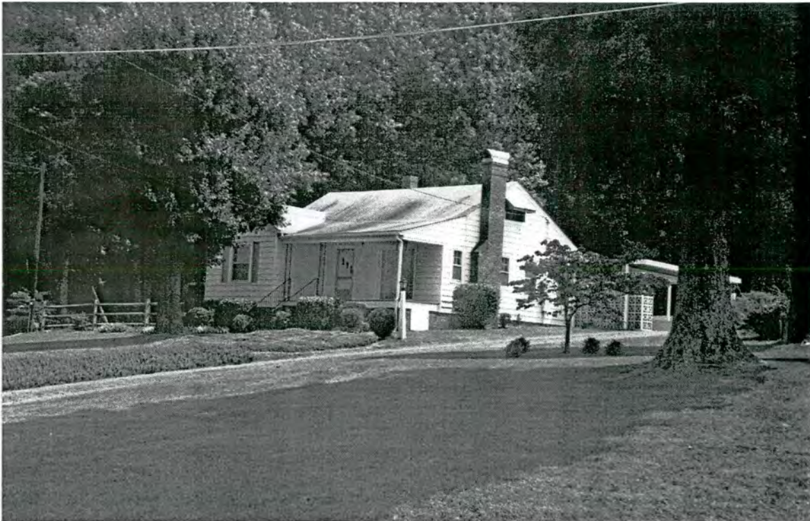
Plate 44: House (URS #23) - 2016 North Fayetteville Street/US220B, Asheboro
