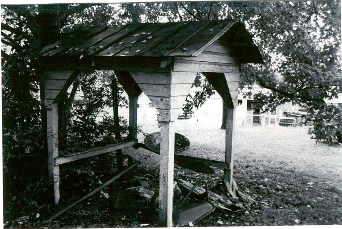
Plate 21: Pritchard House – wellhouse, looking northwest
