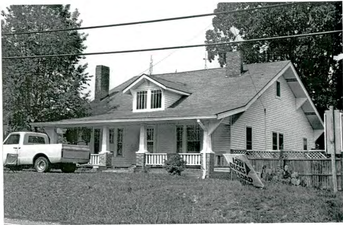
Plate 27: House (URS #5) - 1641 North Fayetteville Street/US220B, Asheboro
