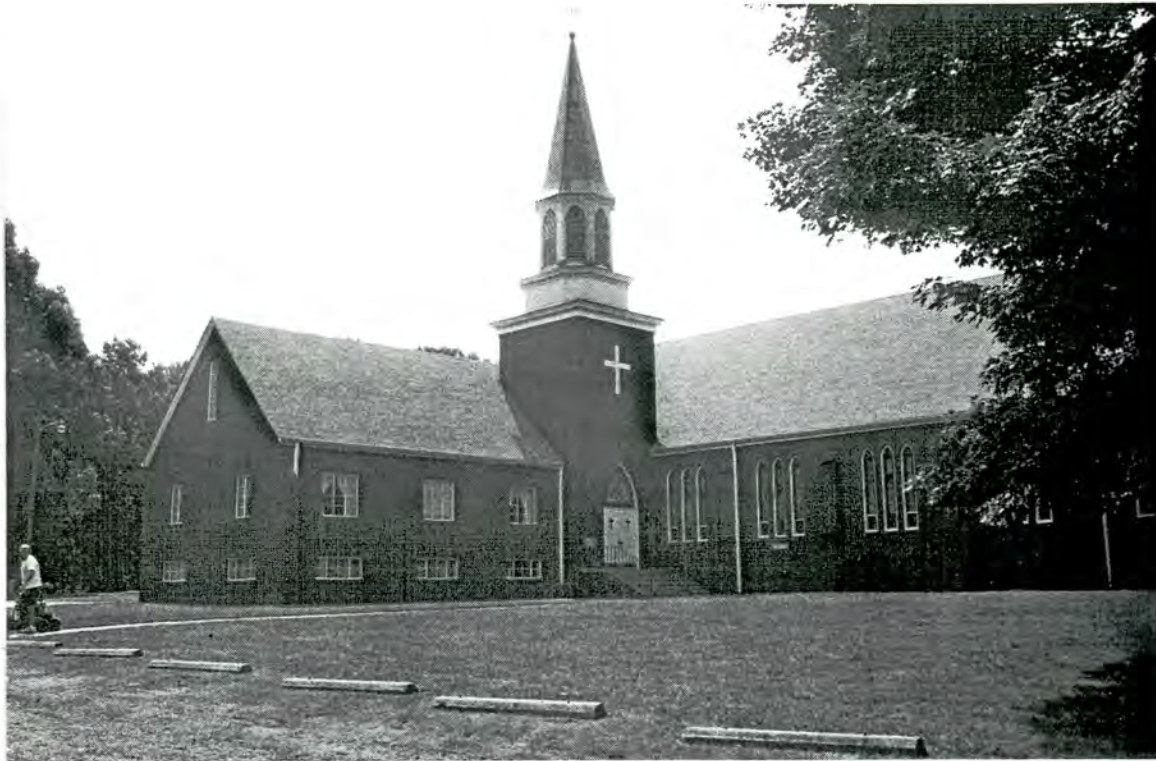
Plate 35: Calvary United Methodist Church (URS #14) (1950) – northeast corner of junction of Francis Street and North Fayetteville Street/US220B, Asheboro
