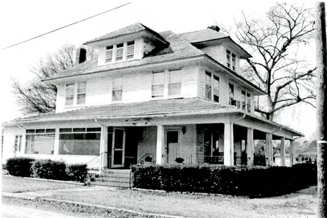
Plate 12: 218 Hillsboro Street - east front and north side elevations
