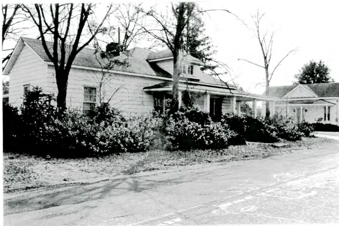
Plate 10: Stedman Baptist Parsonage (227 Hillsboro Street) at left, Horne House (301 Hillsboro Street) at right, looking southeast
