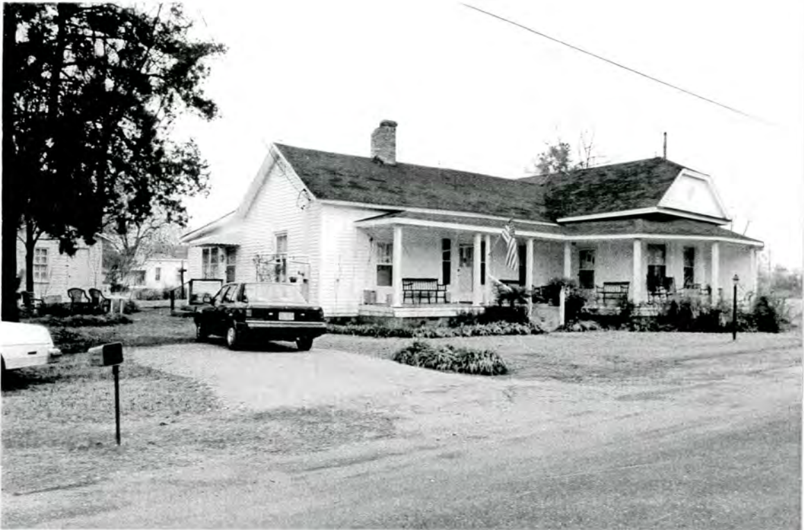
Plate 20: 312 Euclid Street - east front and south side elevations
