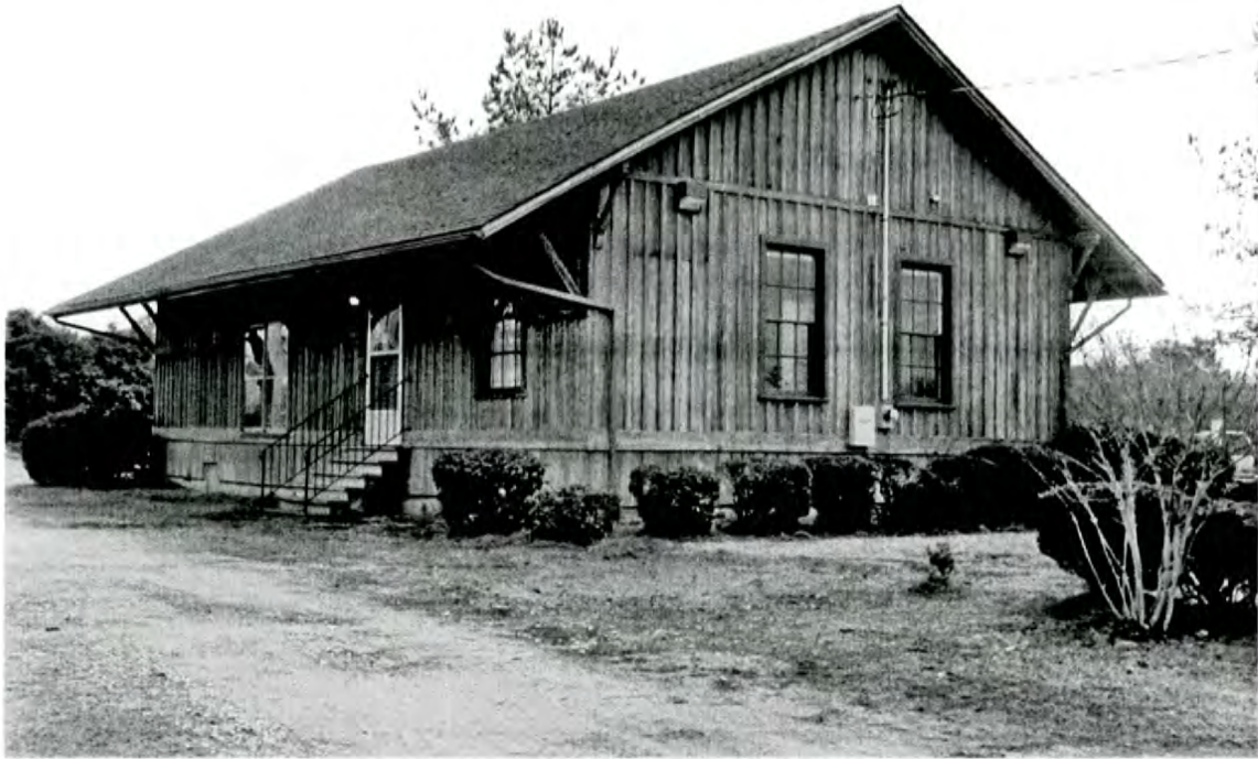
Plate 1: Cape Fear & Yadkin Valley Railroad Depot (193 Euclid Street), looking southeast
