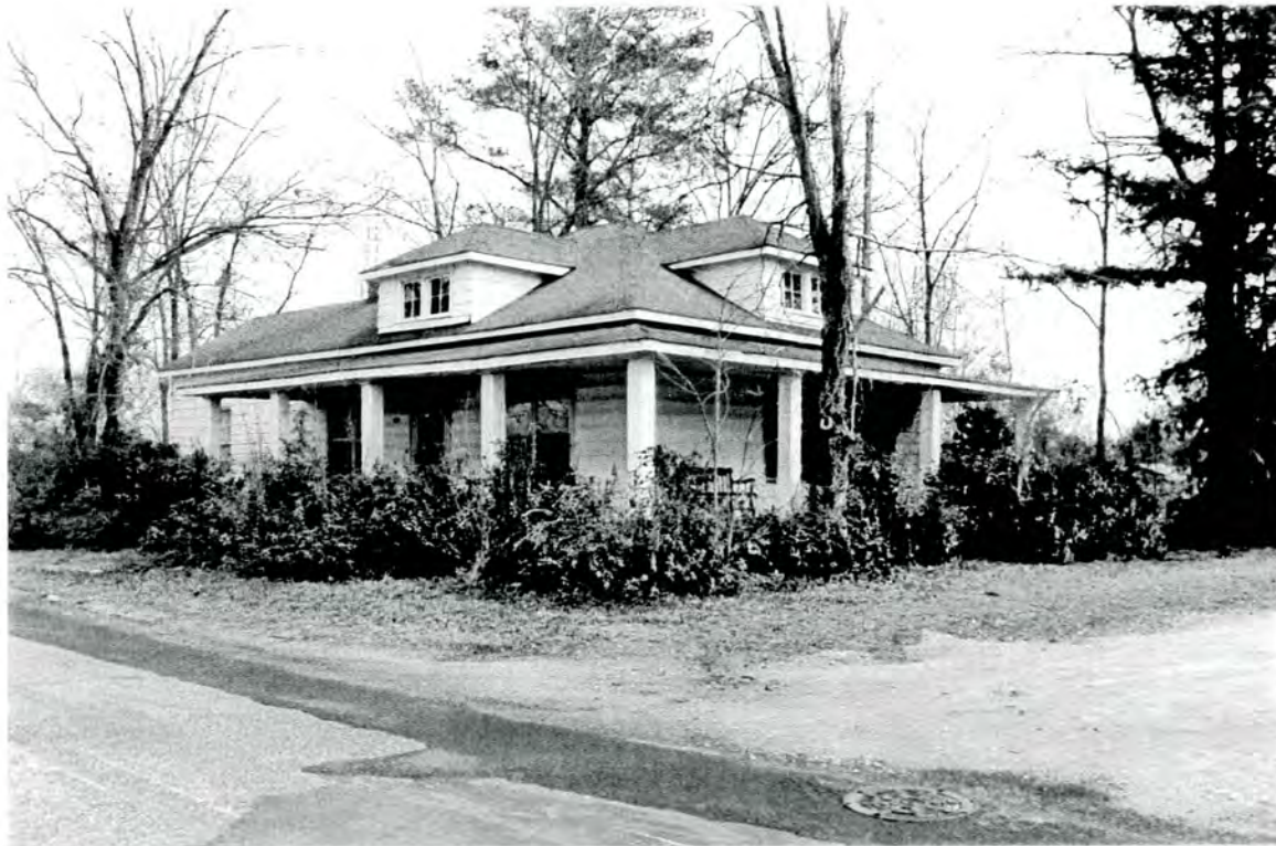
Plate 14: 227 Hillsboro Street - west front and south side elevations
