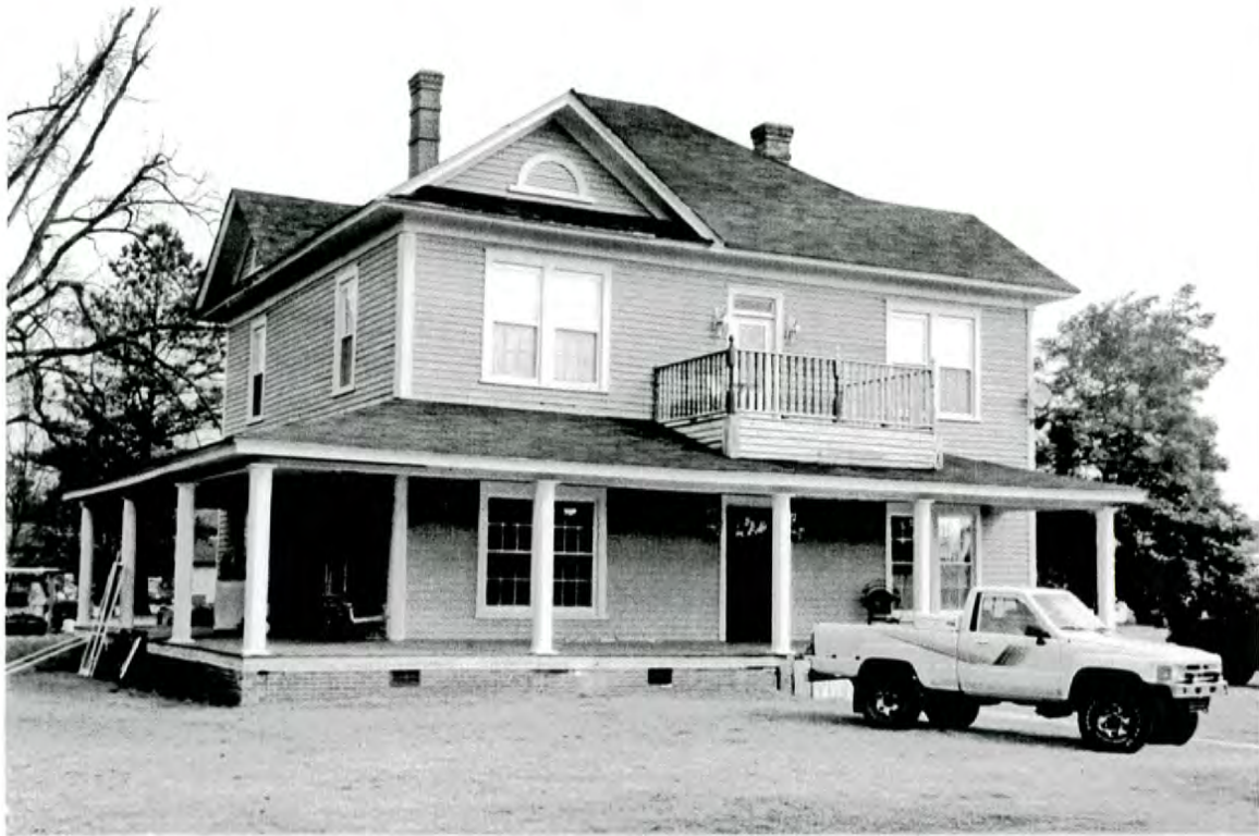
Plate 28: 174 East First Street - south front and west side elevations
