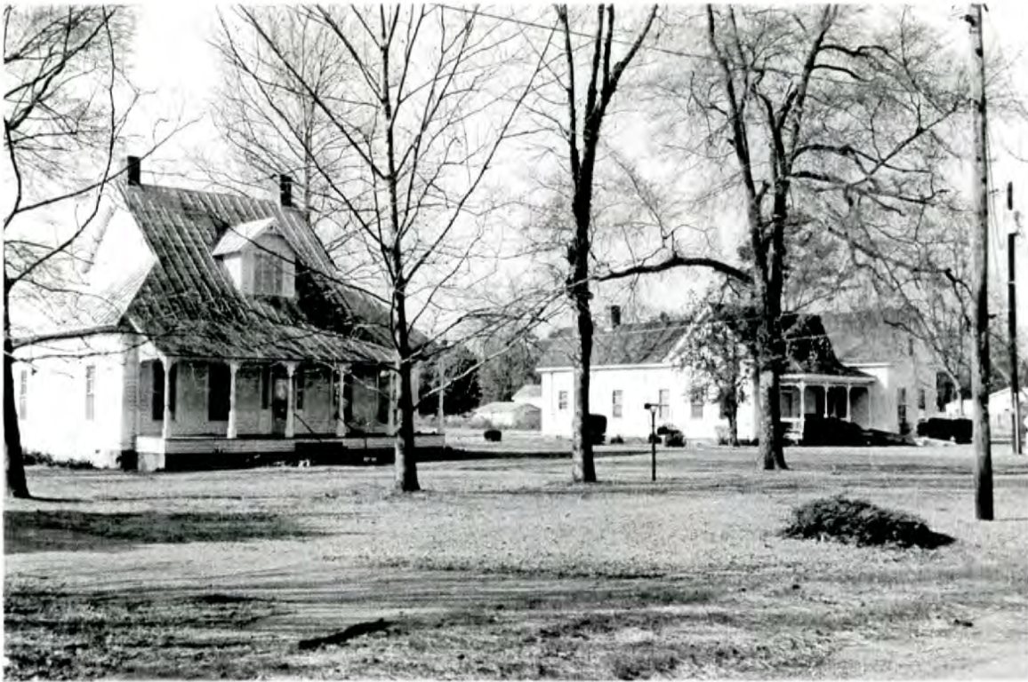
Plate 7: Sessoms House (5100 Jefferson Street) at left, Methodist Parsonage (232 Euclid Street) at right, looking southwest
