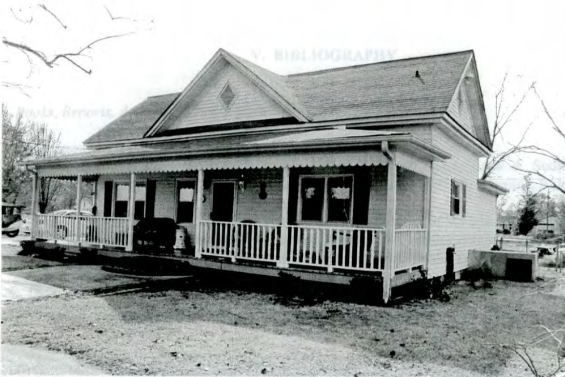
Plate 37: 5040 Blanche Street - north front and west side elevations
