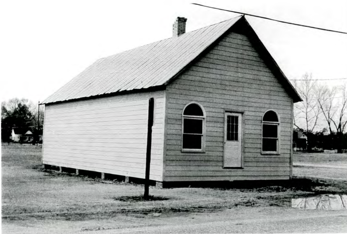
Plate 32: 5050 Front Street - north front and east side elevations
