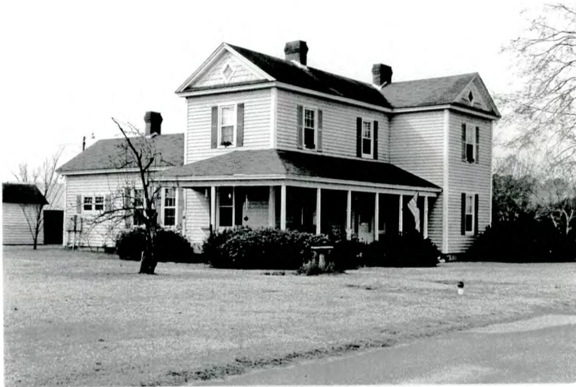
Plate 30: 5026 Front Street - north front and east side elevations
