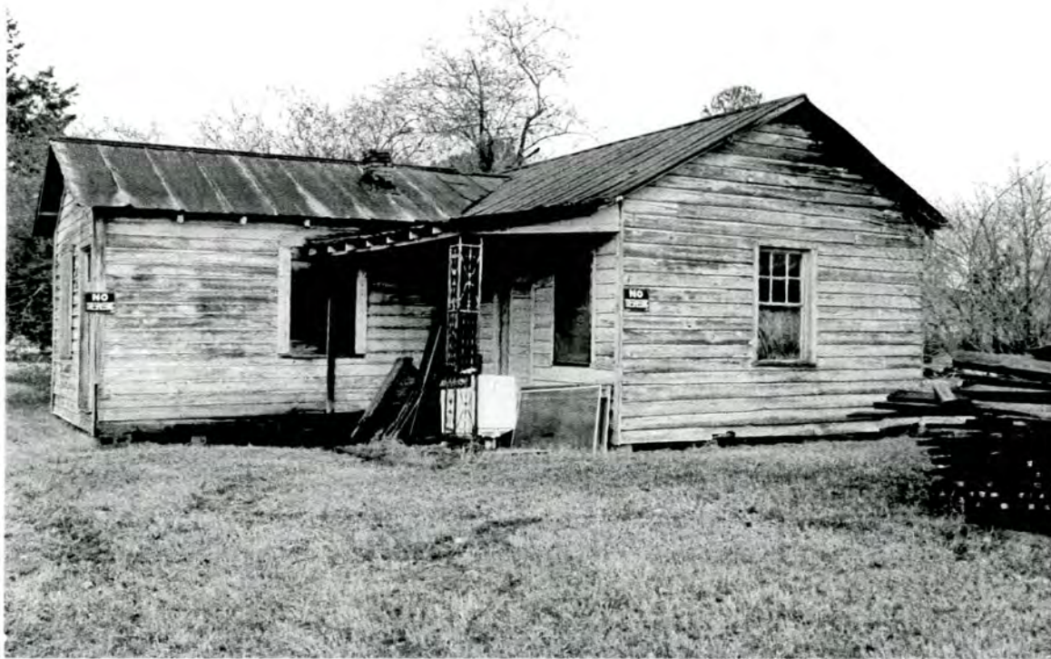
Plate 21: 1** Euclid Street, immediately north of 183 Euclid Street - looking northwest
