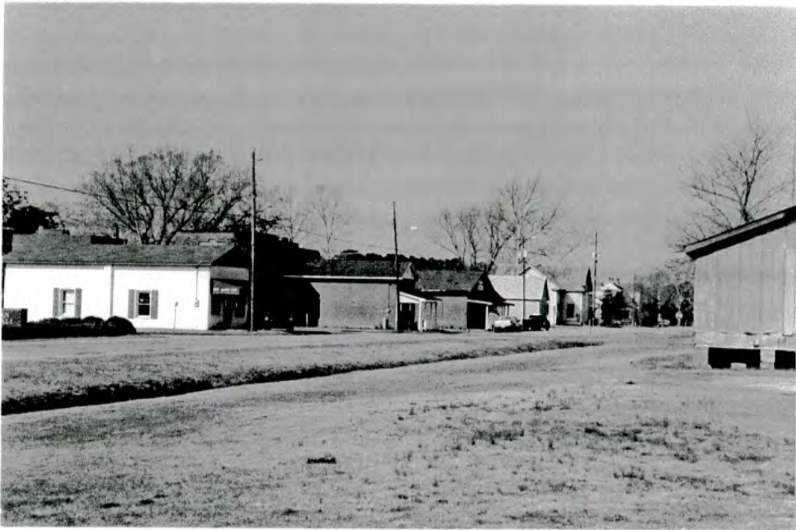
Plate 5: Later commercial buildings at 5102, 5070, and 5064 Front Street at left, looking southwest
