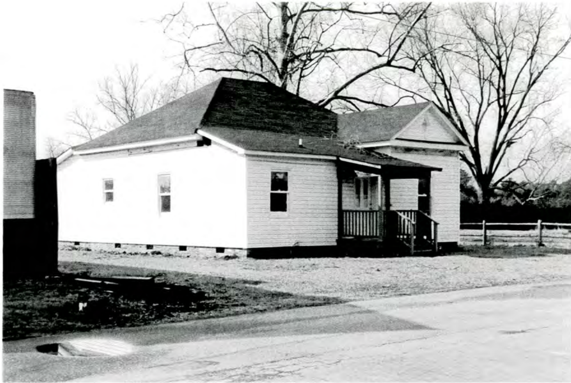
Plate 31: 5042 Front Street - north front and east side elevations
