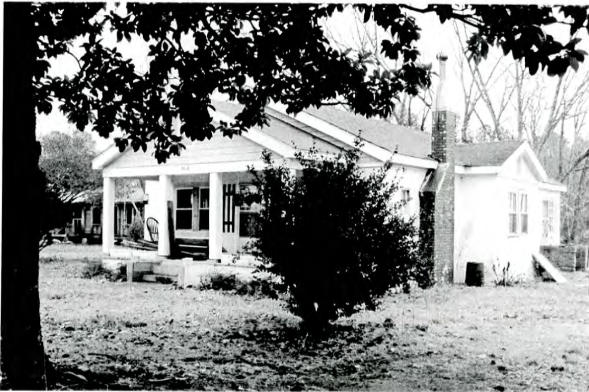
Plate 36: 5118 Jefferson Street - north front and west side elevations
