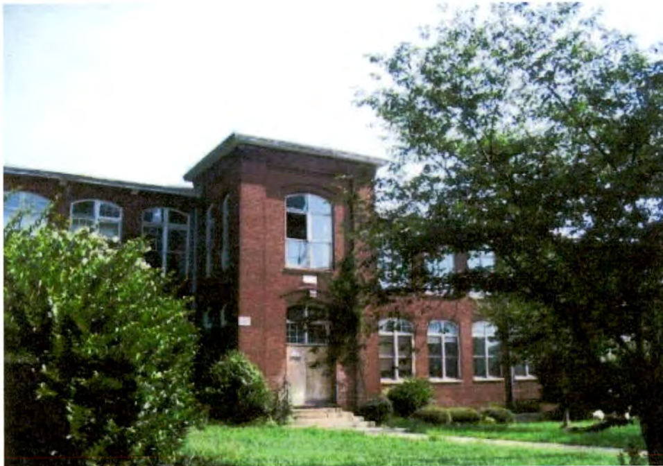
Plate 111. North Charlotte Historic District, Mecklenburg Mill, Looking North.
