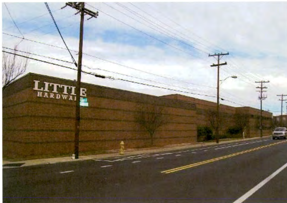
Little Hardware (No. 27), 1400-1416 South Mint Street, Looking North.
