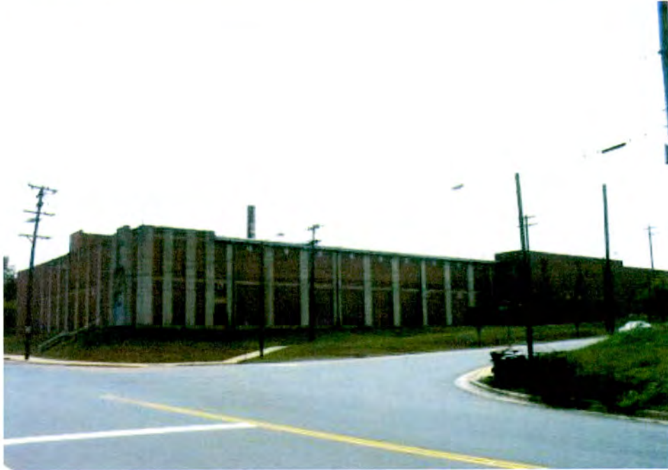
Plate 108. Chadbourn Hosiery Mills, Overall View, Looking Northeast Along North Brevard Street.
