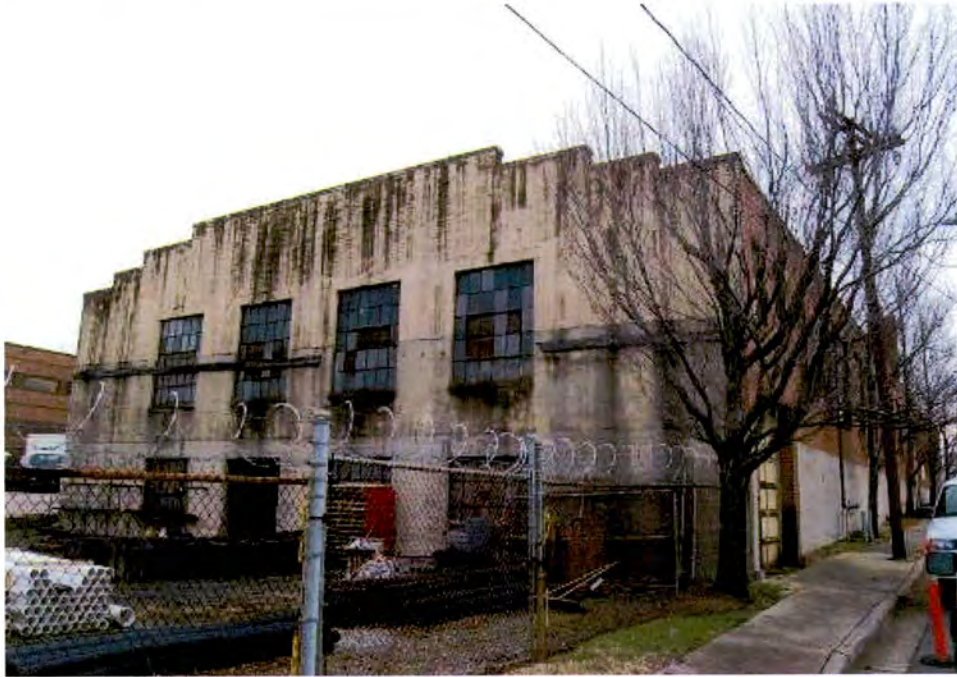
Little Hardware (No. 27), 1400-1416 South Mint Street, Warehouse Section, Looking East.
