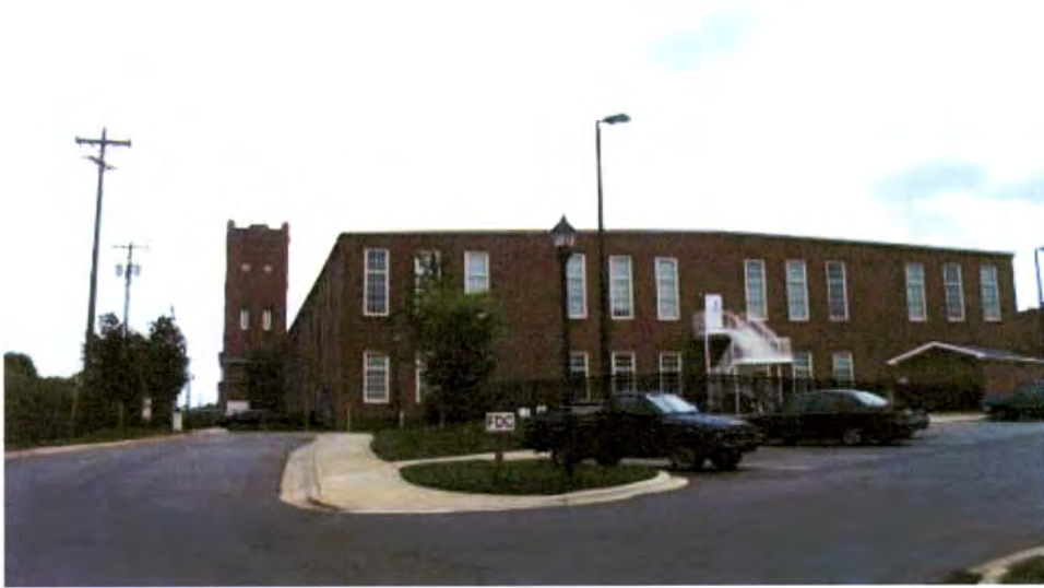
Plate 112. North Charlotte Historic District, Highland Park Manufacturing Company Mill No. 3, Looking Northeast.
