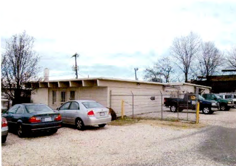
H&S Roofing Company Office Building (No. 24), 506 West Summit Ave., Looking North.
