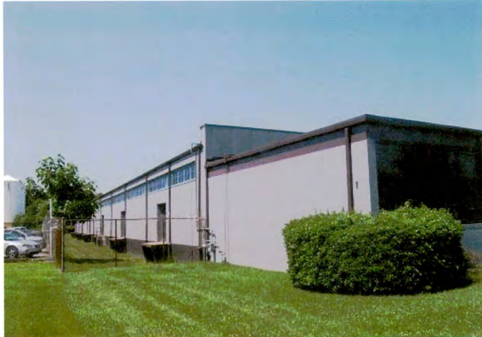
Warehouse (No. 1), 4403 Wilkinson Boulevard, West Elevation, Looking South.
