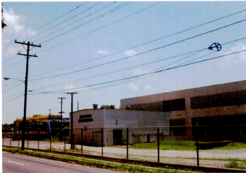
Plate 13. Southern Engineering Company, Looking Southeast.
