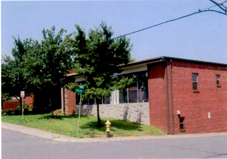
Office Building (No. 34), 1200 South Graham Street, Looking South.
