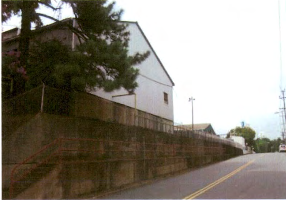
Plate 68. Charlotte Pipe and Foundry Company Complex, Looking Southwest Along South Clarkson Street.
