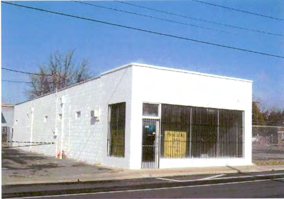
Warehouse (No. 32), 1212 South Mint Street, Looking Northwest.
