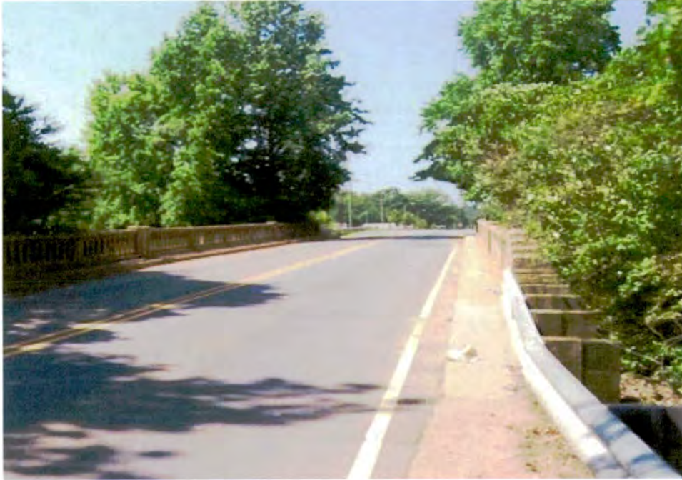
Morris Field Drive Bridge (No. 3), Looking South
