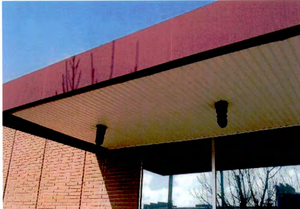
Office Building (No. 34), 1200 South Graham Street, Front Awning.
