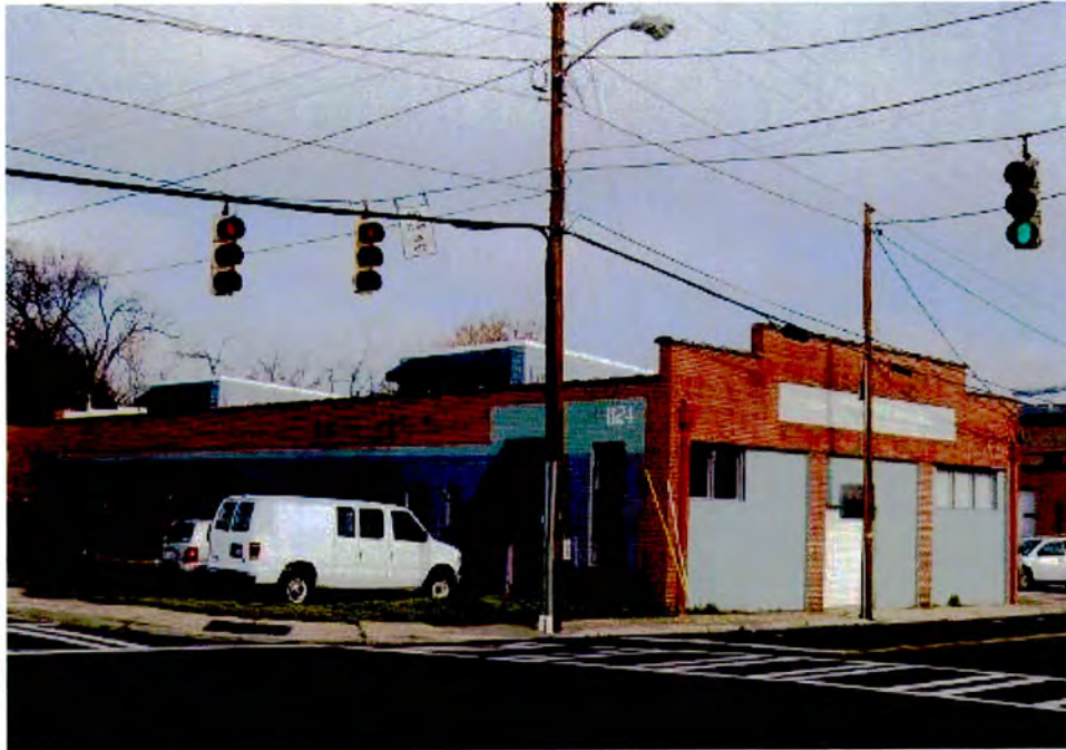
Warehouse (No. 33), 1124 South Mint Street, Looking North.
