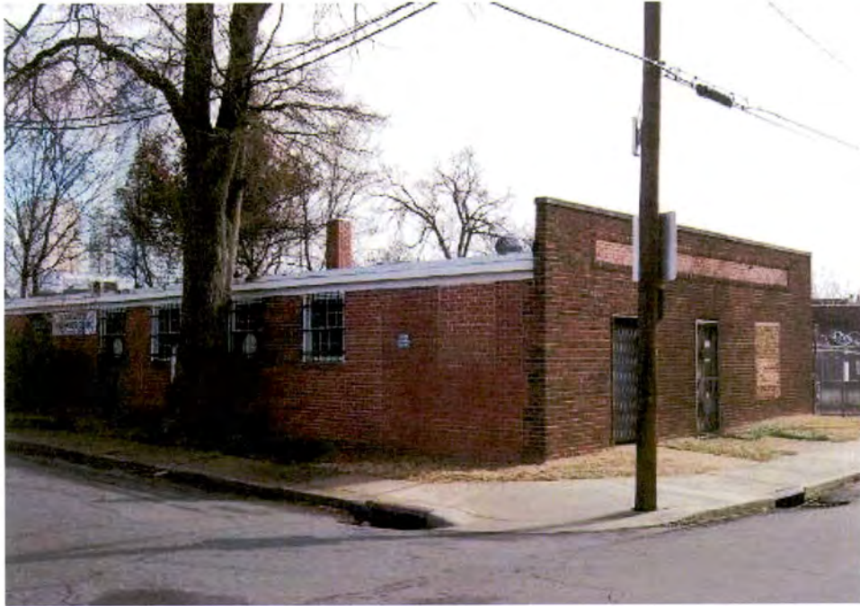
Charlotte Saw and Knife Company Building (No. 36), 418 West Palmer Street, Looking East.
