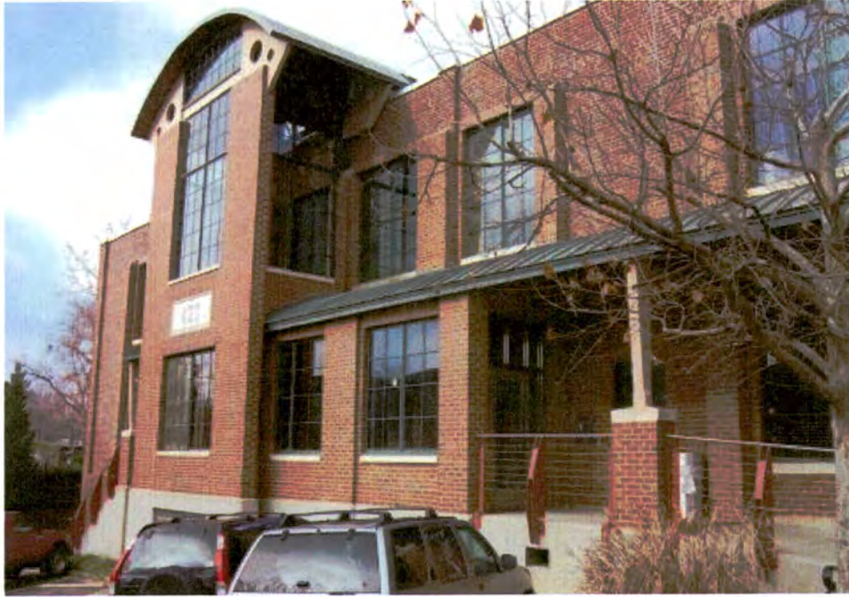
Plate 78. Electrical Supply and Equipment Company Building, East Elevation, Looking West.
