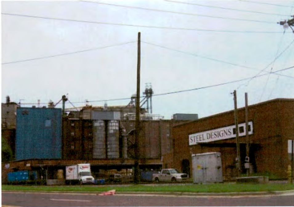
Plate 91. Seaboard Street Historic District, John B. Ross Bag Company Warehouse and Interstate Mills, Looking Southeast.
