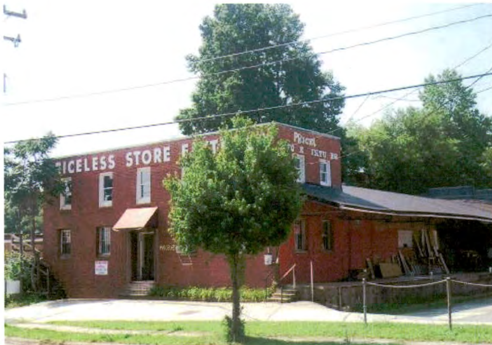
Warehouse (No. 16), 2201 Wilkinson Boulevard, Looking South.
