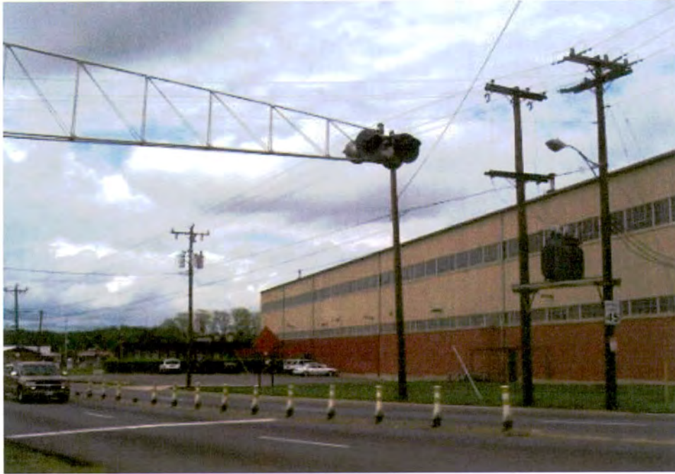
Plate 122. Republic Steel Corporation Plant, Overall View, Looking North From Railroad Corridor.
