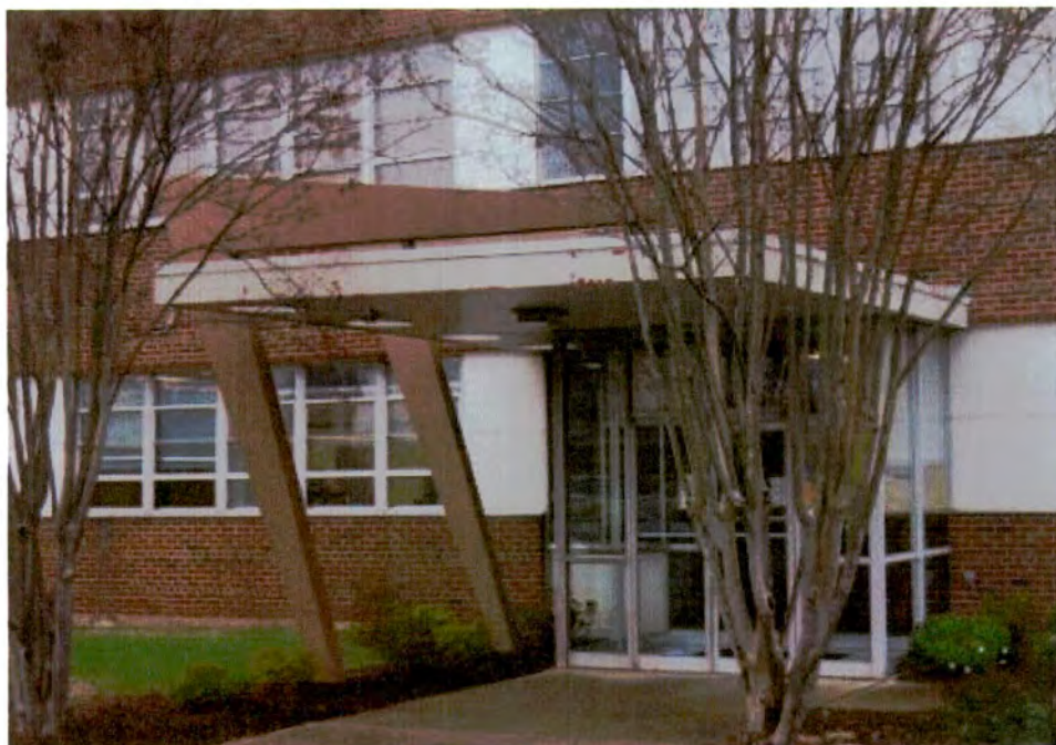
Plate 100. Standard Trucking Company Terminals, 1960 Terminal, Entrance, Looking East.
