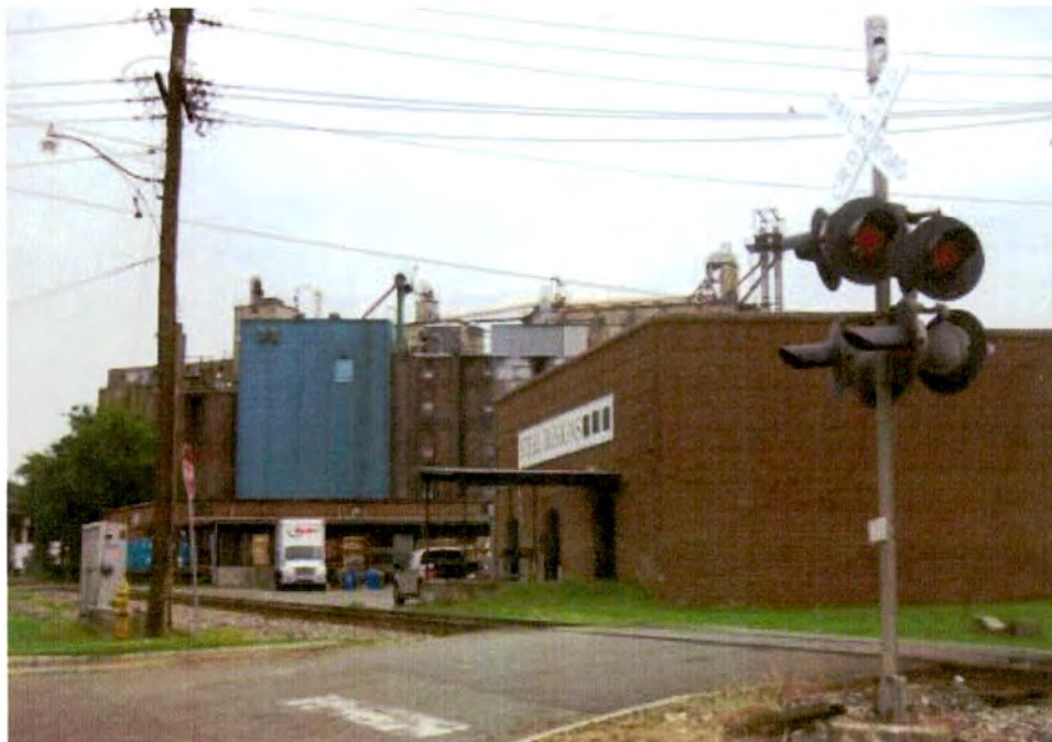
Plate 92. Seaboard Street Historic District, John B. Ross Company Warehouse and Interstate Mills, Looking East.
