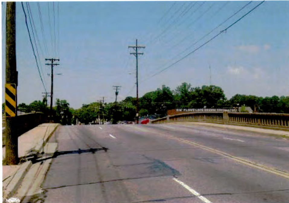
Remount Road Bridge (No. 11), Looking North.
