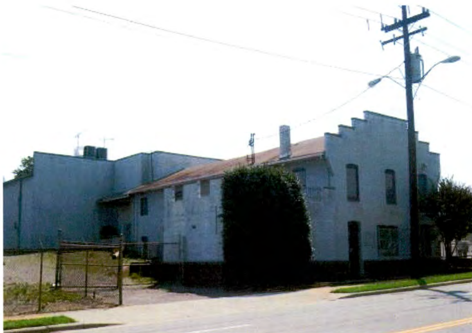
North Carolina Highway Commission Garage and Warehouse (MK2231) (No. 21), 632 West Summit Avenue, Looking East.
