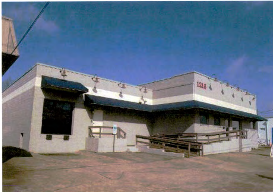
Warehouse (No. 31), 1216 South Mint Street, Looking North.
