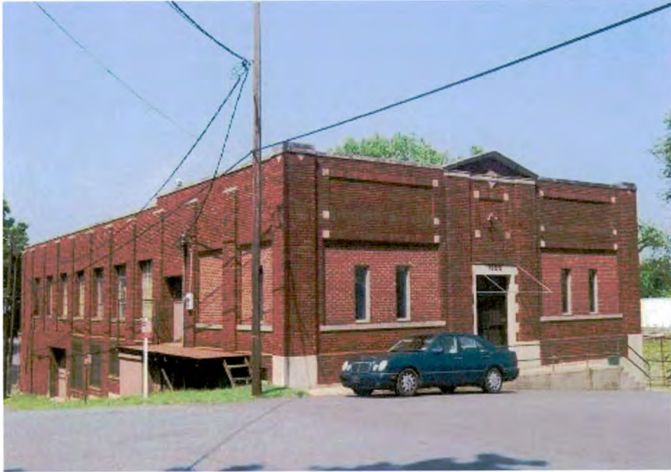
Cathey Lumber Company Warehouse (MK 2252) (No. 29), 501 Penman Street, Looking South.
