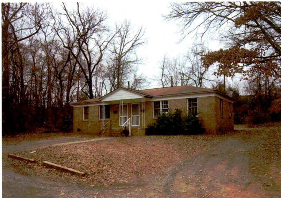
Plate 41. Westover Hills, 1400 Bethel Road (Within APE), Looking North.
