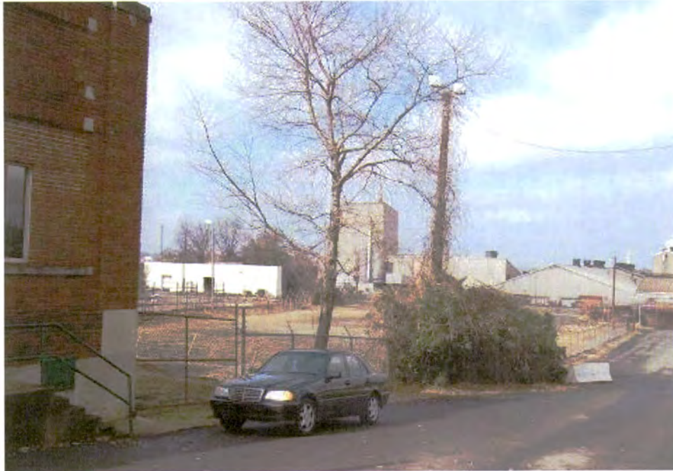
Cathey Lumber Company Warehouse (MK 2252) (No. 29), 501 Penman Street, Looking West Towards Former Lumber Yard.
