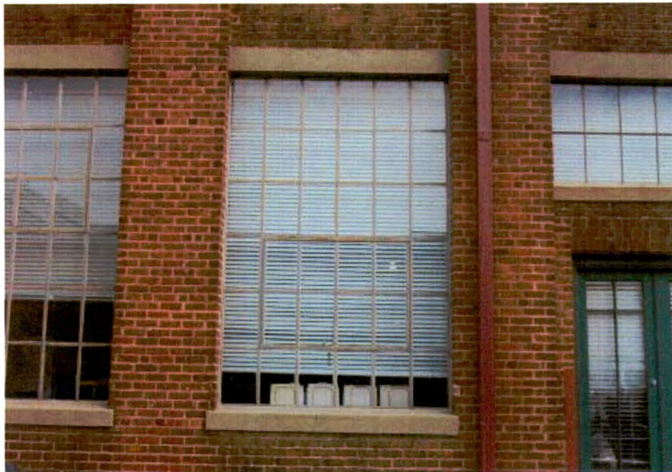
Plate 73. Textile Mill Supply Company Building, Windows, South Elevation, Looking North.
