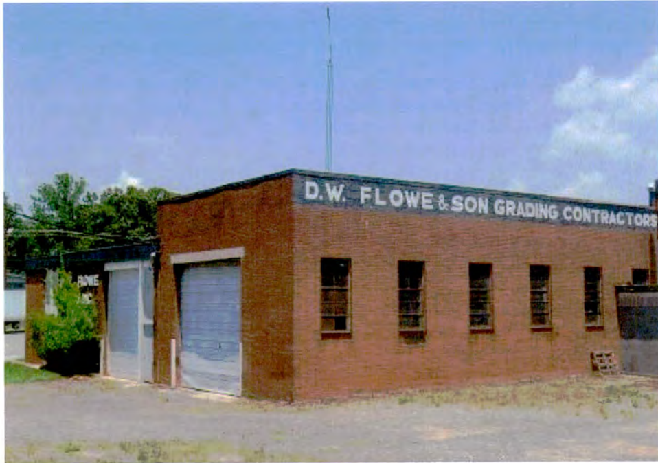
Commercial Building (No. 10), 2020 Remount Road, Looking West.
