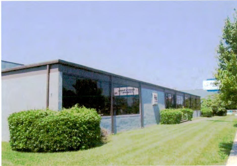
Warehouse (No. 1), 4403 Wilkinson Boulevard, Office, Looking West.
