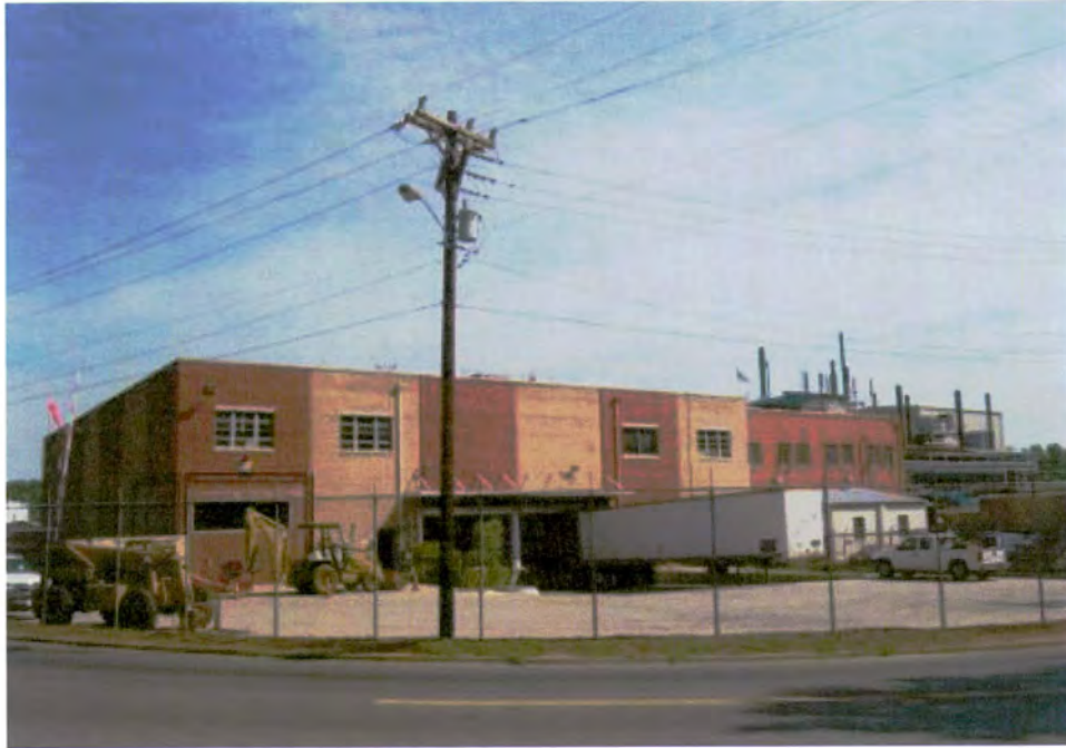
Plate 126. Wica Chemical Company Plant, 1966 Warehouse/Production Addition (1956 Warehouse On East/Right Side), Looking North.
