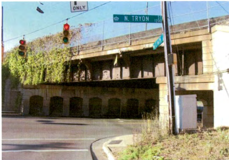
Plate 94. Southern Railway Bridge, North Tryon Street, Looking West.
