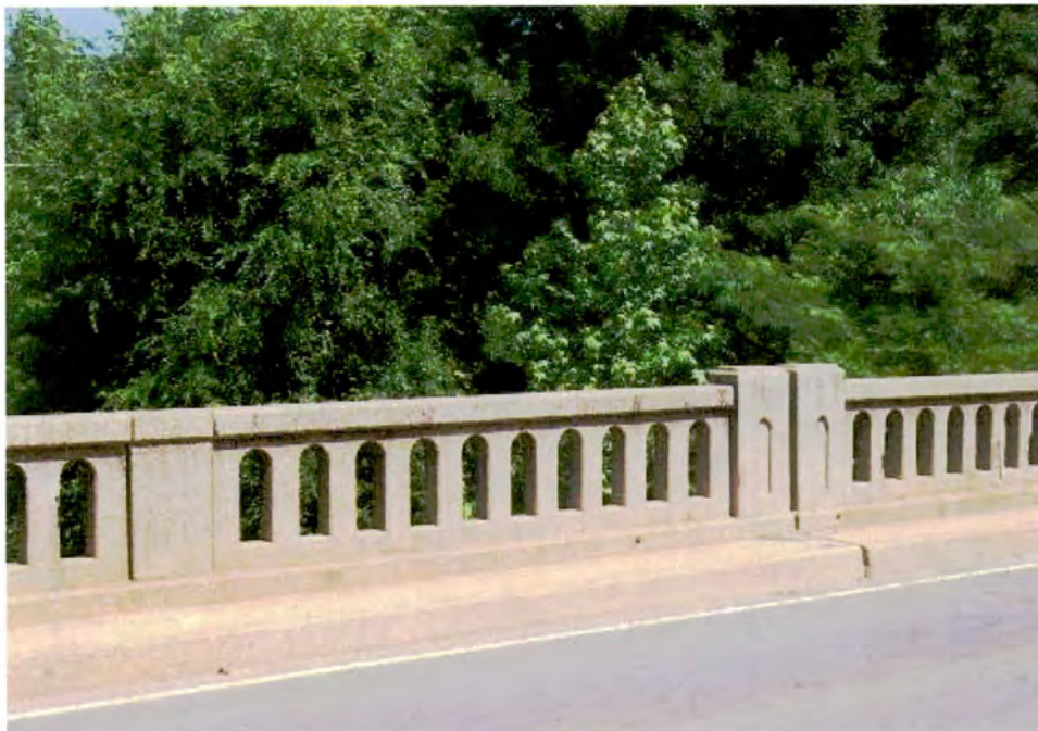
Morris Field Drive Bridge (No. 3), Balustrade, Looking West
