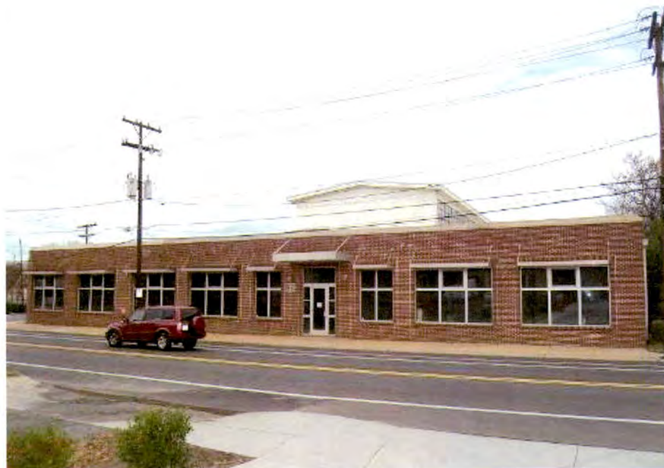
Industrial Building (No. 25), 1430 Mint Street, Looking West.
