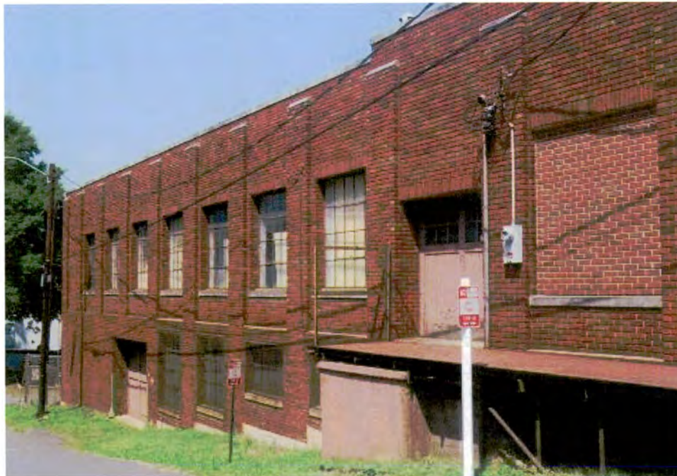
Cathey Lumber Company Warehouse (MK 2252) (No. 29), 501 Penman Street, Looking Southwest.
