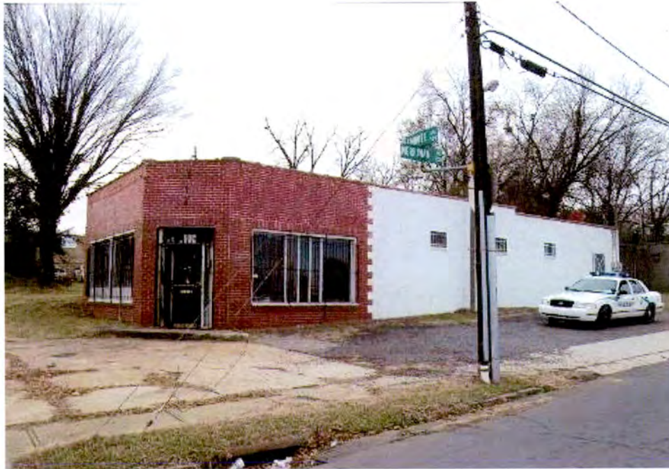
Store (No. 22), 529 West Summit Ave., Looking South.
