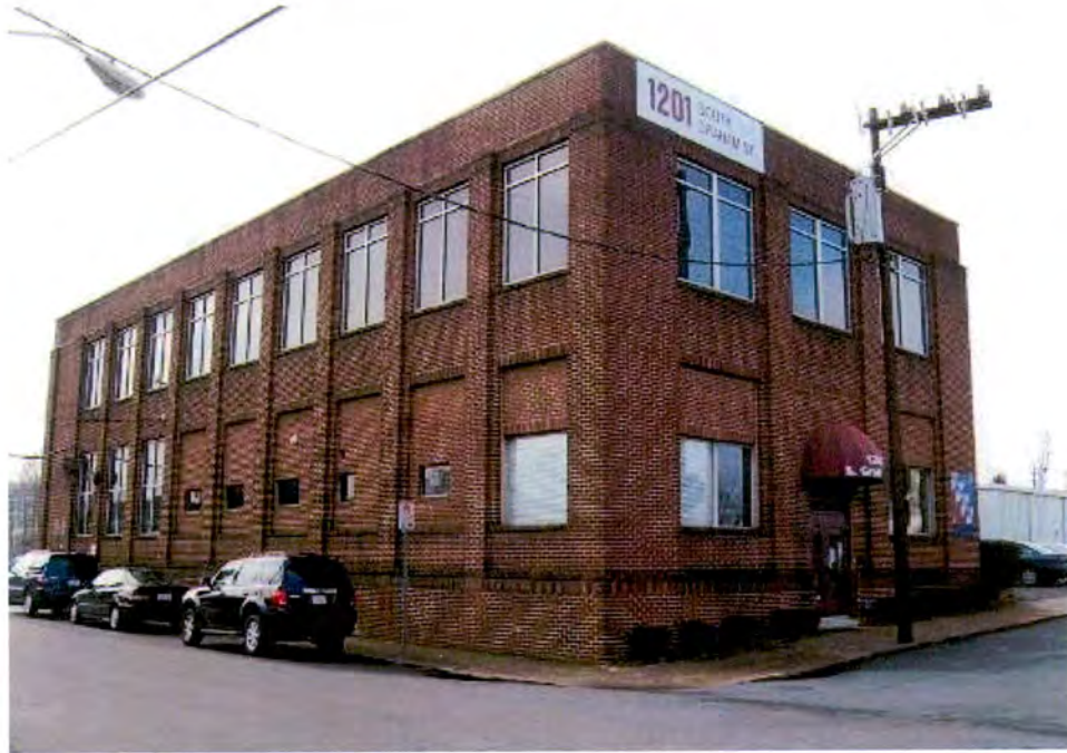
Ashworth Brothers Inc. Warehouse (MK 2255) (No. 35), 1201 South Graham Street, Façade and North Elevation, Looking Southeast.
