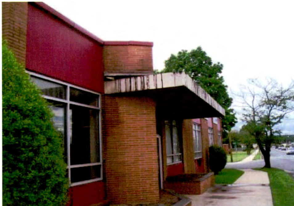
Plate 119. Standard Chemical Products Plant, Office, Front (East) Elevation, Looking North.
