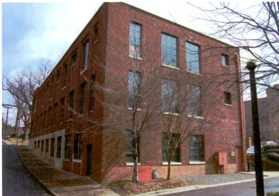
Plate 79. Electrical Supply and Equipment Company Building, Rear and West Elevations, Looking North.
