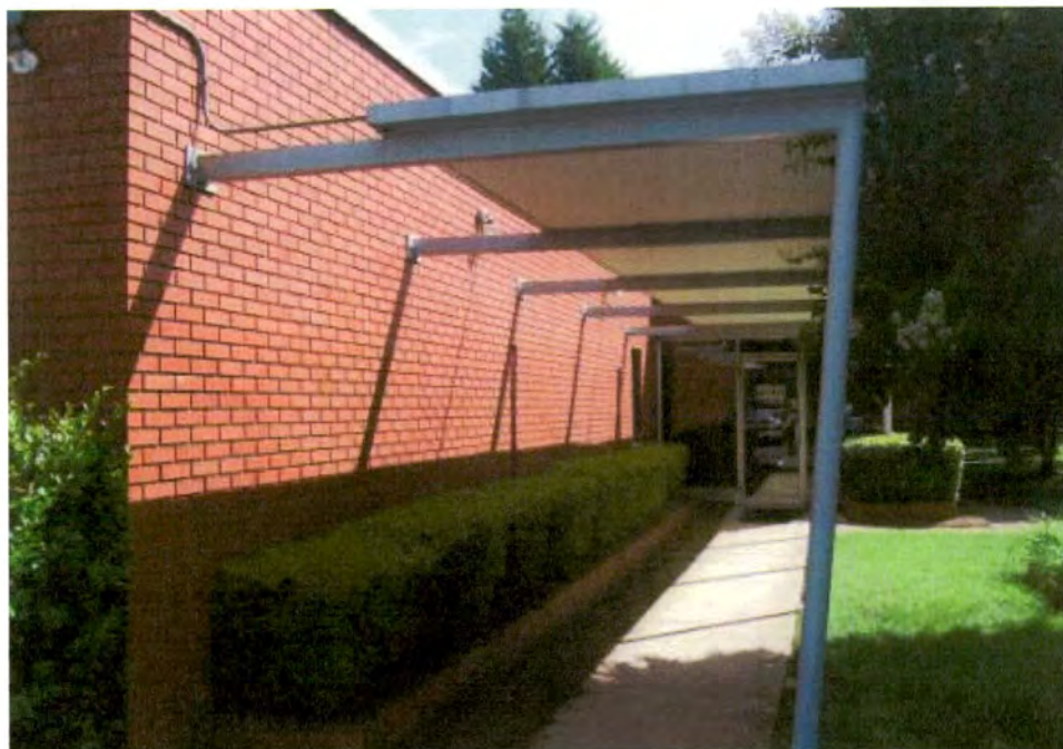
Plate 129. Wica Chemical Company Plant, 1956 Office Canopy, Looking East Towards Entrance.
