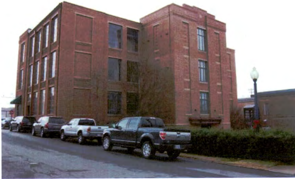
Plate 74. Textile Mill Supply Company Building, Modern Addition, Looking East.
