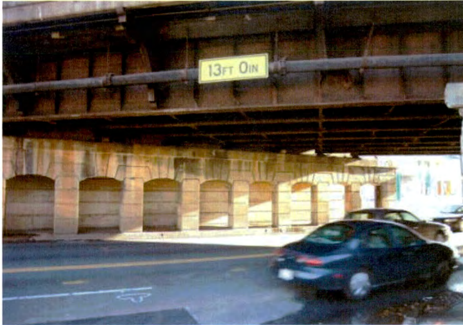
Plate 95. Southern Railway Bridge, North Tryon Street, Looking Southeast.
