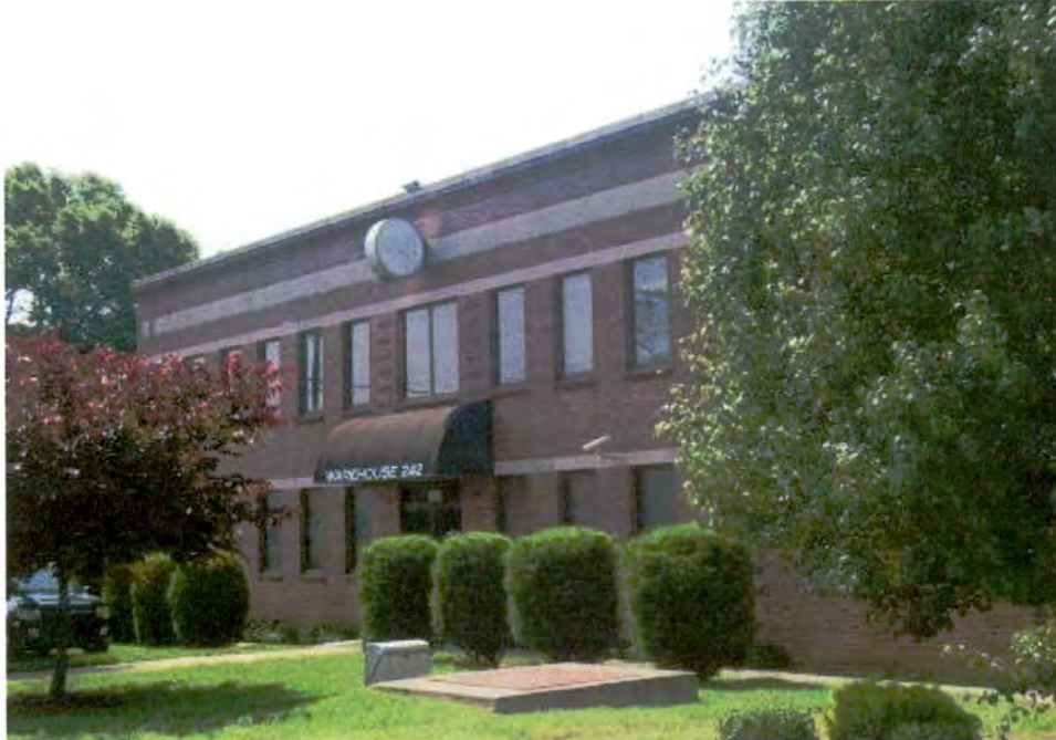
Warehouse (No. 15), 2307 Wilkinson Boulevard, Looking South.
