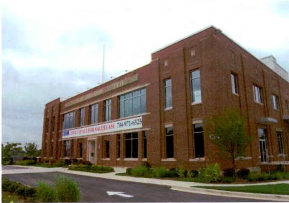
Plate 23. General Dye Stuffs Corporation Building, Façade (North Elevation), Looking Southeast.
