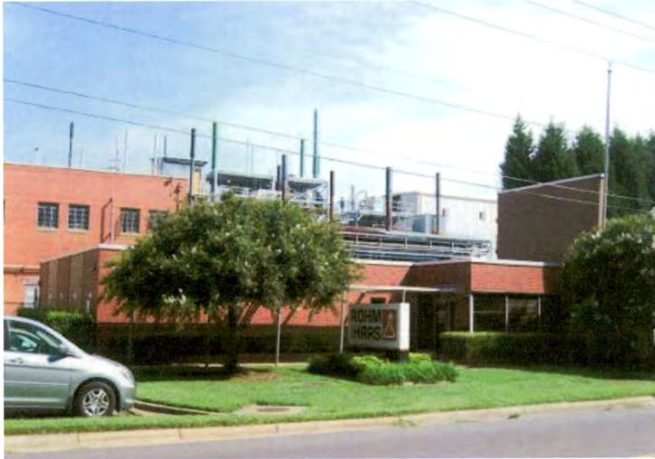
Plate 128. Wica Chemical Company Plant, 1956 Office, Looking Northeast.
