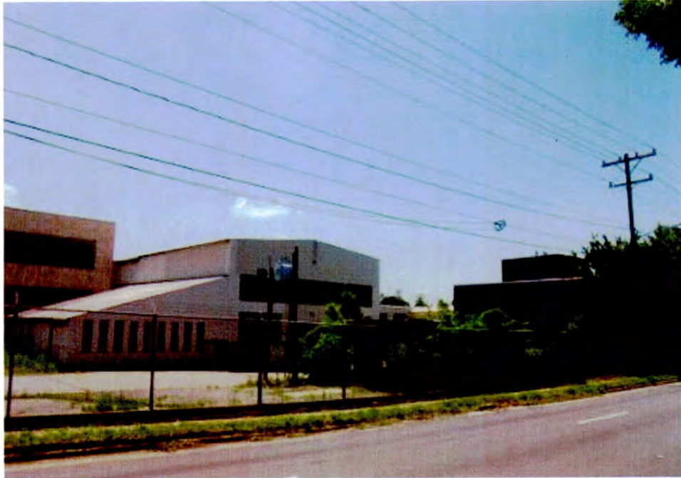
Plate 14. Southern Engineering Company, Office and Fabrication Buildings, Looking Southwest.
