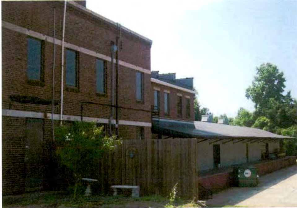
Warehouse (No. 15), West Elevation, 2307 Wilkinson Boulevard, Looking South.
