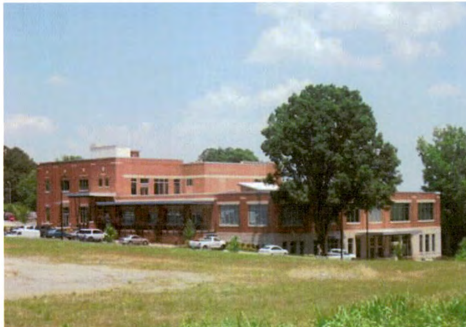
Plate 26. General Dye Stuffs Corporation Building, Rear and West Elevations, Looking Northeast.
