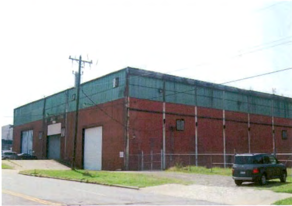
Warehouse (No. 18), 1515 South Clarkson Street, Looking East.
