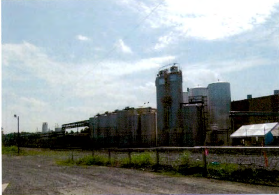
Plate 132. Wica Chemical Company Plant, Modern Storage Tanks Along Rail Corridor, Looking Southeast.
