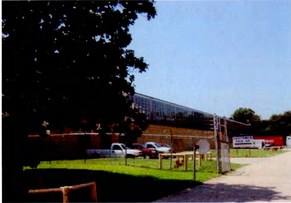
Plate 5. Ford Motor Company Automotive Parts Distribution Center, Warehouse Section, West Elevation, Looking Southeast.
