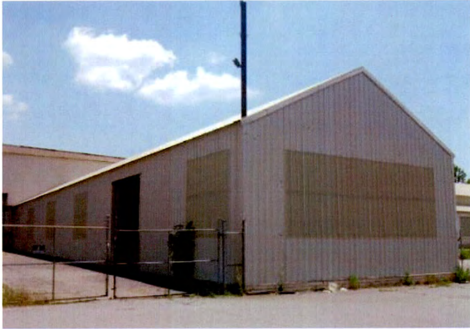
Plate 22. Southern Engineering Company, circa 1970 Fabrication Building, Looking East.
