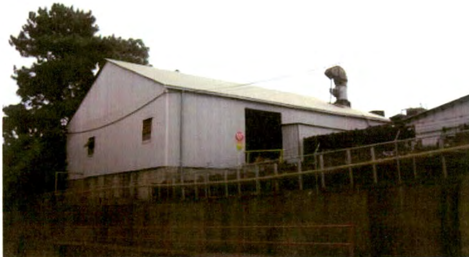
Plate 67. Charlotte Pipe and Foundry Company Complex, Light Manufacturing Facility With Modern Siding and Roofing, Looking East From South Clarkson Street.
