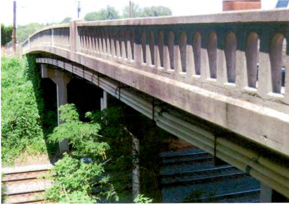
Remount Road Bridge (No. 11), Substructure and Balustrade, Looking North.
