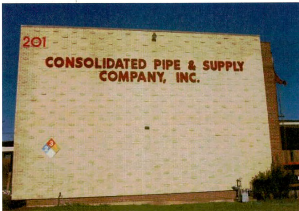
Plate 99. Standard Trucking Company Terminals, 1960 Terminal, South Wall, Looking North.
