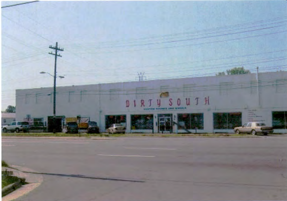
Commercial Building (No. 8), 2639 Wilkinson Boulevard, Looking South.
