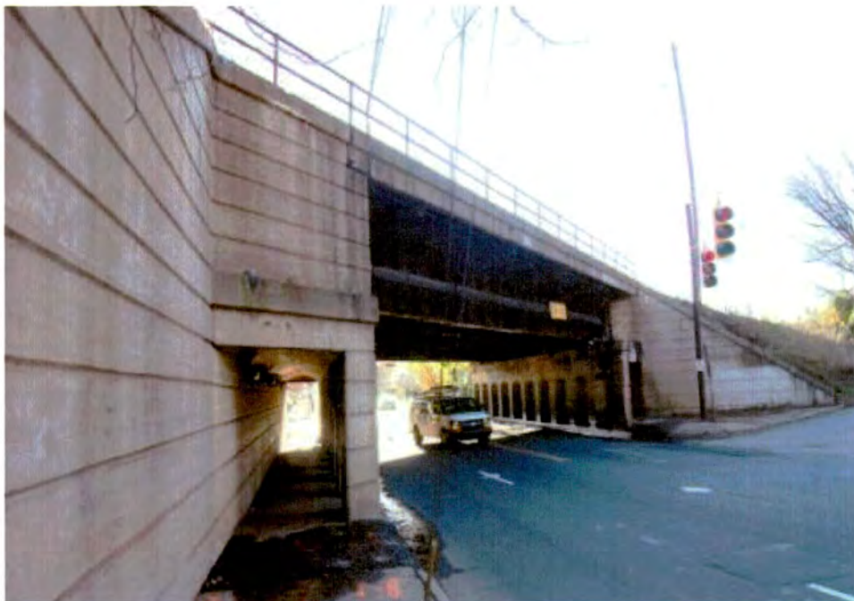
Plate 96. Southern Railway Bridge, North Tryon Street, Looking South.
