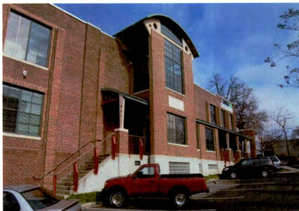
Plate 77. Electric Supply and Equipment Company Building, East Elevation, Looking North.
