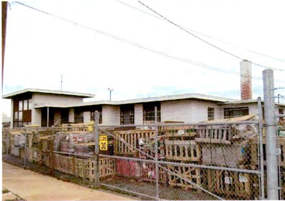
Office Building (No. 23), 520 West Summit Ave., Looking North.
