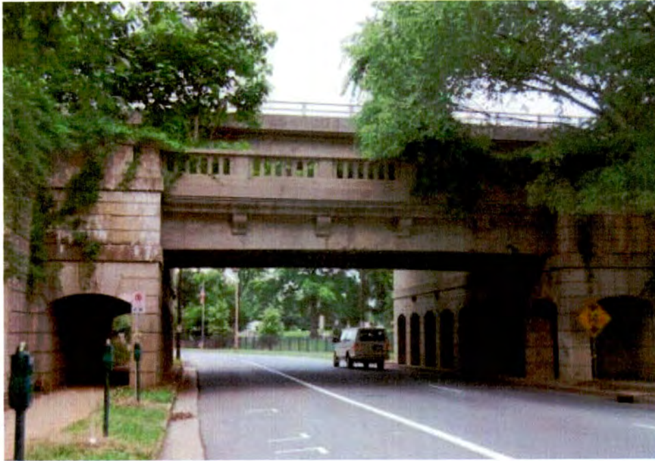
Plate 80. Southern Railway Bridge, Looking West Along West Sixth Street.
