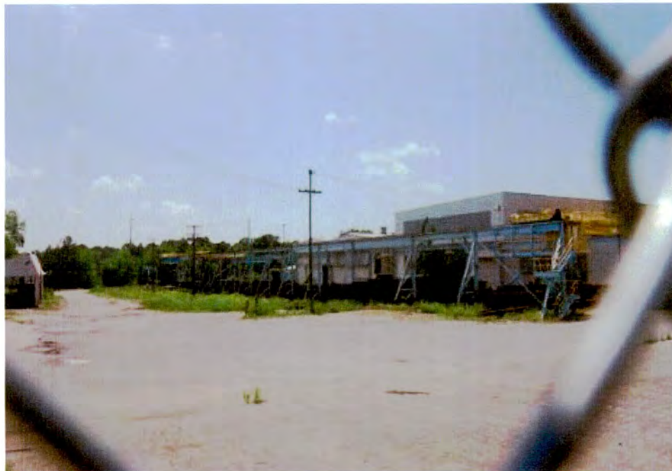
Plate 21. Southern Engineering Company, Travelling Crane, Looking South.
