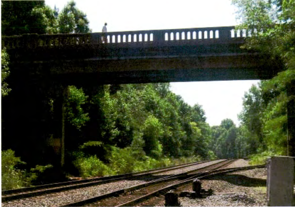
Morris Field Drive Bridge (No. 3), Substructure, Looking East
