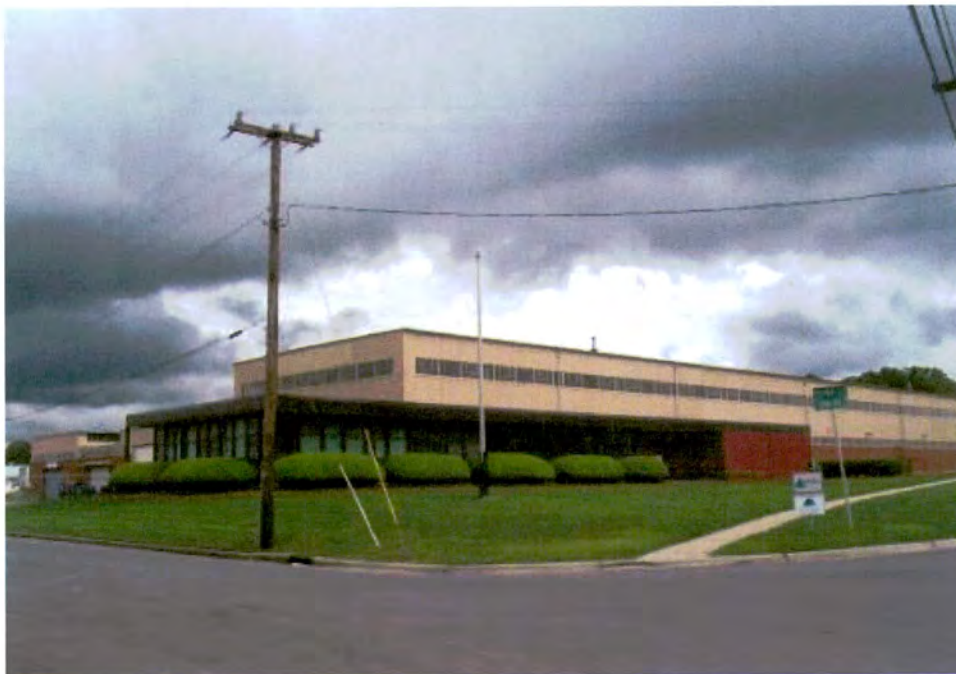
Plate 123. Republic Steel Corporation Plant, Office and Warehouse, Looking Southeast From Sugar Creek Road.
