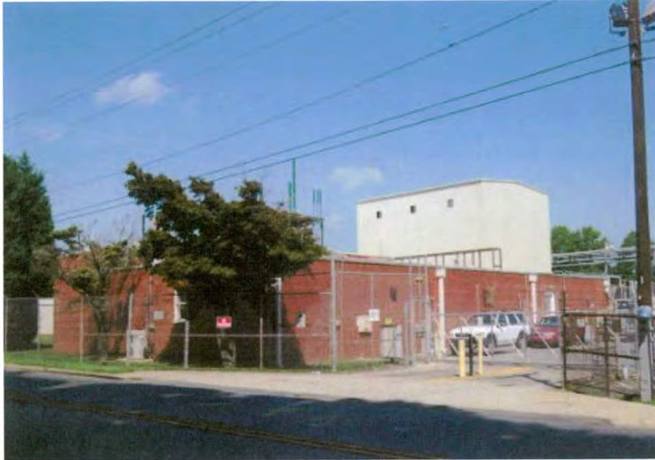
Plate 130. Wica Chemical Company Plant, 1956 Laboratory and Modern Metal Warehouse (to the Rear), Looking Northwest.
