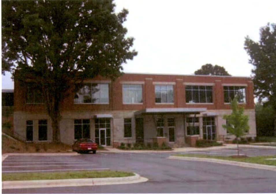
Plate 25. General Dye Stuffs Corporation Building, Rear Elevation Showing New Entrances, Looking North.
