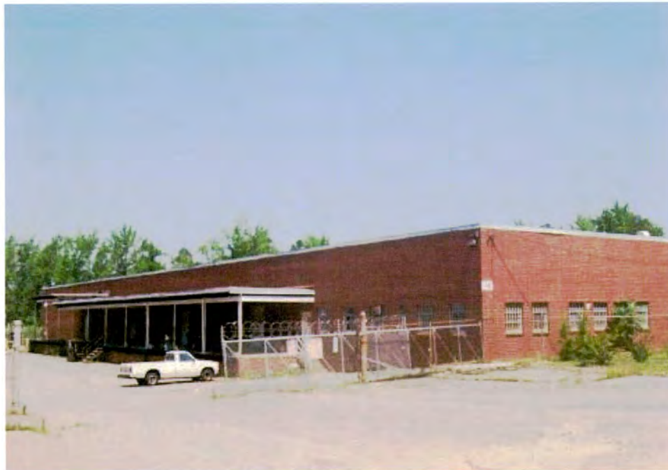
Warehouse (No. 5), 2246 Old Steele Creek Road, Looking West.
