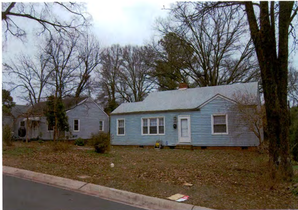
Plate 34. Westover Hills, 1333-1327 Skyview Road (Within APE), Looking Southeast.
