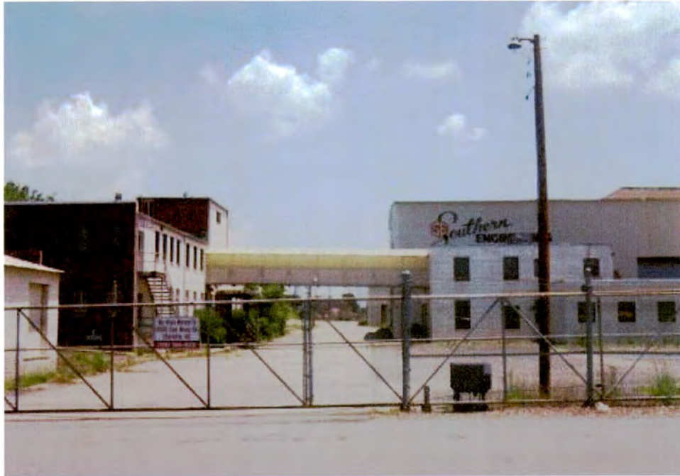
Plate 20. Southern Engineering Company, Office Buildings (on Left) and Fabrication Buildings and Warehouses, Looking East.
