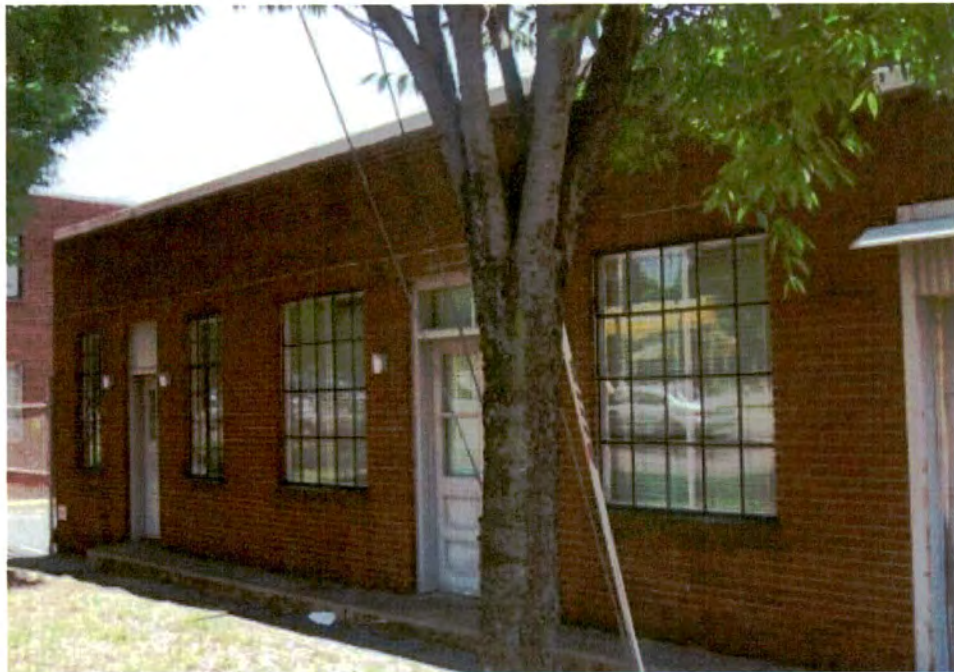
Plate 17. Southern Engineering Company, Office Building, Front Elevation, Looking Southeast.
