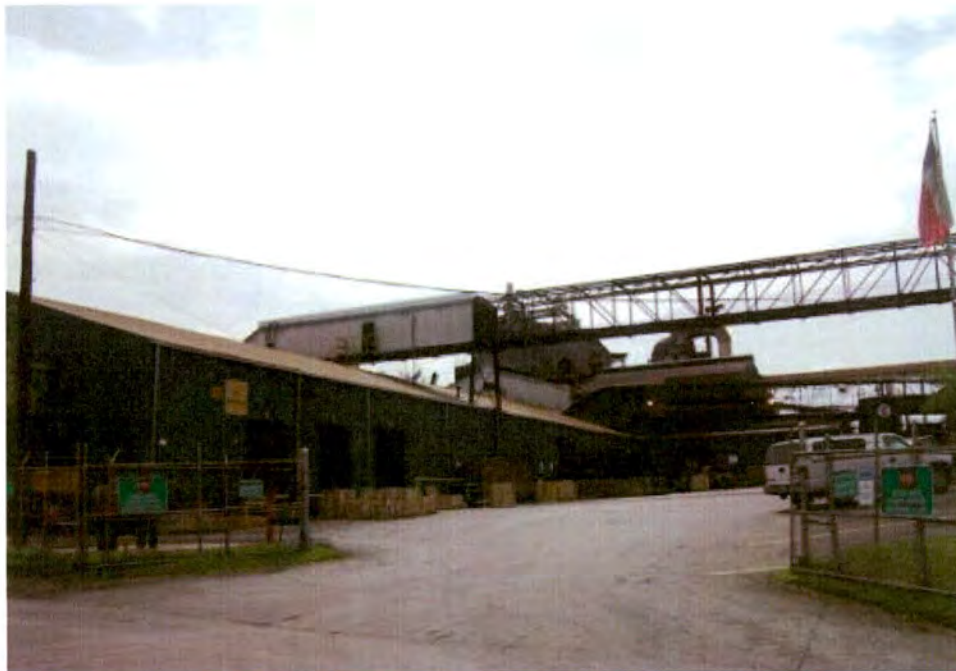
Plate 65. Charlotte Pipe and Foundry Company Complex, Main Gate on South Clarkson Street, Modern Warehouse and Elevated Walkway, Looking Southeast.
