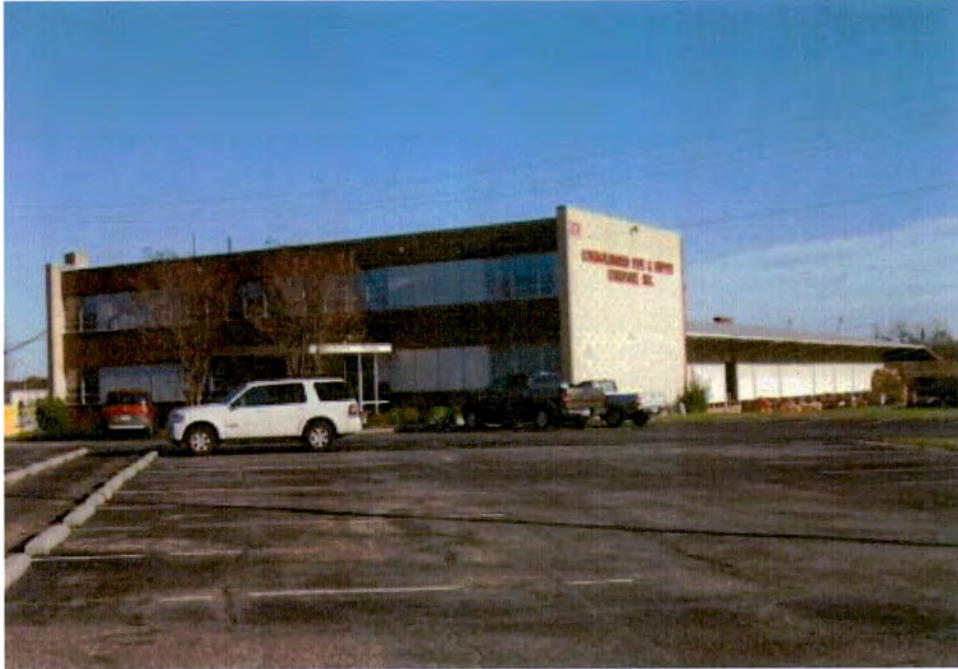
Plate 97. Standard Trucking Company Terminals, 1960 Terminal, Looking East.
