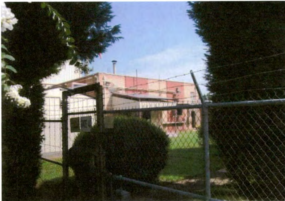
Plate 131. Wica Chemical Company Plant, 1966 Boiler Room, Looking North.
