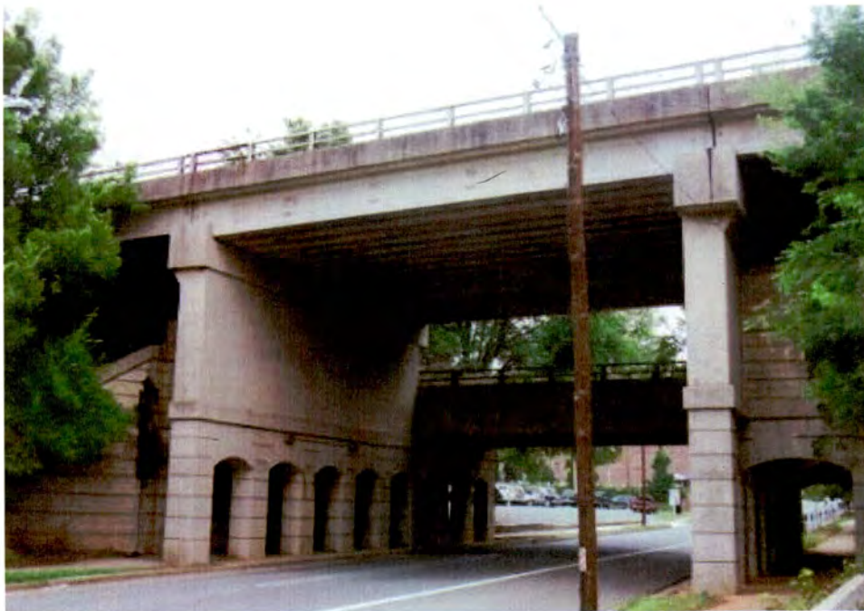
Plate 81. Southern Railway Bridge, Looking East Along West Sixth Street.
