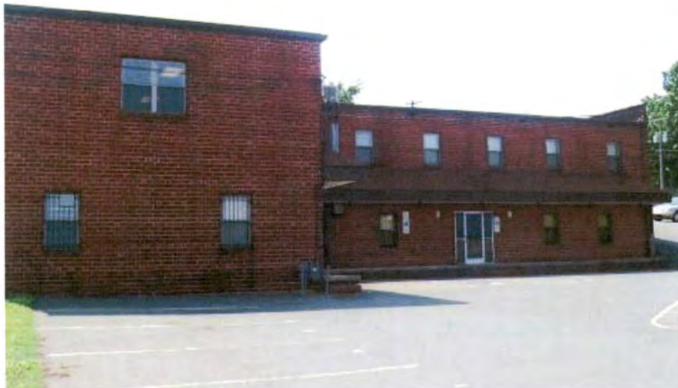
Office Building (No. 34), 1200 South Graham Street, Rear Elevation, Looking East.
