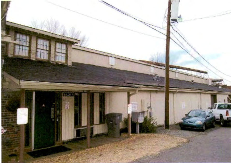
Charlotte Linen Supply Company (MK2210) (No. 26), 1420 South Mint Street, North Elevation, Looking West.
