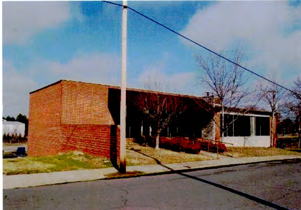
Office Building (No. 34), 1200 South Graham Street, Looking North.
