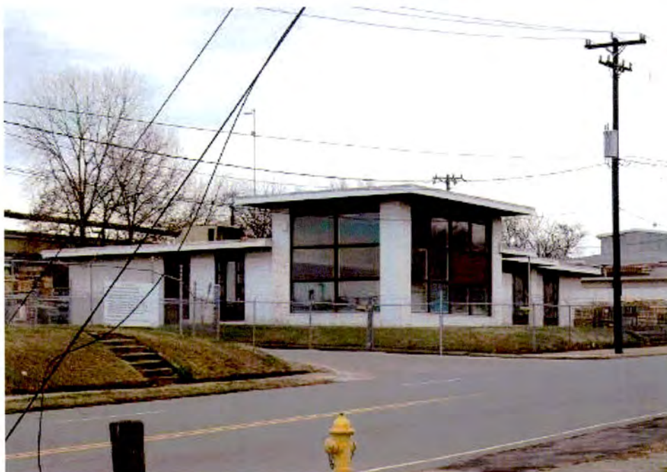
Office Building (No. 23), 520 West Summit Ave., Looking East.
