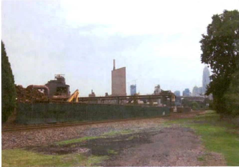
Plate 62. Charlotte Pipe and Foundry Company Complex, Overall View, Looking Northeast Along Railroad Line From Summit Avenue.
