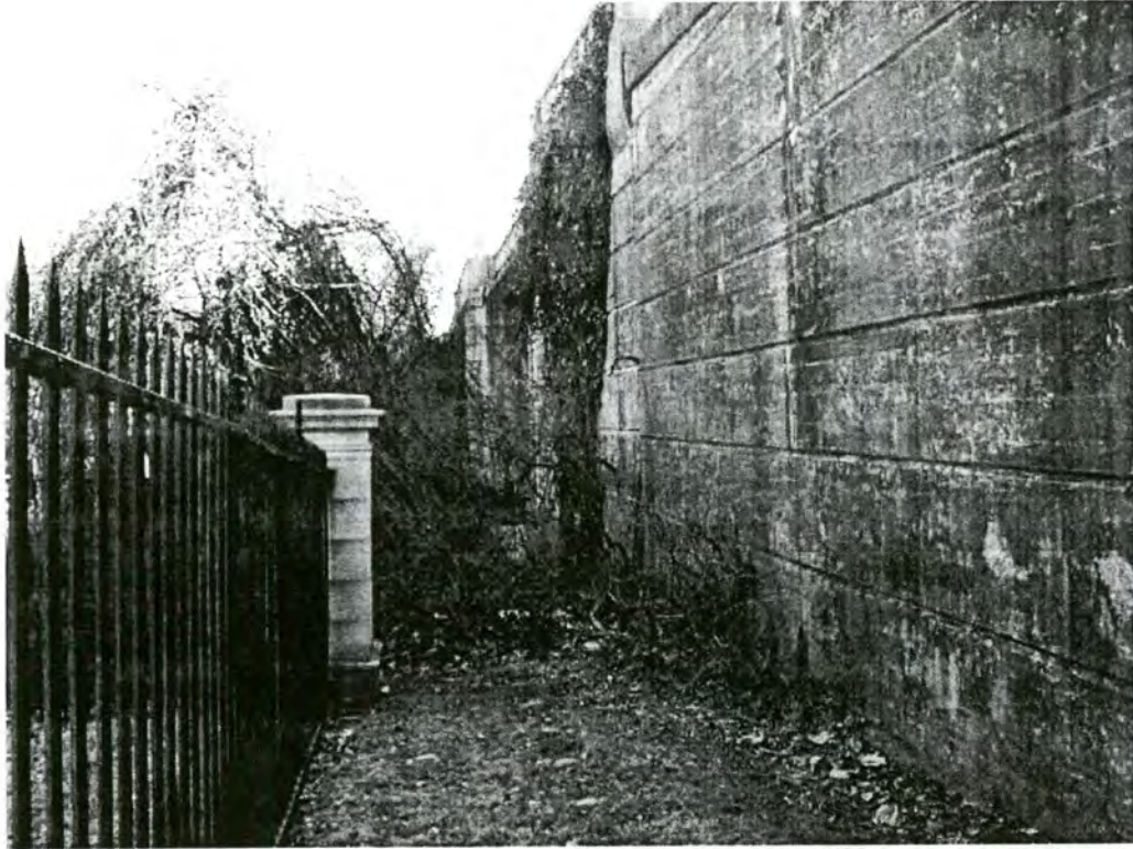
(FIG. 5) WHITE OAK CEMETERY FENCE AND PIER & 16 TH STREET BRIDGE
