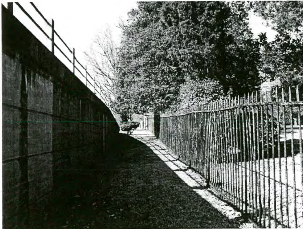
(FIG. 6) WHITE OAK CEMETERY FENCE AND PIER & 16 TH STREET BRIDGE
