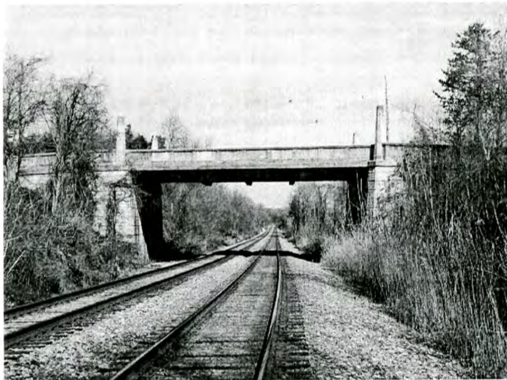
(FIG. 1) 16 TH STREET BRIDGE
