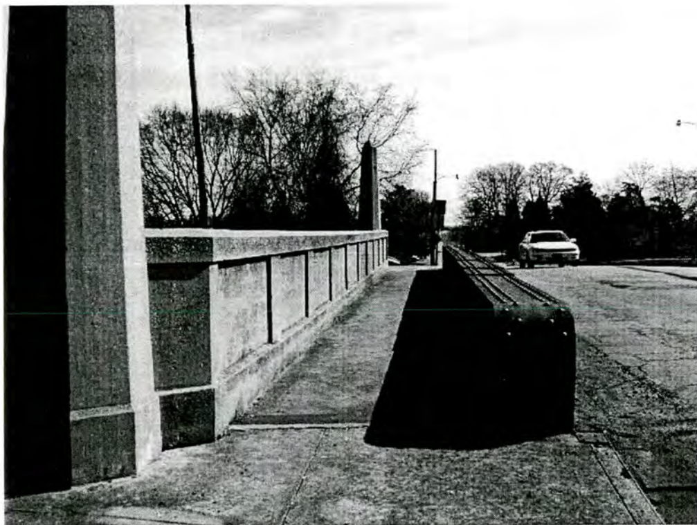
(FIG. 8) 16 TH STREET BRIDGE
