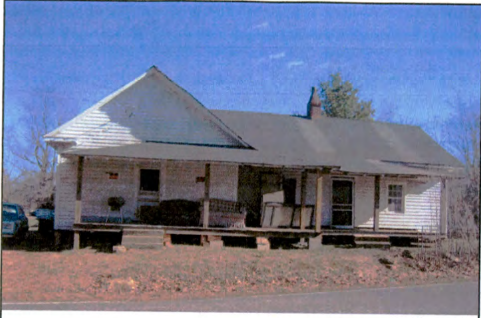
#56 House, ca. 1850; ca. 1900 R-4045 Cleveland County
