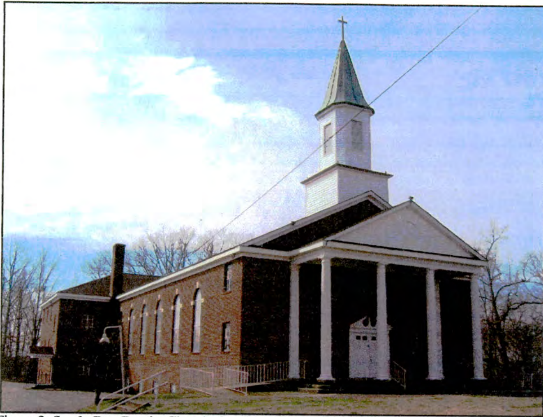
Figure 2: Sandy Run Baptist Church, façade (northeast elevation)
