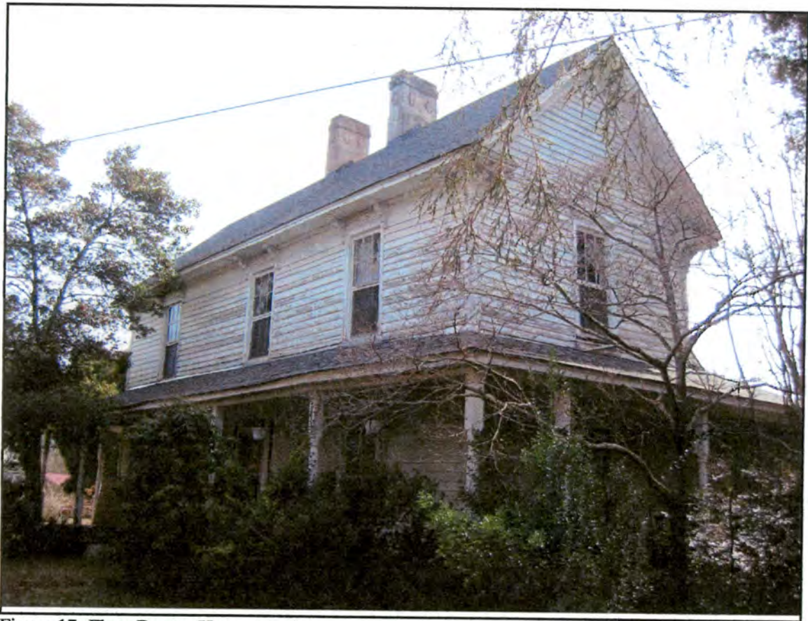
Figure 17: Flora Burrus House, northwest corner
