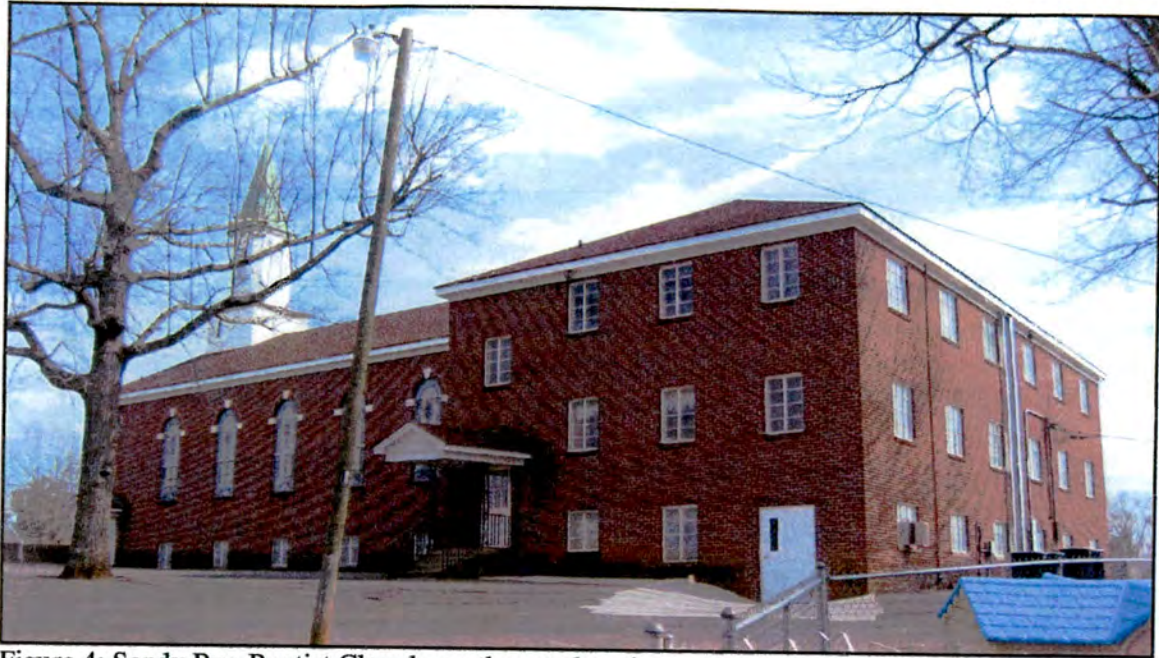
Figure 4: Sandy Run Baptist Church, northwest elevation
