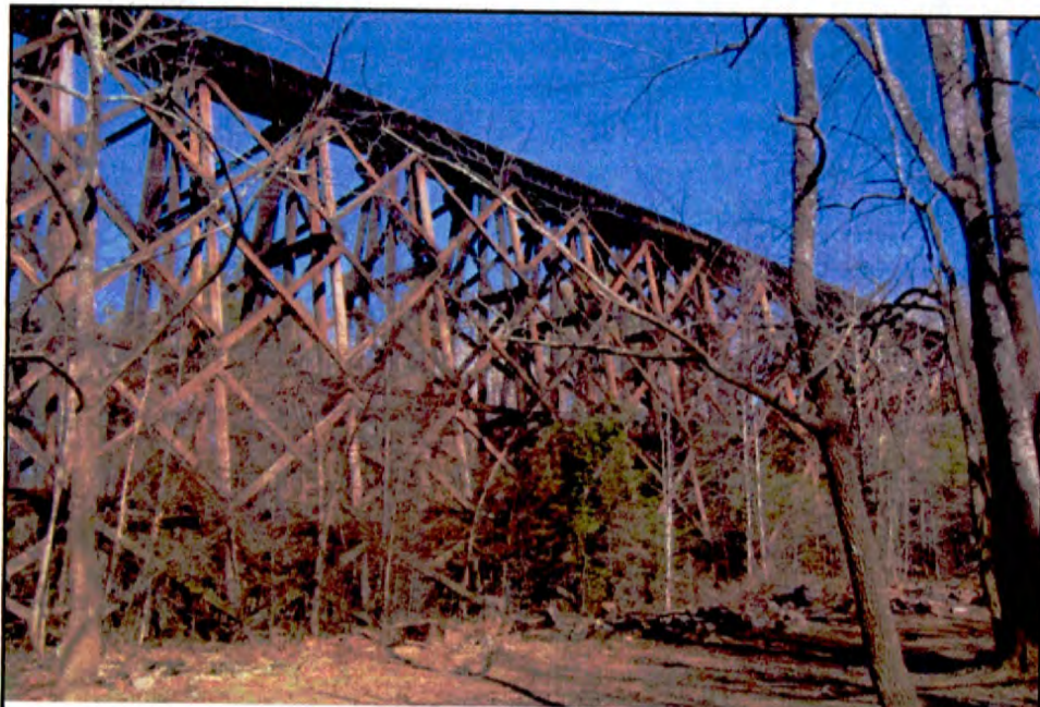
#66 Railroad Trestle, ca. 1960 R-4045 Cleveland County
