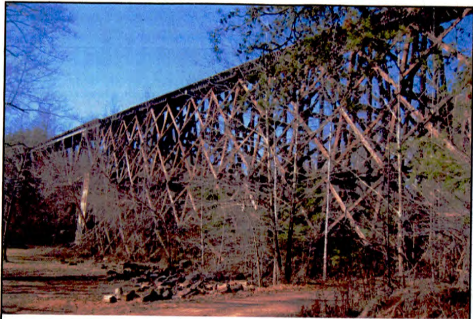
#66 Railroad Trestle, ca. 1960 R-4045 Cleveland County
