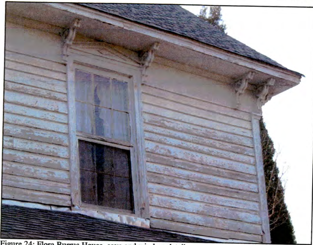
Figure 24: Flora Burrus House, eave and window detail
