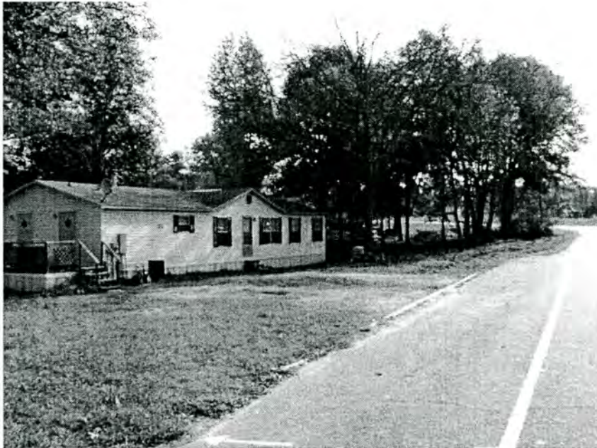
Church Street property located across the street from Property #39
