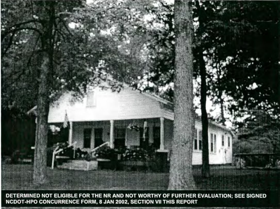
Property #45 - House, 106 Academy St. Lacks Historic or Architectural Significance
