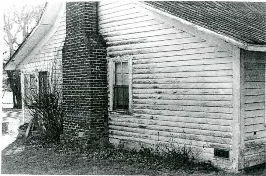
Plate 6. Blair House, East Elevation Looking Southwest.
