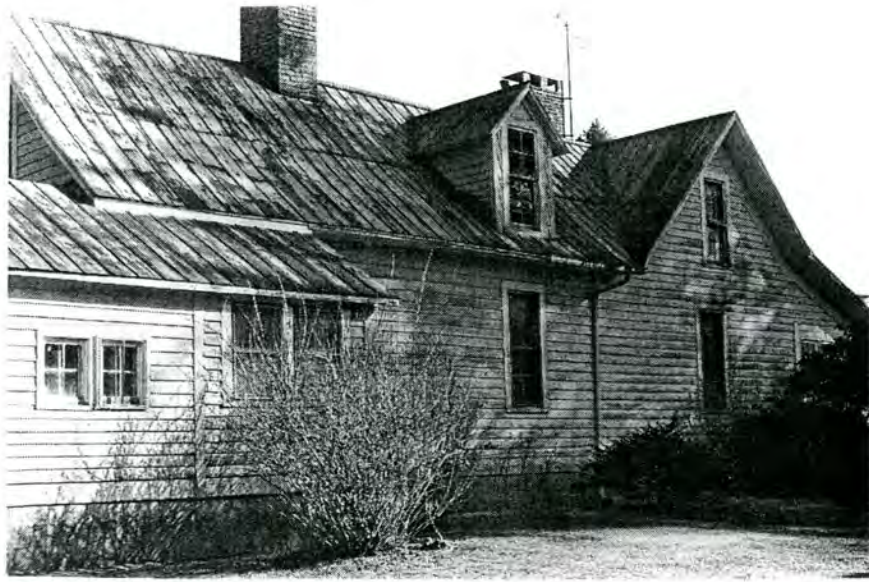
Plate 5. Blair House, West Elevation Rear Ell, Looking East.
