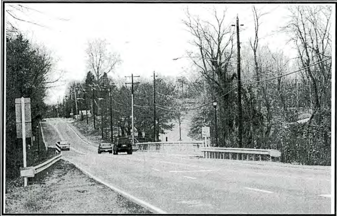
Figure 2- Bridge No. 20 over Deep River, Looking West
