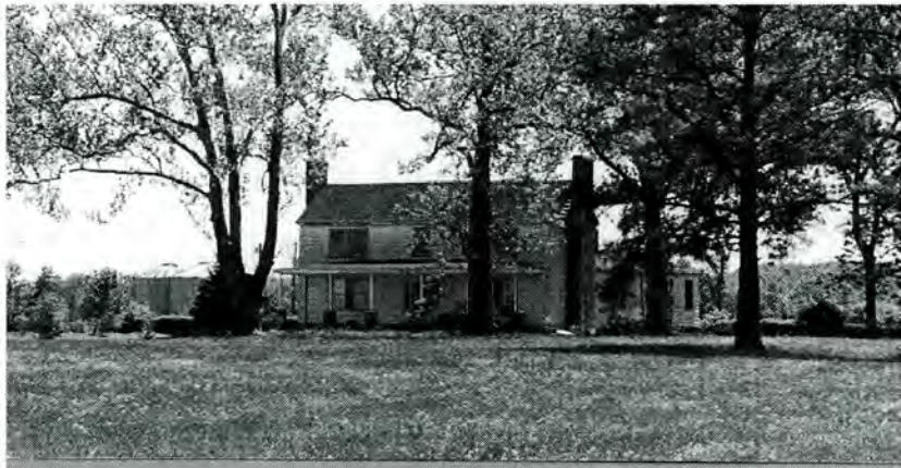
Figure 5. James Alfred White House (Property 1). In both form and placement the dwelling exemplifies typical design choices made by the more prosperous farmers in the Halifax County region during the late nineteenth century. Photographed April 26, 2001.
