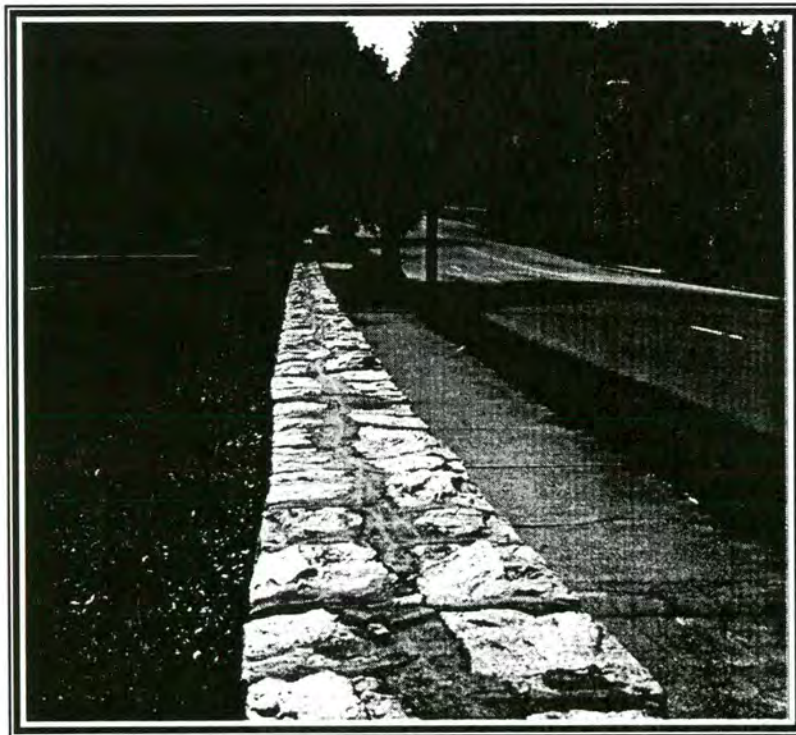
Figure 10 - View of stone wall forming one side of bridge railing
