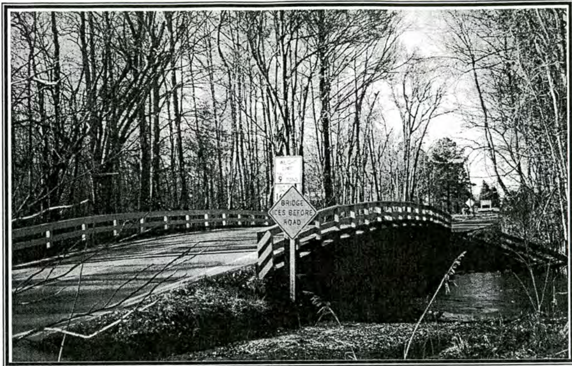
Figure 7 - Bridge No. 28 over Shingle Landing Creek- Looking Northwest
