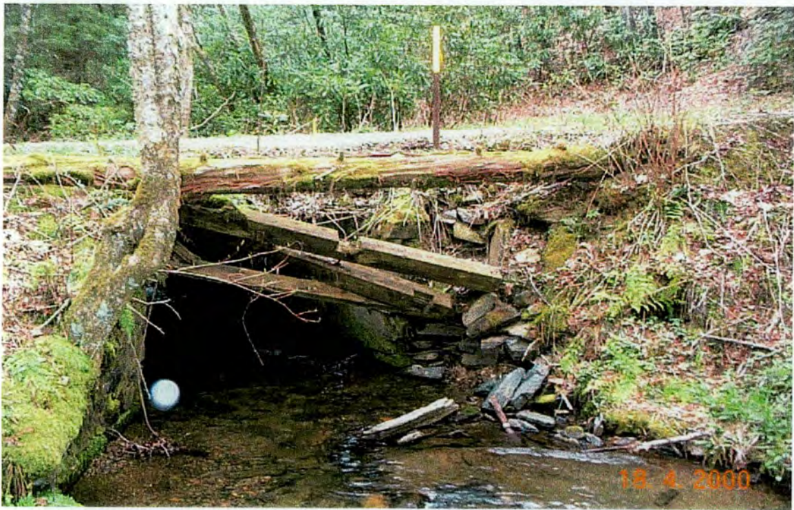
Plate 19: Downstream end of bridge and west wingwall.
