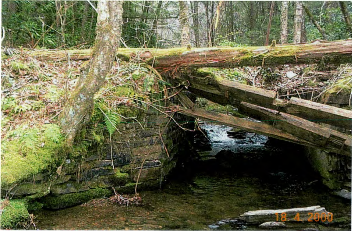
Plate 20: Downstream end of bridge, east wingwall.
