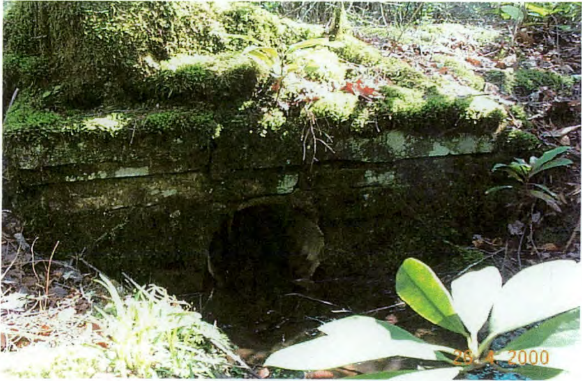
Plate 34: Straight walled style, large size. Located on creek before junction of roads #350/#350A, west side of road. Growth of tree separating stacked rock.
