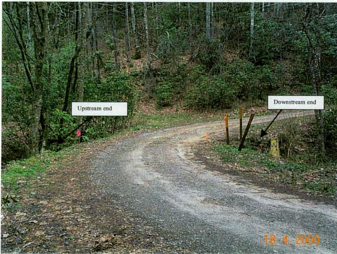
Plate 17: Location of stone bridge on Perry Gap section of road #350.
