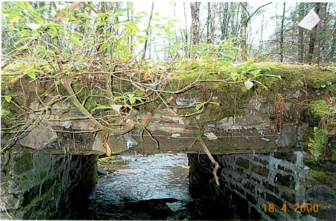
Plate 21: Upstream end of bridge, close up of concrete slab and fill.
