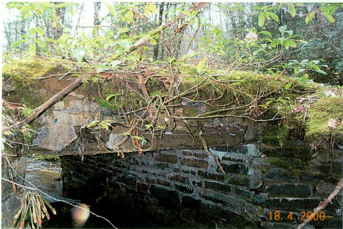
Plate 23: Upstream end of bridge, top and east side.
