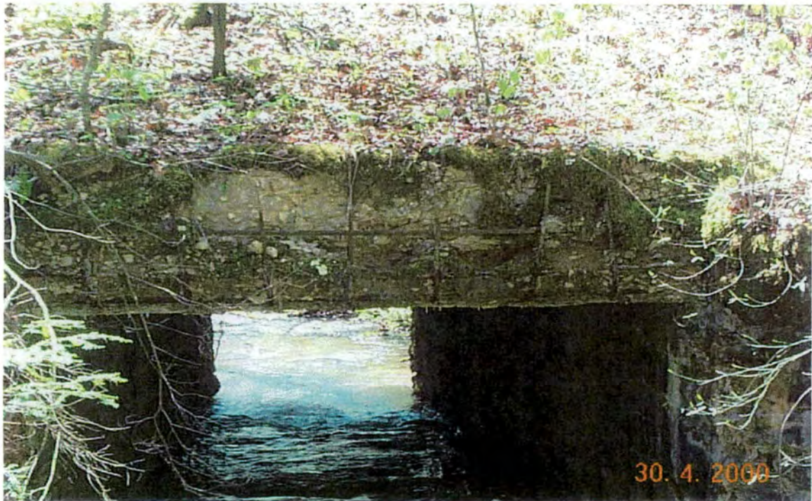
Plate 25: View of interior showing rock construction and poured concrete top.
