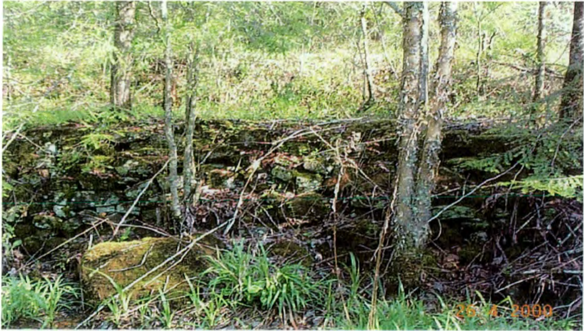
Plate 9: Midsection of retaining wall, close-up.
