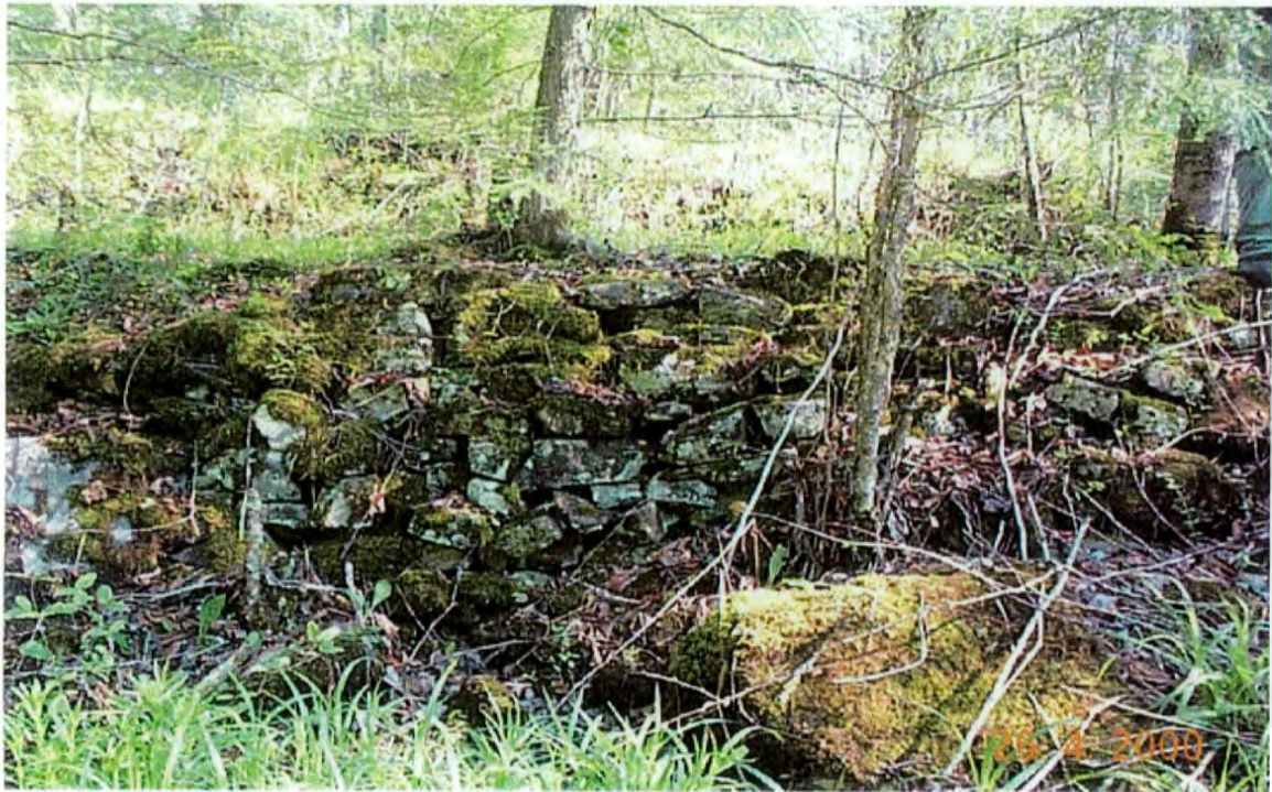
Plate 10: Northern end of retaining wall, close-up.
