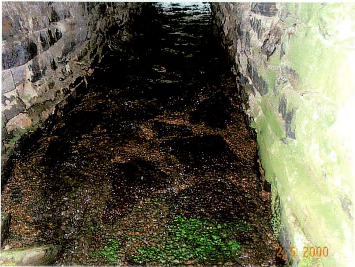
Plate 12: Floor and side walls of box culvert, from upstream (north) side.
