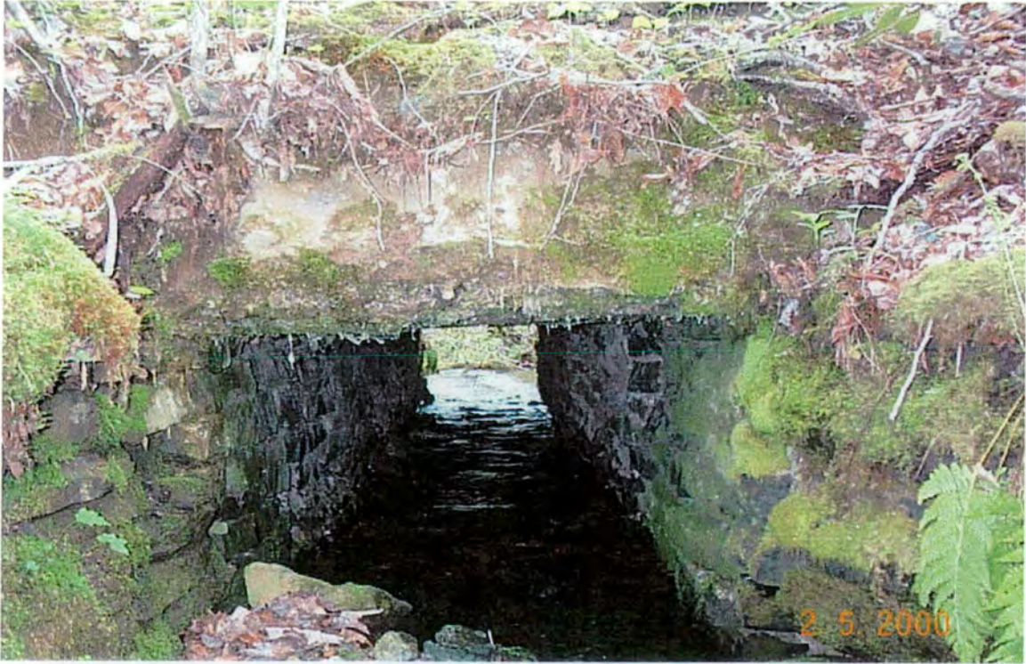
Plate 15: Close-up of downstream end of box culvert
