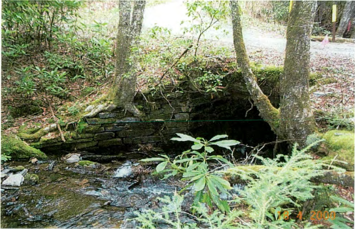
Plate 22: Upstream end of bridge, west wingwall.
