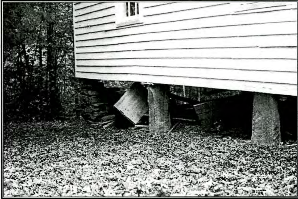
Photograph 3: Golden Valley Church, detail of stone piers, looking southwest
