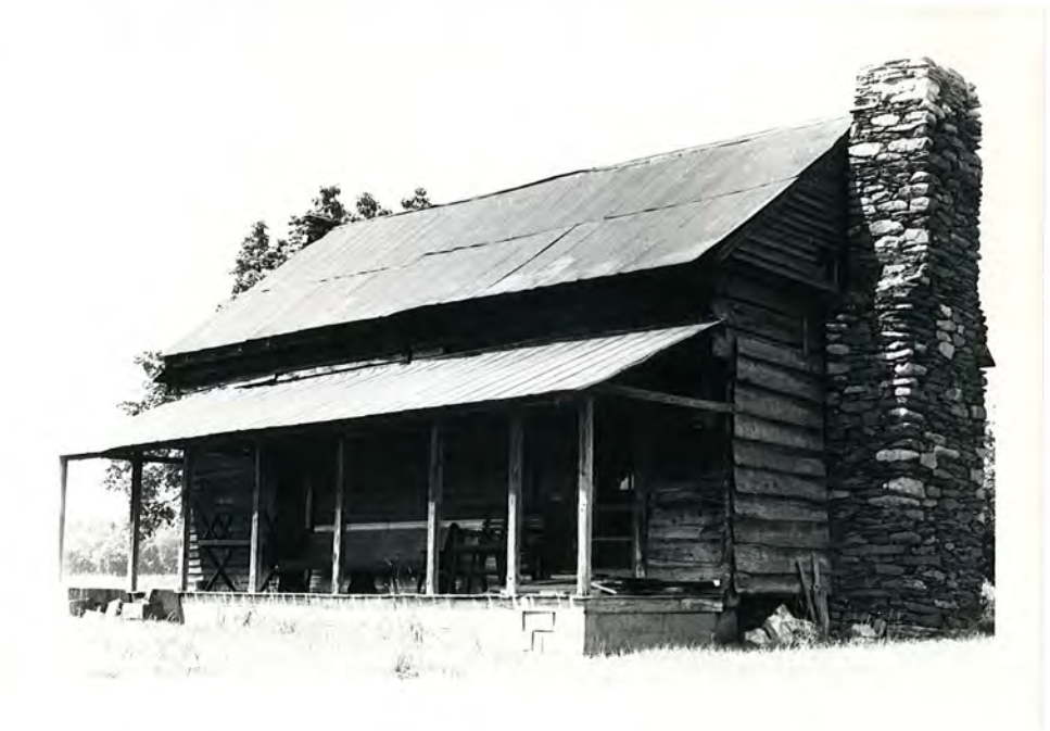
Plate 4. Hodges House, Front and West Elevations, Looking Southeast.
