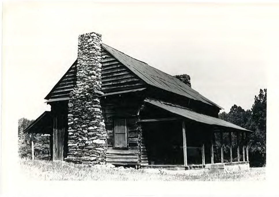
Plate 3. Hodges House, Front and East Elevations, Looking West.
