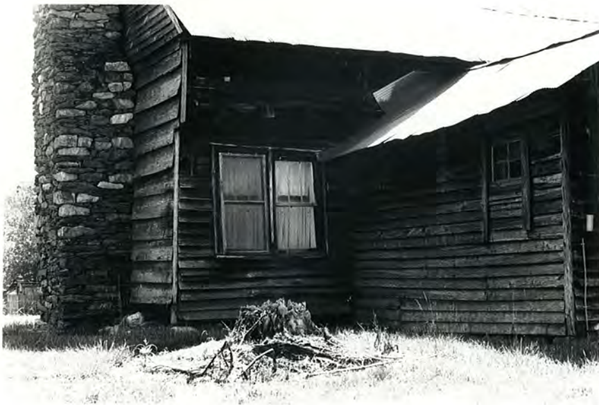
Plate 5. Hodges House, East Elevation, Looking West.
