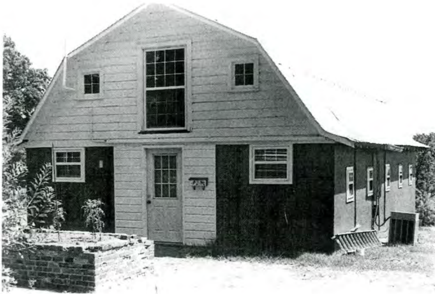
Plate 39. Barn (No. 7), Gable End Entrance and Side (Southeast) Elevation, Looking Northwest.
