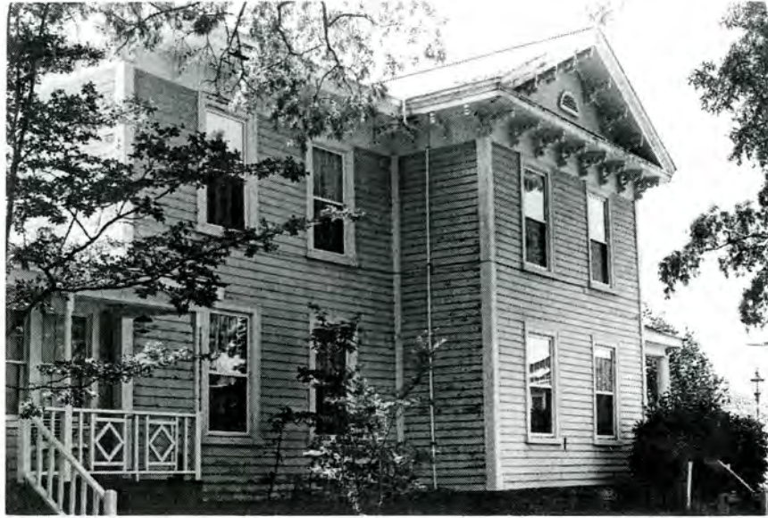
Plate 17. T.S. Eanes House (No. 2), Side (Northwest) Elevation and Rear Ell, Looking Southwest.
