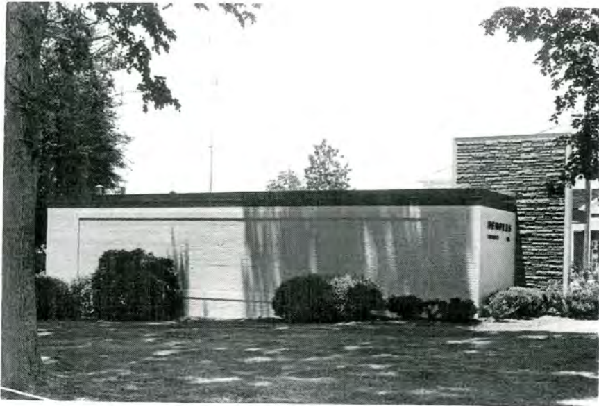
Plate 43. Peoples Finance Company Building (No. 9), Side (Southeast) Elevation, Looking Northwest.
