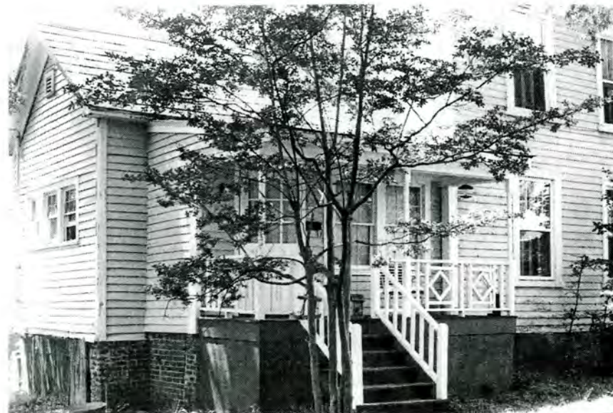
Plate 18. T.S. Eanes House (No. 2), Twentieth Century Rear Ell and Rebuilt Porch, Looking Southwest.
