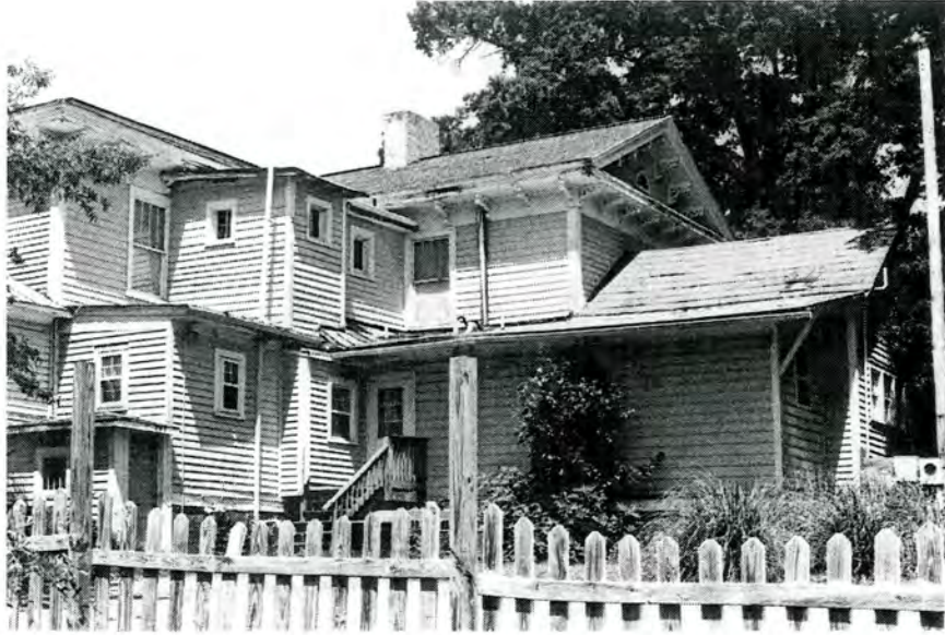
Plate 19. T.S. Eanes House (No. 2), Rear Elevation and Real Ells, Showing Twentieth Century Additions, Looking Northwest.
