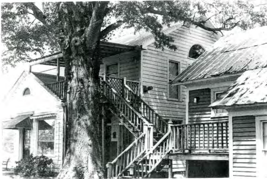
Plate 26. Office (No. 3), Side (Southeast) and Rear Elevations (Fredonia School on Right), Looking West.
