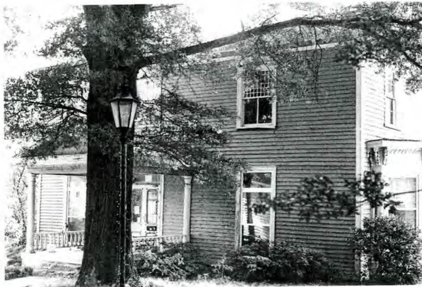
Plate 31. Hargrave-Craven House (No. 6), Facade, Showing Late Nineteenth Century Bay Window and Modern Replacement Window, Looking Southeast.
