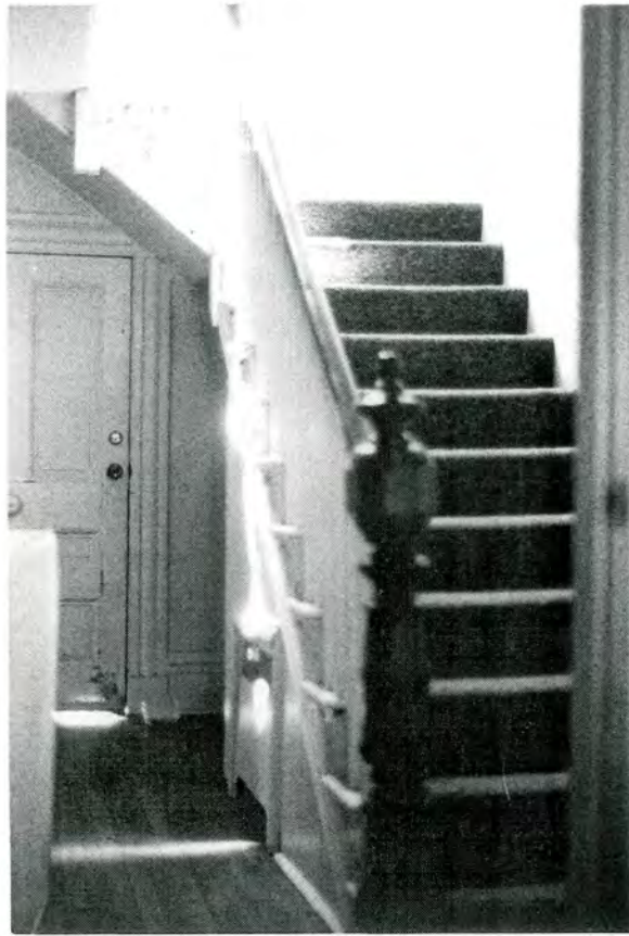
Plate 34. Hargrave-Craven House (No. 6), Interior, Hall, Staircase, and Rear Door.
