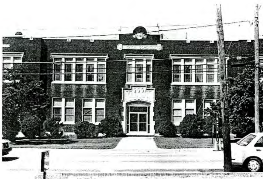
Plate 4. Cecil School (No. 1), Facade, Looking Southwest.
