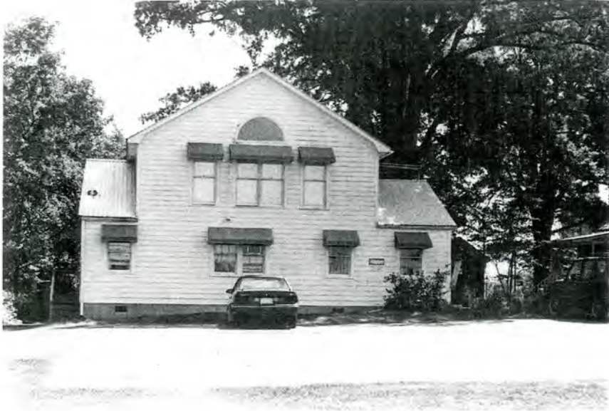
Plate 25. Office (No. 3), Facade (Northwest) Elevation, Looking Southeast Across Parking Lot.
