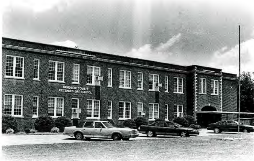
Plate 13. Holly Grove School, Facade, Looking Northwest.
