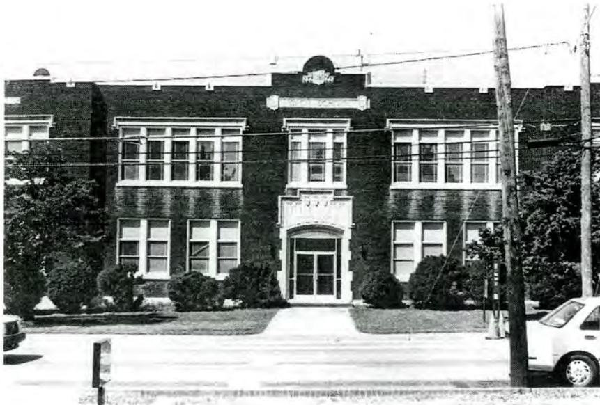
Plate 4. Cecil School (No. 1), Facade, Looking Southwest.
