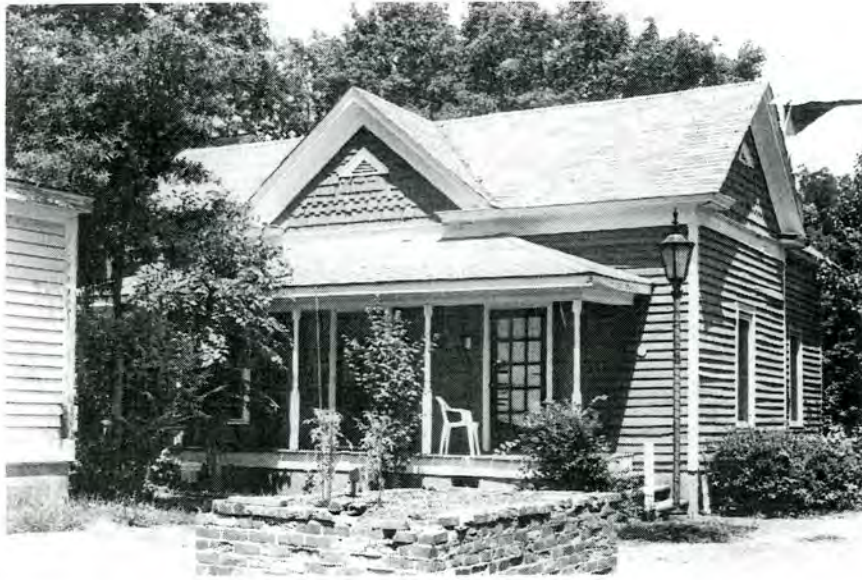
Plate 29. Mill House (No. 5), Facade and Side (East) Elevation, Looking Northwest.
