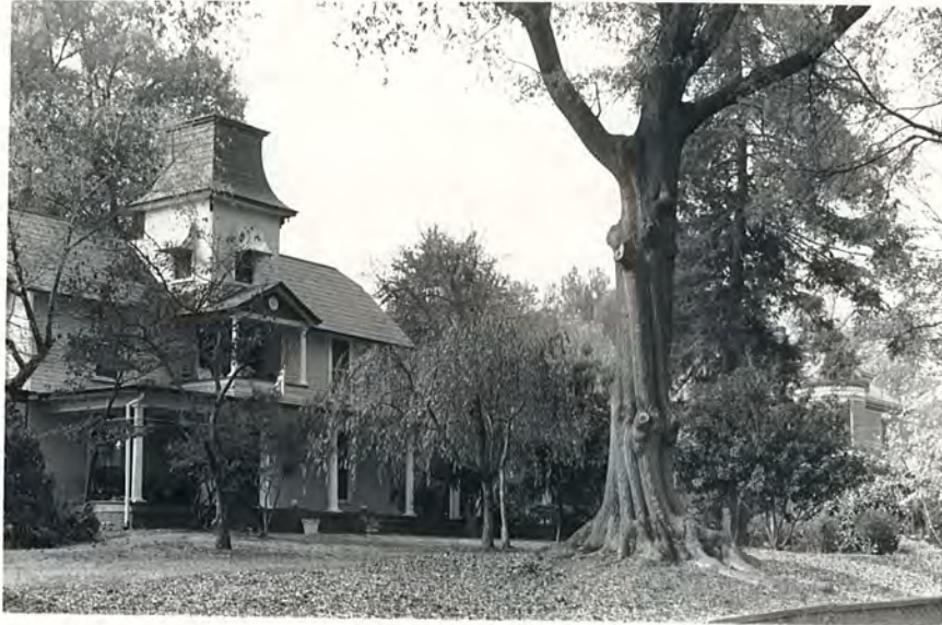
Plate 6. Academy Hill Historic District, West Side of Mulberry Street, Looking North.
