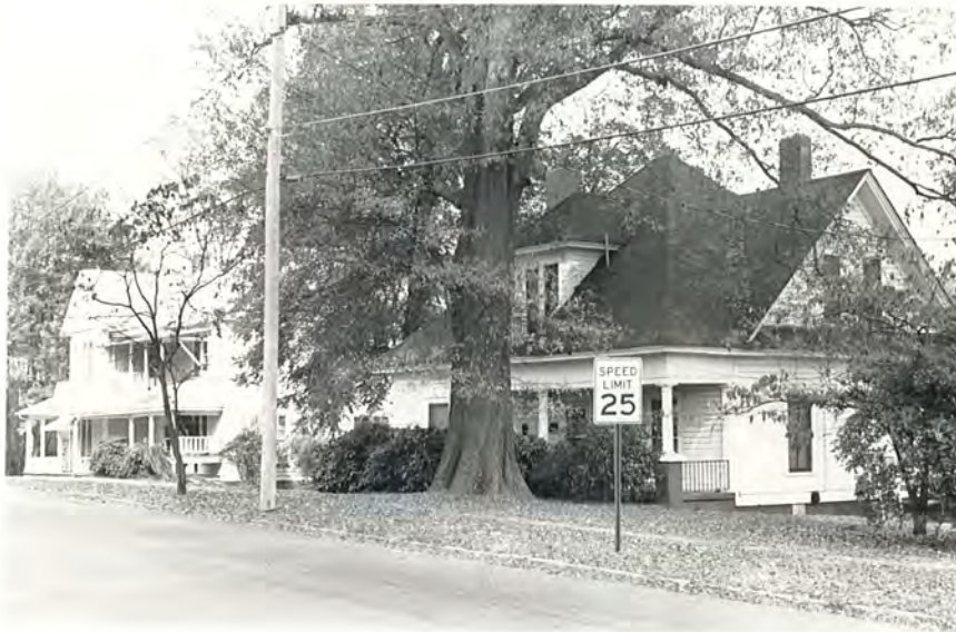
Plate 5. Academy Hill Historic District, East Side of Mulberry Street, Looking North.
