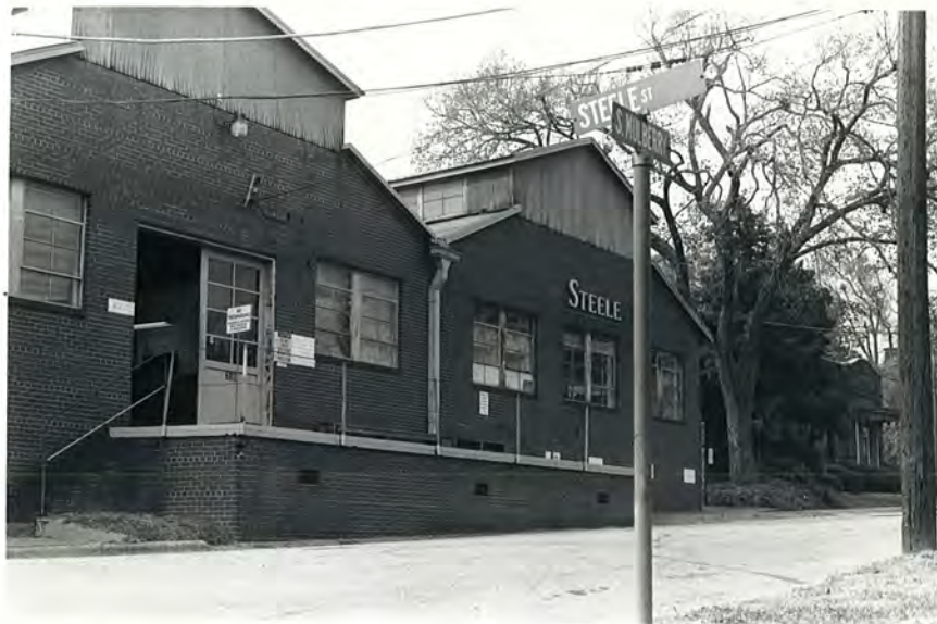
Plate 7. Academy Hill Historic District, J. C. Steele and Sons Brick Machinery Plant, Looking Northwest.
