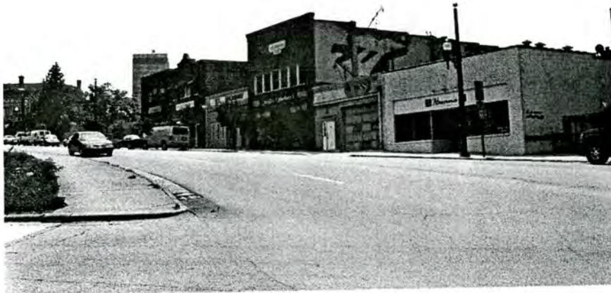
Plate 6. Downtown Asheville Historic District, 107-109 Broadway (South of I-240), Looking South.
