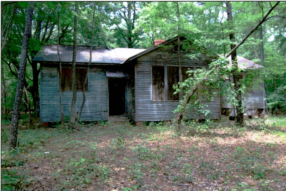
Figure 4. Ivey School: east-facing front elevation; note projecting industrial room with louvered ventilator and boarded-over windows, vestibule entries with canted hoods, and cloakroom windows extended up to eaves
