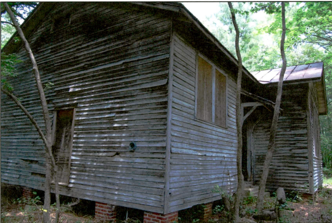
Figure 7. Ivey School: south side and east front elevations; note off-center door at side elevation and entryway with triangular knee-brace-supported hood at front
