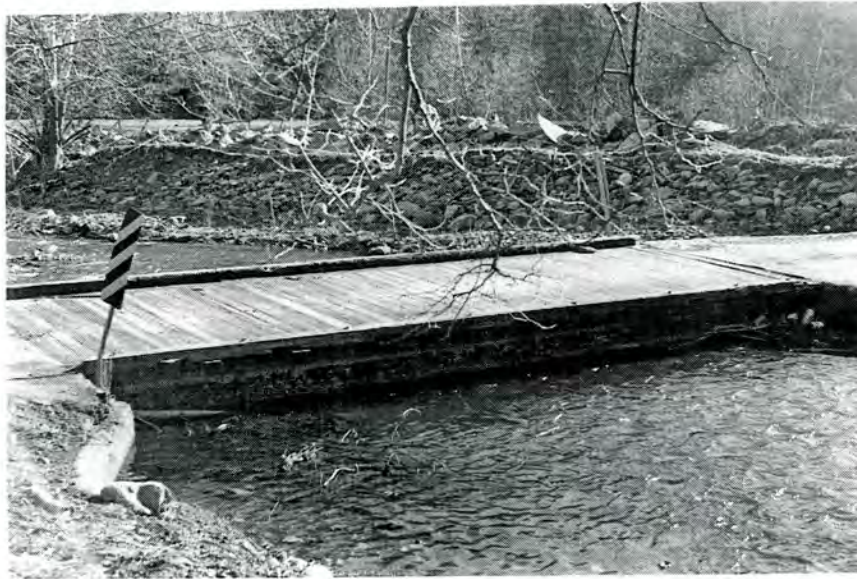
Plate 1. Bridge No. 281, Looking East.
