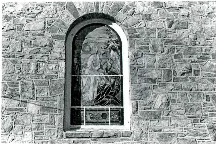
Plate 5. Foster Memorial Presbyterian Church, Detail of Rear Stained Glass Window and Masonry Construction.
